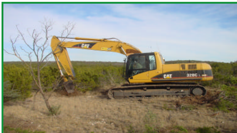
An Excavator is being used for Brush Management
