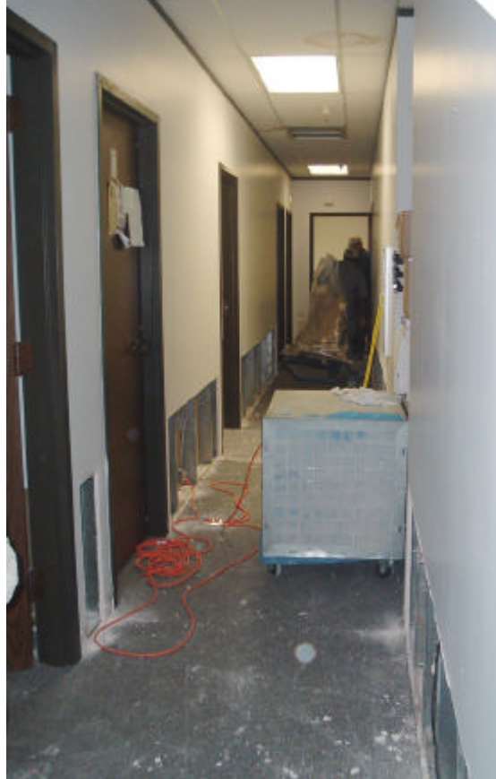
Extensive construction work took three weeks to complete. Photo by TxRC
