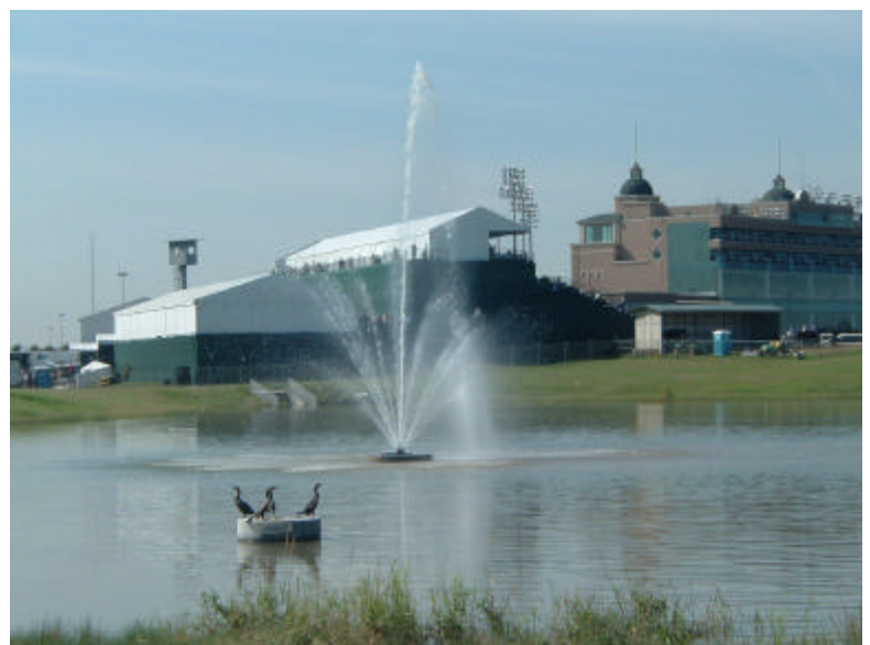
A view from the backside area of some of the newly constructed trackside seating. Photo by TxRC
