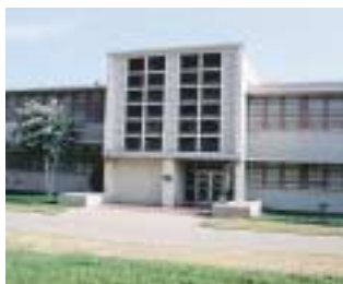
Bowden Building at St. Philip's College, San Antonio
