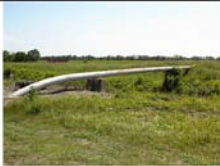
16. 12" HDPE pipeline going over Ditch C-1 between Alvin and Marvel
