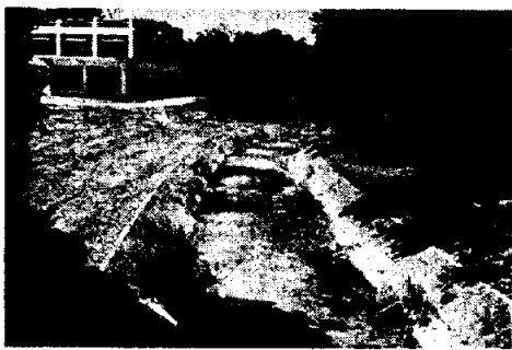
1930s WPA Program Channel Lining Upstream of Broadway
