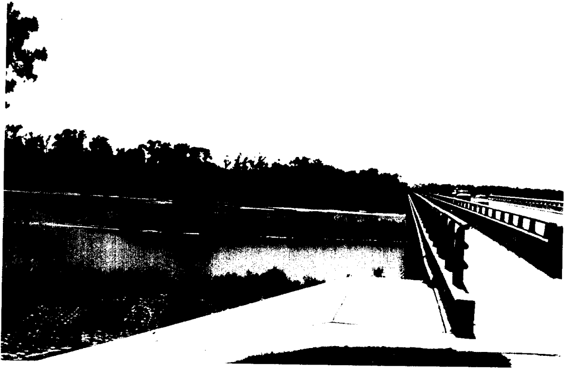
1-15 Island of sediment in channel at north Lake Houston Parkway bridge. View is downstream from north end of bridge.
