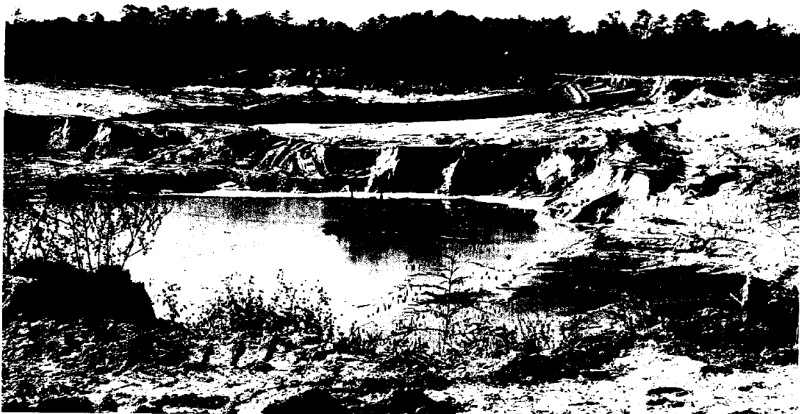
3-6 DDS sand pit active (west) pit. View is from east looking west.
