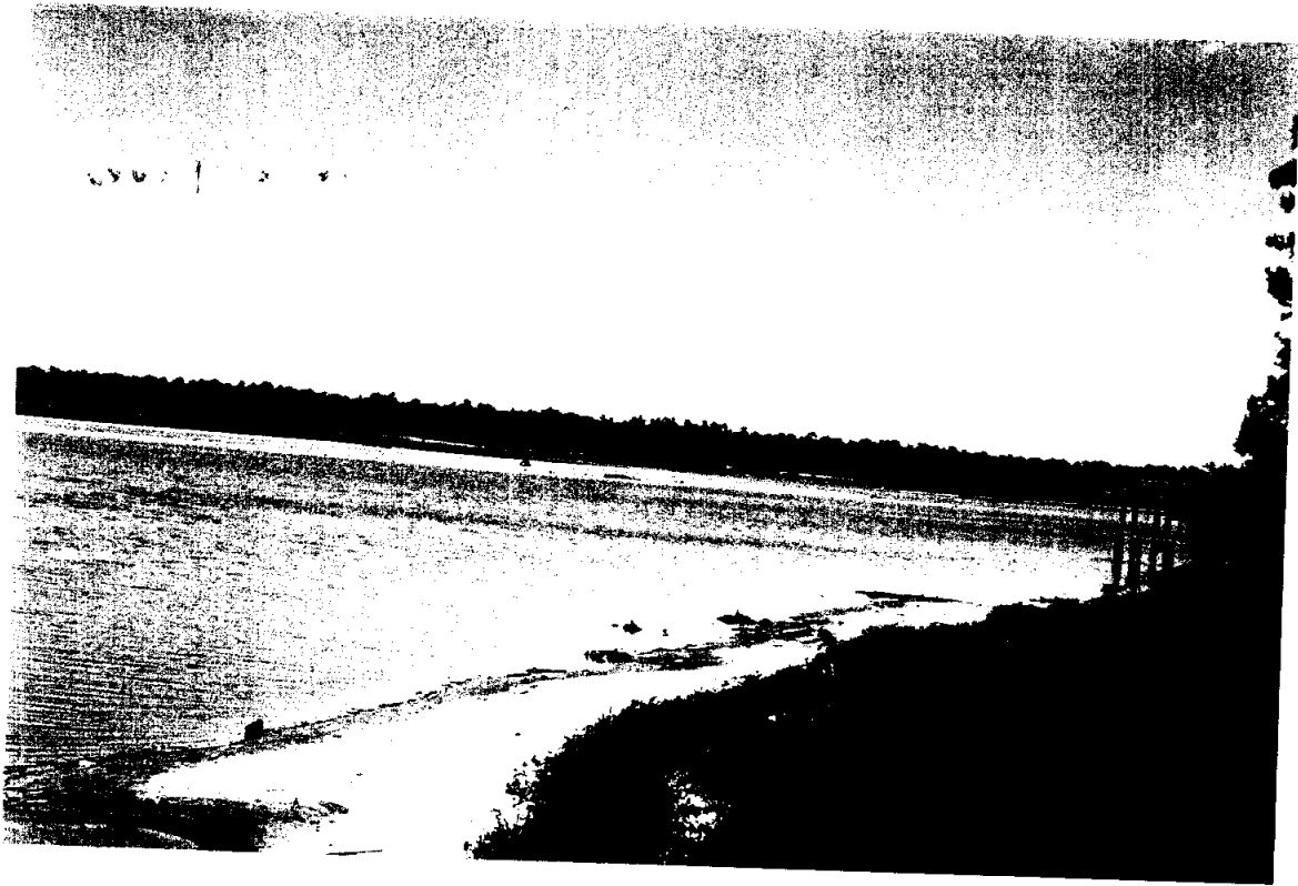
1-5 Photo from northeast side of large point upstream of north Lake Houston Parkway. Photo is looking downstream. South of channel. (Key Map 337-M)
