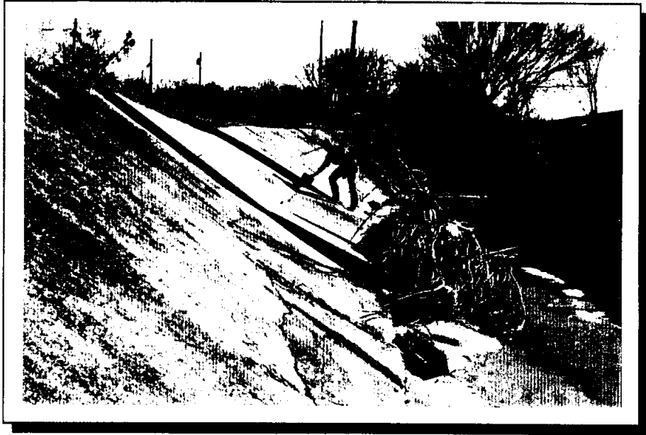
Figure III-4a - Sideslope Failure (Heaving and Sliding)
