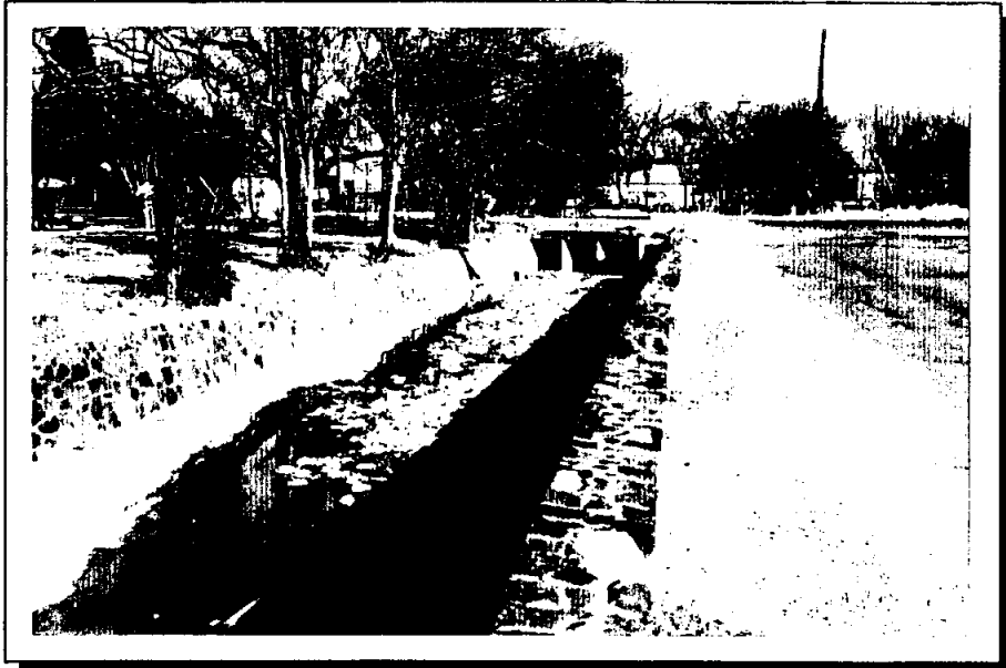
Figure III-9a - Upper PEC-4 Upstream of Wainwright Street
