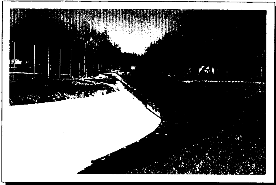
Figure III-11a - Typical Concrete Section in Lower PEC-4 Channel
