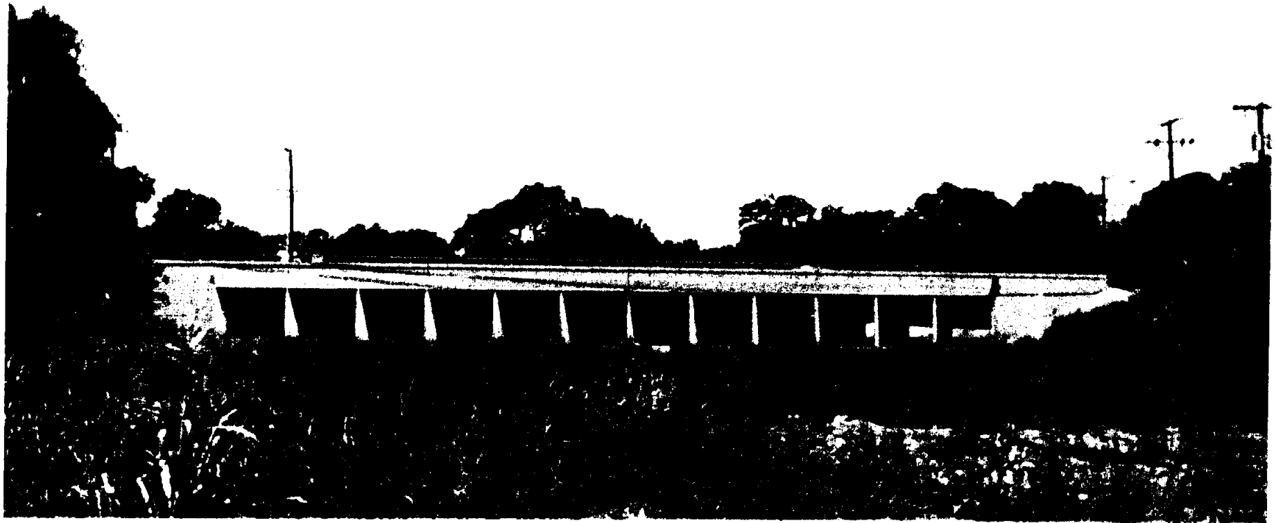
East Olmos Creek Downstream of Wurzbach Road 12-10'x10' Box Culverts Looking Upstream
