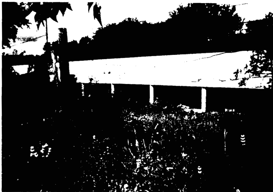
SITE 30 Leslie Road at French Creek Downstream
