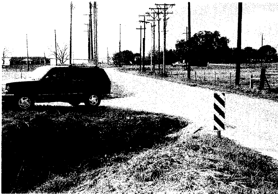
PHOTO 28 - LYTLE CANAL AT OLD FRIO ROAD
