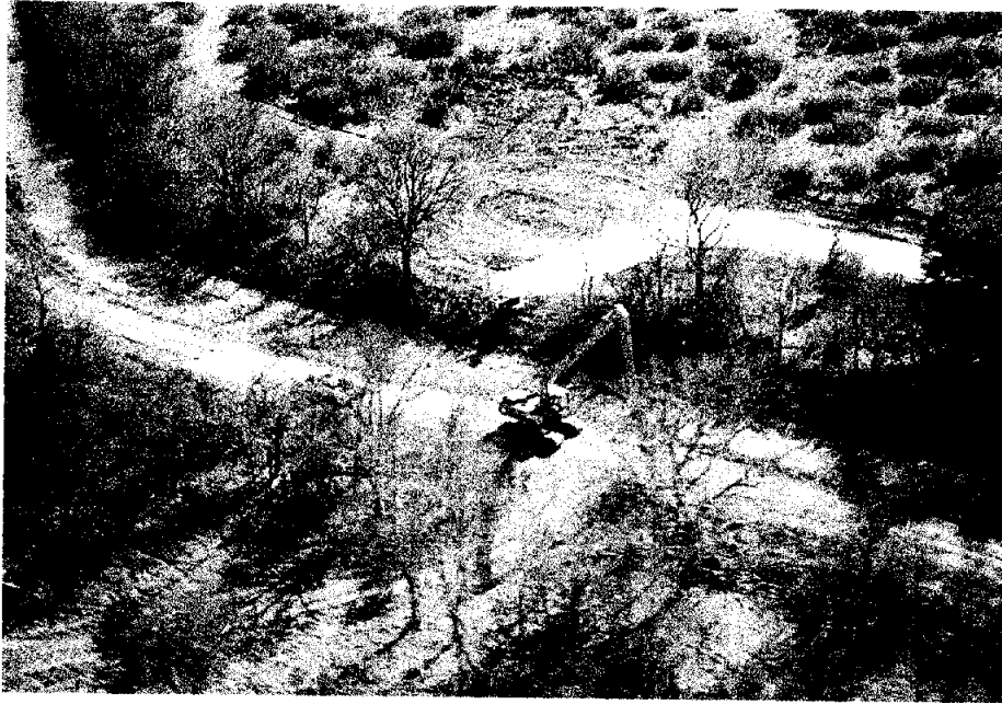
PHOTO 15 - EXCAVATOR CLEANING MAIN CANAL (Note Excessive Vegetation on Far Canal Bank)
