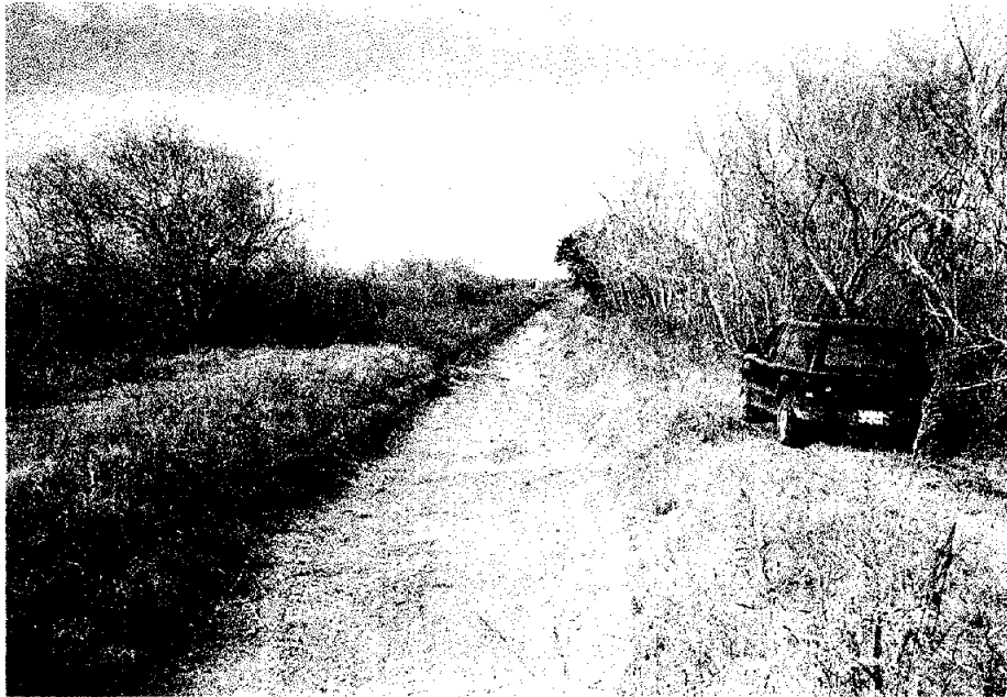
PHOTO 2 - TYPE B CANAL (Upper Portion of D - 1)
