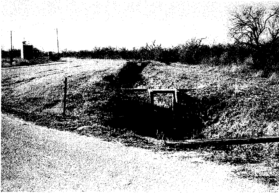
PHOTO 27 - CANAL B-1-K AT TOUCHSTONE ROAD
