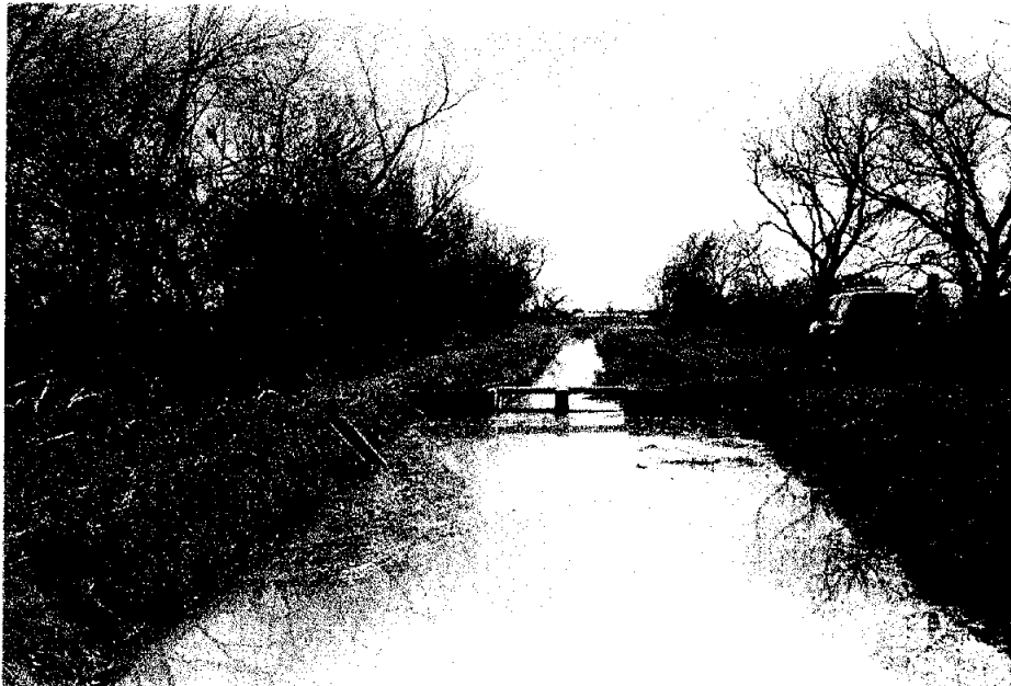
PHOTO 4 - TYPE D CANAL (Beyond Check, Natalia Canal)
