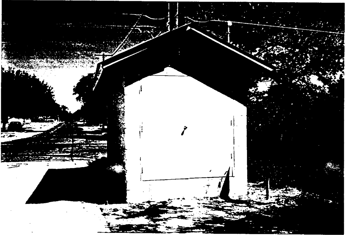
PIERCE AND HOLMIG STREETS SEWAGE LIFT STATION
