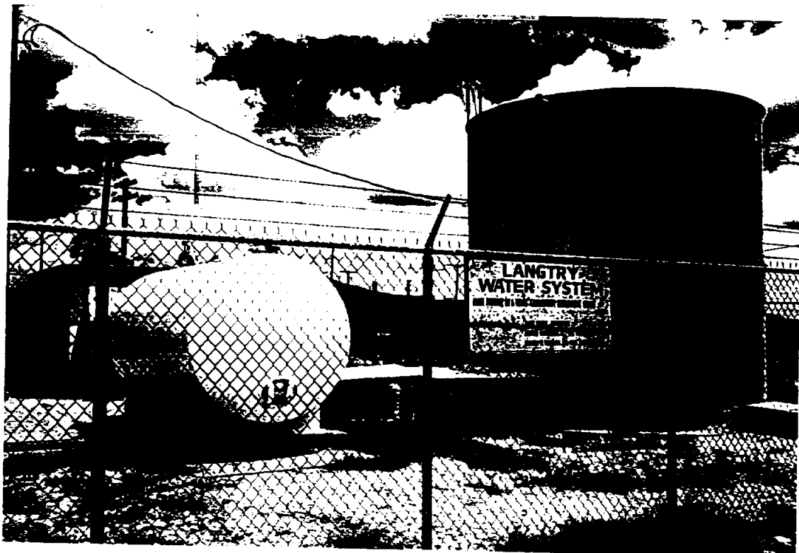
27,500 - GALLON GROUND STORAGE TANK (RIGHT) 2,500 - GALLON PRESSURE TANK
