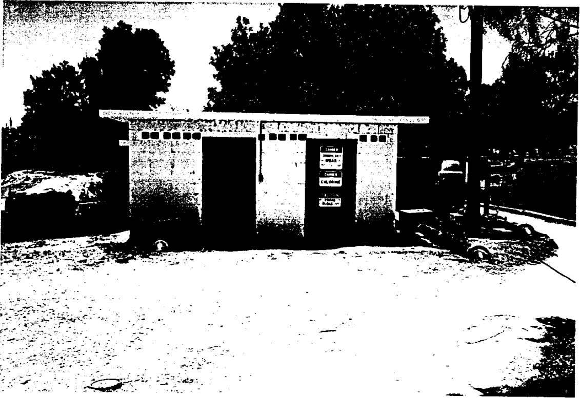
SAN FELIPE WELL PUMPING STATION - NORTH ELEVATION (WEST FACILITY)
