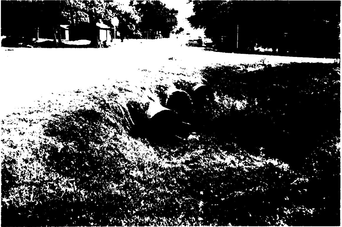
PHOTO III.9 View of Tanglewood Culverts
