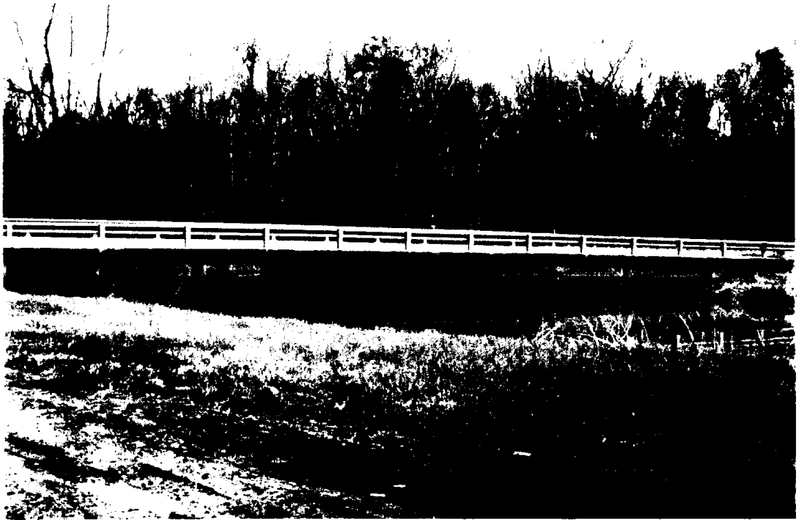
PHOTO III.1 Western Ave. Bridge
