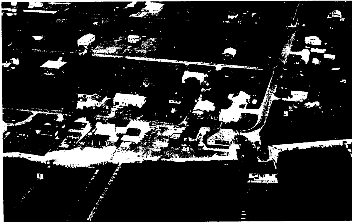
MAINLAND - SAN LEON: BAY SHORE EROSION
