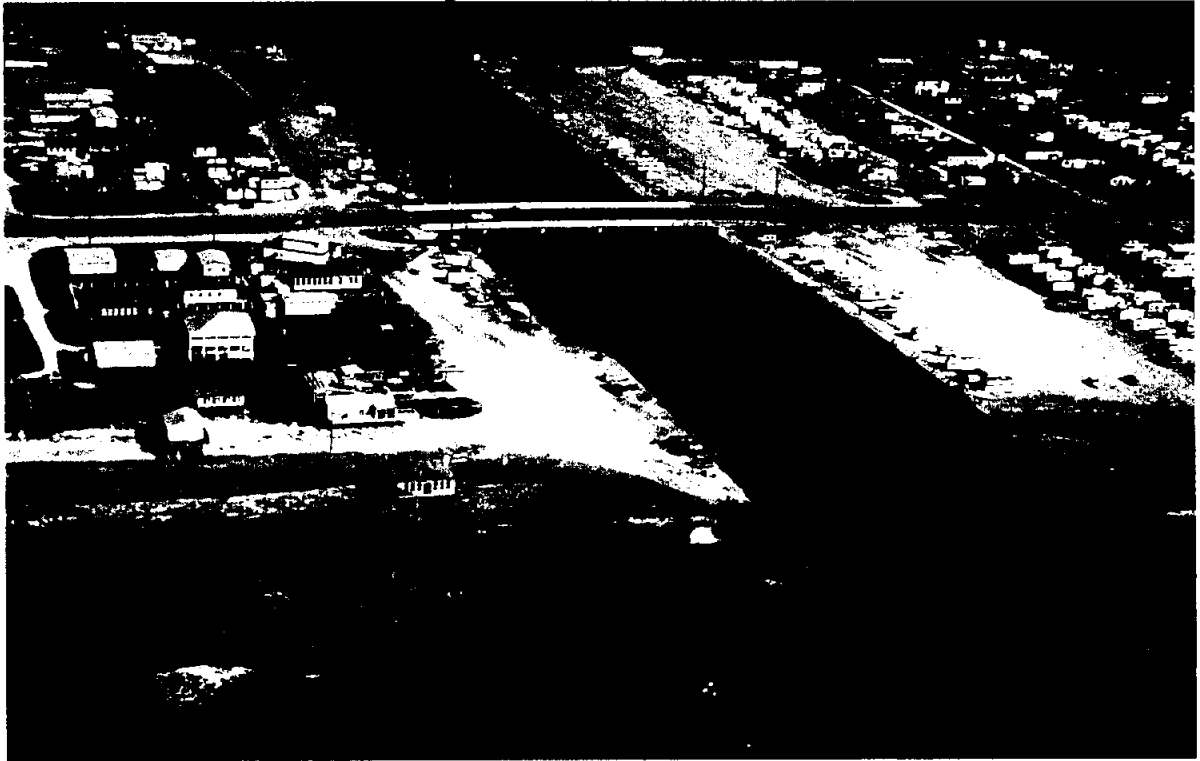
BOLIVAR - ROLLOVER PASS: HOUSES THREATENED
