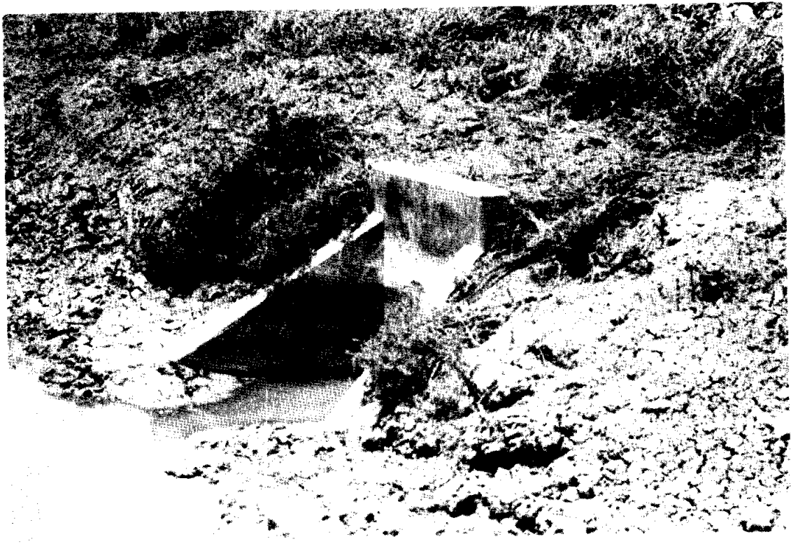
AIRPORT DRAINAGE Airport Drainage Outlet Headwall Note Sediment Line on Headwall After Recent Ditch Cleanout
