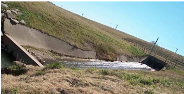
Figure 2-26 Storm Drainage Outfall TXR1
