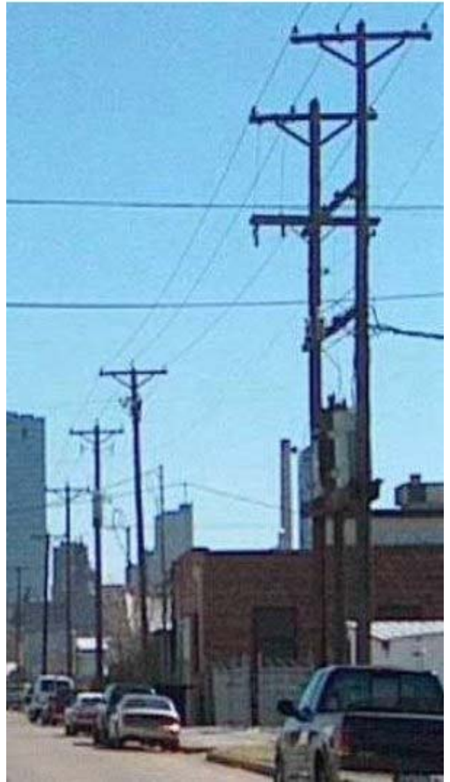
Figure 2-31 Overhead Power Lines
