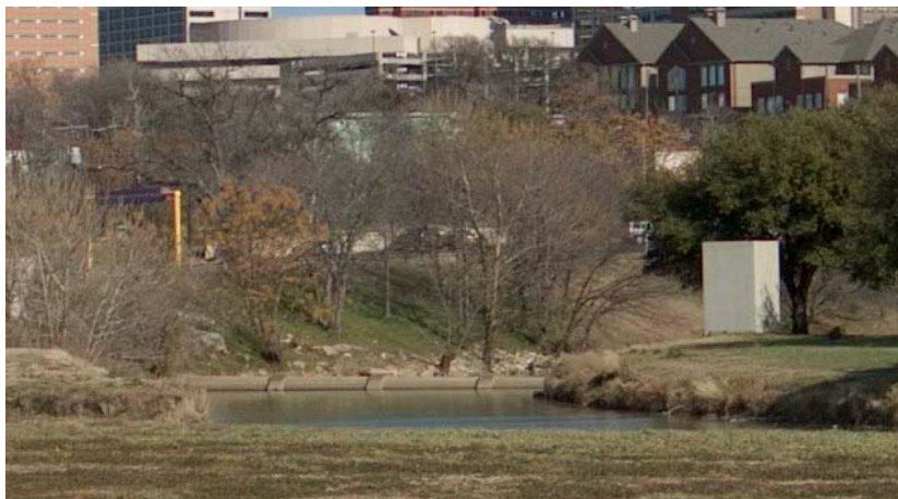
Figure 2-19 Sanitary Sewer Main 272-B Siphon Crossing of Inlet to the Clear Fork Trinity River, Located North of Forest Park Blvd.
