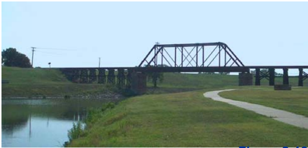
Figure 2-13 Railroad Bridge – Fort Worth and Western RR
