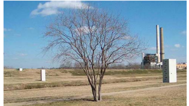
Figure 2-17 Sanitary Sewer Main 132 Siphon Crossing, (now abandoned), of The West Fork Trinity River Located North of The TXU Power Plant.
