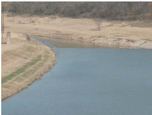
Figure 2-7 Upstream view of Nutt Dam
