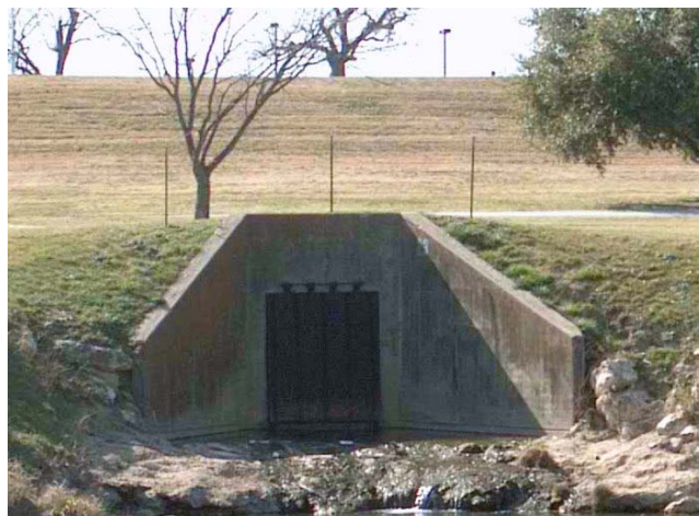
Figure 2-24 Storm Drainage Outfall MW2
