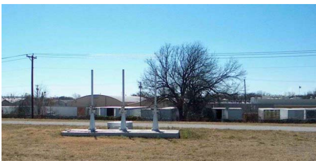
Figure 2-22 Gate Operators for Storm Drainage Sumps
