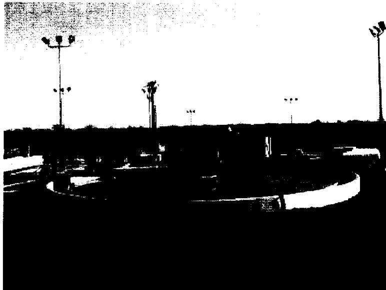
Figure A-17: Orbital System Aeration Basin and Aerobic Digester.
