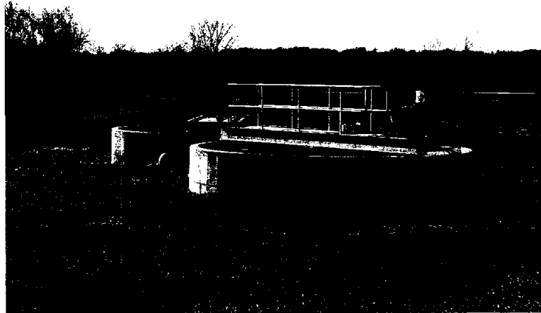
Figure A-7: Mixed liquor final clarifiers.
