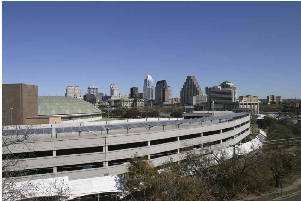
Figure 7-4.3-1 Solar Power Array on a Parking Lot Rooftop in Austin, Texas
