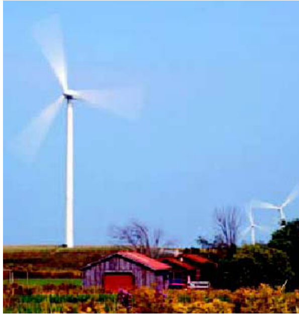
Figure 7-3-1 Turbines Generating Power on the Fenner, NY Wind Farm
