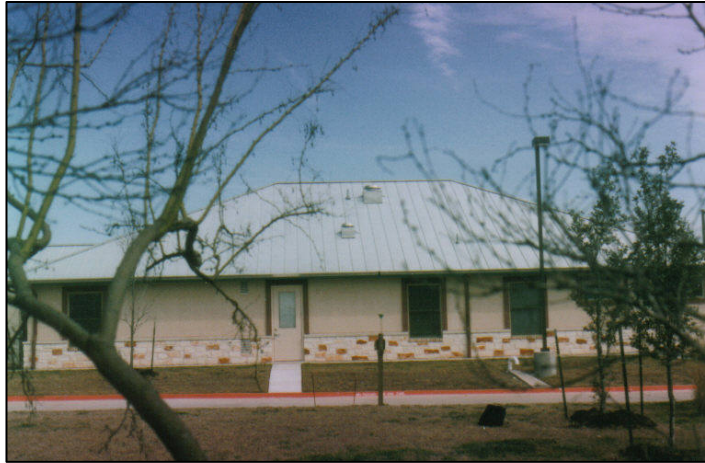
The Feather & Fur Animal Hospital in South Austin features a standing-seam metal roof for rainwater harvesting.
