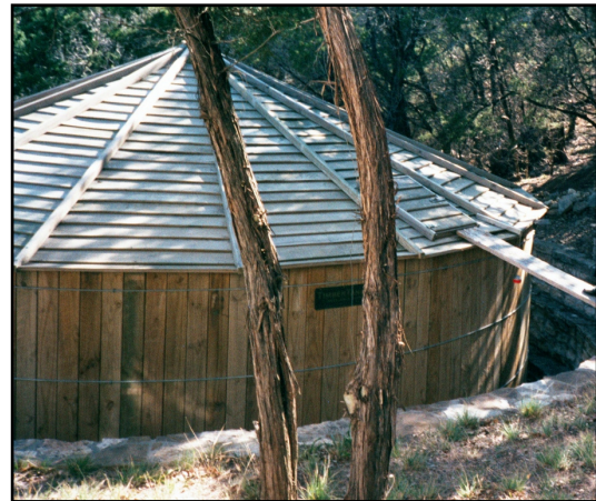
Figure 2-7. Installation of a 25,000-gallon Timbertank in Central Texas showing the aesthetic appeal of these wooden tanks
