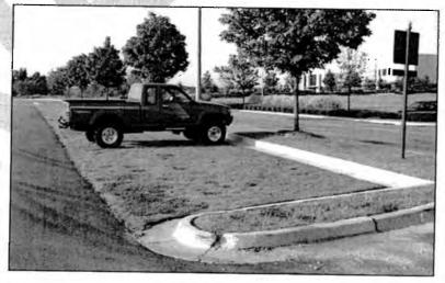
Figure 1.3.2-21 Grass Paver Surface Used for Parking
