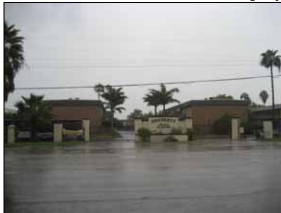
University Manor Apartments
