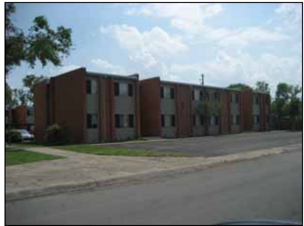
North Star Village Apartments
