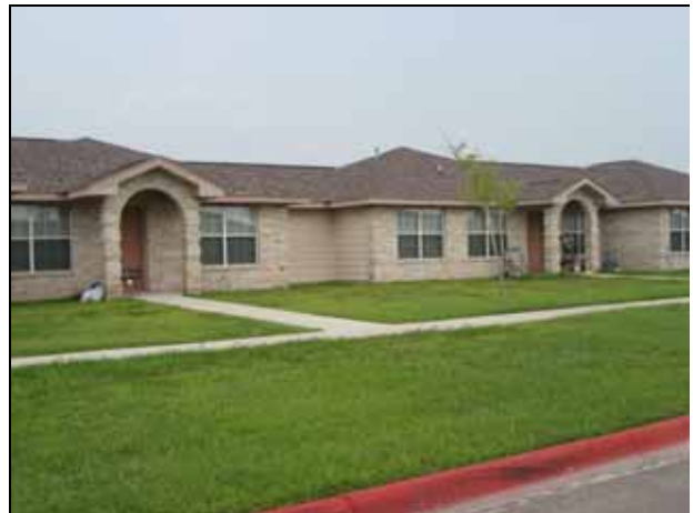
Valley View Apartments
