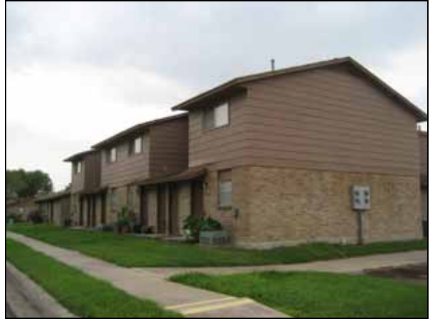
Valley View Apartments
