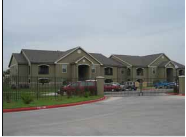
Rudy Villareal Oak Square Apartments
