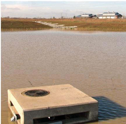
Hickory Creek Fire Station, best management practices in the City of Denton.
