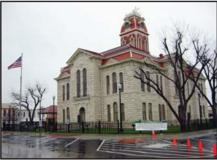
Architectural Barriers staff worked with the Texas Historical Commission to ensure accessibility of historic county courthouses, such as this one in Lampasas
