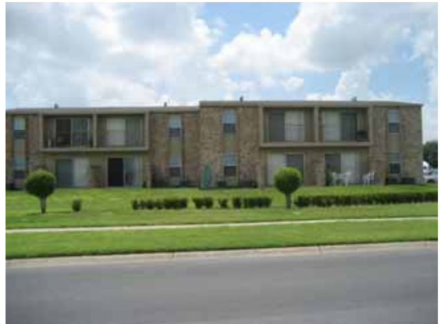
La Vista Apartments
