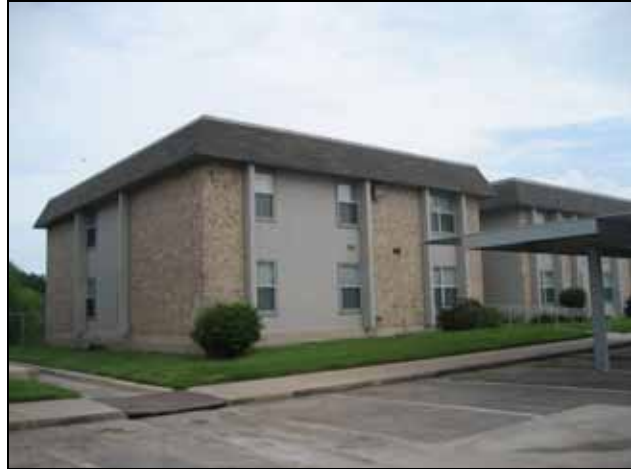
Rockwell Manor Apartments
