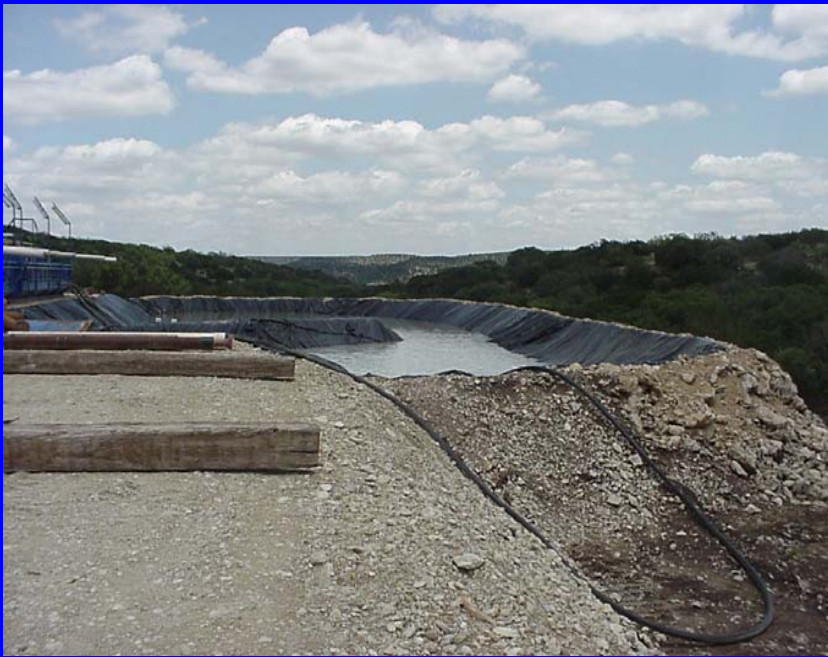
Lined Drilling Mud Pit
