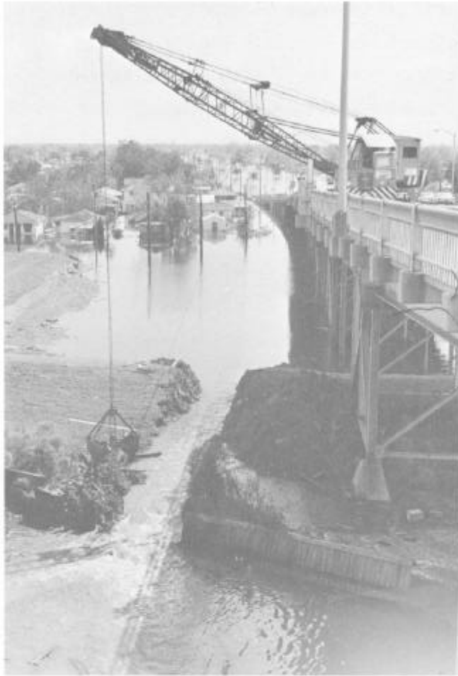
Figure 40. Clamshell breaching the levee to drain floodwaters
