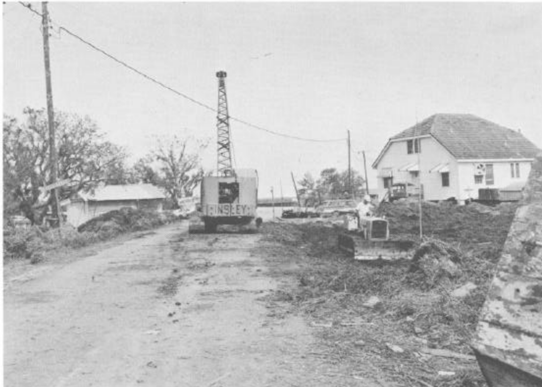
Figure 49. Small bulldozer gathering debris for pickup by crane
