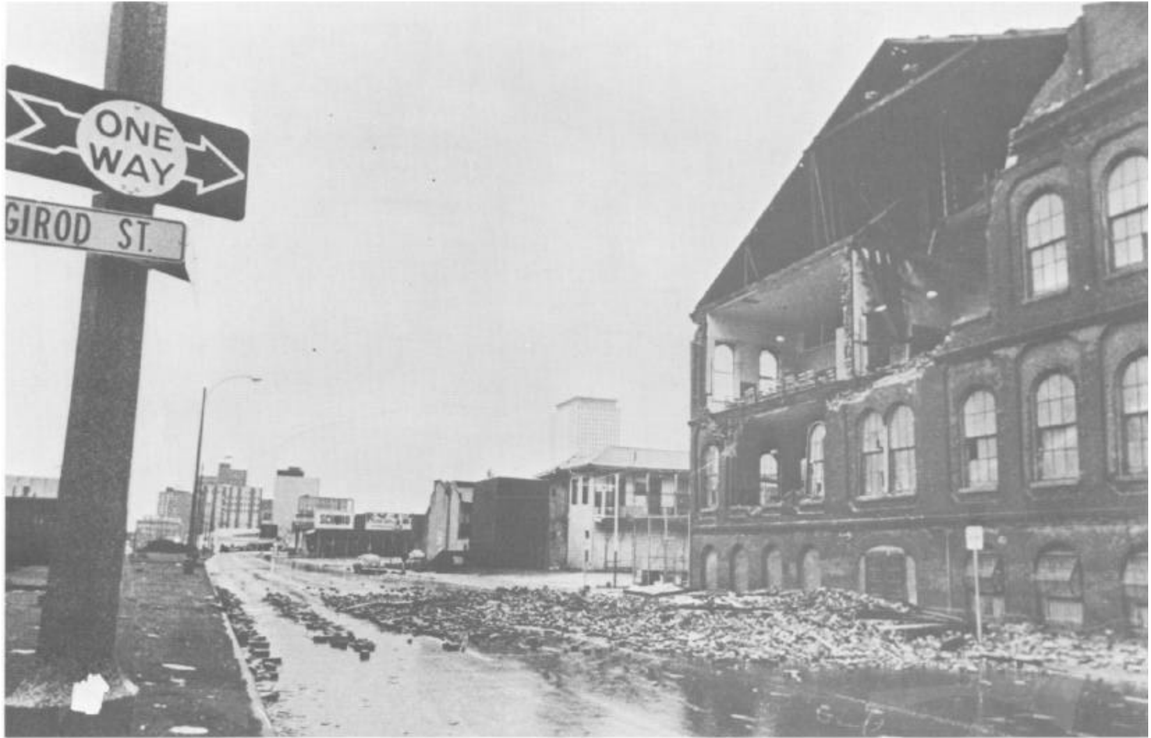
Figure 41. School buildings suffered heavily from Betsy's fury (Photo by Times-Picayune Pub. Co.)
