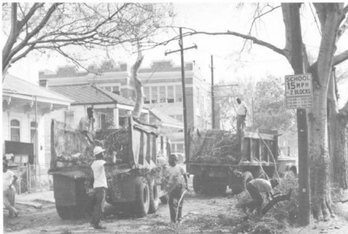
Figure 19. Corps of Engineers' contractor removing debris from New Orleans streets
