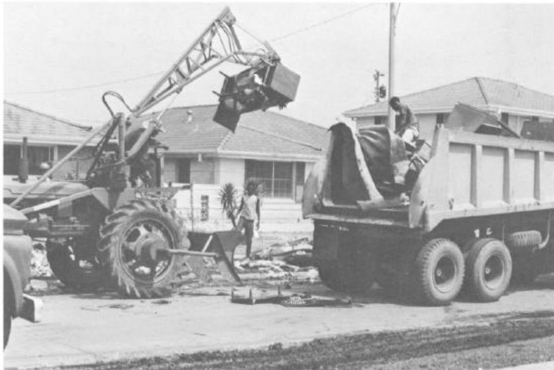
Figure 50. Cane loaders were used for loading of bulky items
