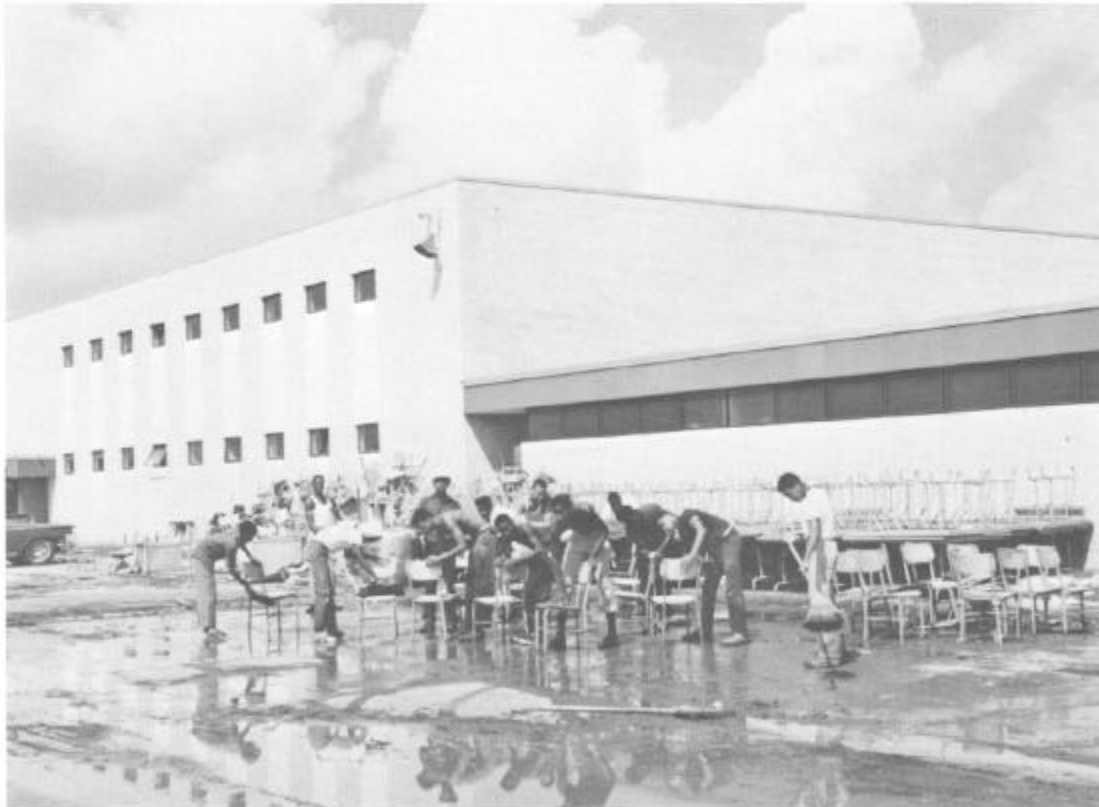
Figure 35. Corps of Engineers contractor cleaning school furnishings in New Orleans
