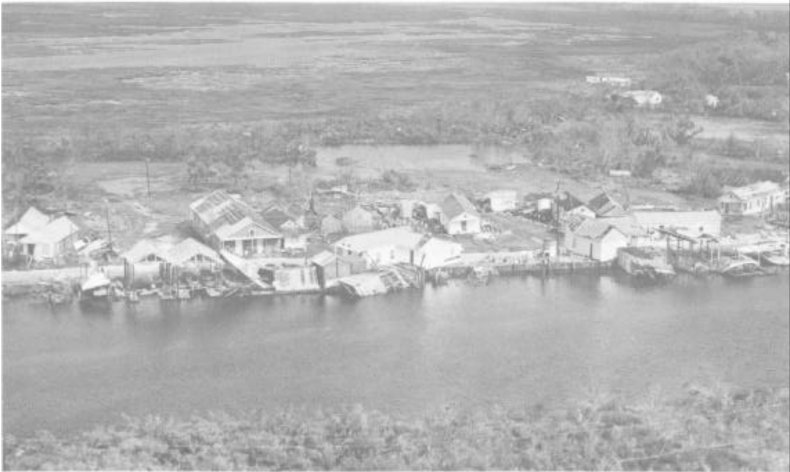
Figure 9. Wind damage along Bayou Terre aux Boeufs in St. Bernard Parish
