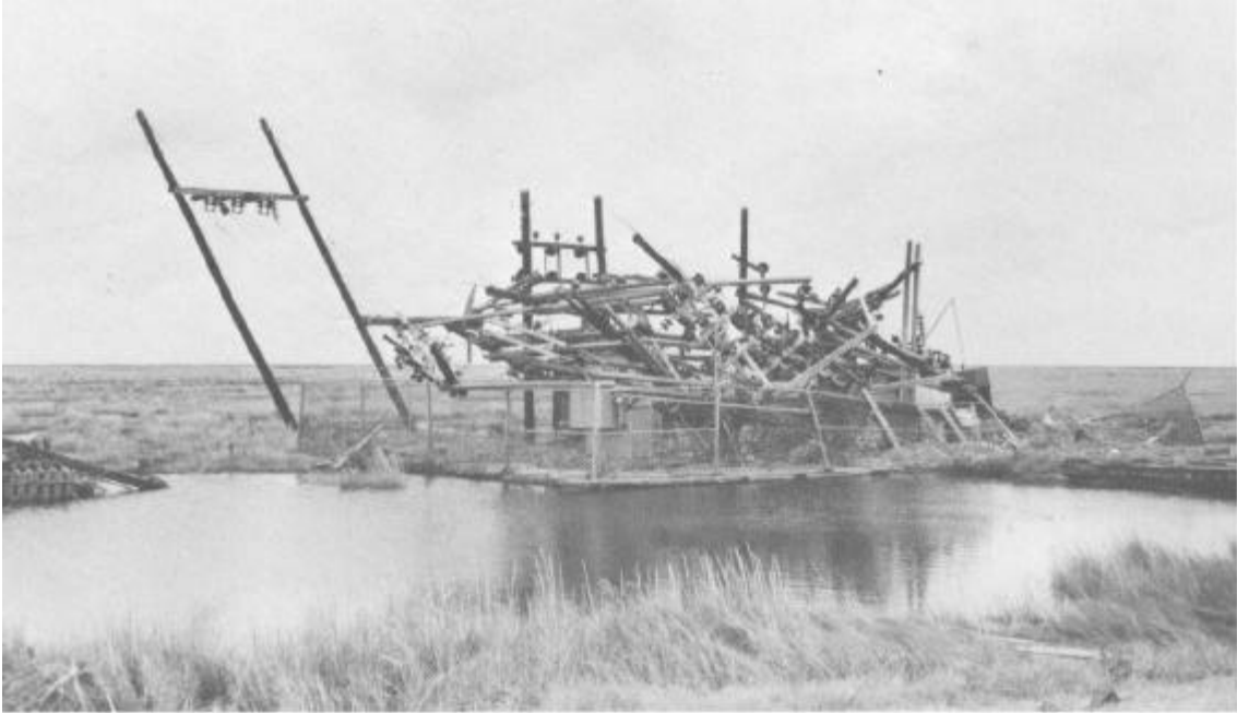
Figure 11. Electrical substation in Lafourche Parish
