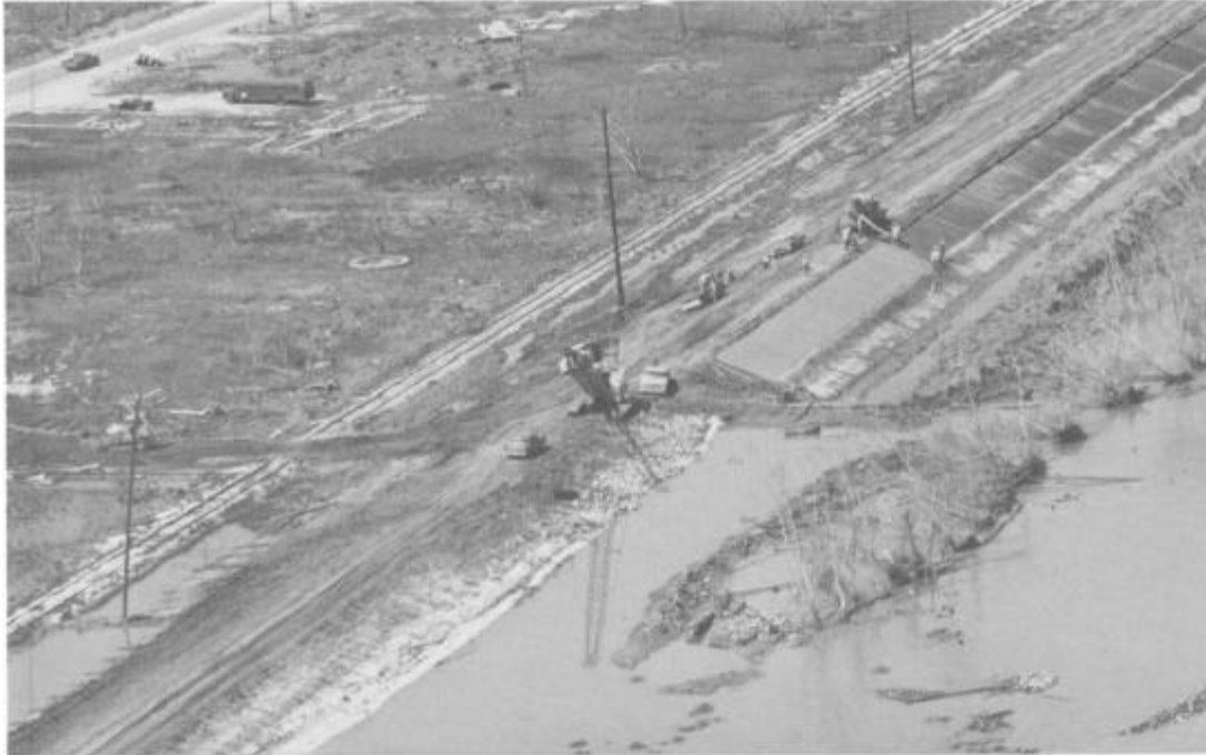
Figure 54. Repairs being made on a main line levee
