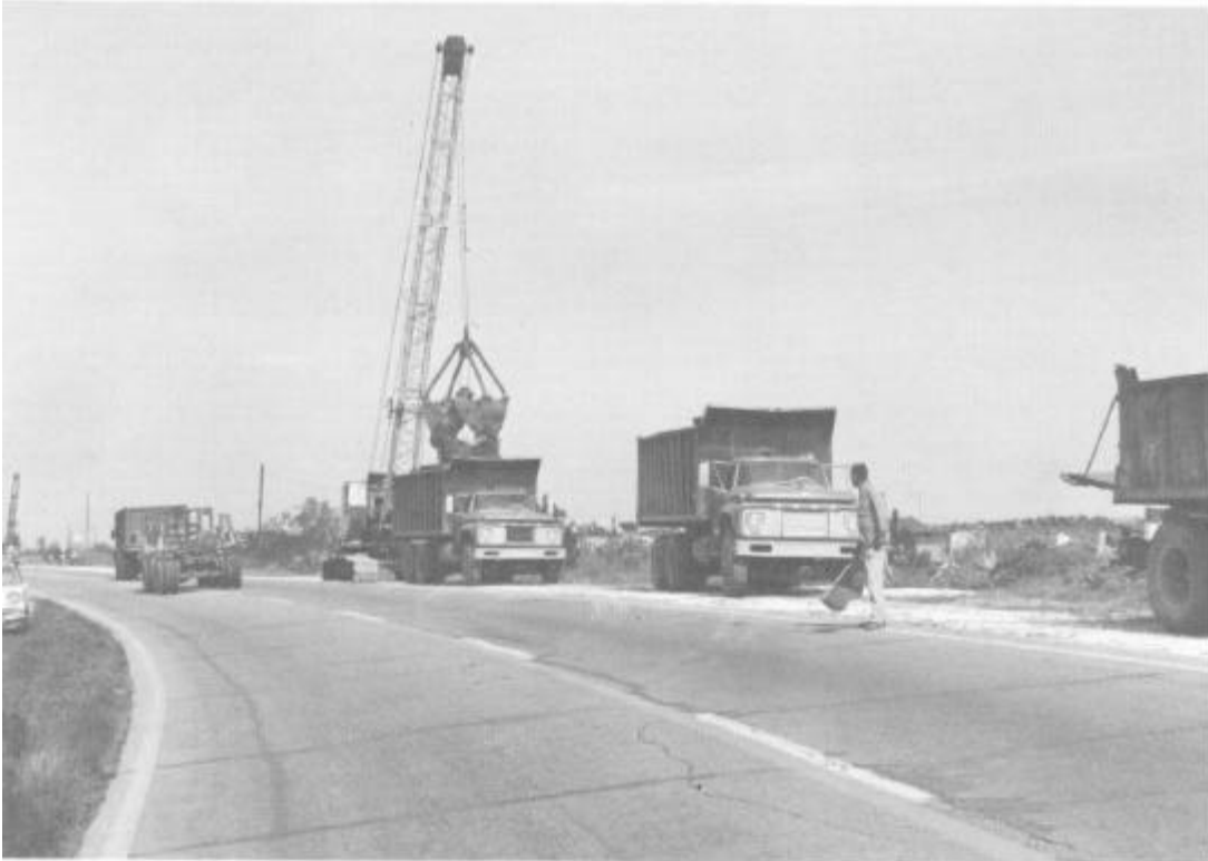
Figure 47. Crane with clamshell bucket loading waterborne debris
