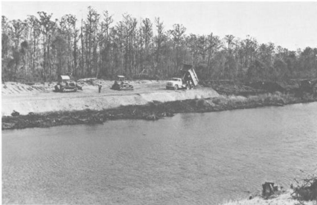
Figure 55. Repair of Chalmette Back Levee (Carolyn Park)
