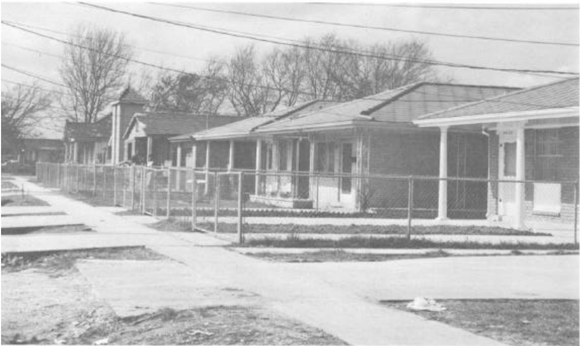
Figure 28. After Corps of Engineers cleanup, Orleans Parish
