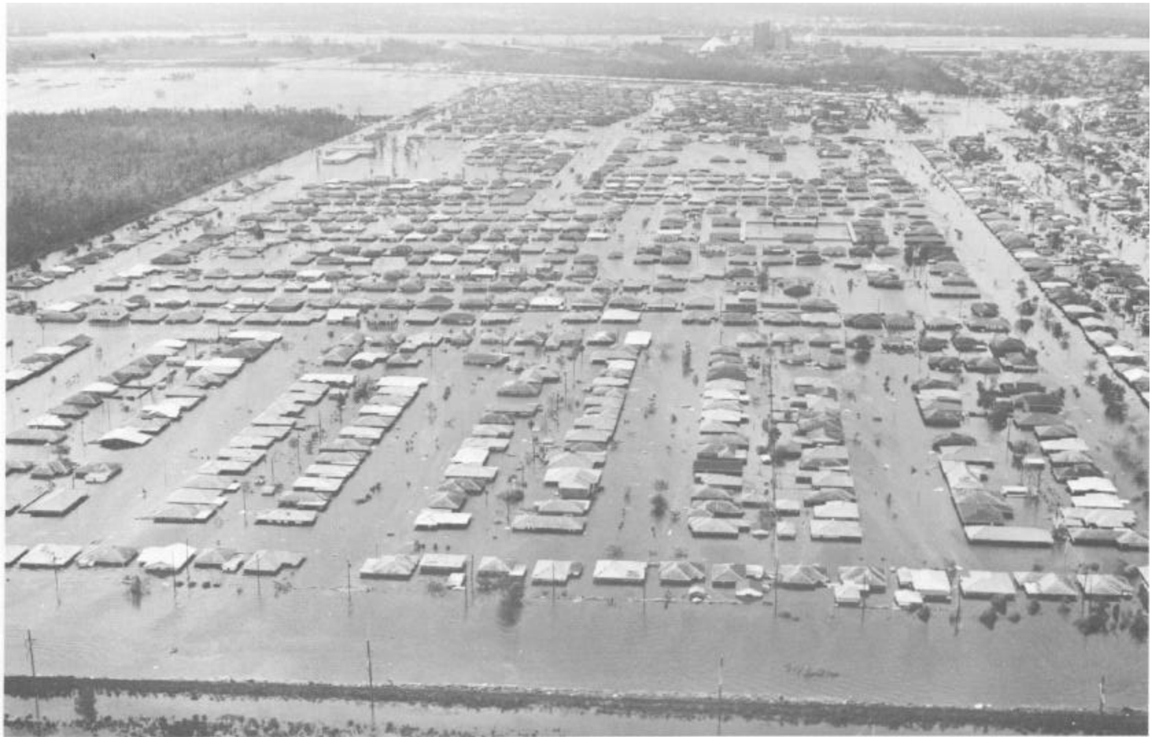
Figure 13. Flooding of Carolyn Park in St. Bernard Parish
