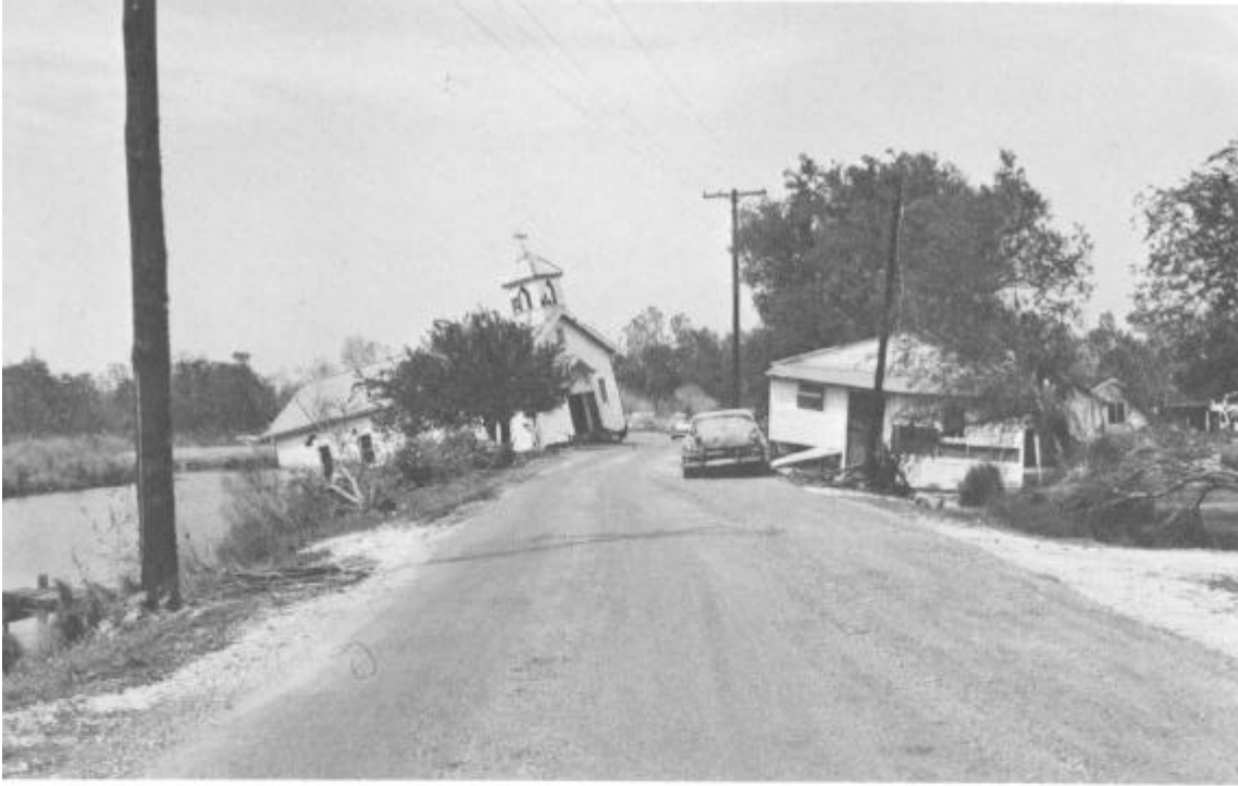
Figure 30. Church blown across road near Reggio, La.
