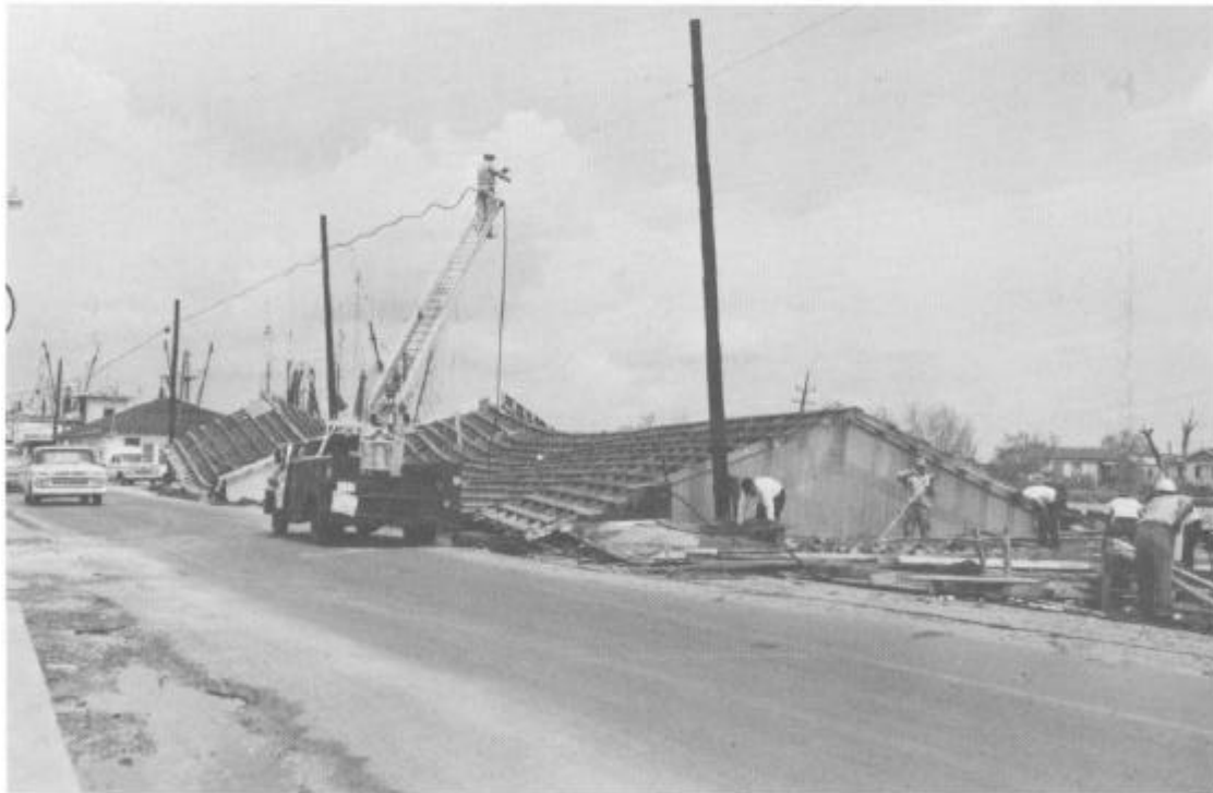
Figure 6. Oyster house and seafood plant in Lafourche Parish destroyed by the hurricane winds
