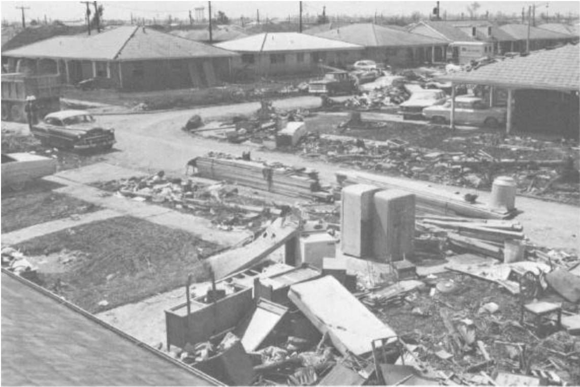
Figure 25. Before Corps of Engineers cleanup, St. Bernard Parish
