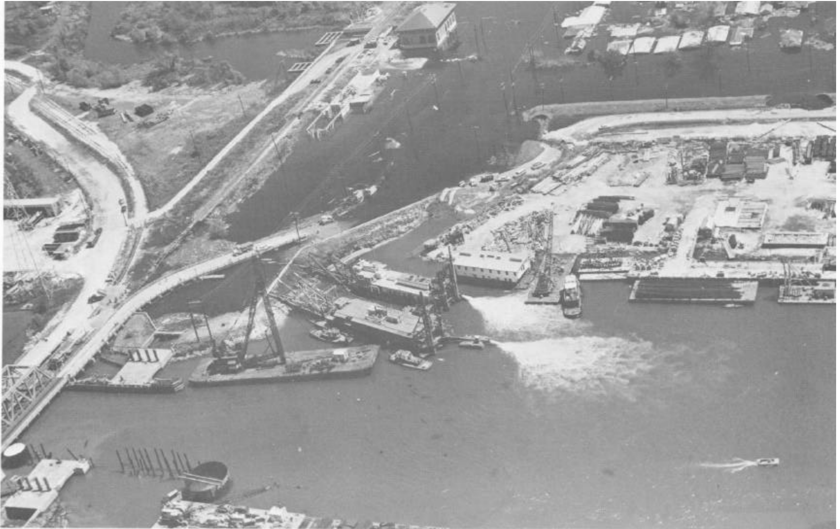
Figure 37. Corps of Engineers leased dredges pumping out floodwaters in New Orleans
