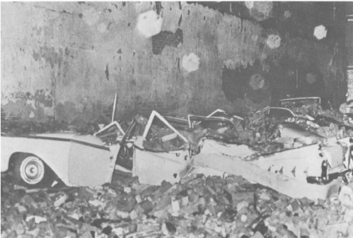
Figure 12. Brick wall collapses during hurricane, New Orleans, La.
