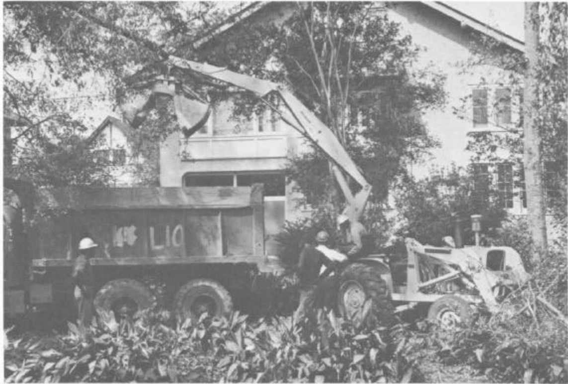
Figure 51. Pulpwood loaders were easily adapted for debris loading
