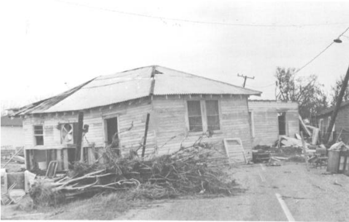
Figure 31. House blocking road near Shell Beach on Lake Borgne
