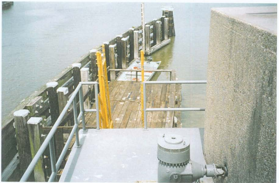
PHOTO NO. 36 – NEW BOAT DOCK DECK.
