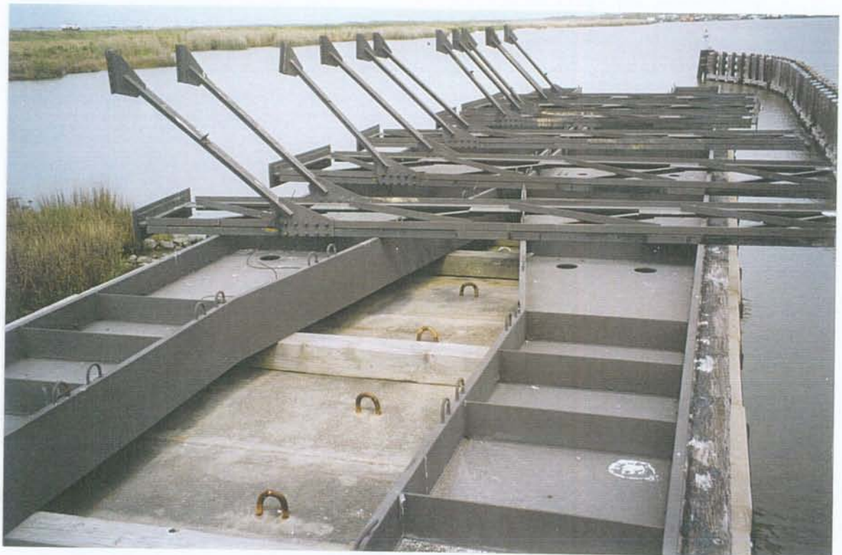
PHOTO NO. 32 – DEWATERING ELEMENTS STACKED ON STORAGE RACK.
