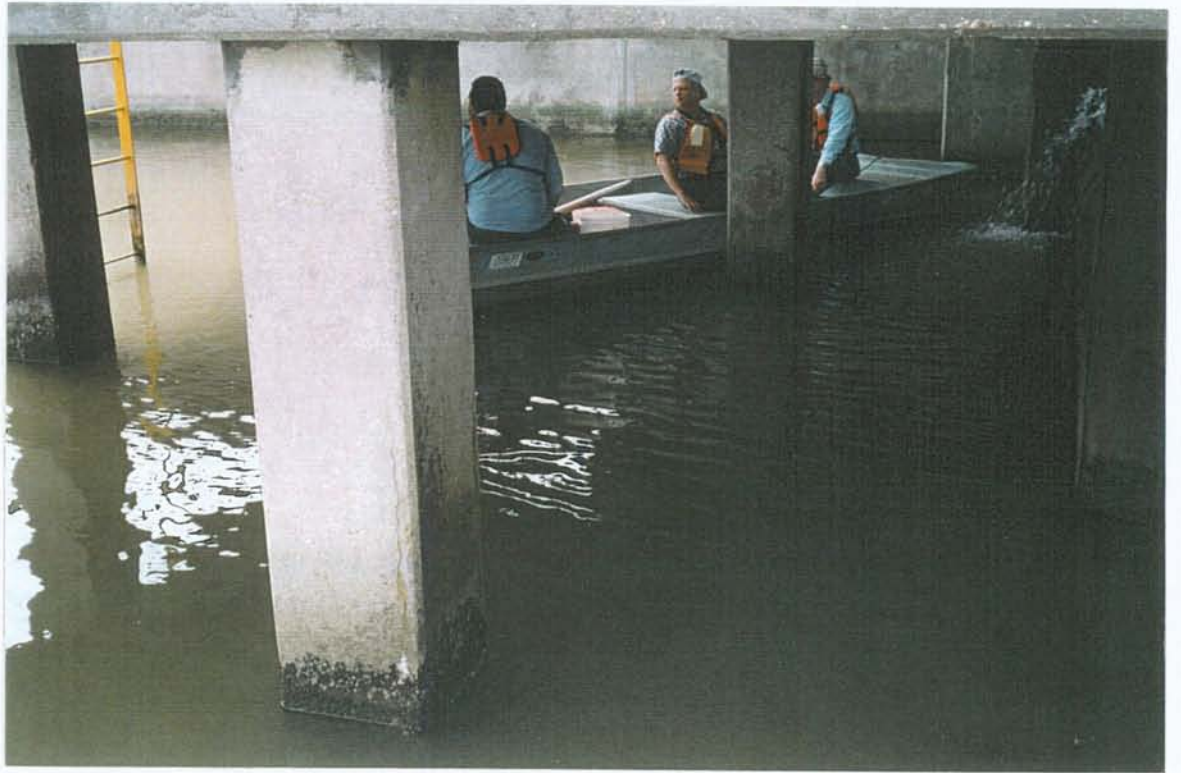
PHOTO NO. 12 – LOOKING SE AT CRACK IN NORTH FACE OF PUMP PLATFORM PILE NO 7.
