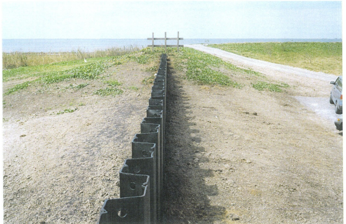
PHOTO NO. 40 – WEST SHEET PILE FLOODWALL.
