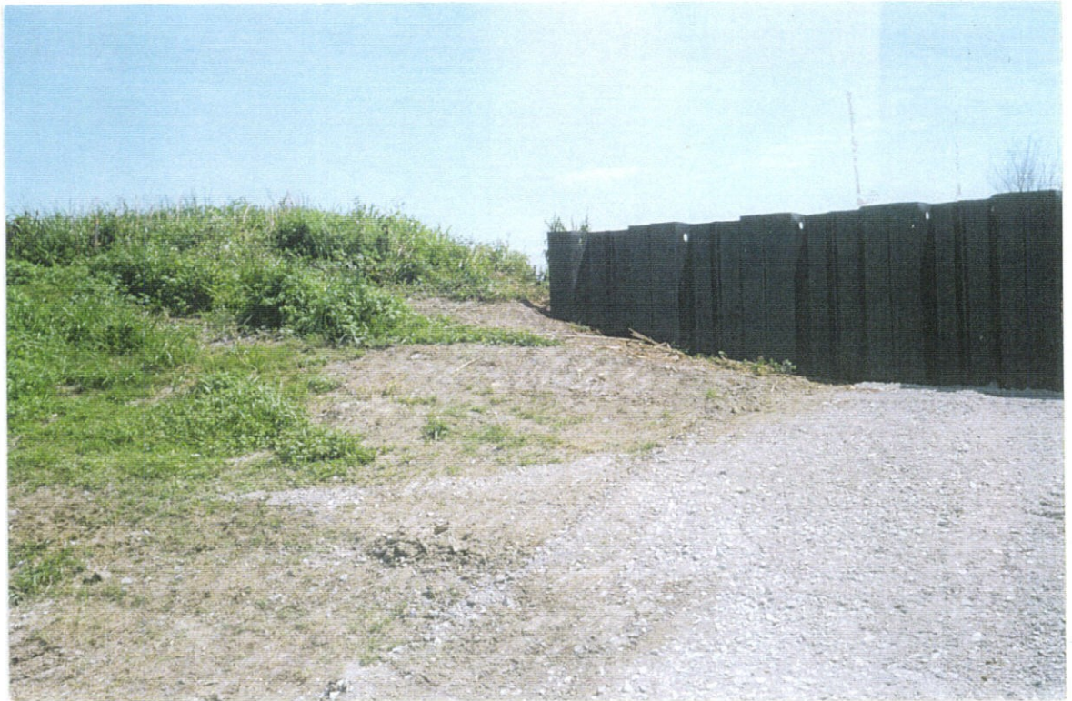
PHOTO NO. 41 – EAST END OF EAST SIDE SHEET PILE FLOODWALL. NOTE LOW LEVEE EMBANKMENT AREA.
