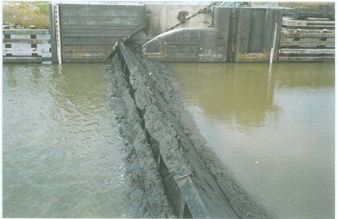
PHOTO NO. 22 - GATE BEING CLOSED (RAISED). NOTE SILT SLIDING OFF.
