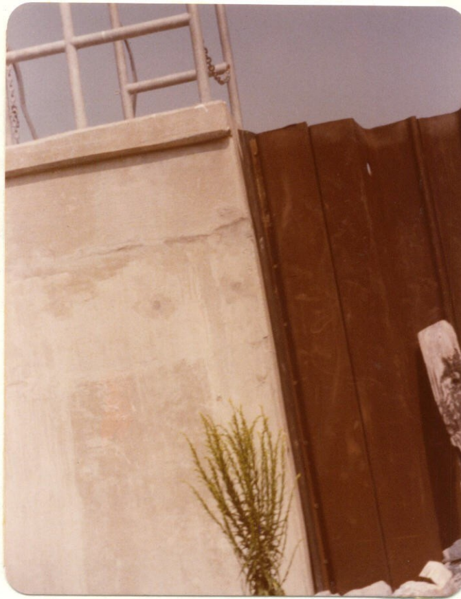
PHOTO NO. 4 - Location of Waterstop Between T-Wall Monolith and Sheetpiling
