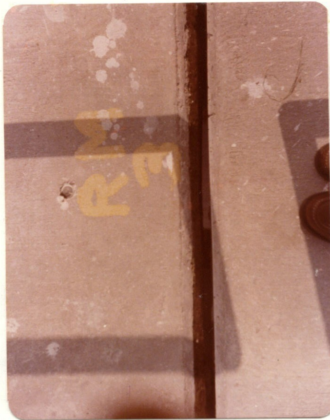
PHOTO NO. 3 - Joint Between Reference Mark RM2-RM3
