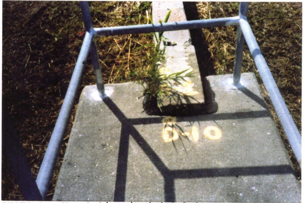
PHOTO 3 - Vegetation in joint between concrete sheetpile and T-wall on the east side
