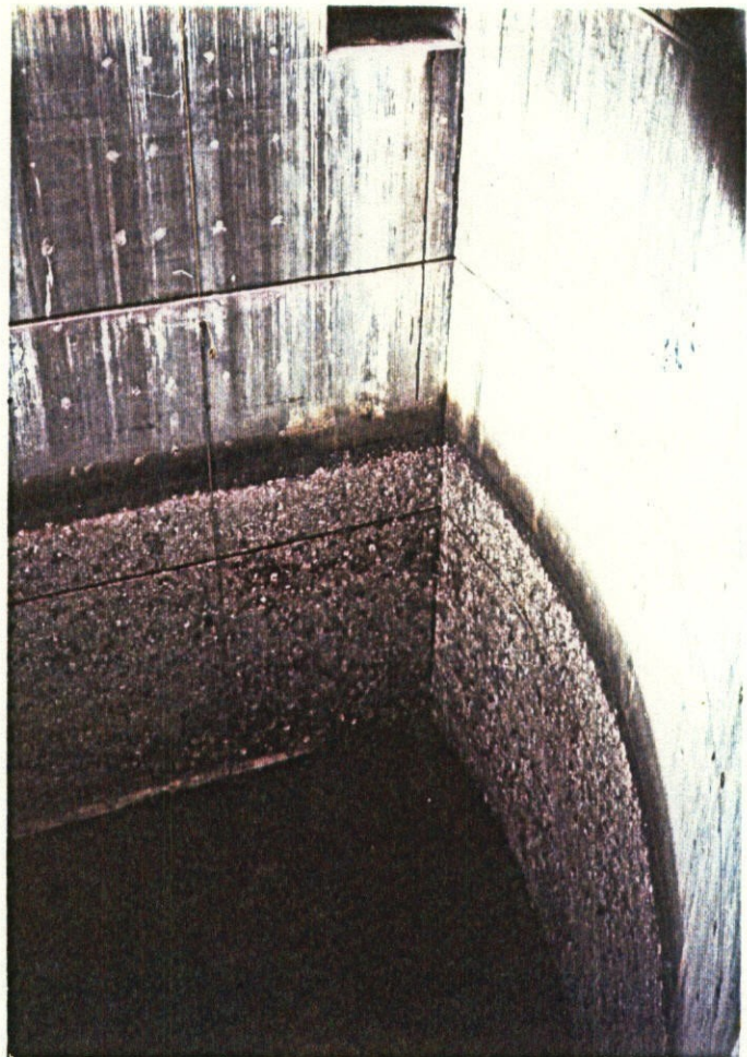
Photo No. 6 - Notice marine growth on concrete walls of gate recess. (18 March inspection)
