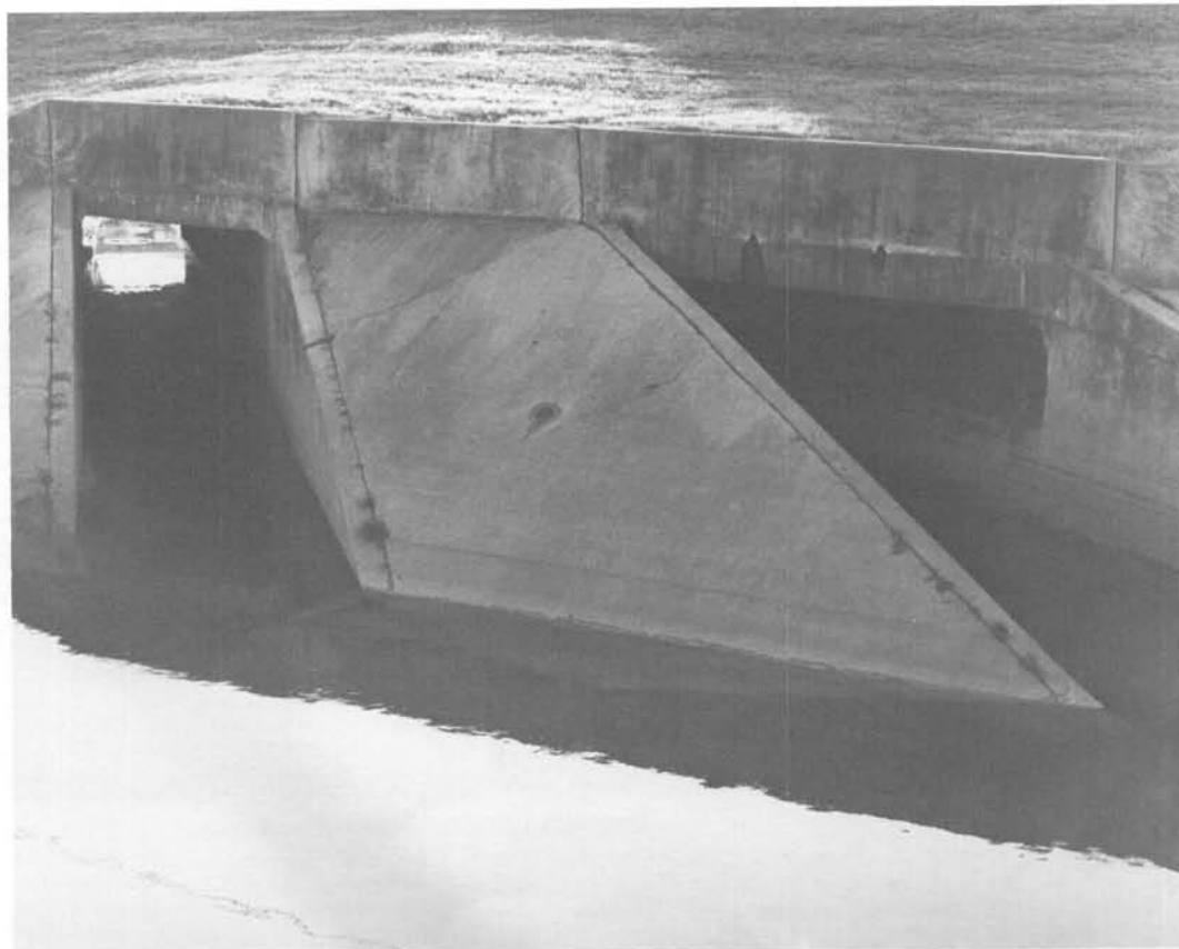
Box Culvert at Hoey's Canal Entrance to Seventeenth Street Canal
