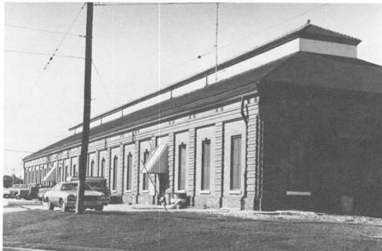
Drainage Pumping Station No. 1
