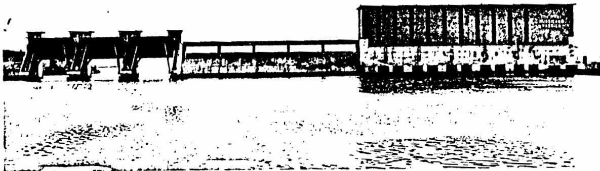
Looking downstream at Fox Point Barrier river gates, the non-overflow section and the pumping station
