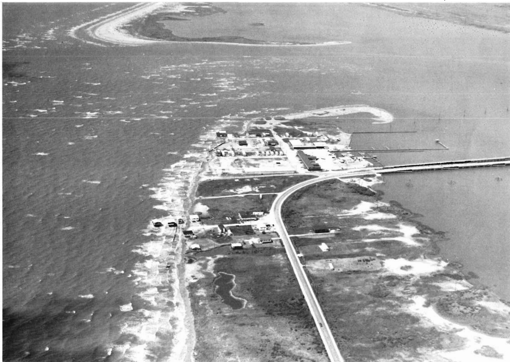
Photograph 1 Critically eroding West End of Grand Isle
