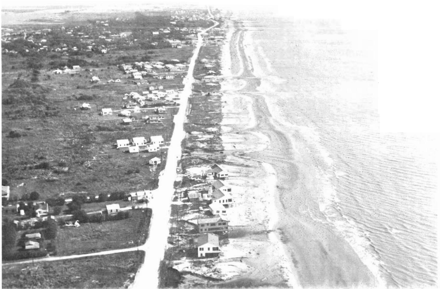
Photograph 8 Grand Isle after Sheet Flow from Hurricane Flossy
