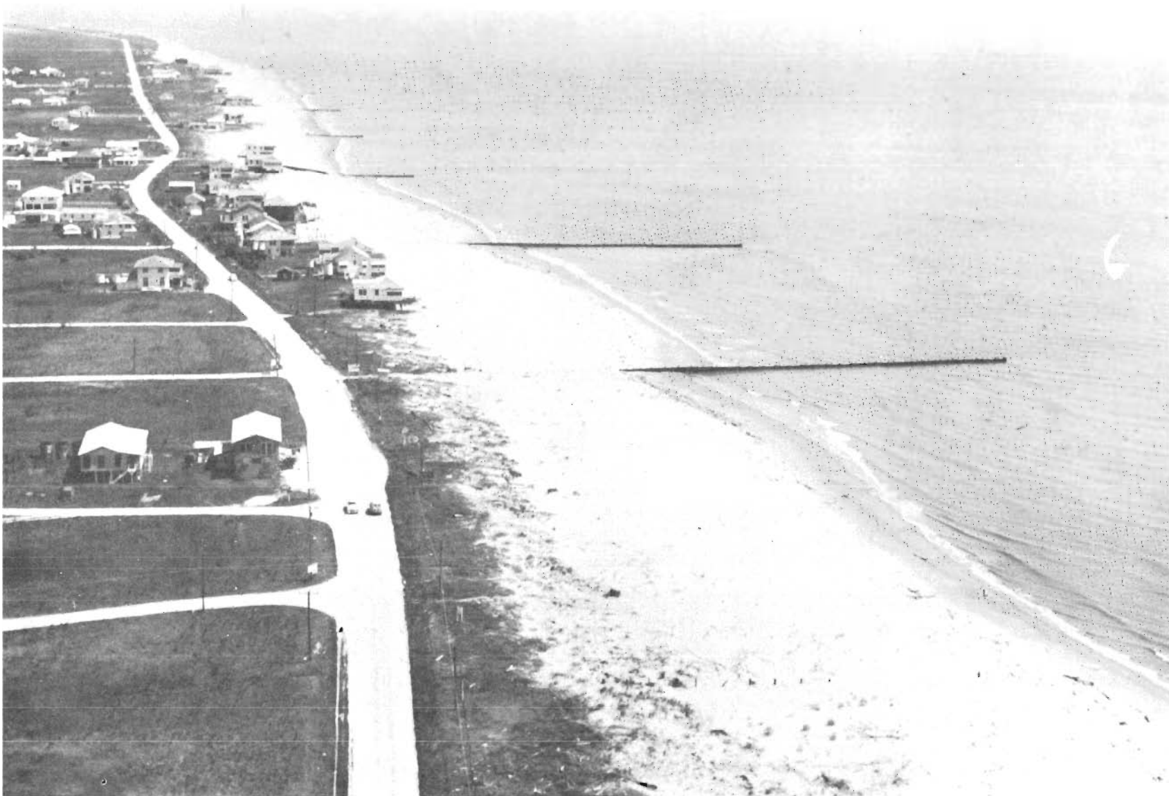
Photograph 6 Groins 7 through 14 after Artificial Beach Nourishment
