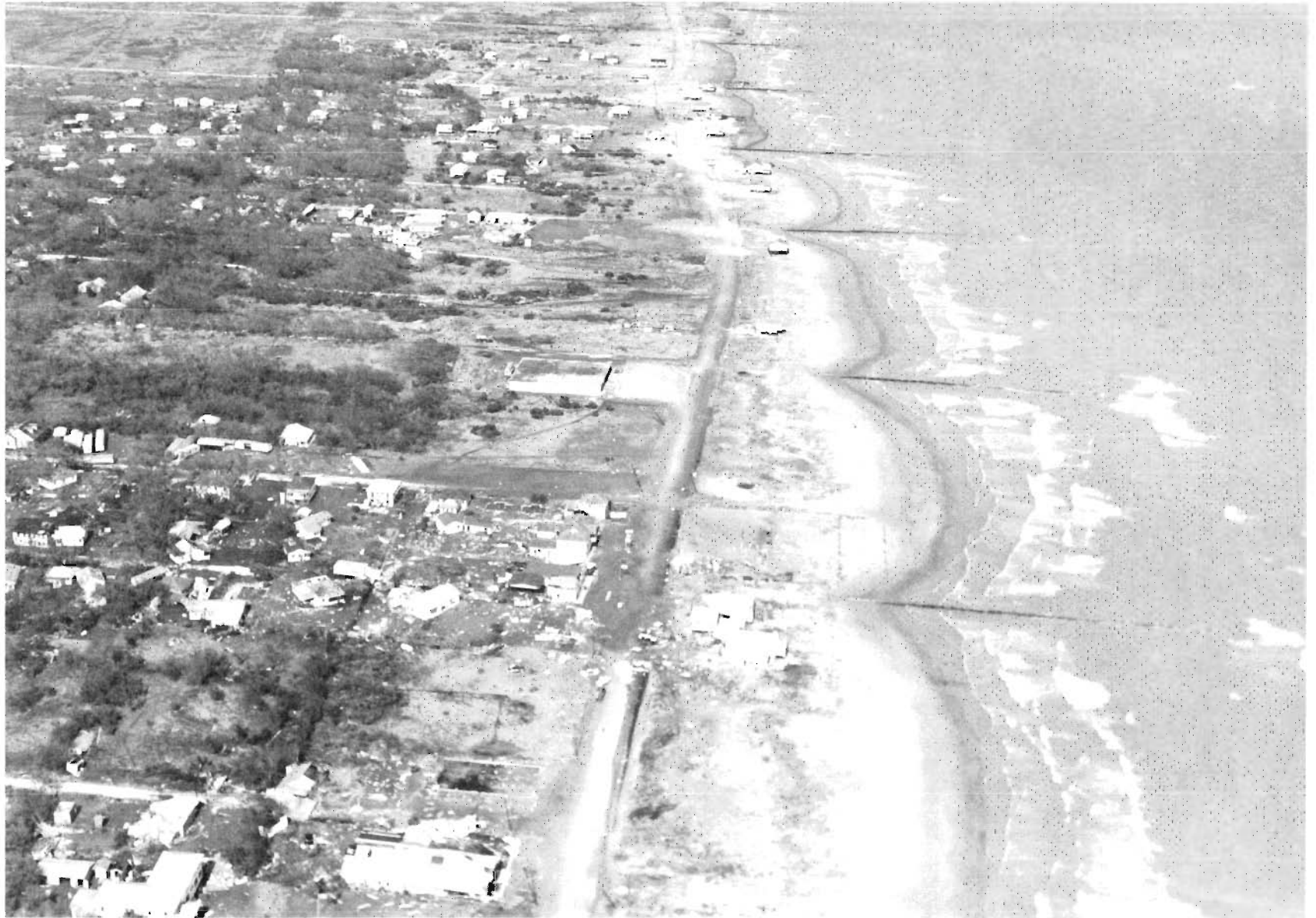
Photograph 4 Damage on Grand Isle after Hurricane Betsy
