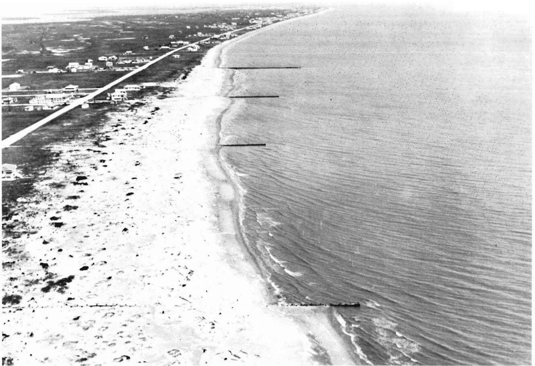
Photograph 5 Groins 1 through 4 after Artificial Beach Nourishment
