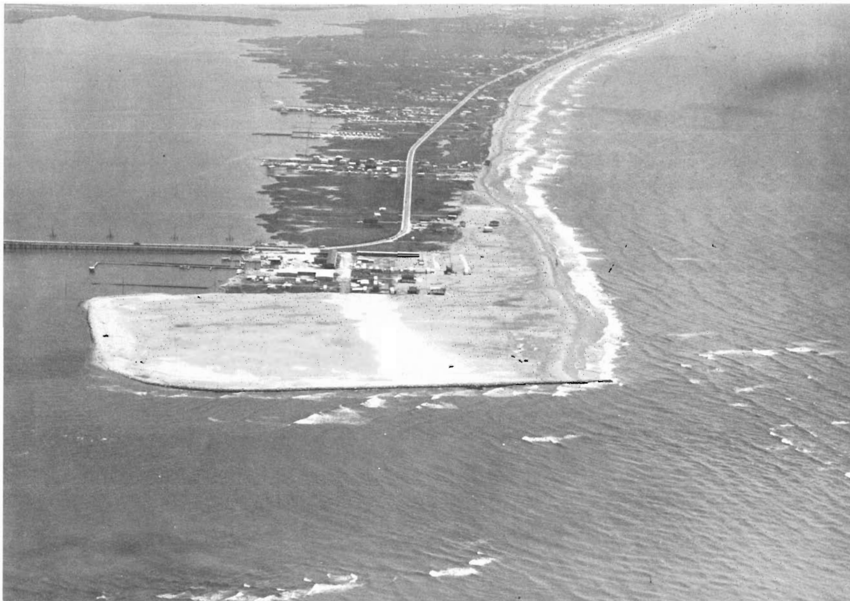
Photograph 2 West End of Grand Isle after Completion of Emergency Work.
