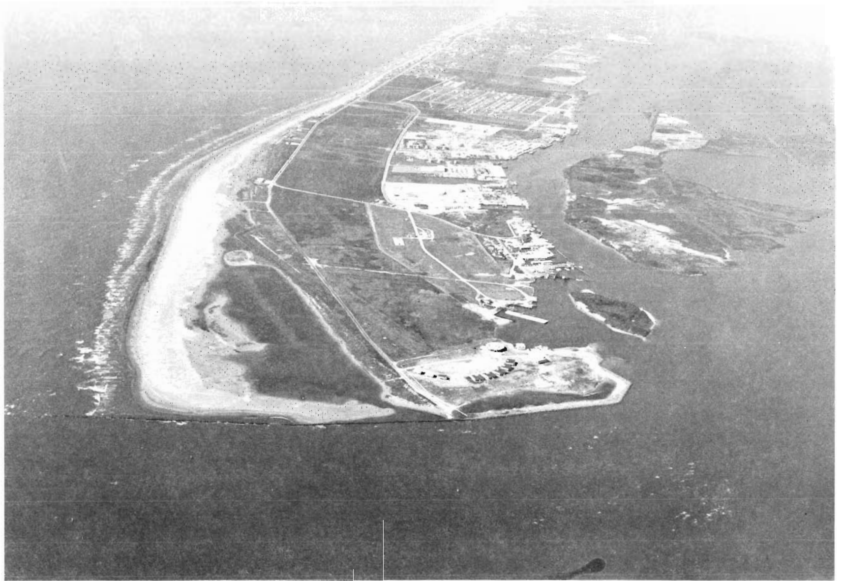
Photograph 13 East end of Grand Isle after construction of U. S. Coast Guard revetment
