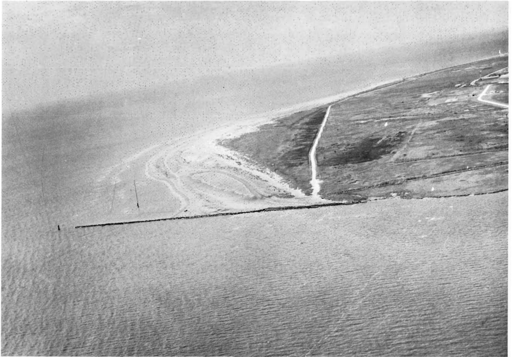
Photograph 10 East end jetty approximately 3 years after construction
