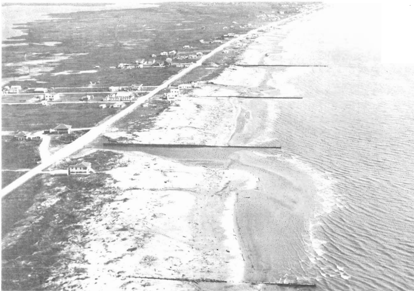
24 Photograph 7 Grand Isle after Sheet Flow from Hurricane Flossy
