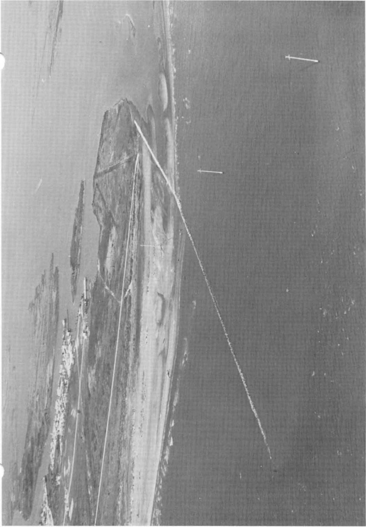
Photograph 11 East end jetty after its extension in 1964
