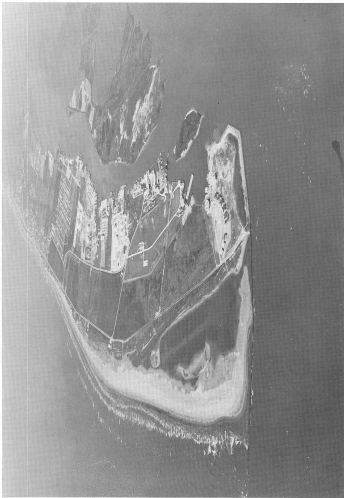
Photograph 13 East end of Grand Isle after construction of U. S. Coast Guard revetment
