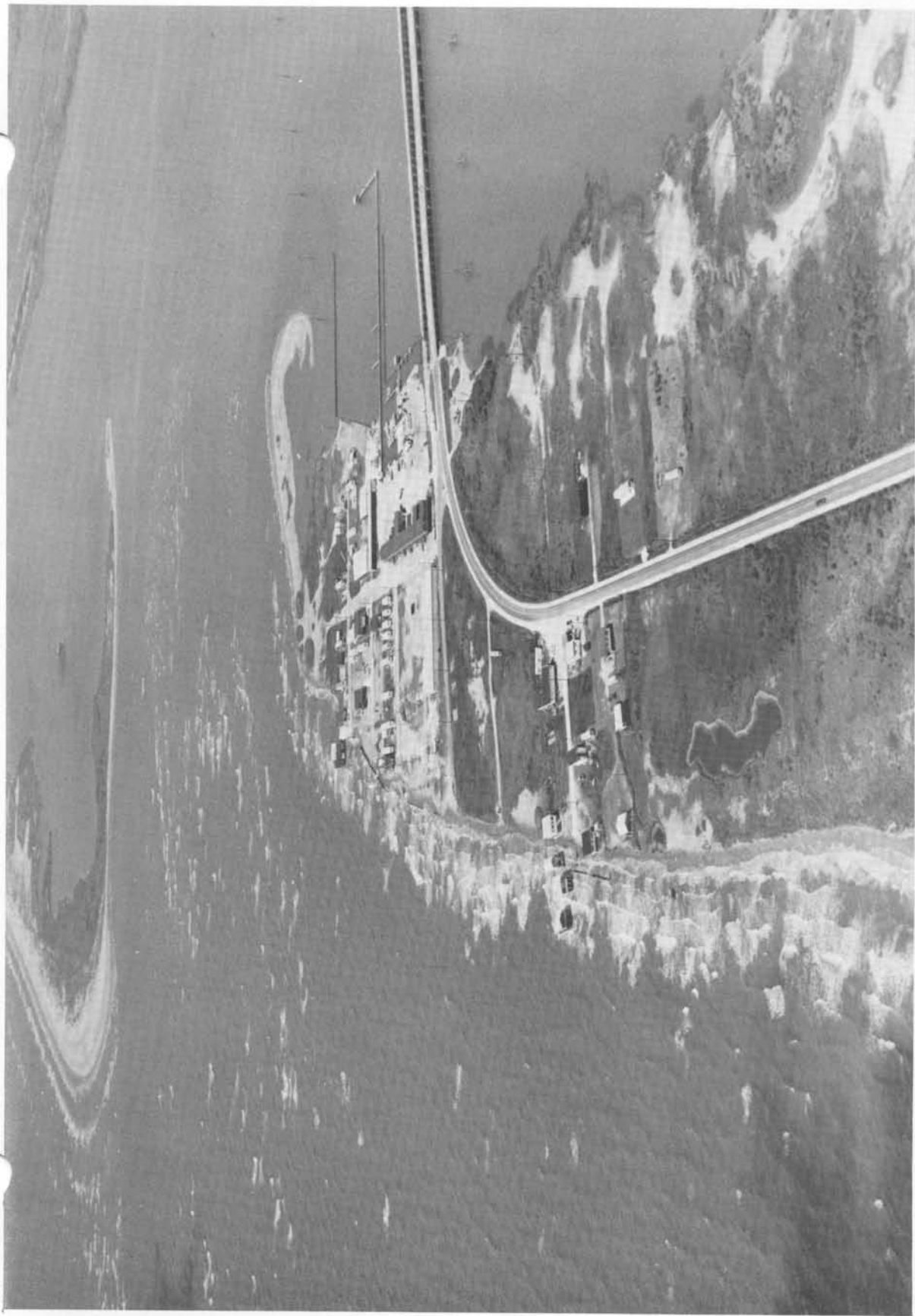
Photograph 1 Critically eroding West End of Grand Isle
