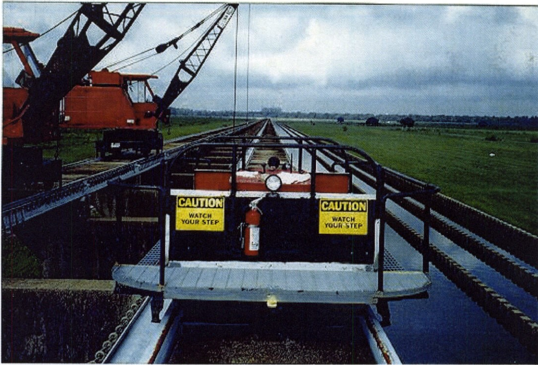
PHOTO 1 – Spillway looking west.
