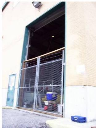
Photo 1—Missing Roll Up Door Photo 2—Damaged Down Spout
