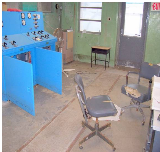
PHOTO 2—DAMAGED TILE IN CONTROL ROOM
