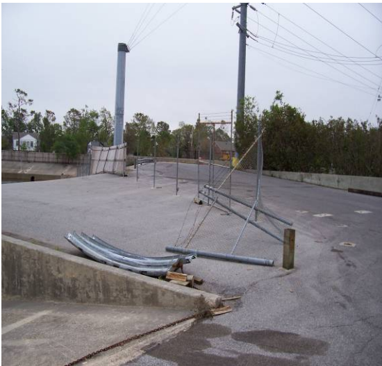
Photo 3 – Damaged fence on Maryland side.
