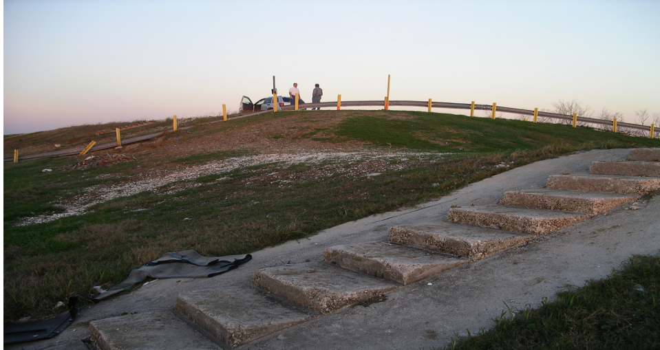
Figure J-B5. Begin Lakefront Levee at Citrus Lakefront and Paris Road (Lakefront Levee @ El. 19.0 +/- and Citrus Lakefront Levee @ 13.5+/-)
