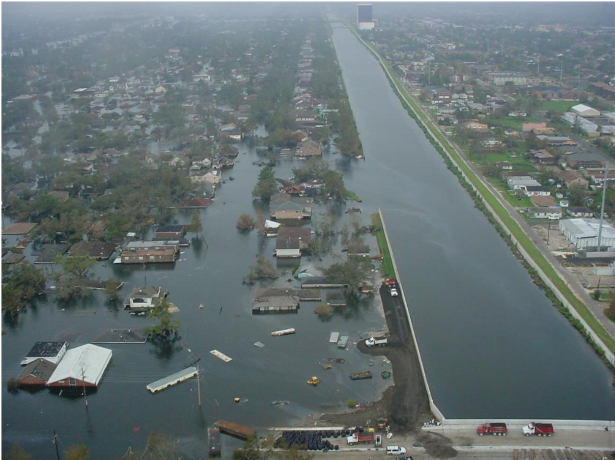
Figure VI-1. Aerial photograph of the 17th Street Canal breach looking south from Old Hammond Road bridge
