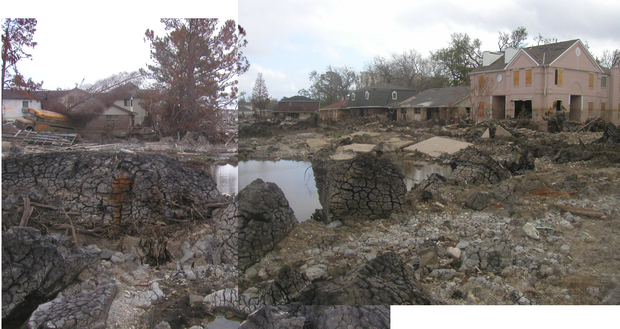
Figure VI-7. Peat blocks from the levee embankment
