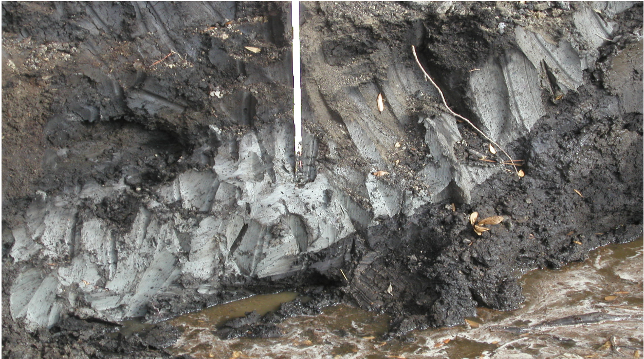
Figure VI-9. Exposed failure plane
