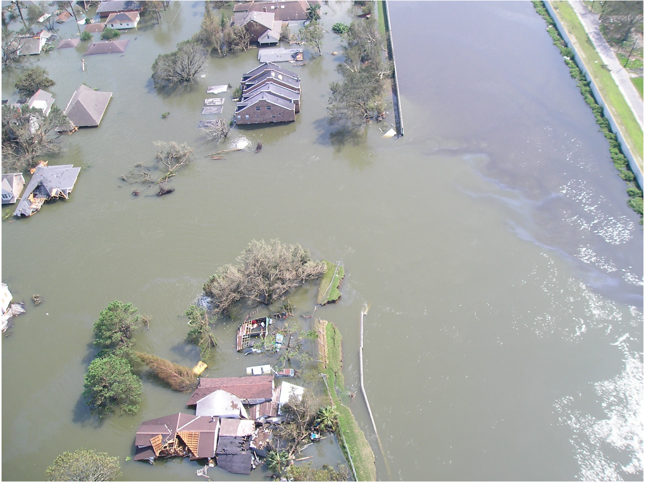
Figure VI-3. Aerial photograph of the 17th Street Canal breach showing I-wall and embankment translation
