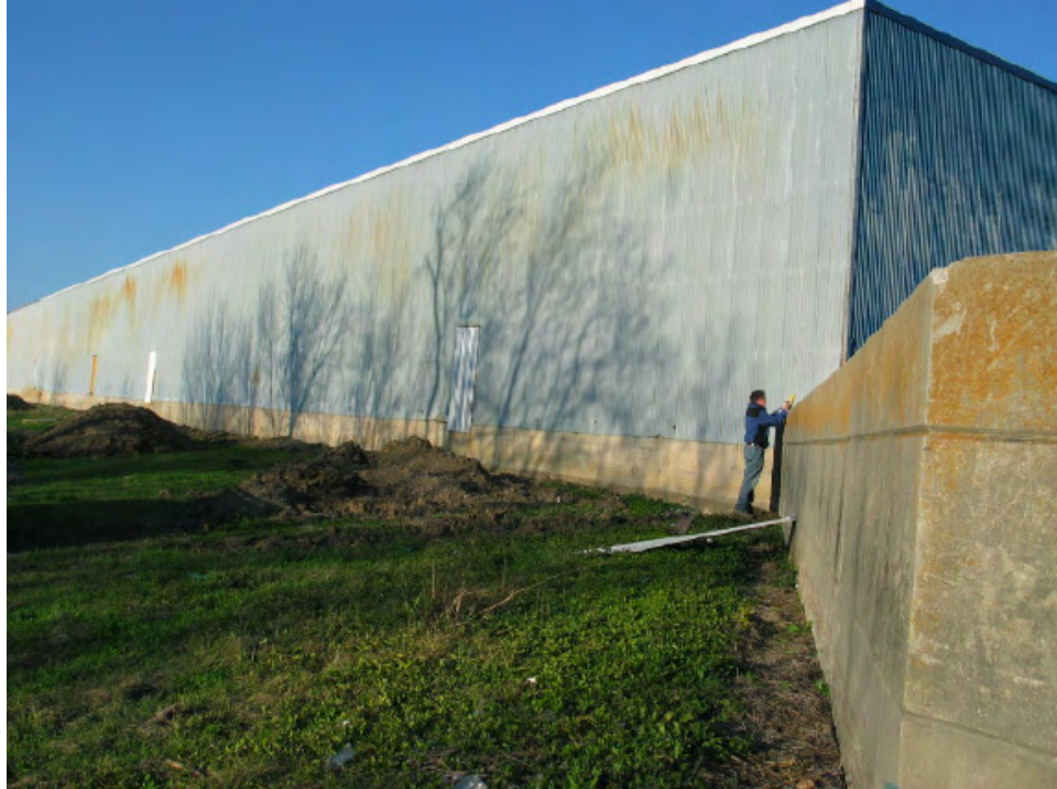
Figure J-B13. Floodwall Serves as Building Foundation (Dupuy Storage Facility – IHNC East)
