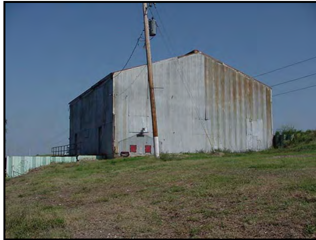
Pre-Hurricane Katrina - View to the North
