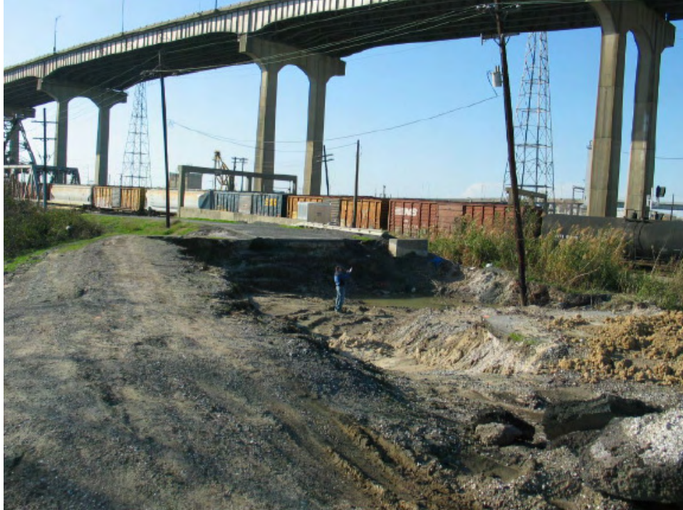
Figure J-B12. Major Washout Area from Overtopping Near I-10 Overpass (Citrus Back Levee)
