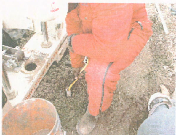
Photo 10 - Small Hydrophone receiver on tape in 1 inch PVC casing installed by Geoprobe Rig at IHNC
