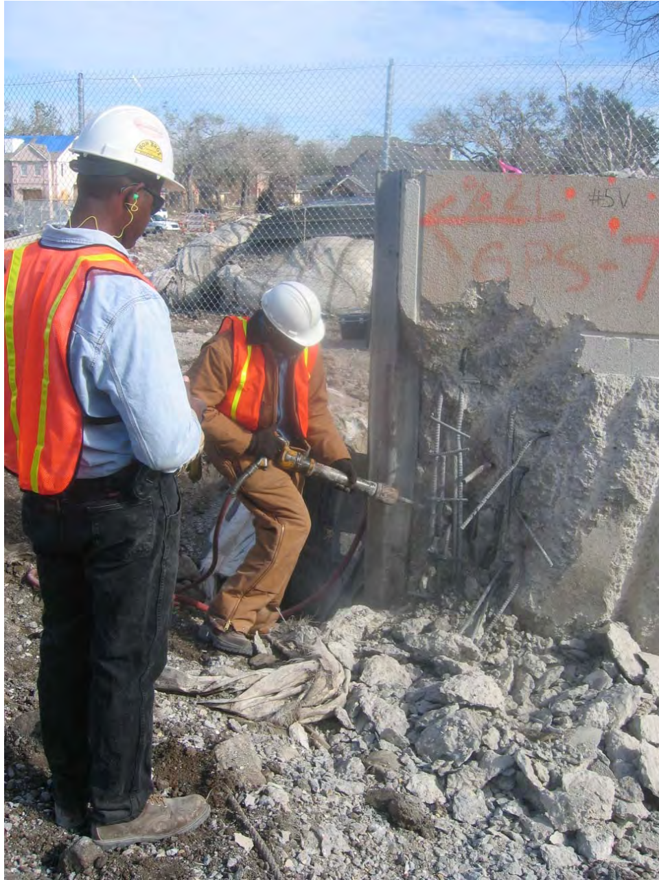
Figure K4-13. Demolition of concrete around rebar sample at panel H38
