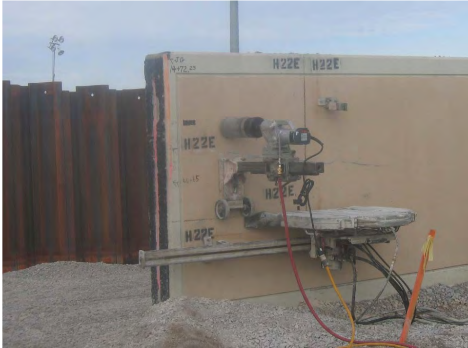
Figure K4-8. Core drill and saw mounted at panel H22
