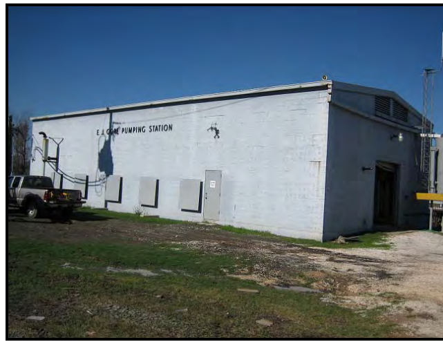
Post-Hurricane Katrina – View to the North
