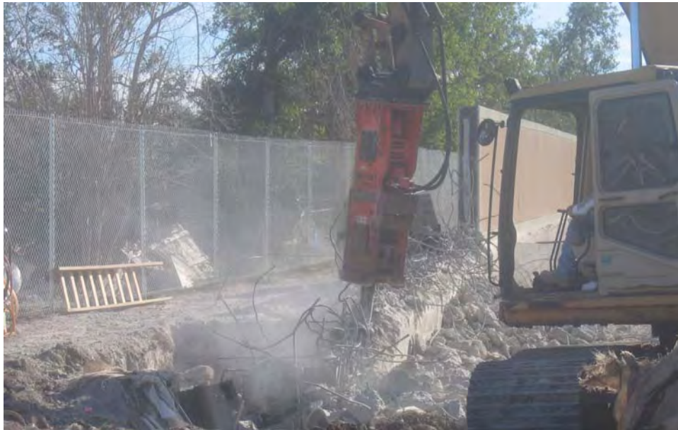
Figure K4-18. Hoe ram demolishing lower portion of wall panel H38
