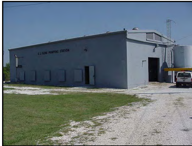
Pre-Hurricane Katrina – View to the North
