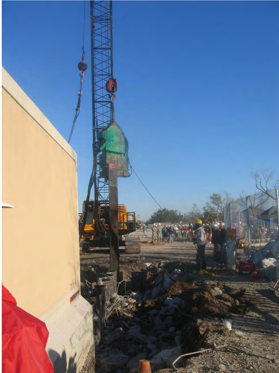
Figure K4-20. Extraction of sheet piles MH38SP2 and MH38SP3
