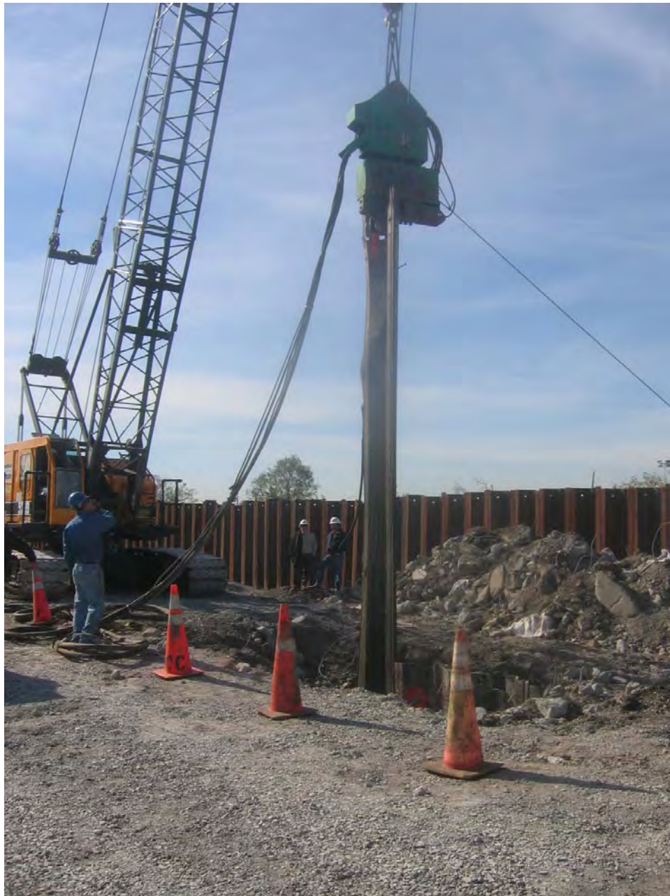
Figure K4-23. Extraction of sheet piling MH22SP1 and MH22SP2
