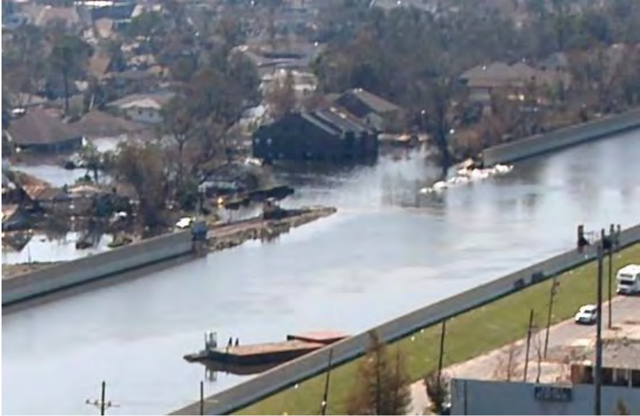
Figure K4-1. 17th Street canal breach
