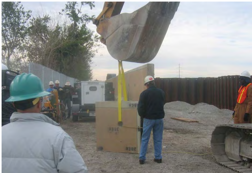
Figure K4-7. Removal of sample from wall panel H38
