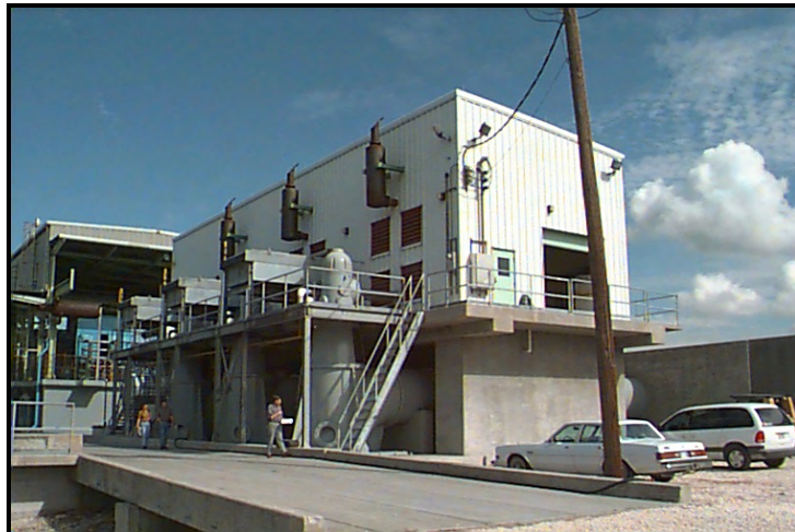
Post-Hurricane Katrina – View from the Inlet Canal
