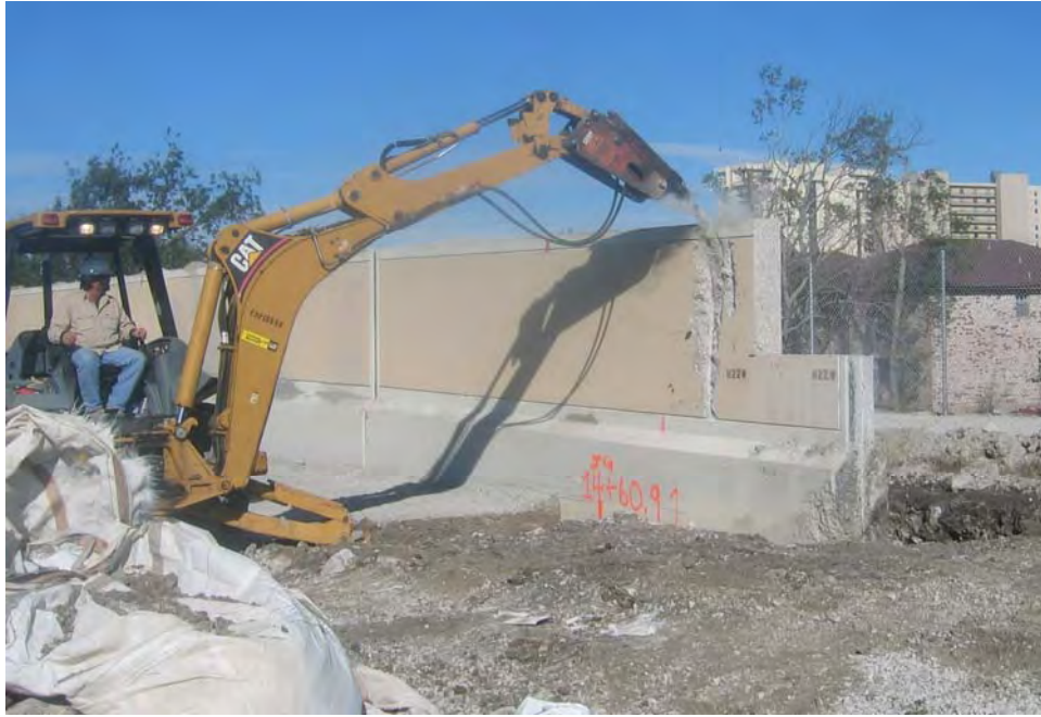
Figure K4-12. Demolition of concrete for rebar sampling at panel H22
