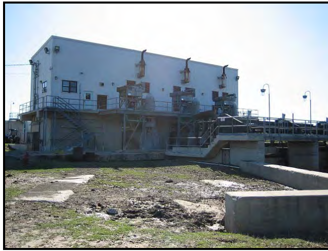
Post-Hurricane Katrina – View from the Inlet Canal
