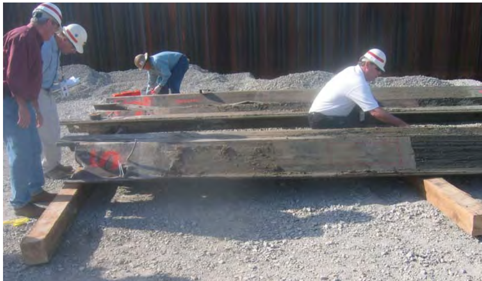
Figure K4-25. Sheet piling extracted from north end of breach
