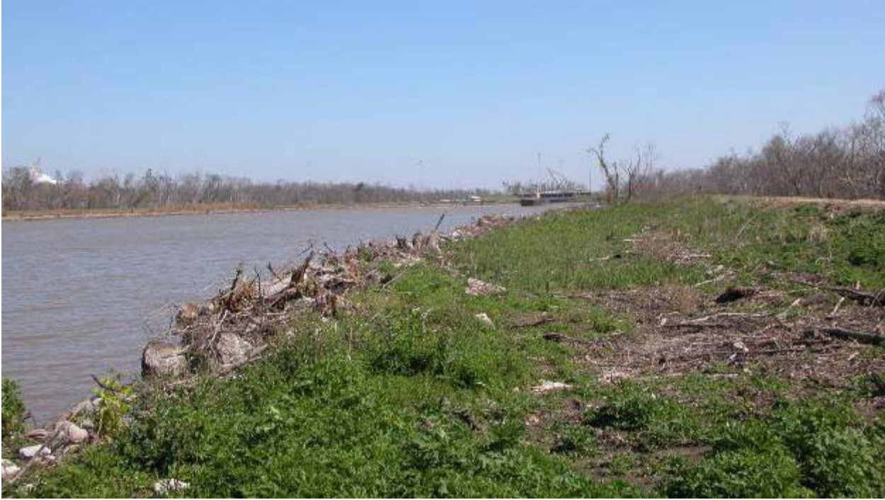
Typical Algiers Canal levee; no armor
