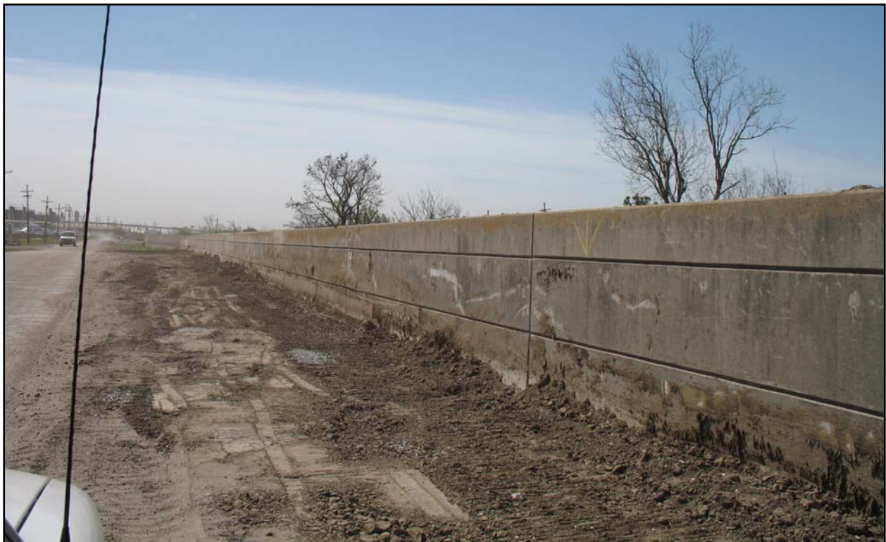
Repair to Scour Along Floodwall.
