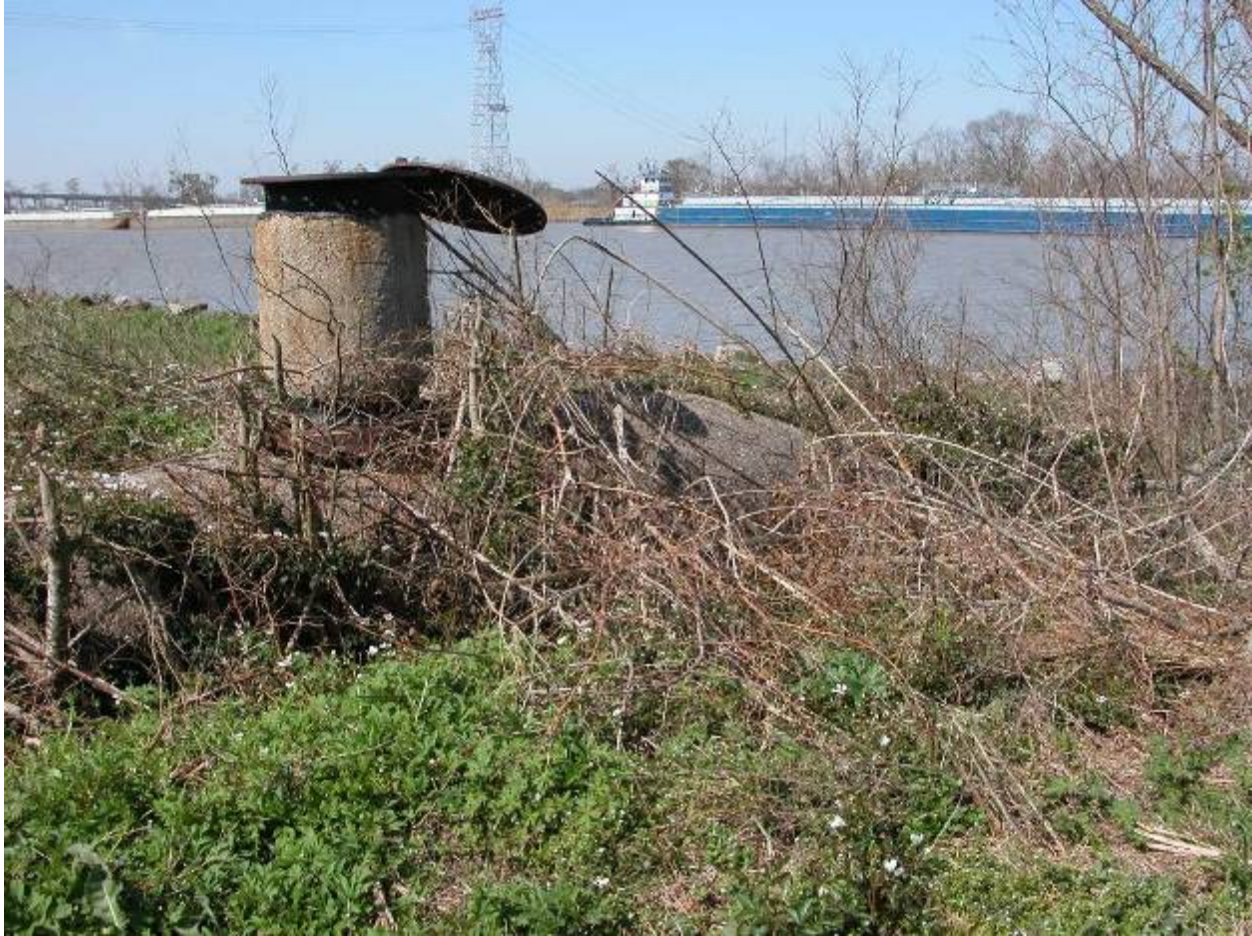
Abandoned pipe crossing through the Algiers Canal
