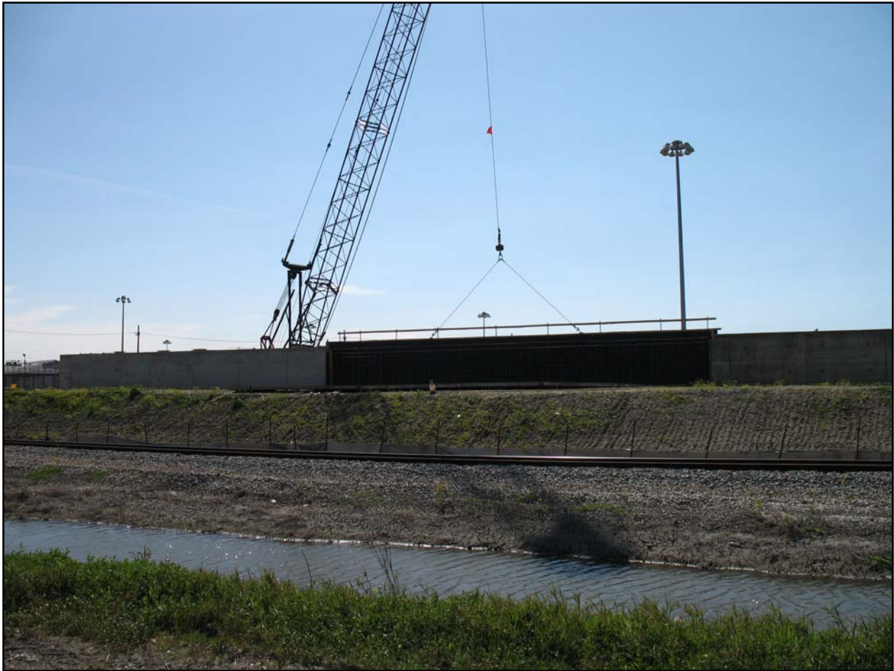
Repairs Along the IHNC Where The Floodwall Breached Levee Section.
