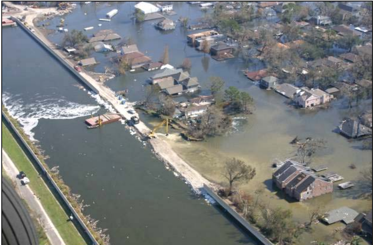
Figure 1. Breach in the 17th Street Canal
