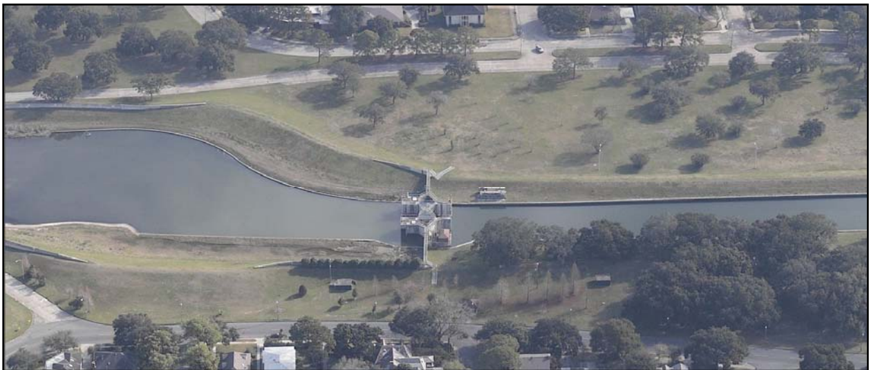
Protection Gate Structure at Bayou St. John
