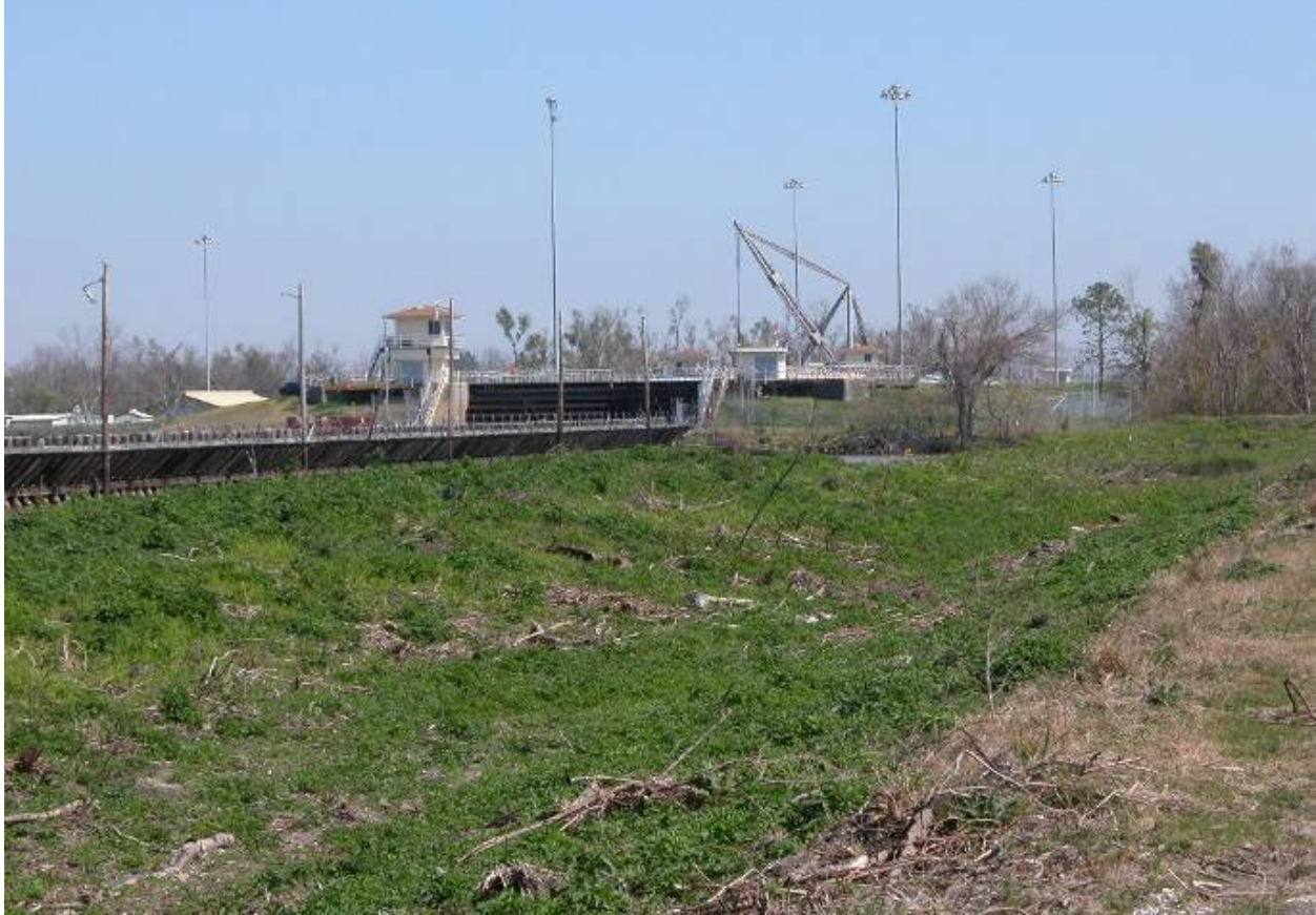
South end of Algiers Lock
