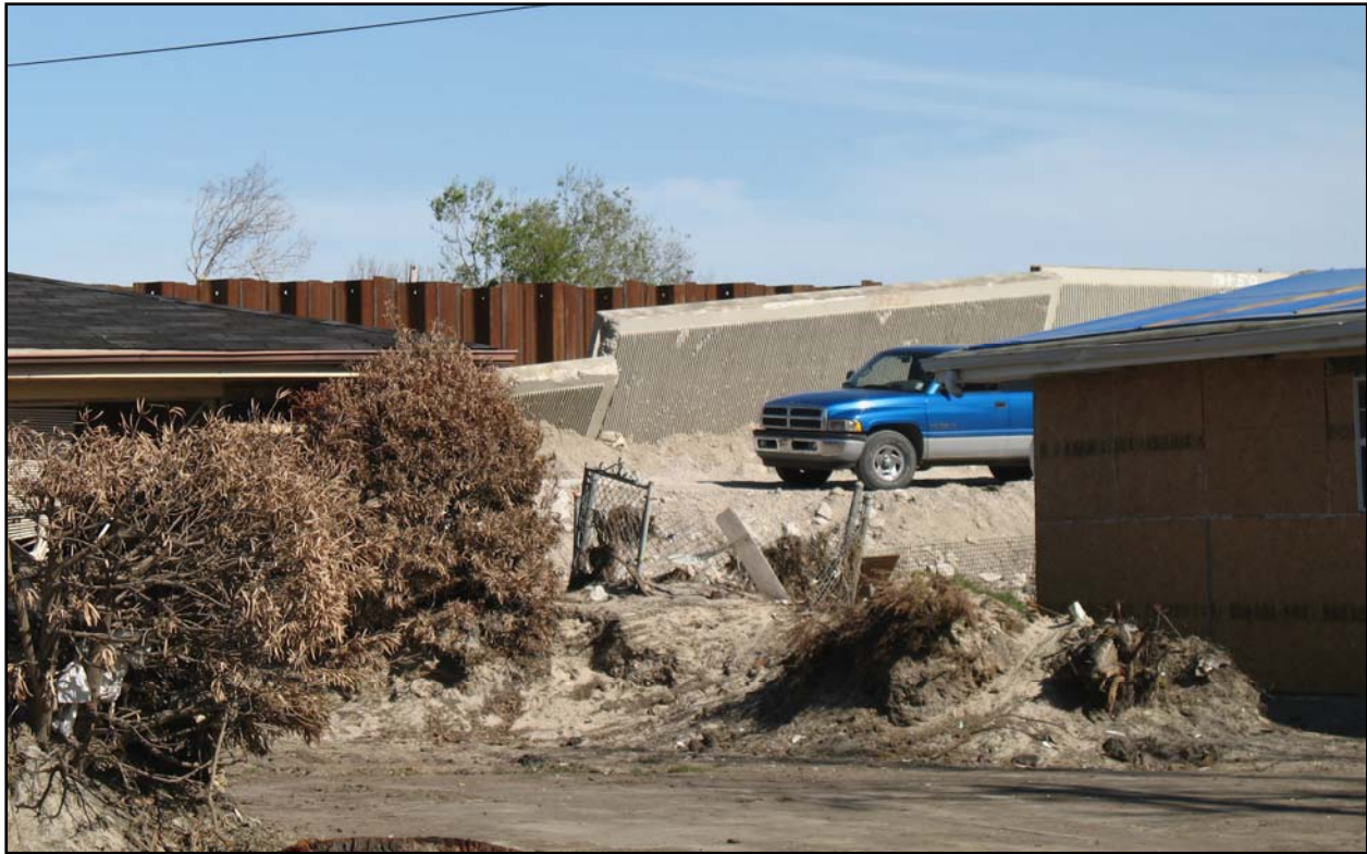
Figure 4. Sheetpile repair along the London Ave Canal – West Side Failure
