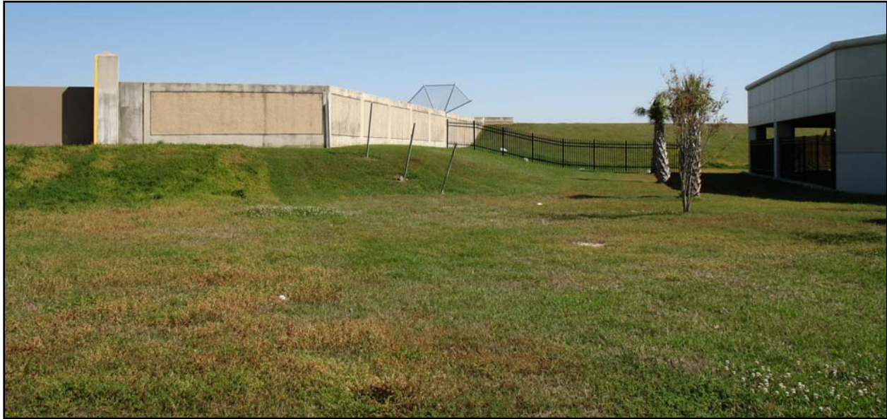
Figure 5. Floodwall and Levee behind the University of New Orleans
