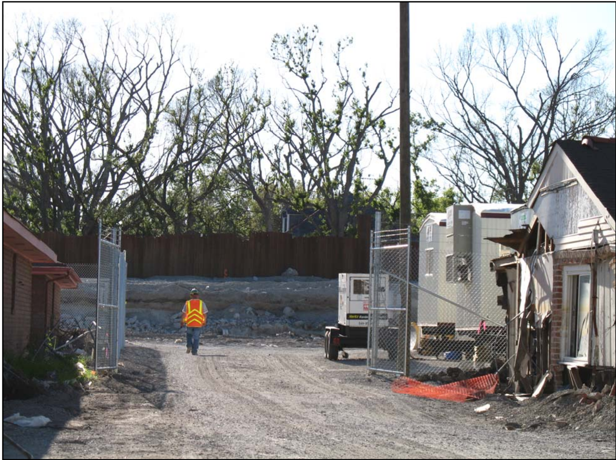
Figure 3. Sheetpile repair along the London Ave Canal – East Side Failure
