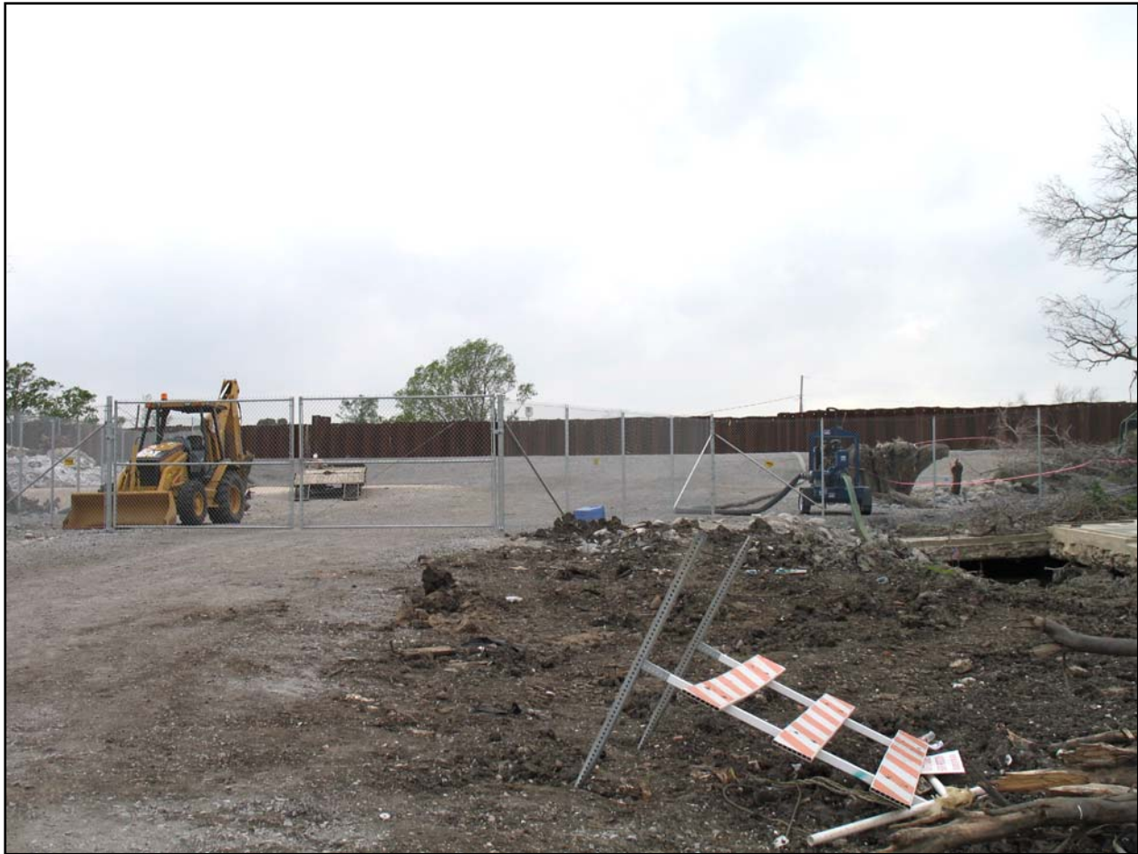
Figure 2. Sheetpile repair along the 17th Street Canal
