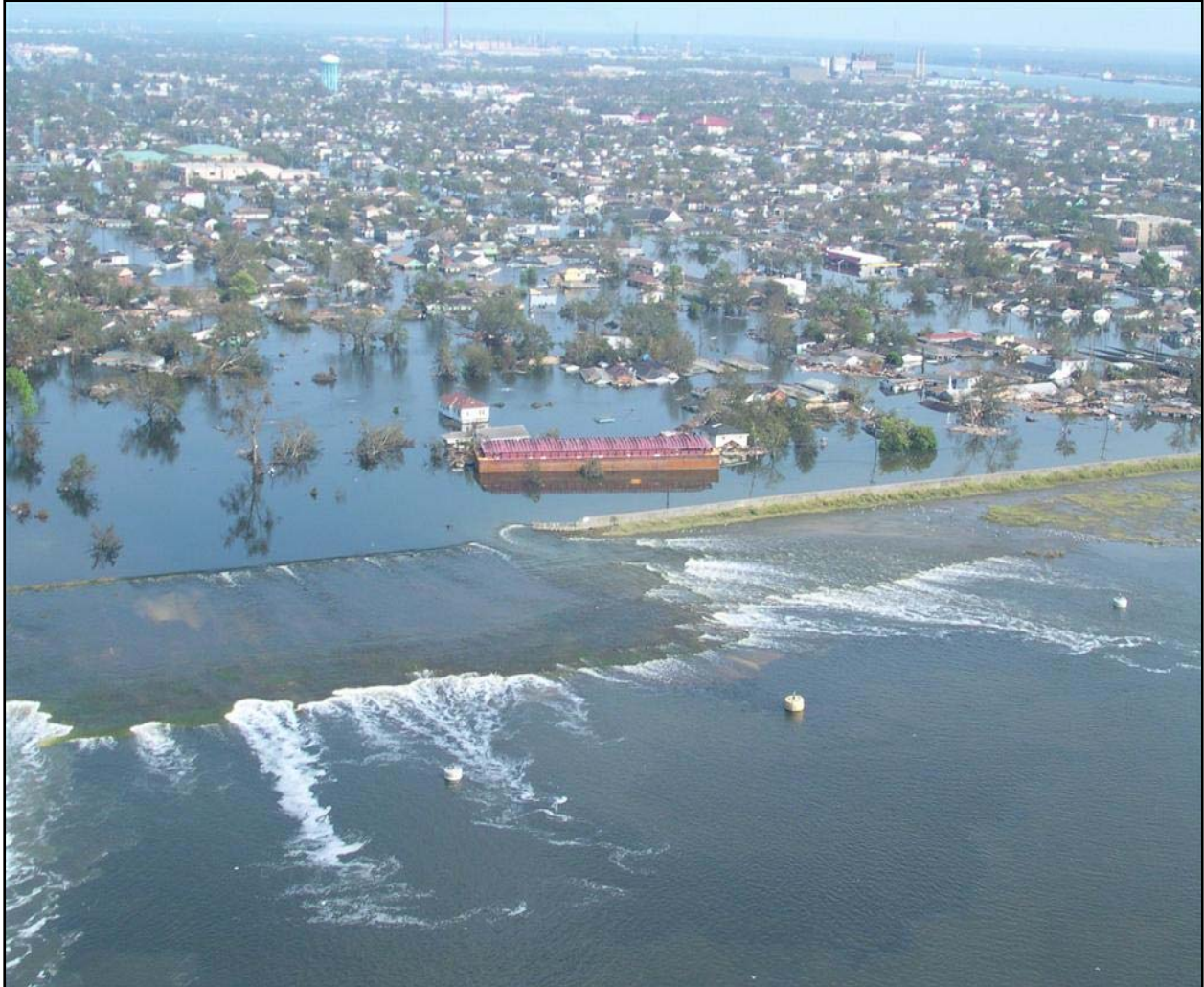
Figure V-17-36. Aerial view of the south breach at east bank of the IHNC (at the west end of the Lower Ninth Ward), showing turbulent water flow coming out of the Lower Ninth Ward after the hurricane passed
