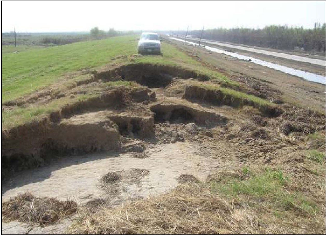
Figure 20. Stage C breach along Plaquemines Parish levee
