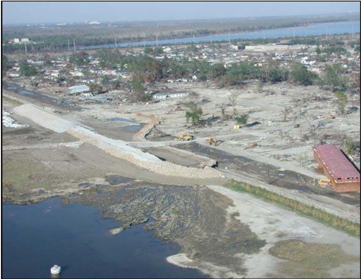
Figure V-17-35. Aerial view of the south breach at east bank of the IHNC (at the west end of the Lower Ninth Ward), showing in crevasse splay generated by reverse drainage flow. (Figure 6.45, NSF-Berkeley report (ILIT Final Report, July 31, 2006)
