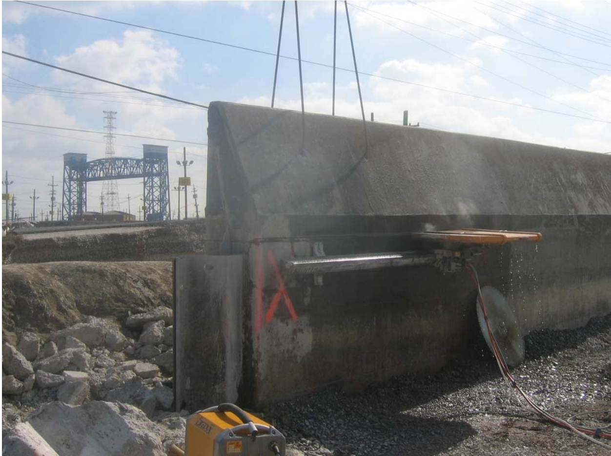
Figure 16-1. Sawcutting Concrete Wall Sample
