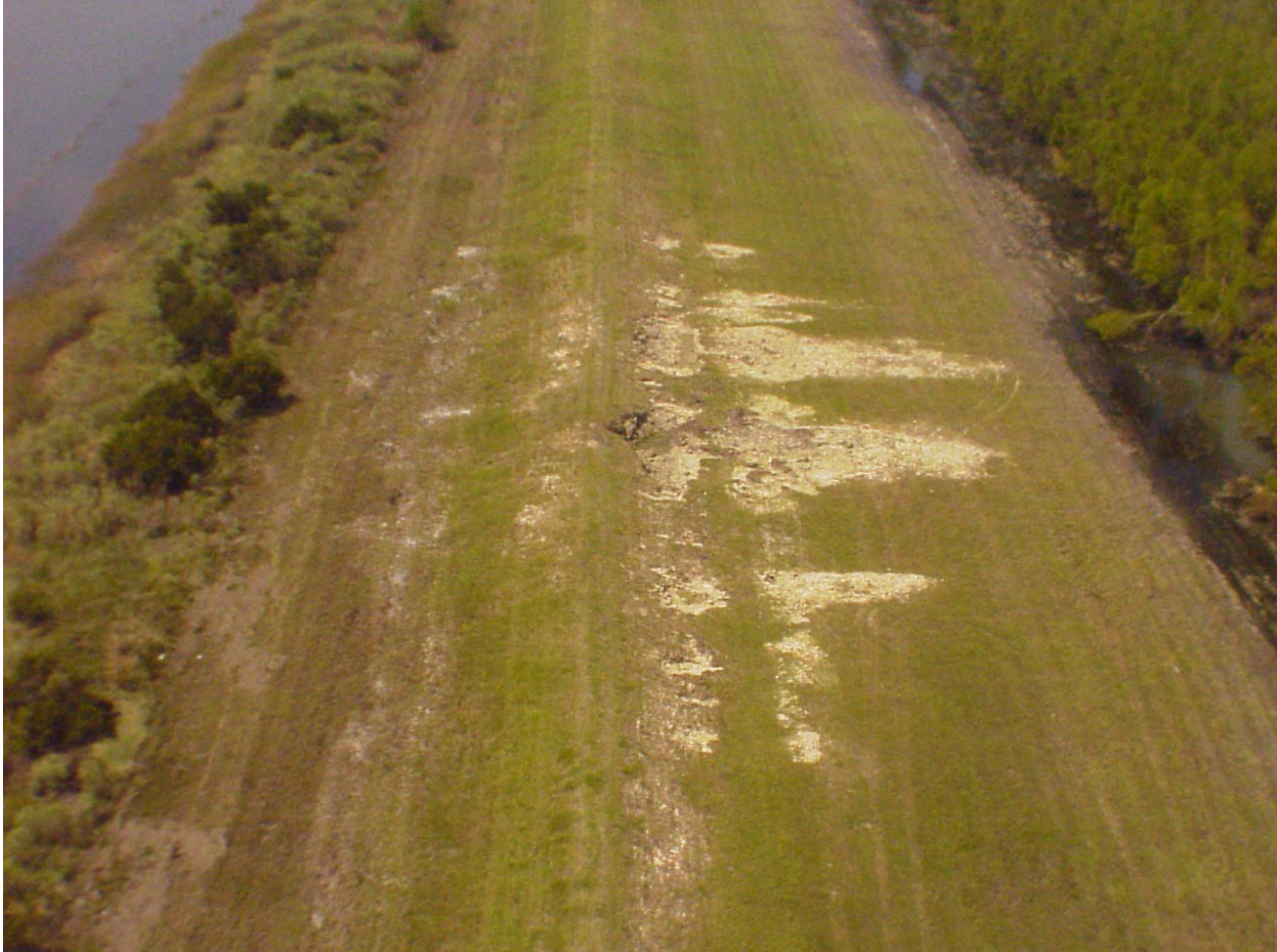
Figure 6. 600' reach of levee along the north bank of the GIWW (Citrus Back Levee, New Orleans East) between Elaine Pump Station and Paris Road.
