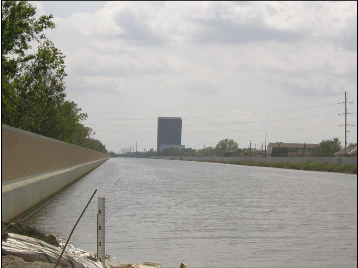
Figure 26. View of the 17th Street Canal looking south toward Veterans Avenue. Note the Orleans Parish side (left) of the canal has no embankment section above the water level, while the Jefferson Parish side (right) has an exposed embankment section. Approximately 20 measurements were made from top of wall in a southerly direction from the breach on the Orleans Parish side with a weighted tape measure to determine the water depth to the top of the embankment. These measurements indicate the water level was approximately 1 ft deep on the canal side adjacent to the I-wall.
