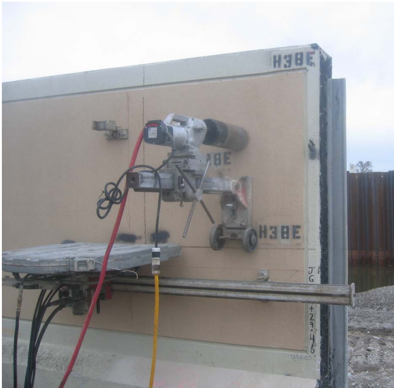
Figure 15-3. Core Drill and Saw Mounted to Wall Panel H38
