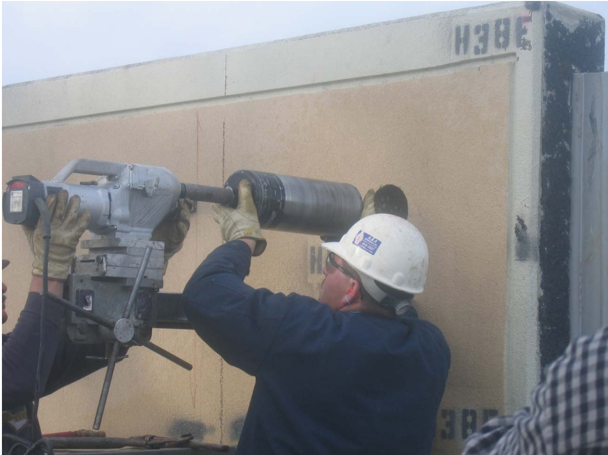
Figure 15-4. Core Being Removed from Panel H38
