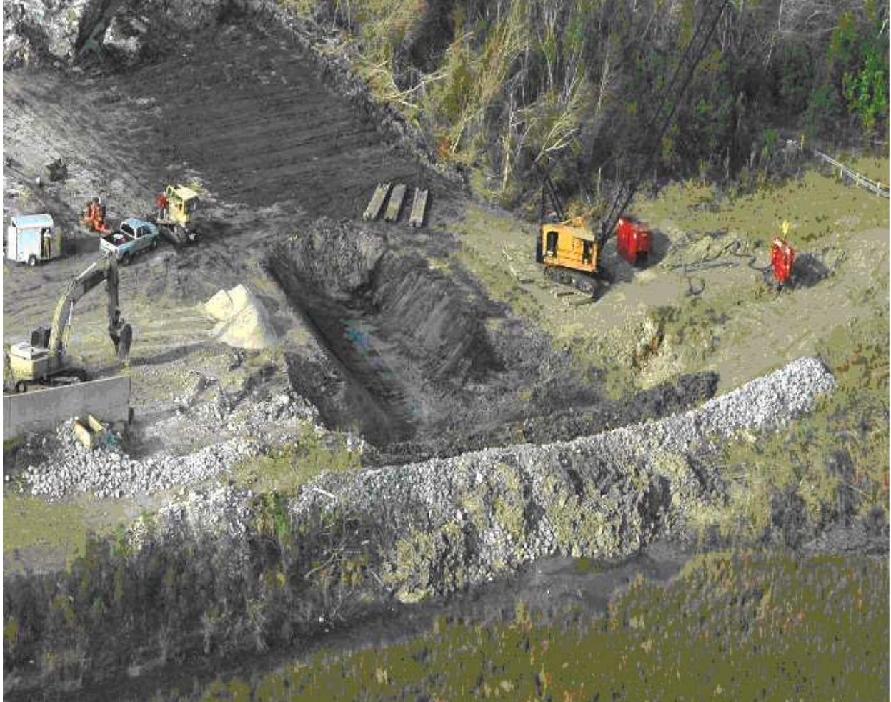
Figure 12-49. NOE3_I. Repair Progress
