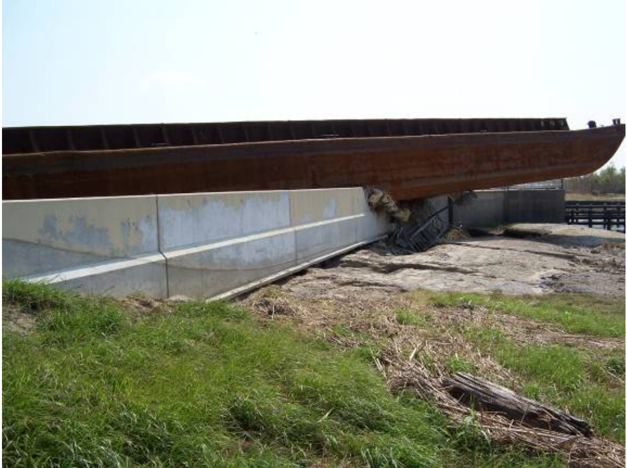
Figure 14-111. View East, From Protected Side
