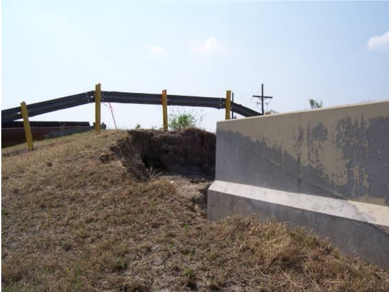
Figure 13-73. Floodgate S5 Near Bienvenue Control Structure
