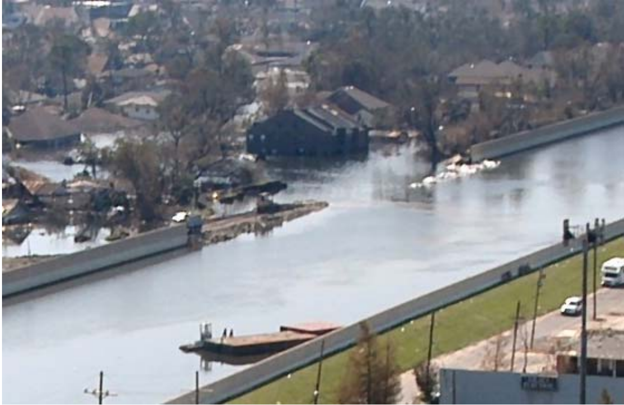
Figure 15-1. 17th Street Canal Breach
