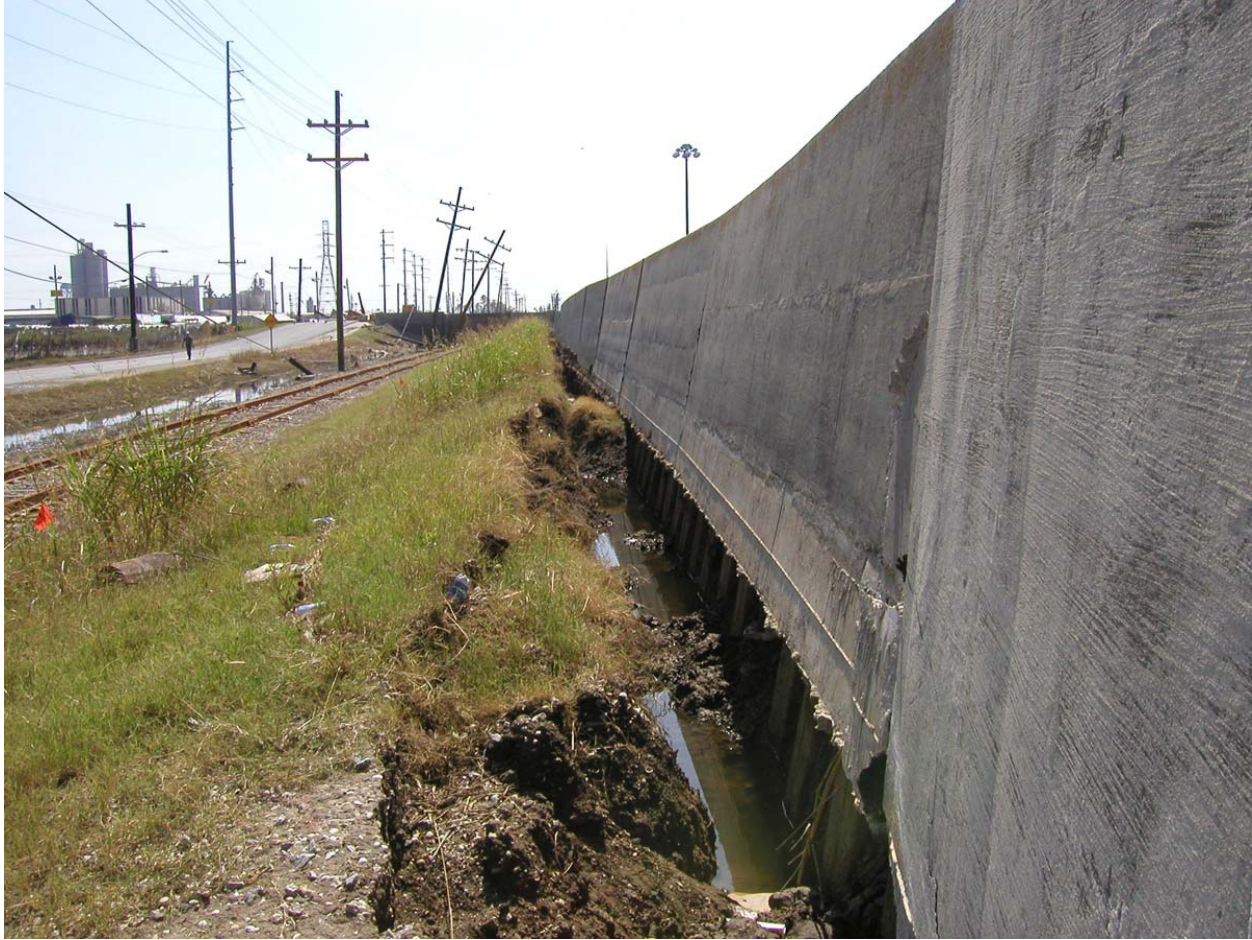
Figure 14-60. View South From Benefit St. Gate Toward France Rd Ramp. Approximate W/L Sta 5+56 (B/L Sta 205+44). Top of I-wall elevation 15 ft, levee crown 9 ft, bottom of concrete 7 ft, bottom of pre-existing Z-27 sheet pile (by Orleans Levee Board) at -10ft (MSL). From drawing file H-2-24111, plate IV-15. Nearest soil boring is 30W at B/L Sta 203+00
