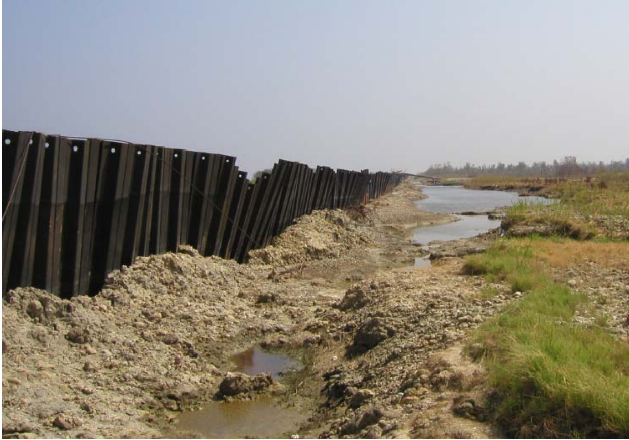
Figure 14-123. Note Sheetpile Elevation Differences
