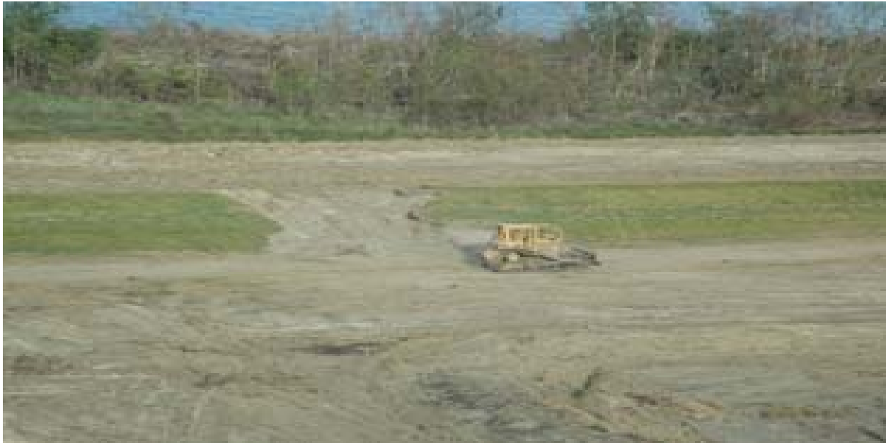
Figure 14-130. Repairs Underway, Filling Scour Holes
