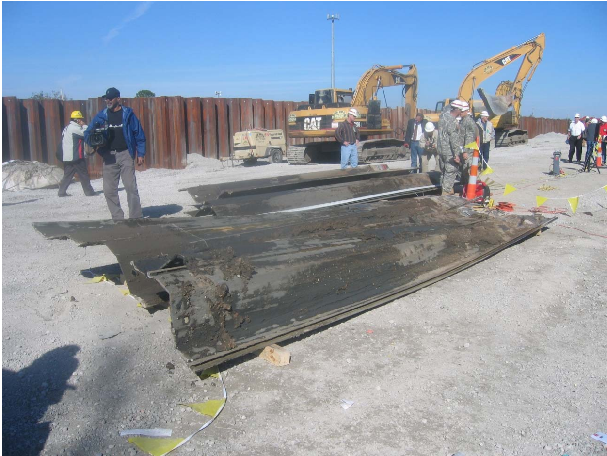
Figure 15-24. Sheet Piling Extracted from South End of Breach
