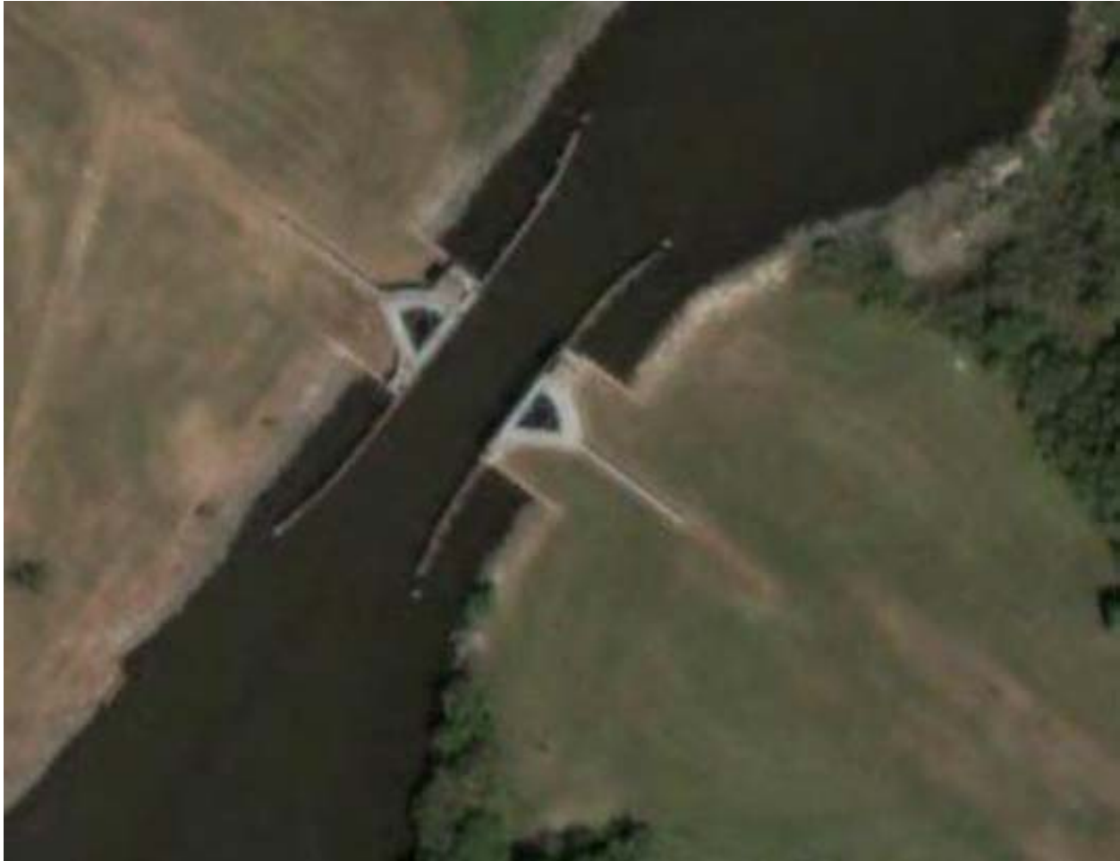
Figure 14-138. Bayou Dupre Control Structure, Pre-Katrina View. Note the concrete walls transitioning to earth levee on both sides of the structure
