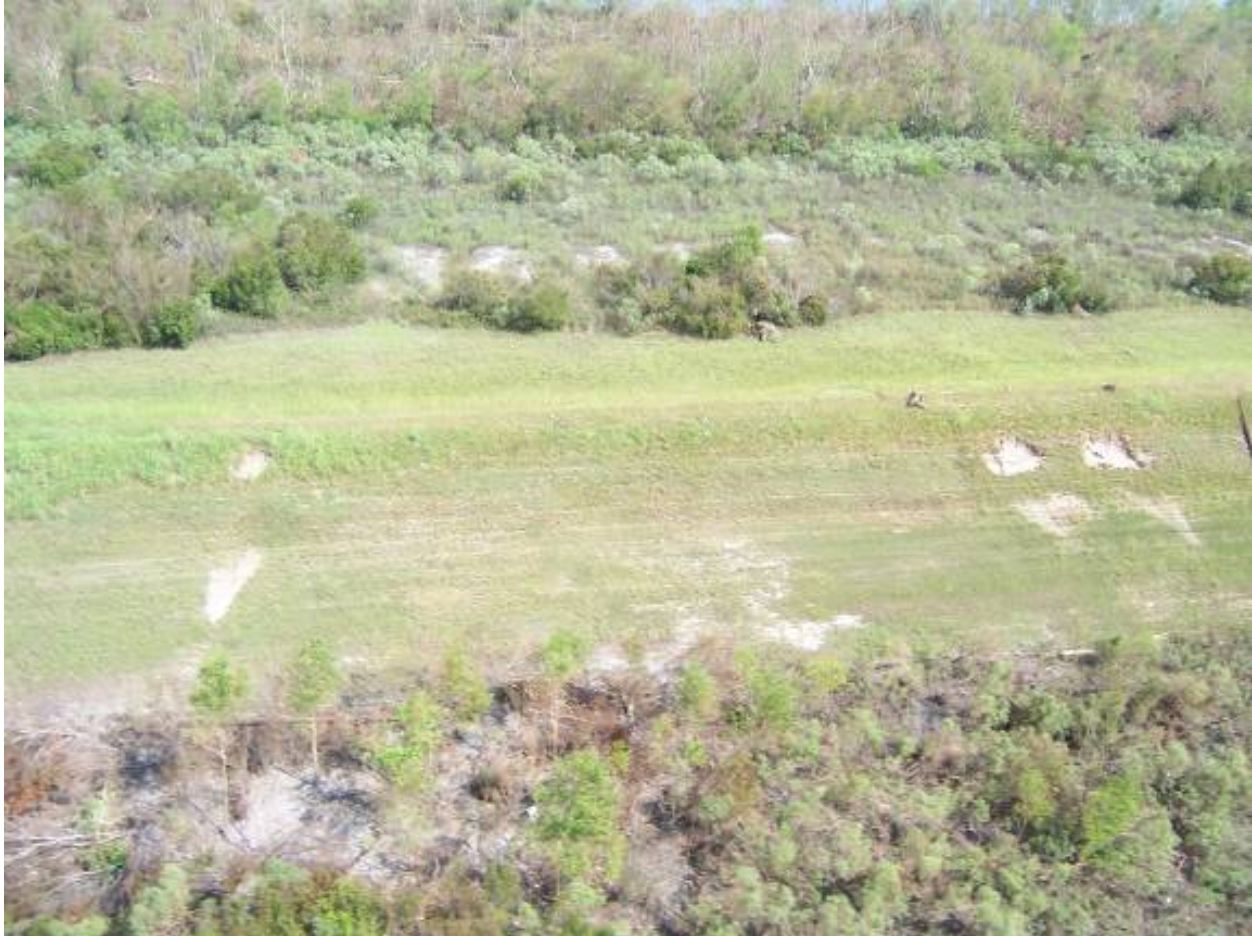
Figure 13-46. Scour on the Backside of the South Bank GIWW Levee Between STA. 65+008 and STA. 277+20, St. Bernard Parish, Minor Scour on the Protected Side Levee Transition Slope. The Paris Rd (I-510) high rise bridge is over approximate B/L Sta 270+00
