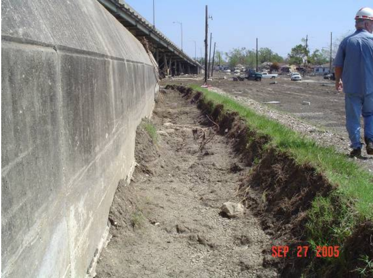
Figure 14-49. East Side IHNC Near N. Claiborne Ave, Approximate B/L Sta 11+00. I-wall elevation designed 15 ft (MSL), bottom of concrete elevation 7 ft (MSL), and levee crown elevation 9 ft (MSL). Nearest soil boring, No. 3, shows fat clay (CH) at surface
