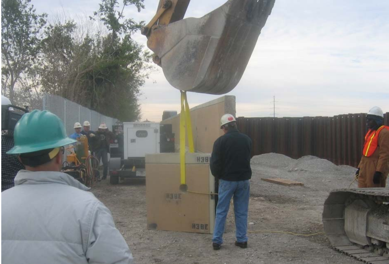
Figure 15-7. Removal of Sample from Wall Panel H38
