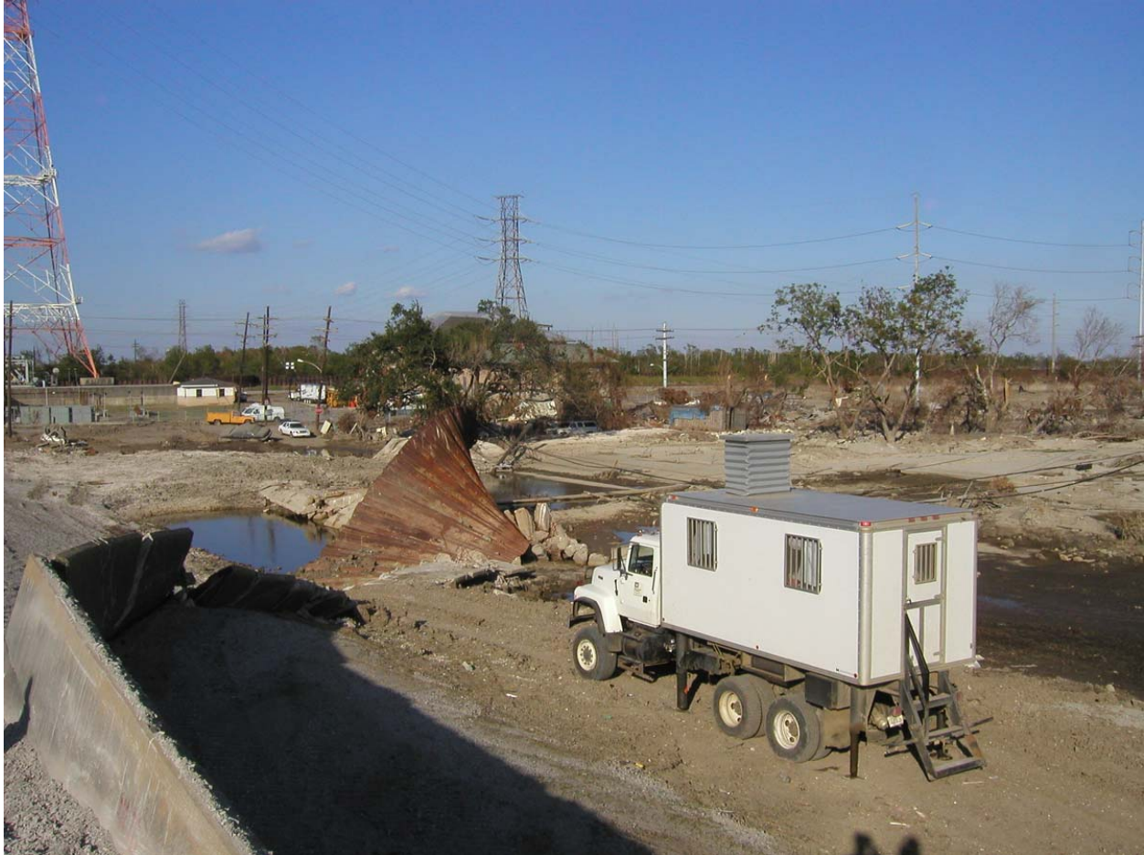
Figure 14-31. CPT Truck at Levee Toe on Protected Side at the Southernmost I-Wall Failure Transition Between Florida Ave and Claiborne Ave., View Toward Pump Station
