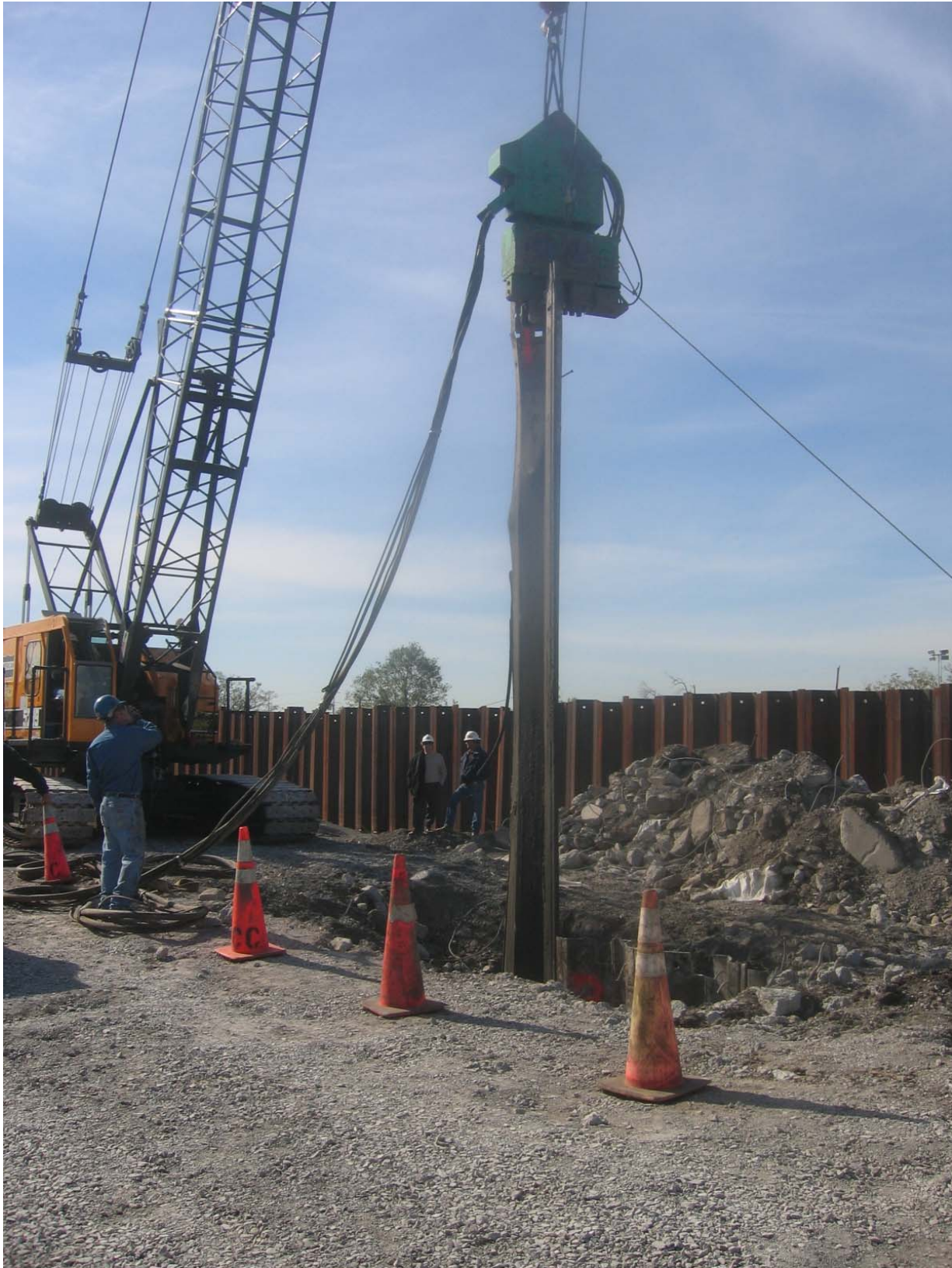
Figure 15-23. Extraction of Sheet Piling MH22SP1 and MH22SP2
