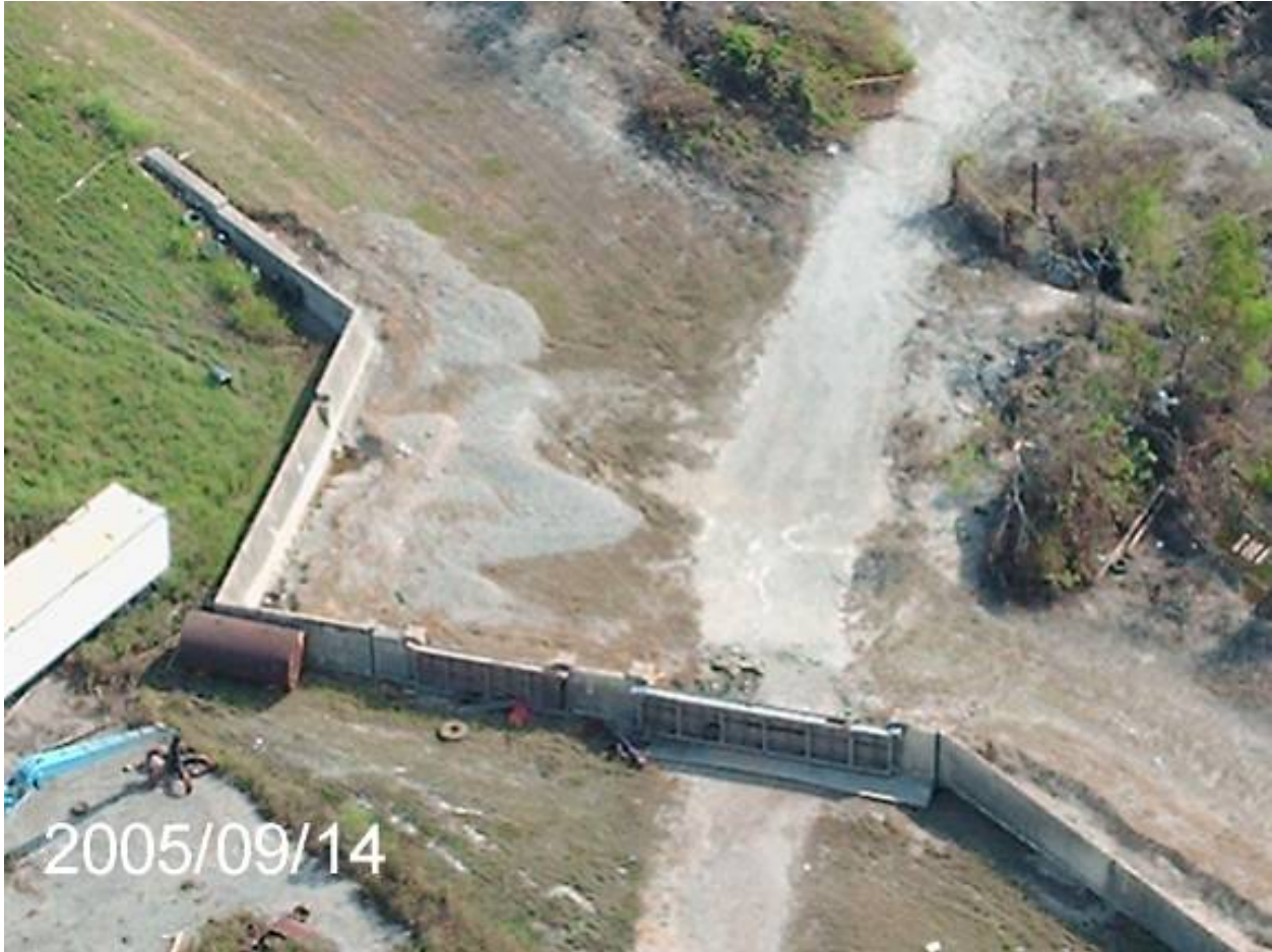
Figure 13-70. Southern Scrap Facility Gates S2 and S3
