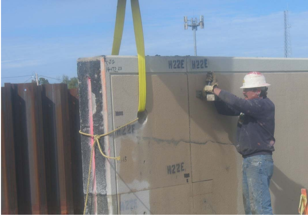
Figure 15-9. Sample Being Removed from Wall Panel H22
