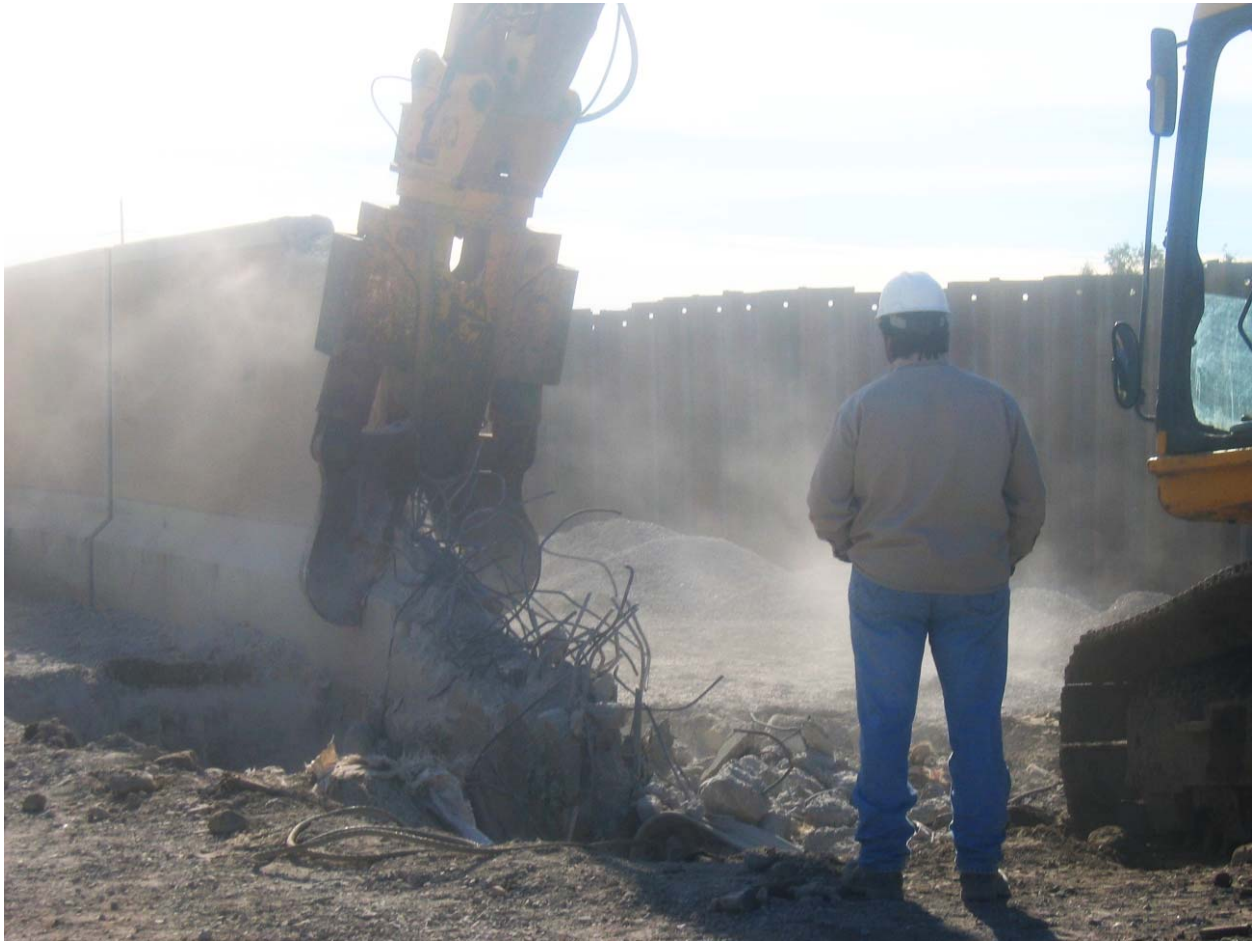
Figure 15-17. Demolition of Top Portion of Wall Panel H38
