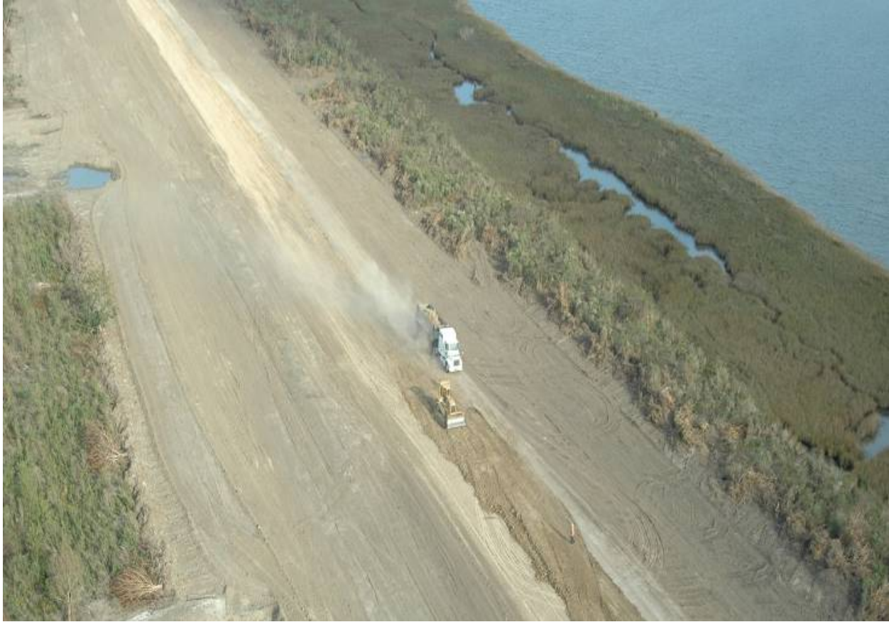
Figure 12-39. NOE1_F Rebuilding to Initial Elevation 10'
