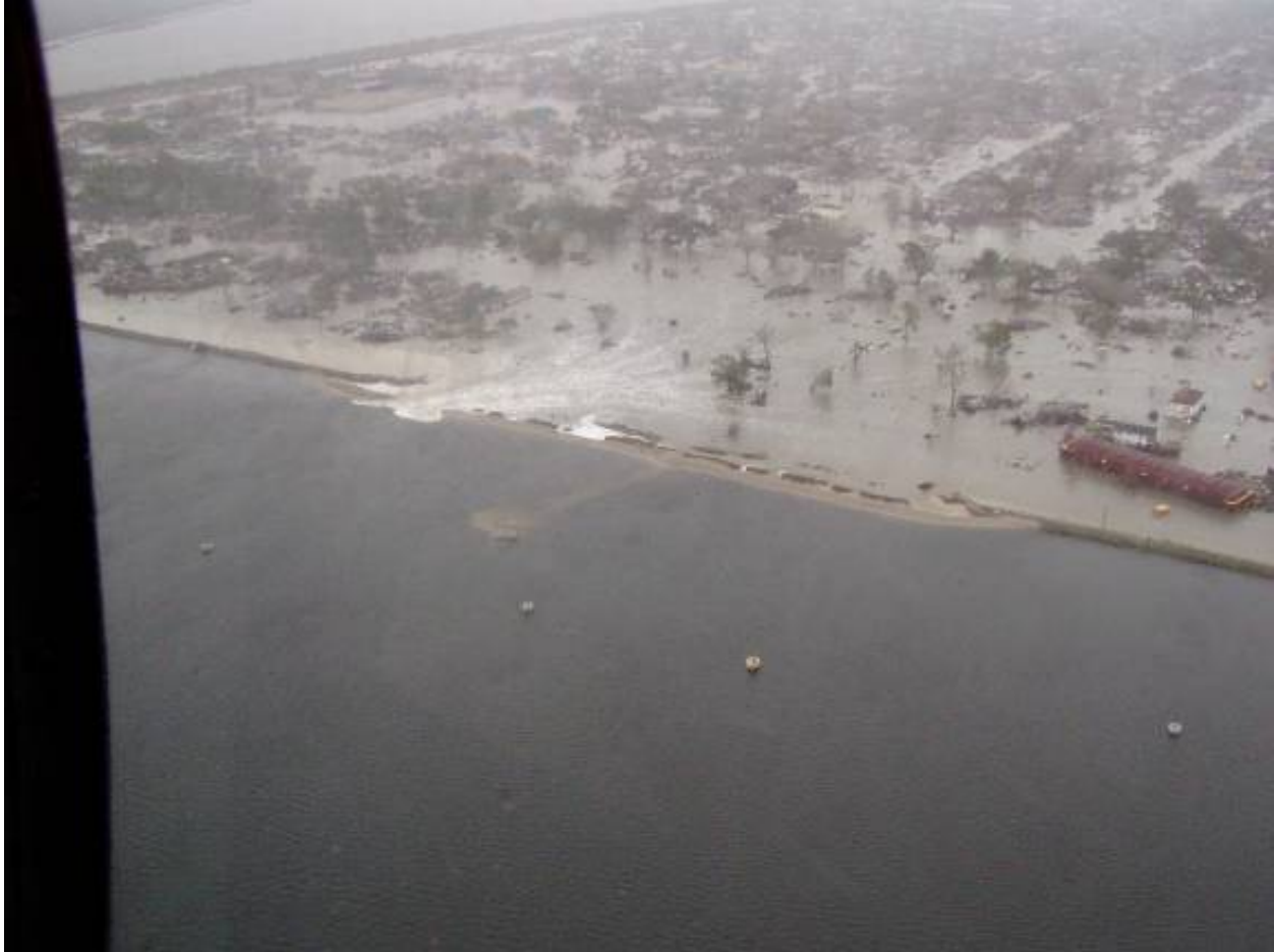
Figure 14-23. During Katrina; View to East Side of IHNC South of GIWW. Breach began approximately 300 ft north of Claiborne Ave.
