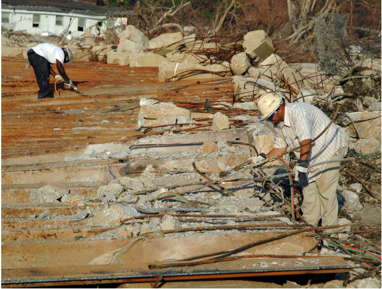
Figure 14-27. Demolishing Flattened I-Wall North of Claiborne Ave.
