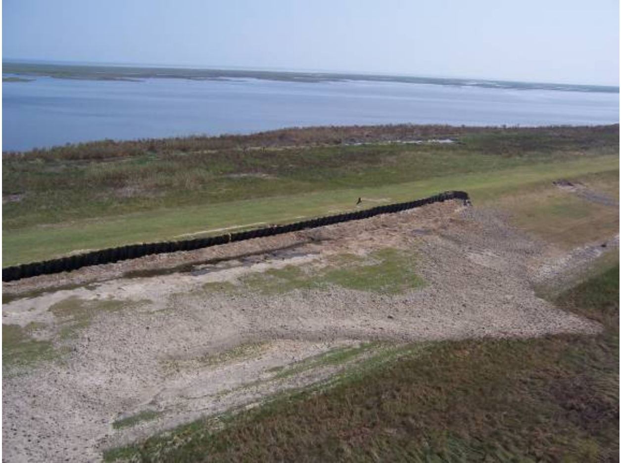
Figure 14-151. End of Sheetpile Wall at B/L Sta 980+58
