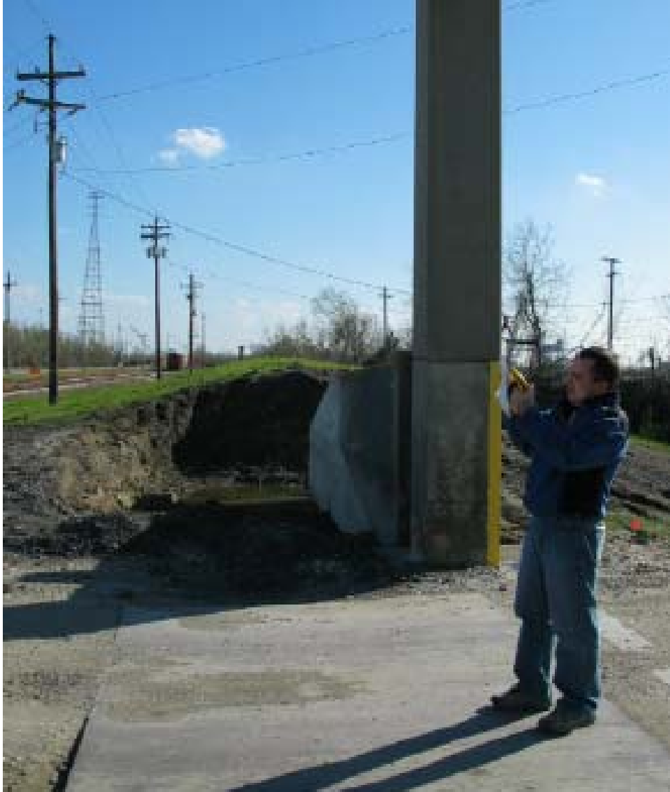
Figure 13-75. IHNC Floodgate E5 Transition to Levee
