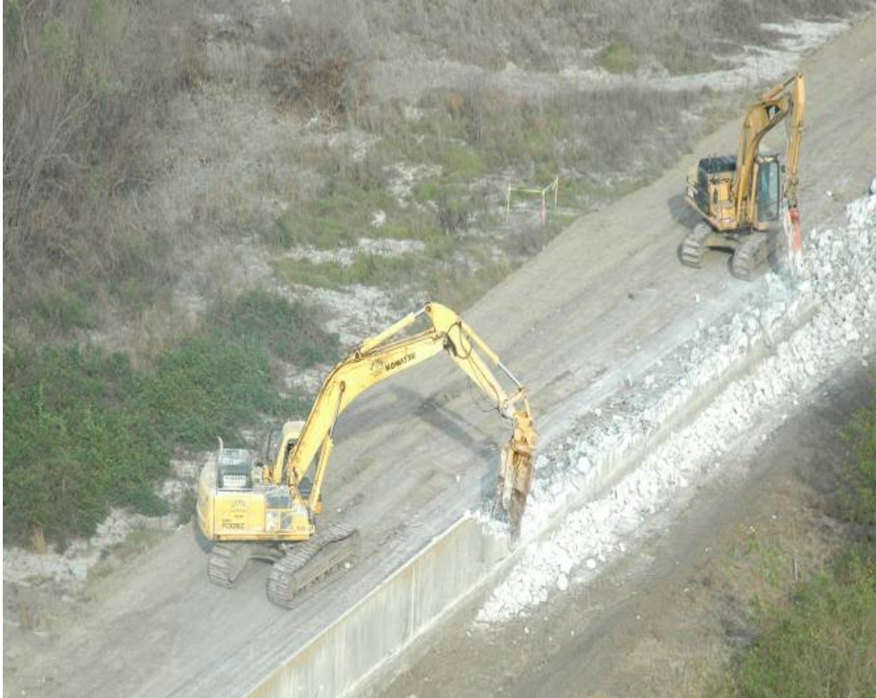
Figure 12-62. NOE4_I. I-Wall Demolition to Replace with New “L” Wall
