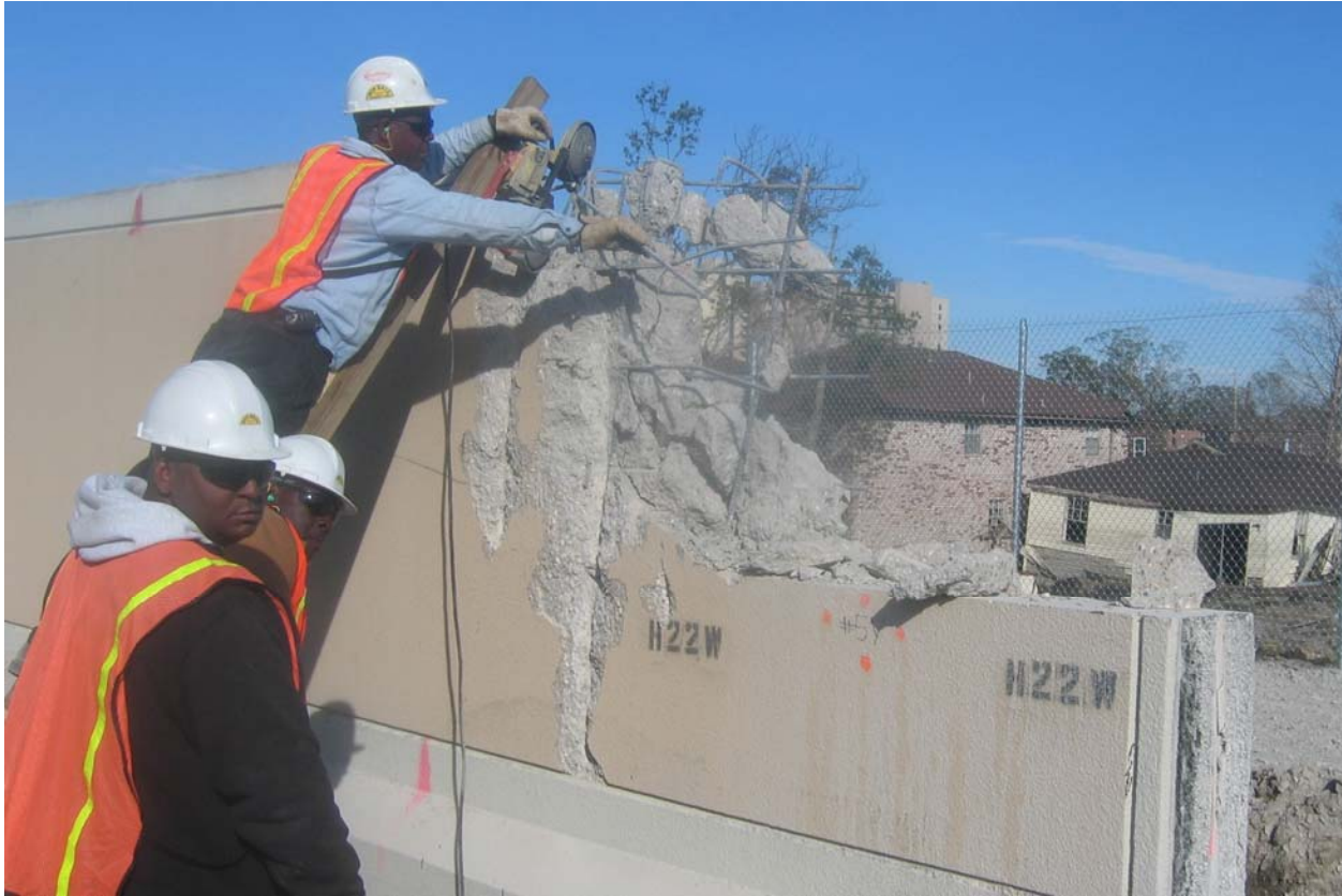
Figure 15-14. A Portable Electric Bandsaw is Used to Cut Rebar Samples
