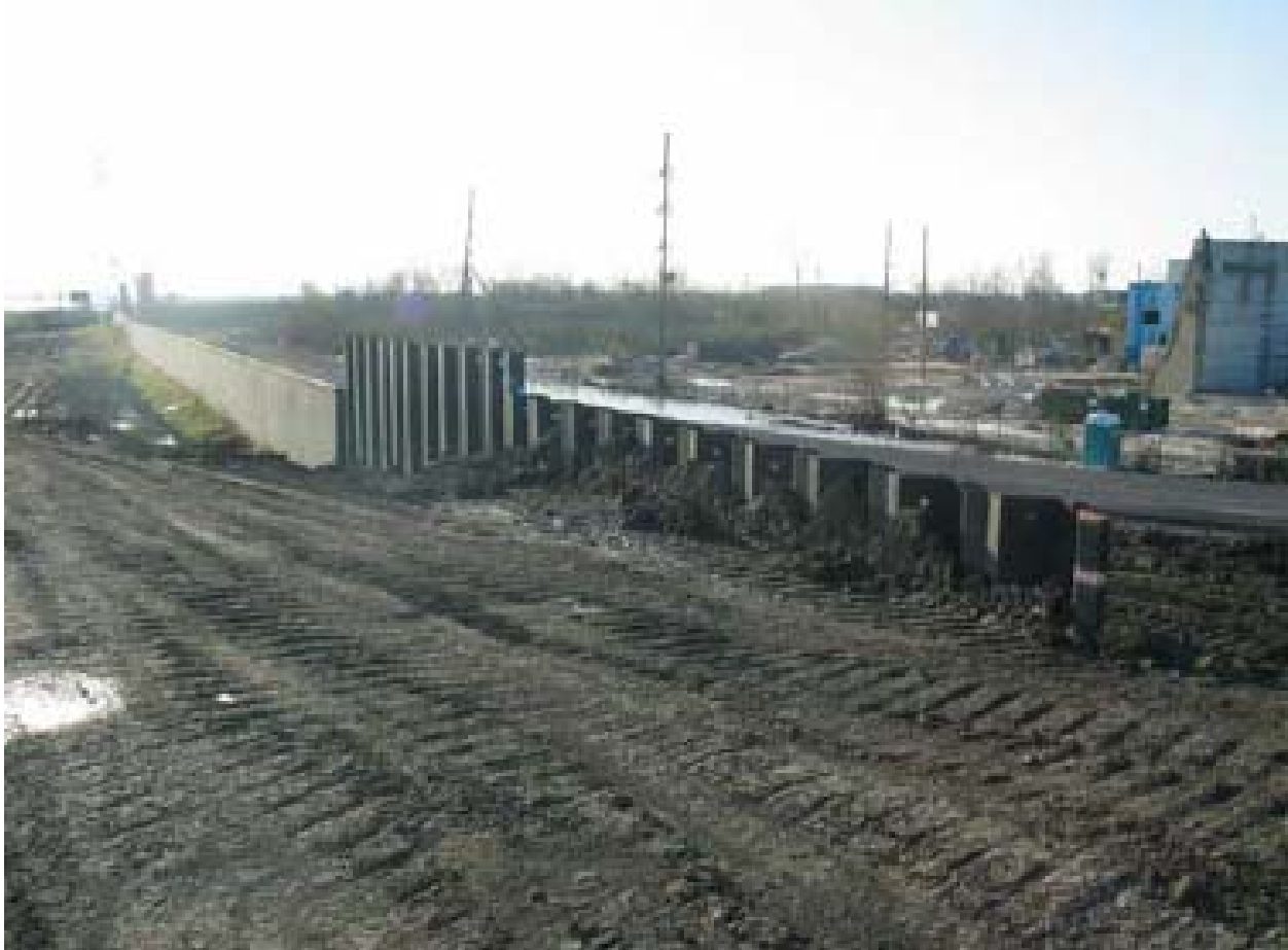
Figure 12-50. NOE3_J. Repair Sheetpile View to the West
