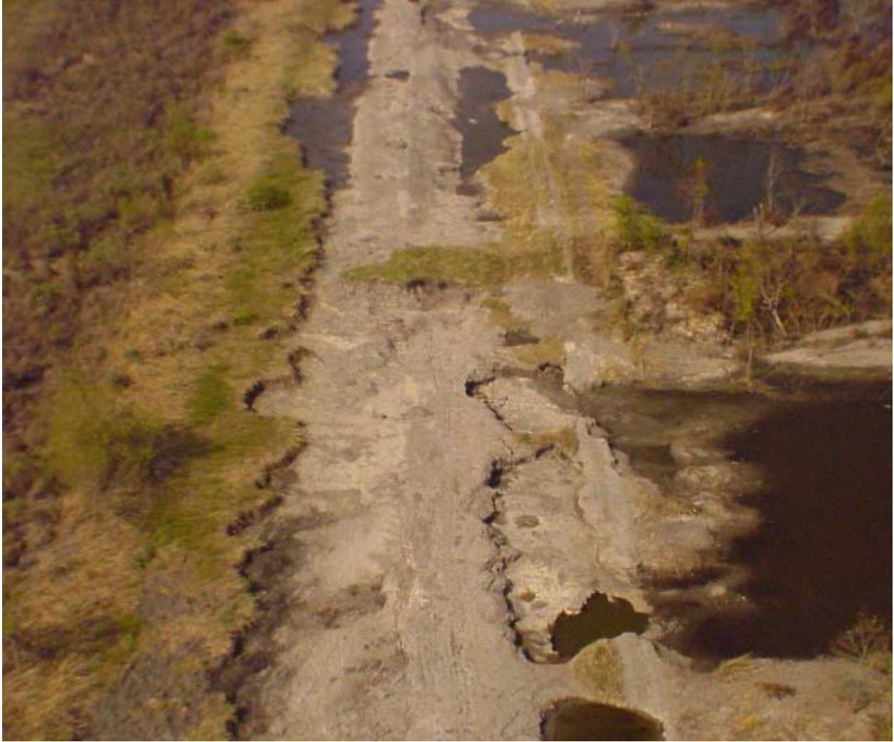
Figure 13-60. East of Pump Station 15 (N.O. East Back Levee), North Bank of GIWW. 12,750 feet of levee east of Pump Station #15 was completely degraded (Station 876+87 B/L to 1101+90 B/L). West of the pump station, 9,800 feet of levee was completely degraded (approx Sta 778+00 to 876+00). The levees in these reaches were constructed from GIWW hydraulic fill in stages over three years
