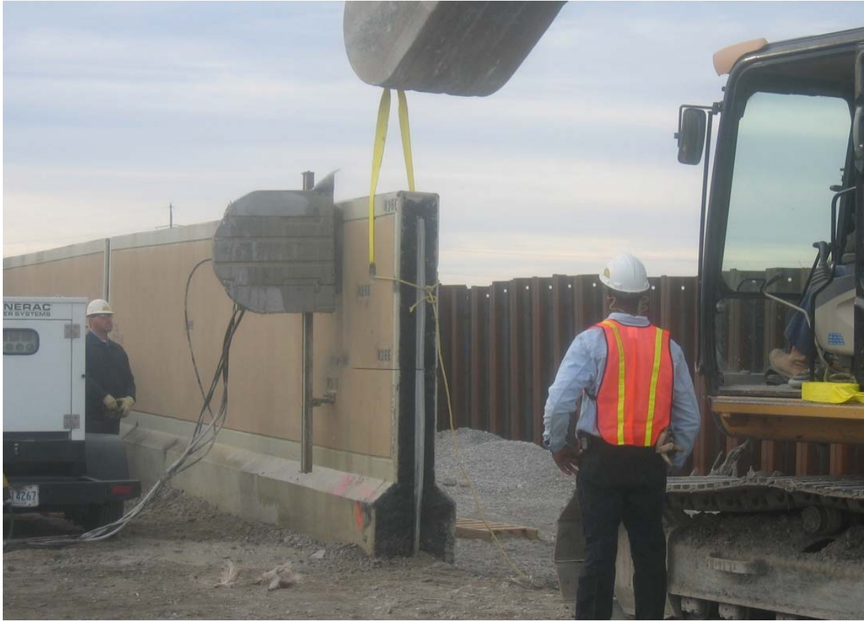
Figure 15-6. Sawing of Sample from Wall Panel H38
