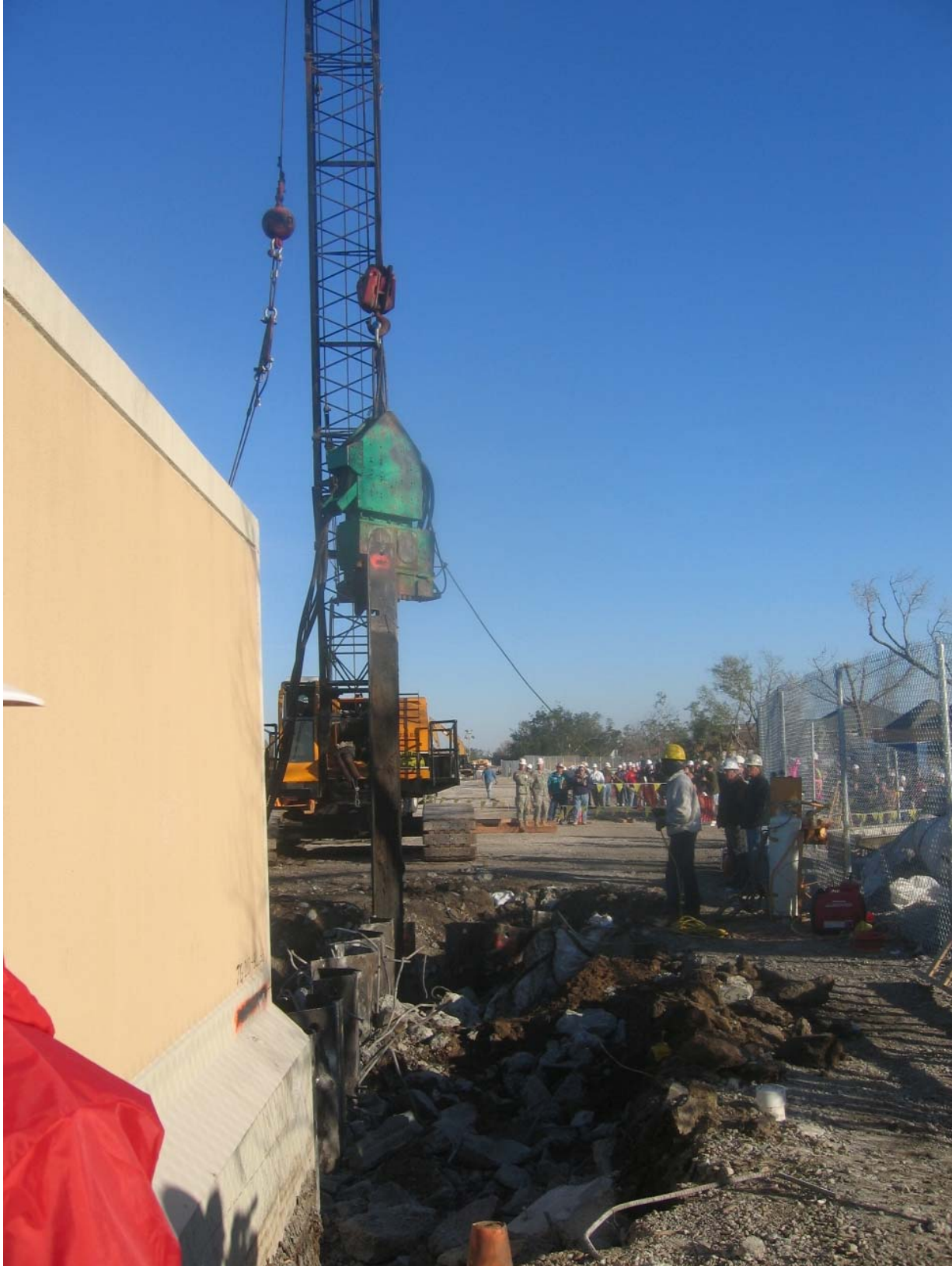
Figure 15-20. Extraction of Sheet Piles MH38SP2 and MH38SP3
