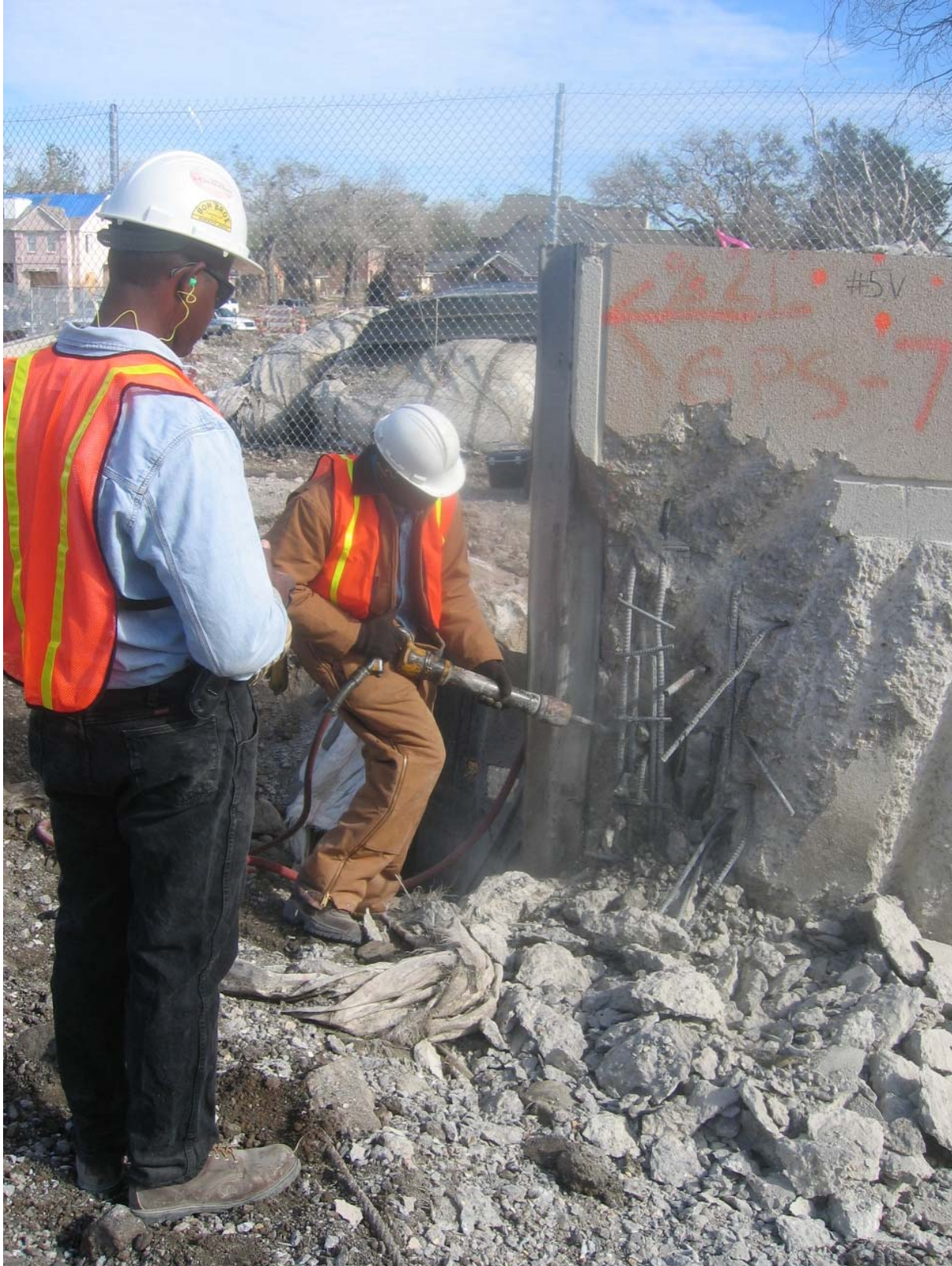
Figure 15-13. Demolition of Concrete Around Rebar Sample at Panel H38
