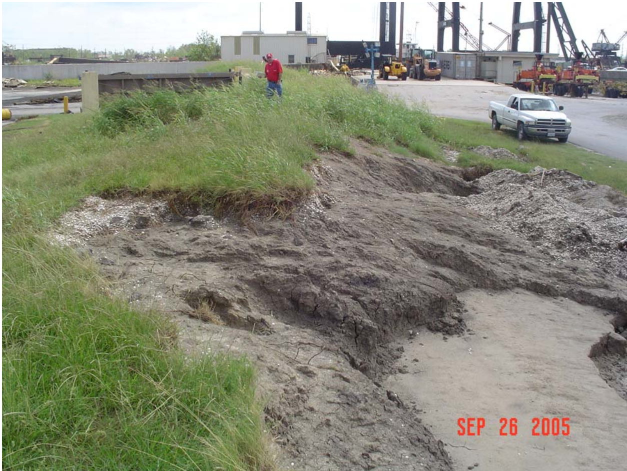
Figure 14-53. Overtopped Levee Section With Scour. View west from approximate CL Sta 14+00, B/L Sta 222+00
