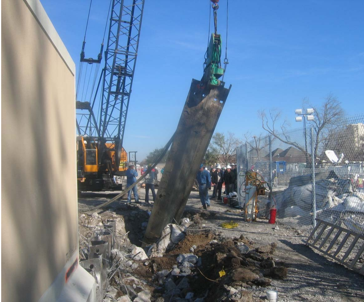
Figure 15-21. Extraction of Sheet Piles MH37SP1 and MH37SP0
