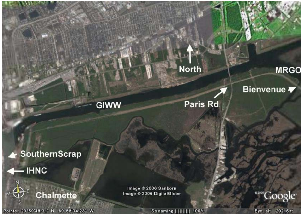
Figure 14-82. Photo of St. Bernard and Orleans Parish Levee System From IHNC East (north of Florida Ave.) to Bayou Bienvenue
