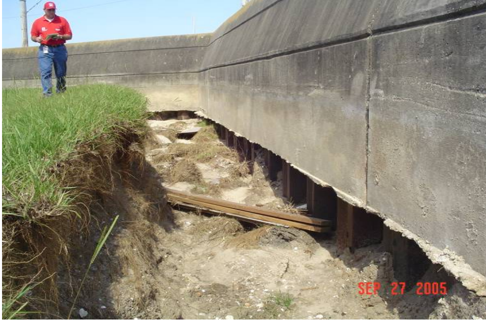
Figure 13-14. IHNC East, Approximate B/L Sta 101+00 (from drawing file H-2-24111, plate IV-23, DM2 Supp 8 IHNC Remaining Levees), North of Chef Menteur Hwy Bridge. Top of I-wall is elev 14.75, bottom of concrete is elev 7, and levee crown is elev 9. Nearest B/L boring is Sta 96+00 (No. 9EU), 500 feet distant. Approximate storm surge impact was a 2.5-ft water crest cascading over the 6-ft concrete wall. Note that the scour was deeper than the concrete base, indicating that the structural backfill and the original levee material eroded
