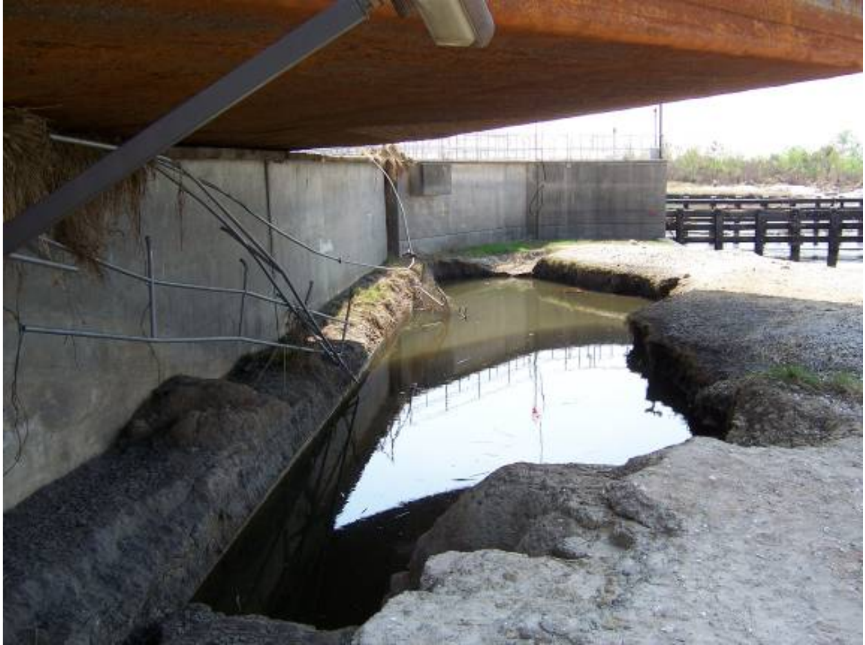
Figure 14-110. Barge Resting on T-Wall
