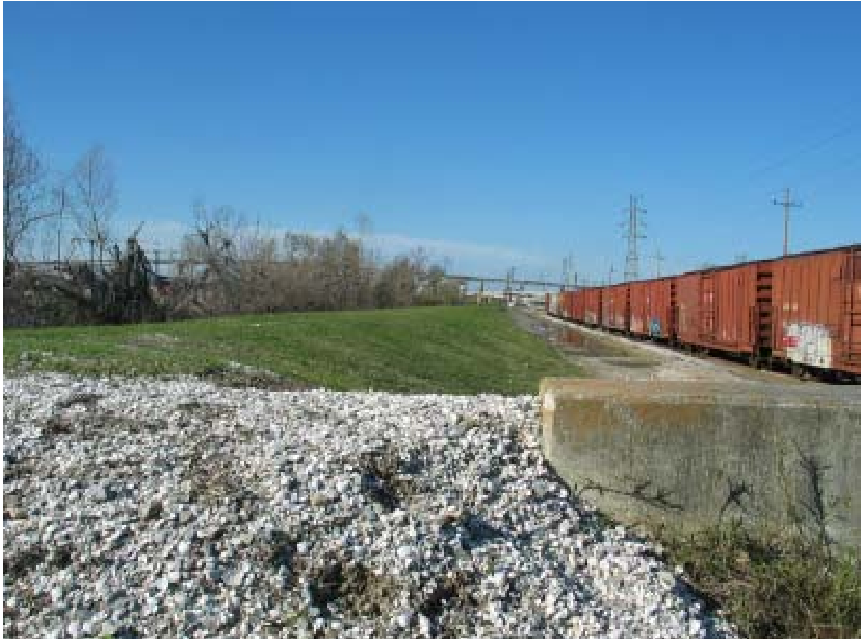
Figure 14-44. E4 Scour Repaired
