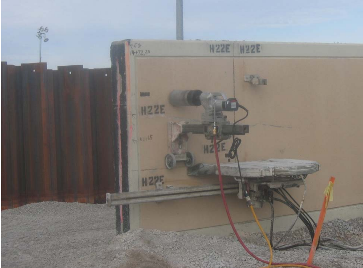
Figure 15-8. Core Drill and Saw Mounted at Panel H22
