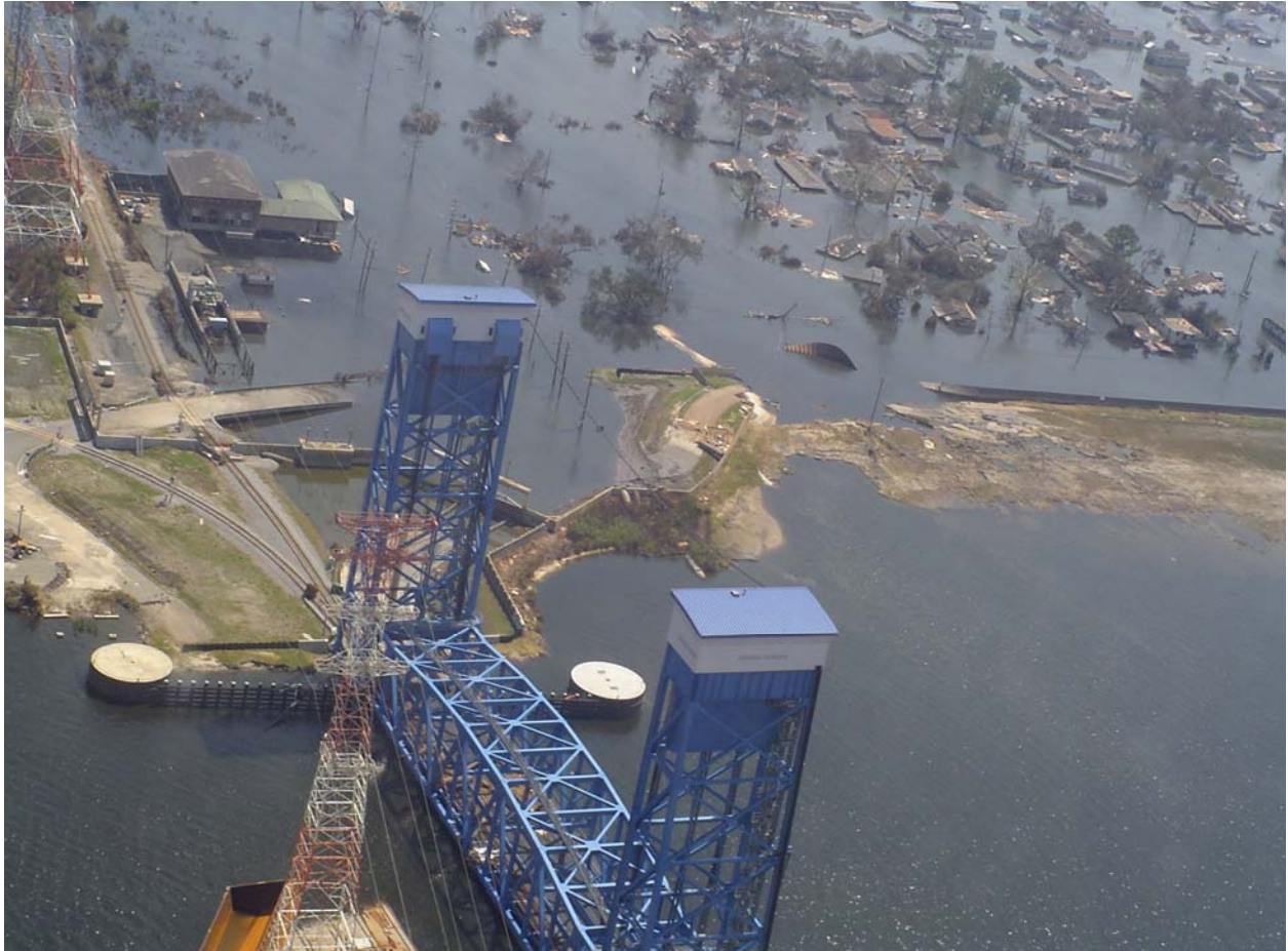
Figure 14-29. Florida Ave Bridge, View East. I-Wall Failure is Seen to Right of Bridge
