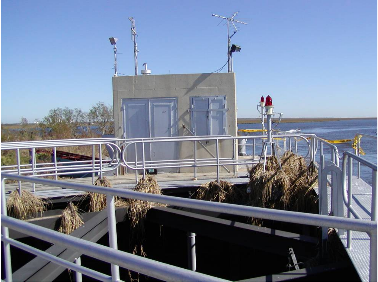
Figure 19. Bayou Bienvenue gauge house.
