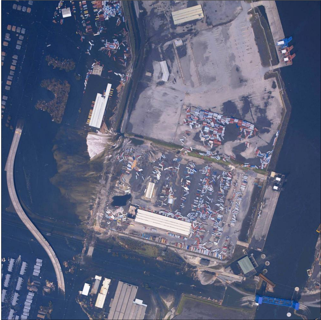
Figure 127. Floodwall and earth levee breaches on west side of the Inner Harbor Navigation Channel.
