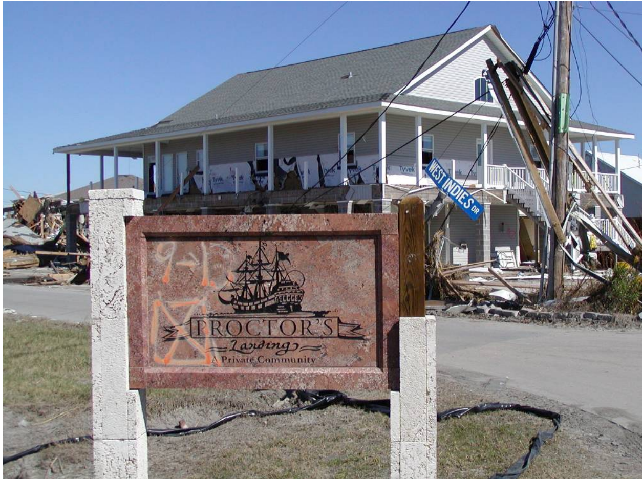
Figure 21. Home in Shell Beach containing high-water mark LA 1087 at 31 in. (2.6 ft) above second level floor.
