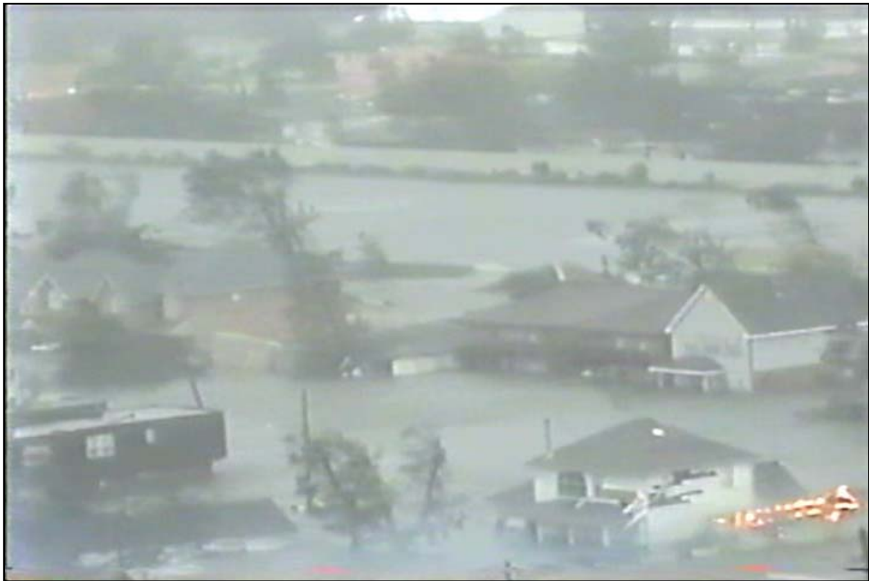
Figure 119. This video frame shows the breach in the 17th Street Canal floodwall and flooding in Lakeview about 1620 UTC (11:20 a.m. CDT) on Monday, 29 August 2005. The portion of the breach shown in this image is near the intersection of Bellaire Drive and Stafford Place. (Video provided by National Geographic Television).
