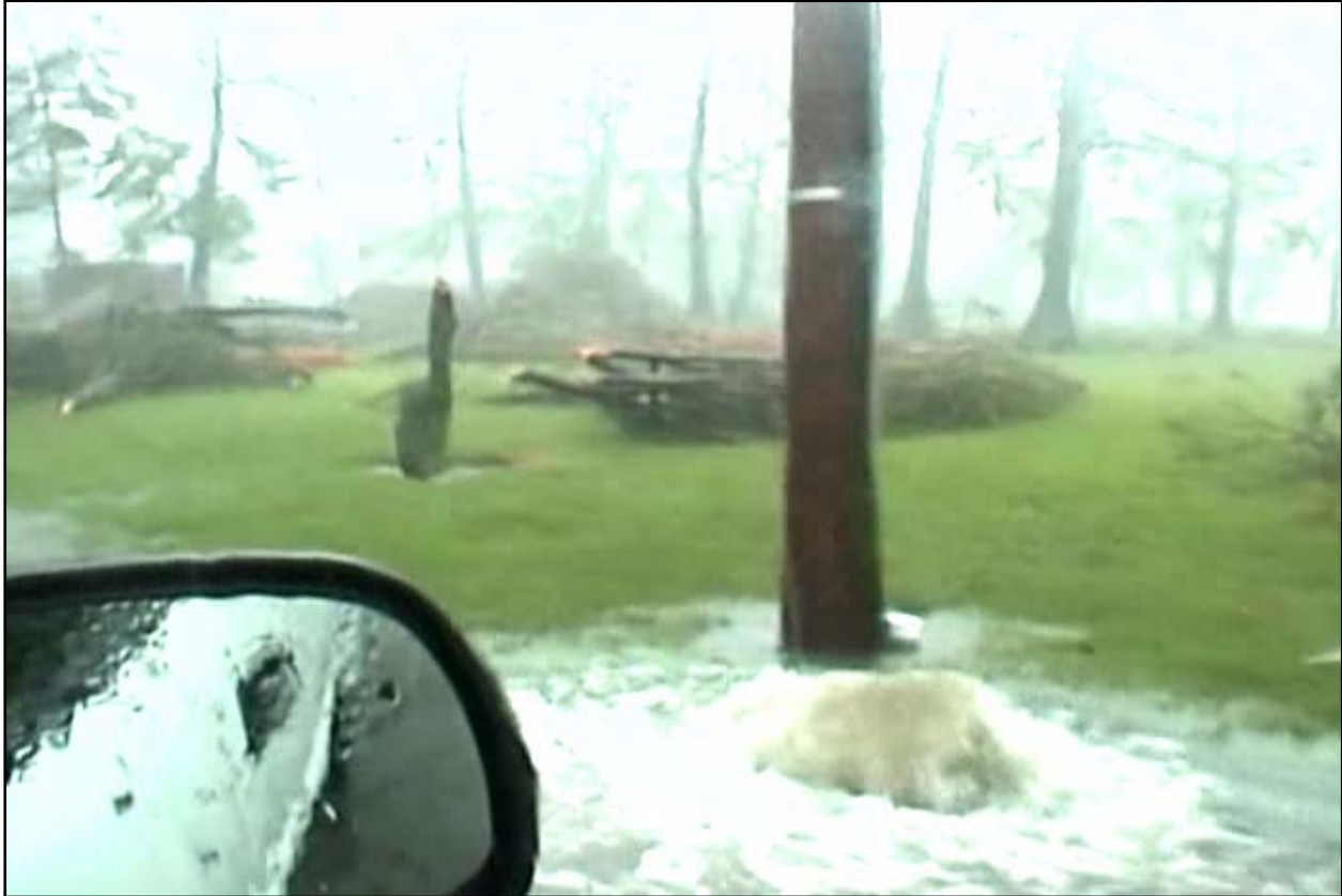
Figure 132. Water backing up through storm drain on the campus of the Baptist Theological Seminary on Monday afternoon.
