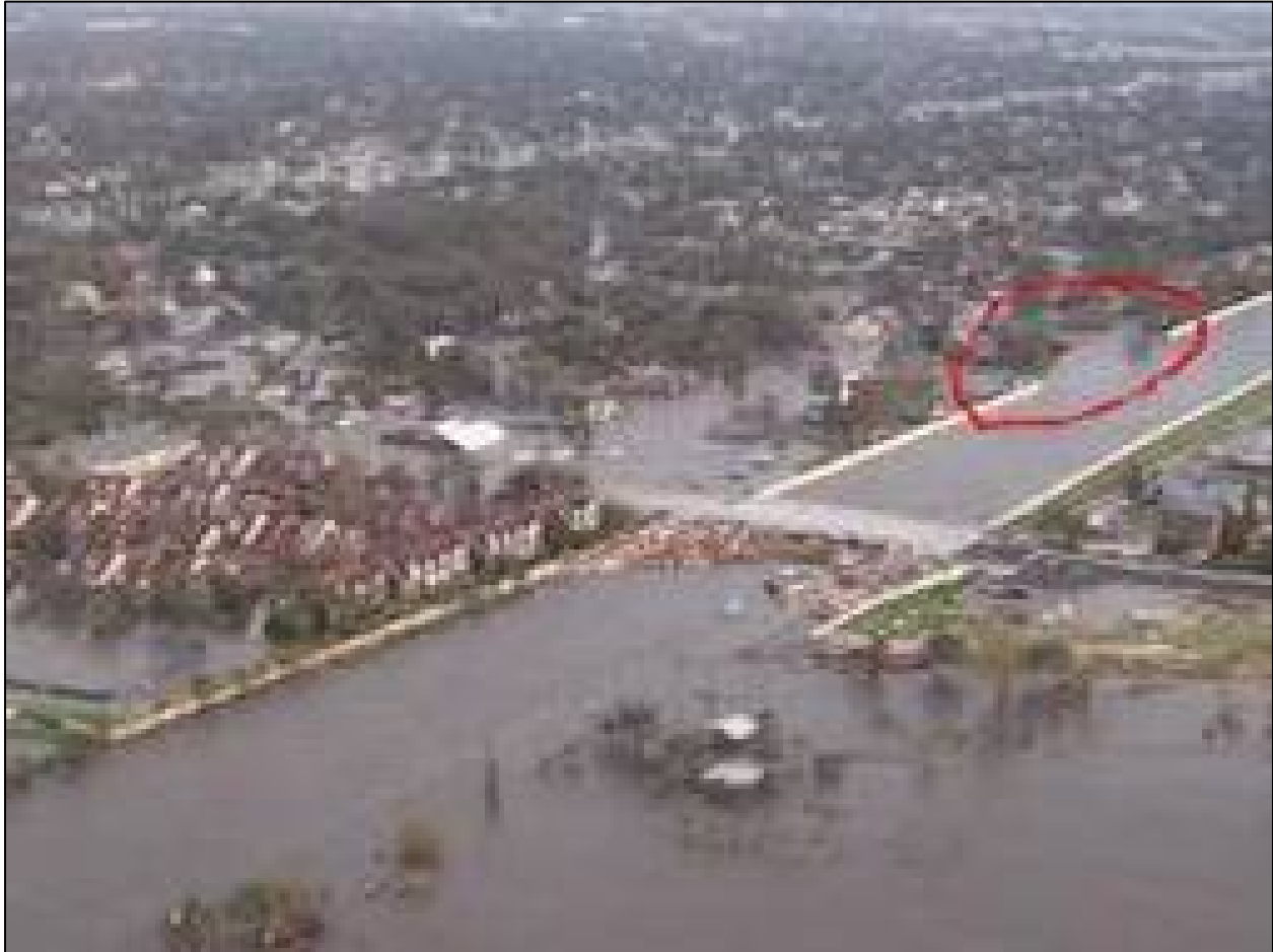
Figure 143. 17th Street Canal on 29 August 2005. Looking south showing breach and debris accumulated against lake side of Hammond Highway bridge.
