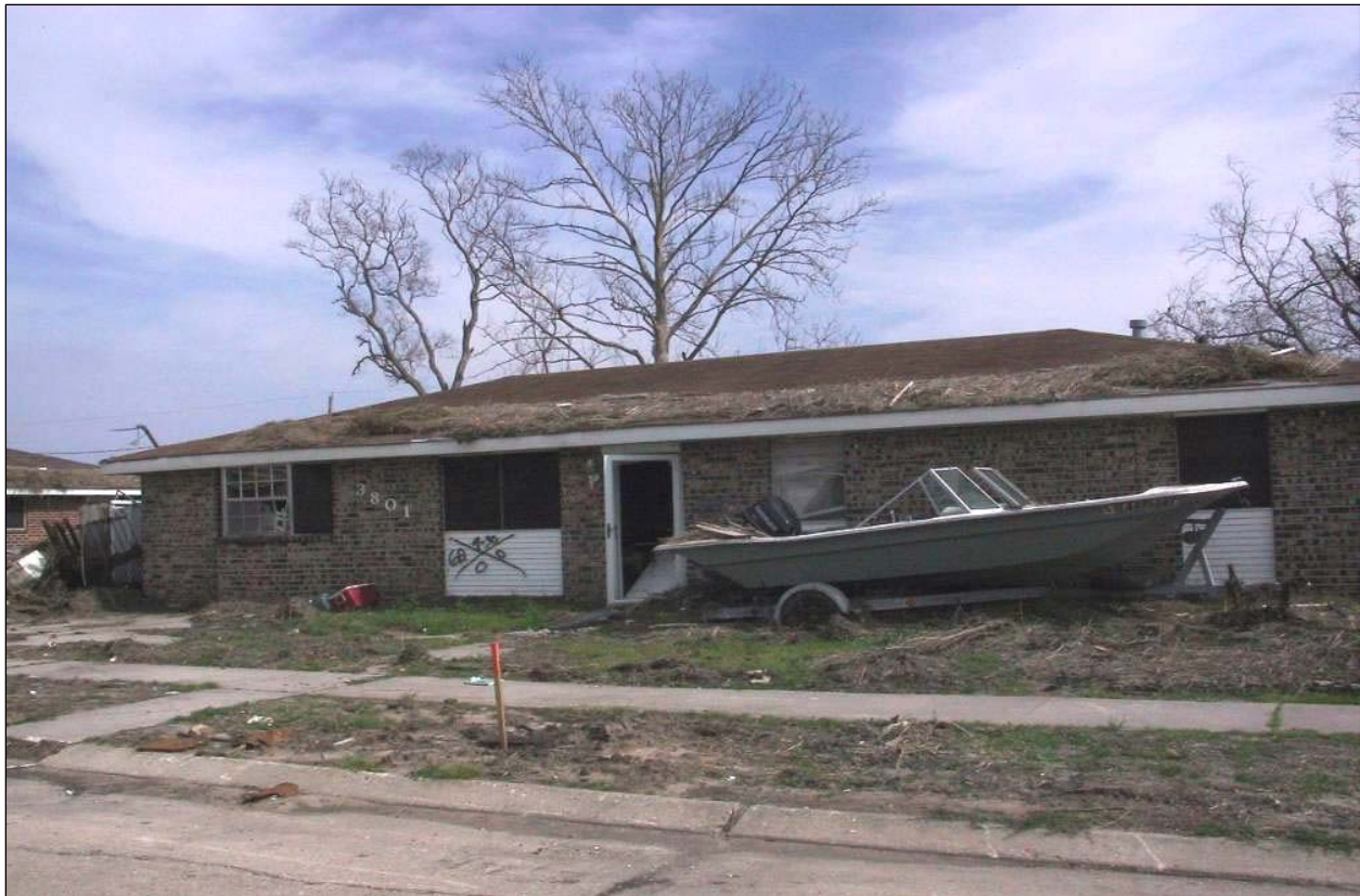
Figure 138. Marsh grass and typical inundation level for the homes in Chalmette area.
