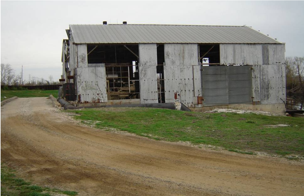
Guichard Pump Station #2
