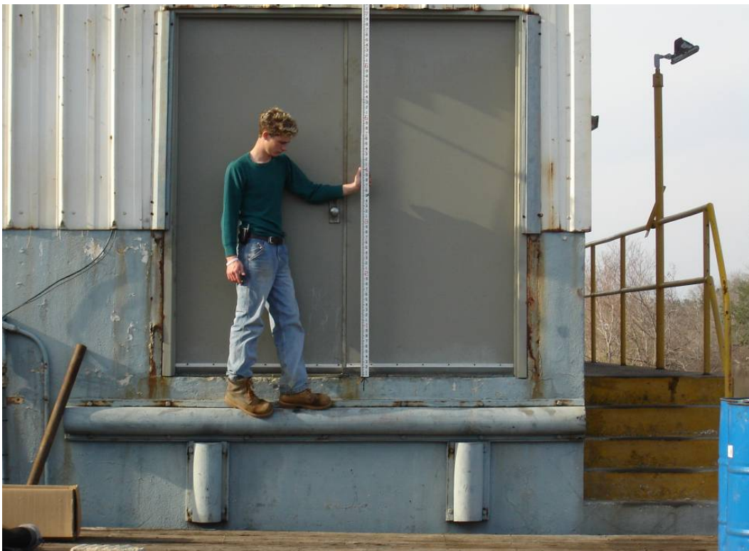
Finished Floor = 6.74 feet NAVD88(2004.65) Field Book 060854
