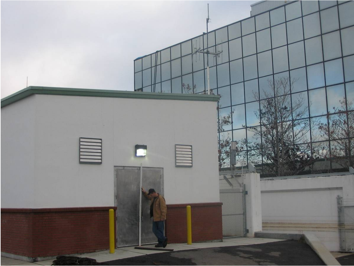
OP 12 Finished Floor = 2.63 feet NAVD88(2004.65) Field Book 060851
