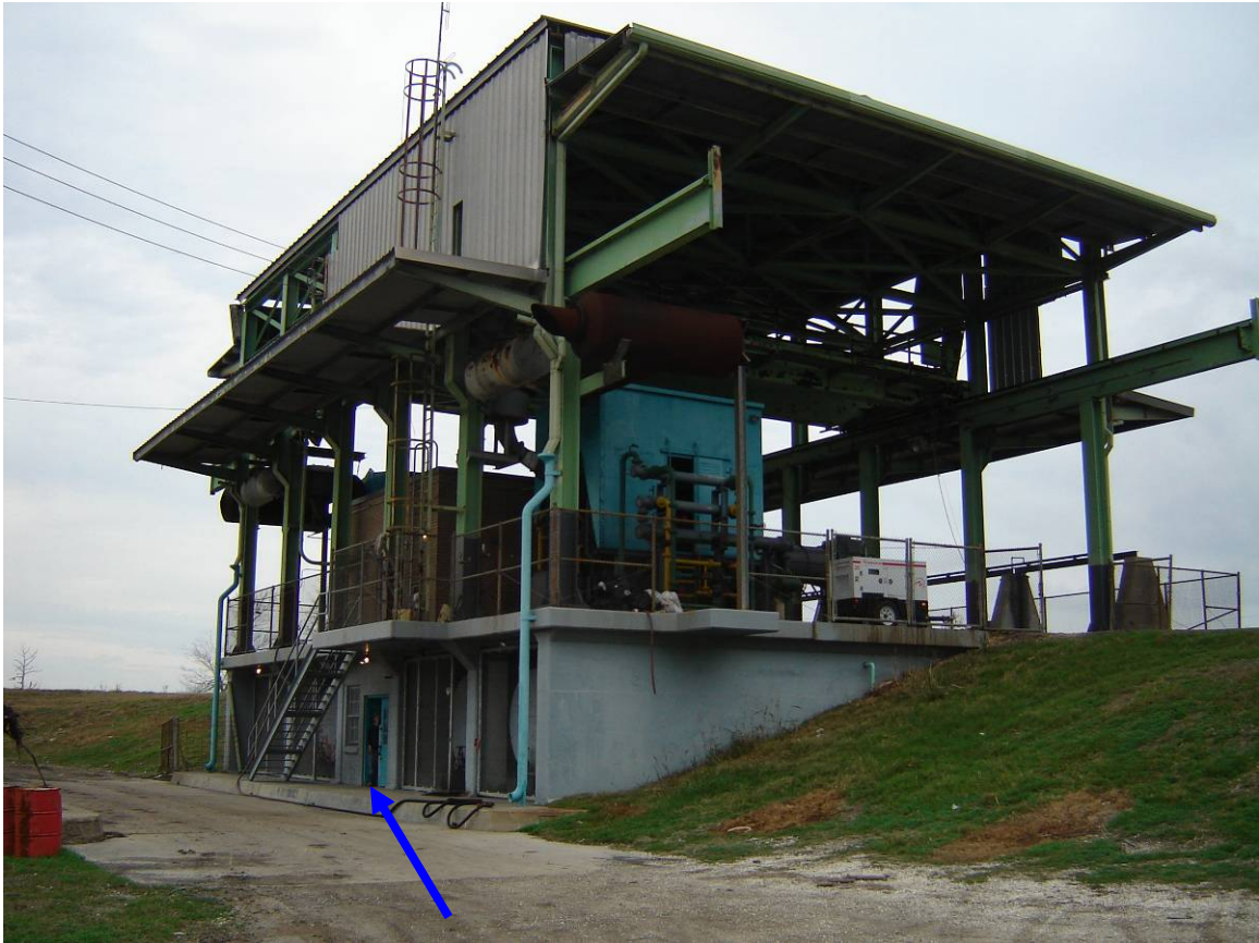
Finished Floor #2 = 2.43 feet NAVD88(2004.65) Field Book 060851
