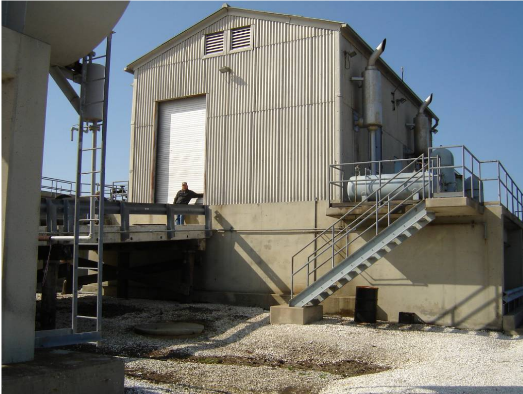
SUNRISE #2 PUMP STATION
