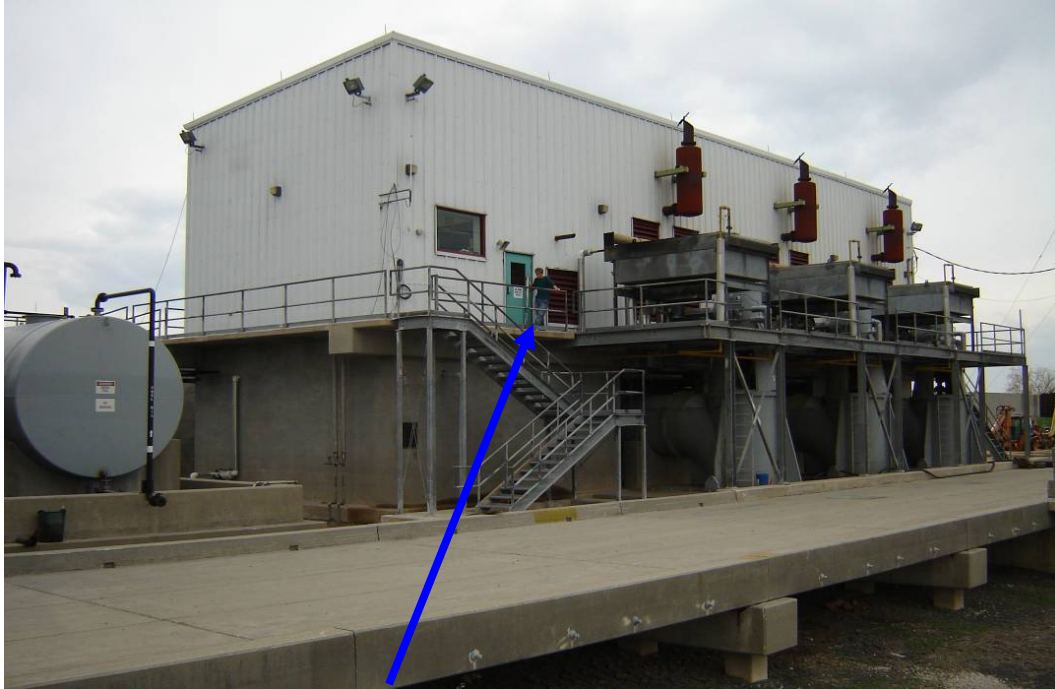
Finished Floor #1 = 15.52 feet NAVD88(2004.65) Field Book 060851
