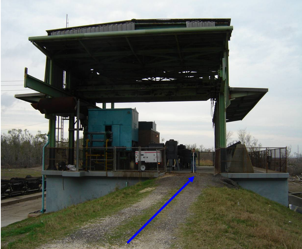
Finished Floor #1 = 13.92 feet NAVD88(2004.65) Field Book 060851
