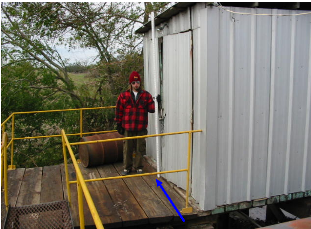
Finished Floor #2 = 8.11 feet NAVD88(2004.65) Field Book 060852
