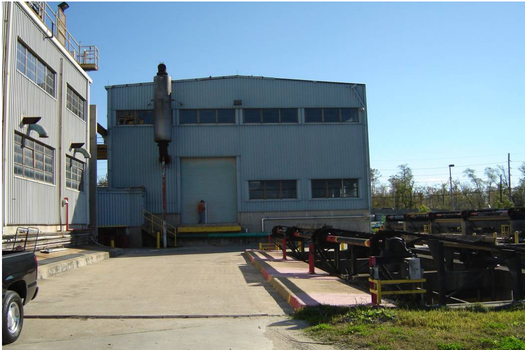
Cousins #2 Pump Station
