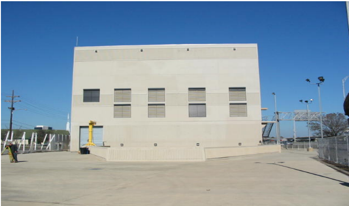
I-10 Pump Station
