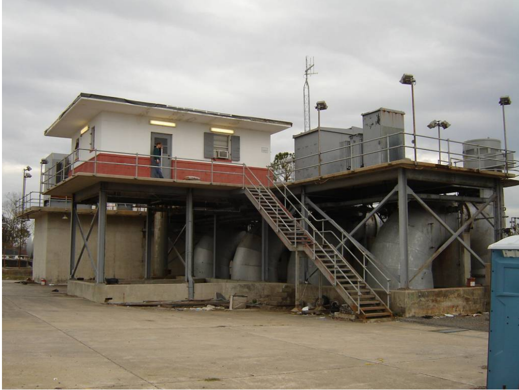
OP #16 -- ST. CHARLES PUMP STATION
