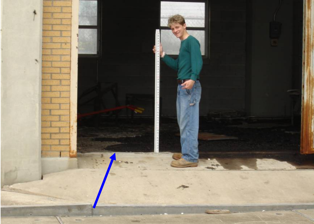
Finished Floor = 3.69 feet NAVD88(2004.65) Field Book 060851
