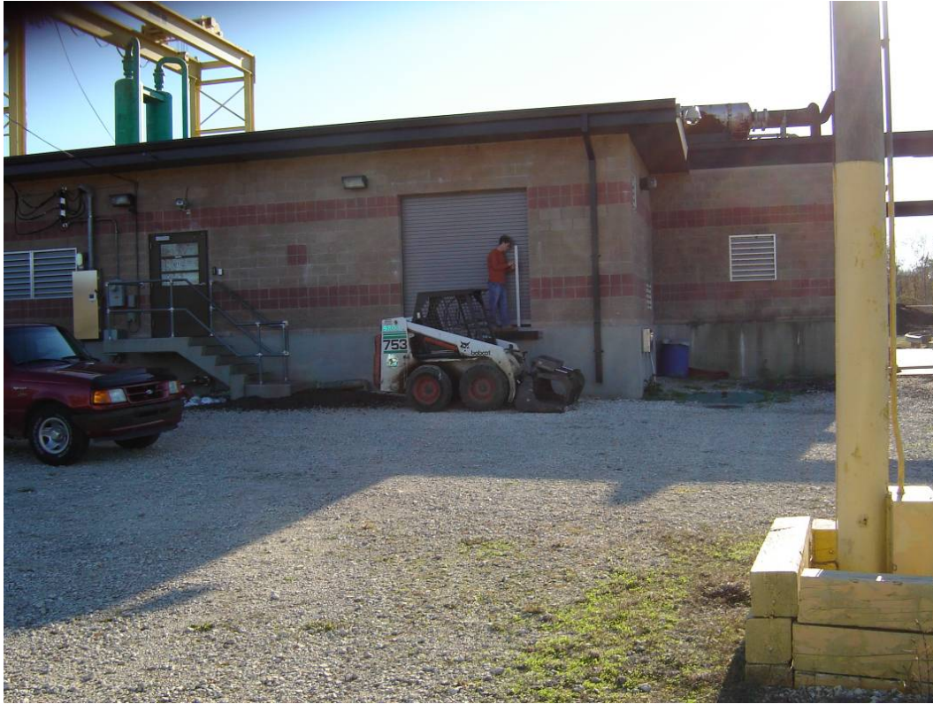
Estelle #2 Pump Station
