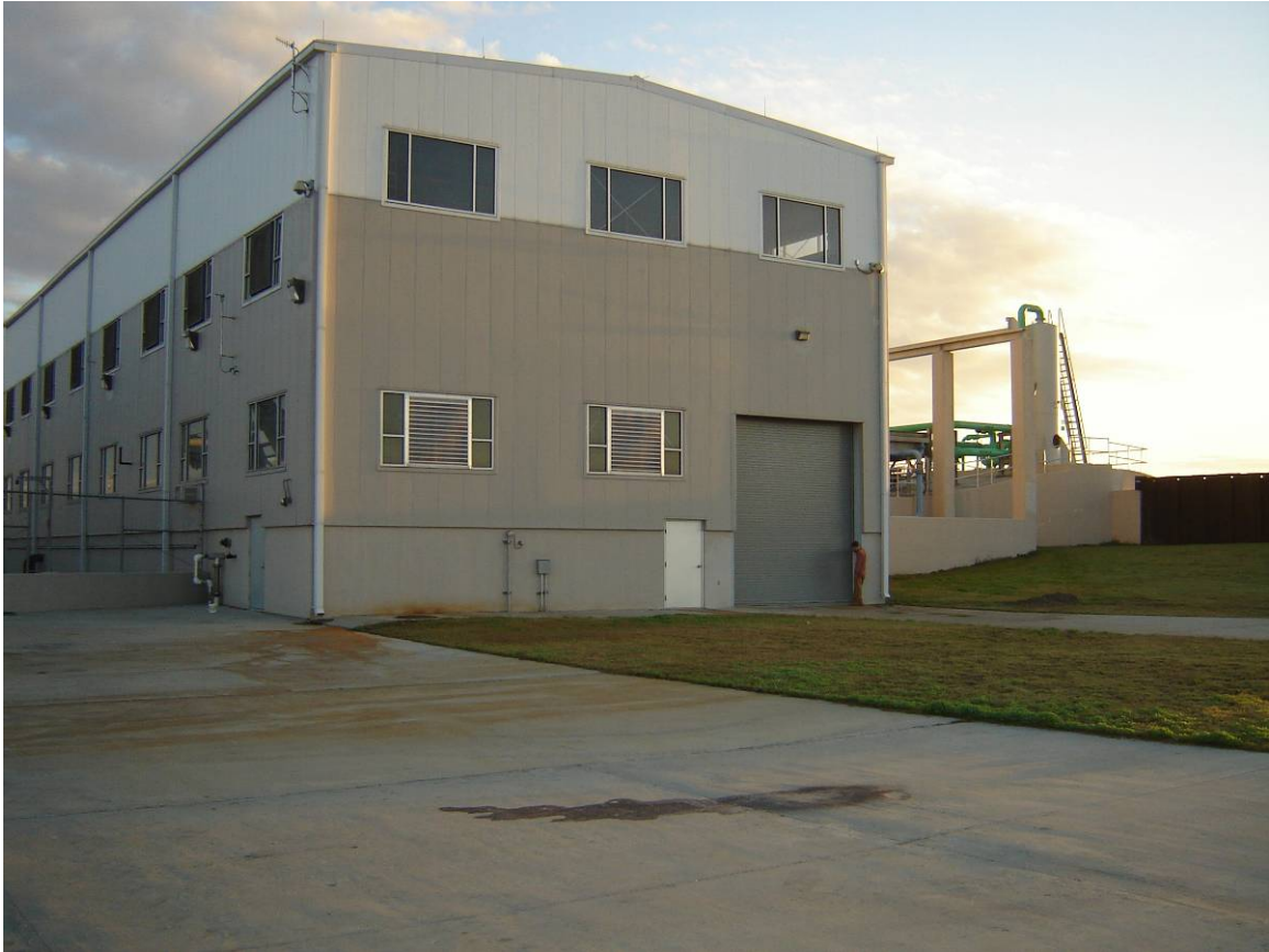
Whitney-Barataria Pump Station
