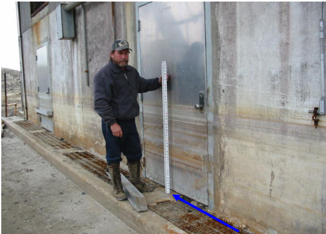
Finished Floor #1 = -0.18 feet NAVD88(2004.65) Field Book 060851
