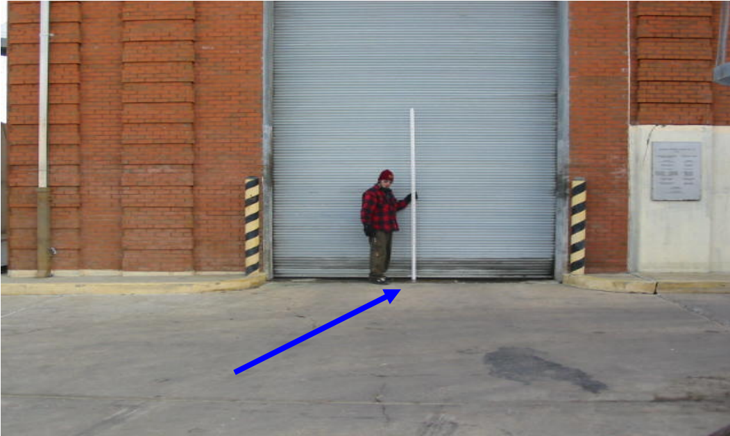
OP 19 Finished Floor #1 = -3.79 feet NAVD88(2004.65) Field Book 060851
