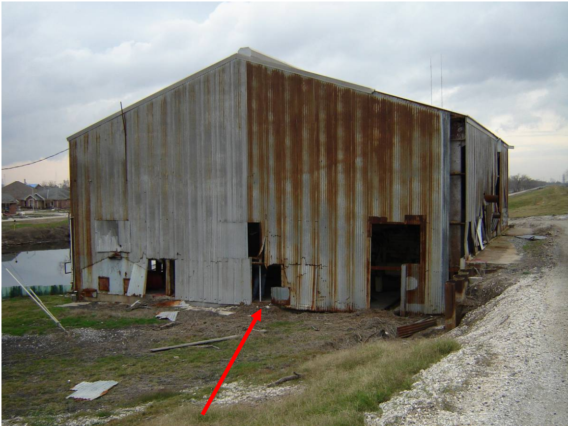
Bayou Villere Pump Station #3 Finished Floor = 2.16 feet NAVD88(2004.65) Field Book 060851
