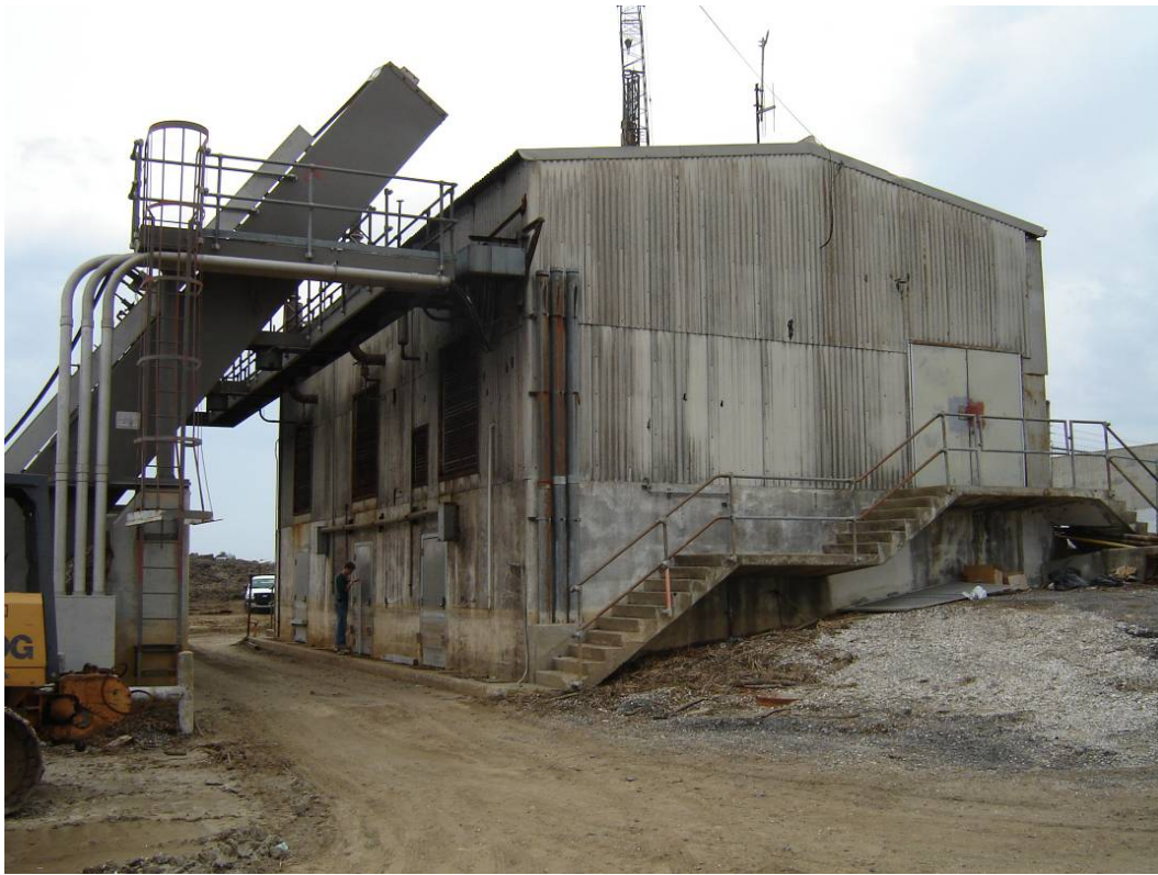
OP 15 Pump Station
