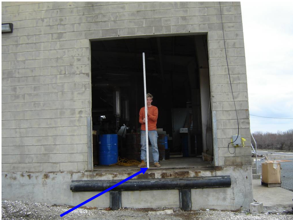
Finished Floor = 12.59 feet NAVD88(2004.65) Field Book 060852
