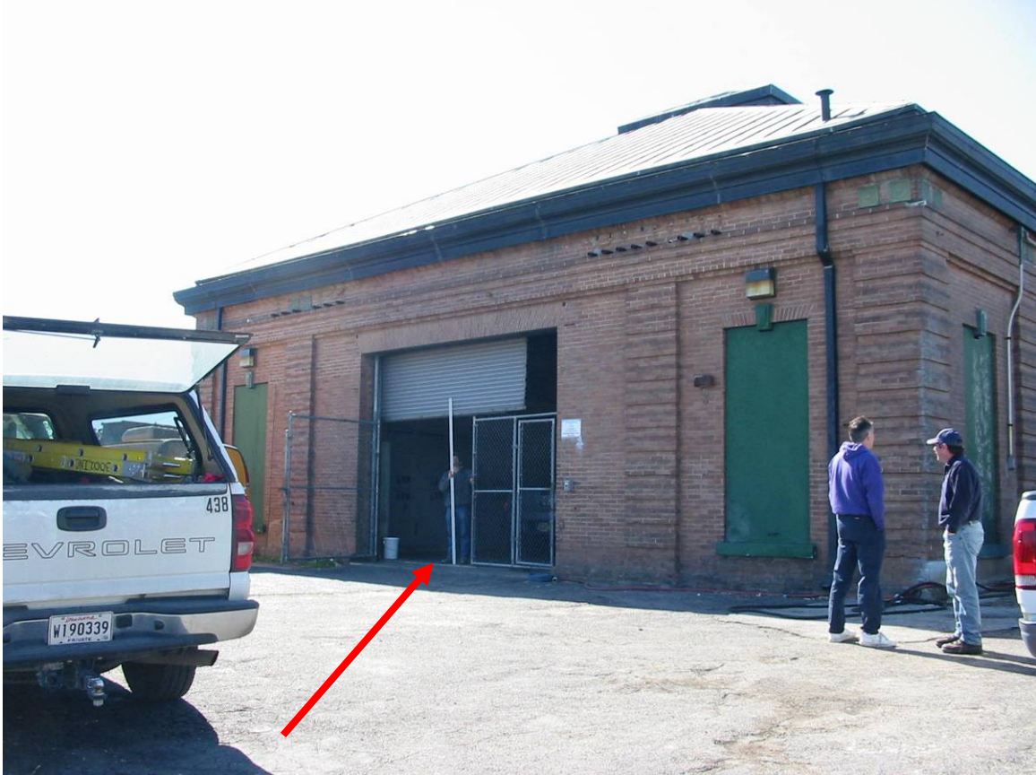
Finished Floor = 2.03 feet NAVD88(2004.65) Field Book 060851
