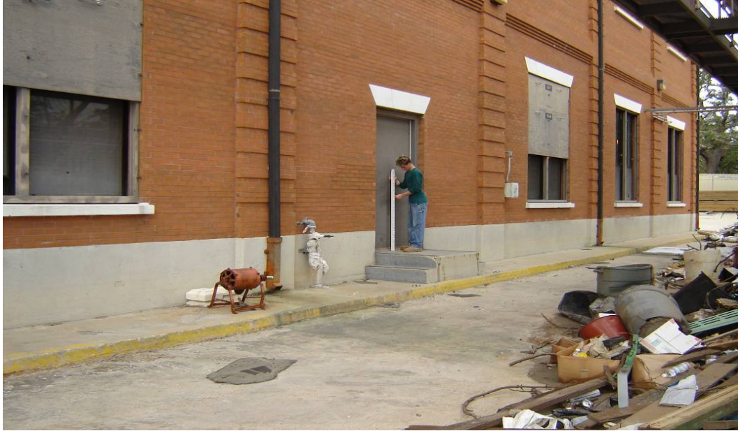
Finished floor = -1.50 feet NAVD 88 2004.65 Field book 060851
