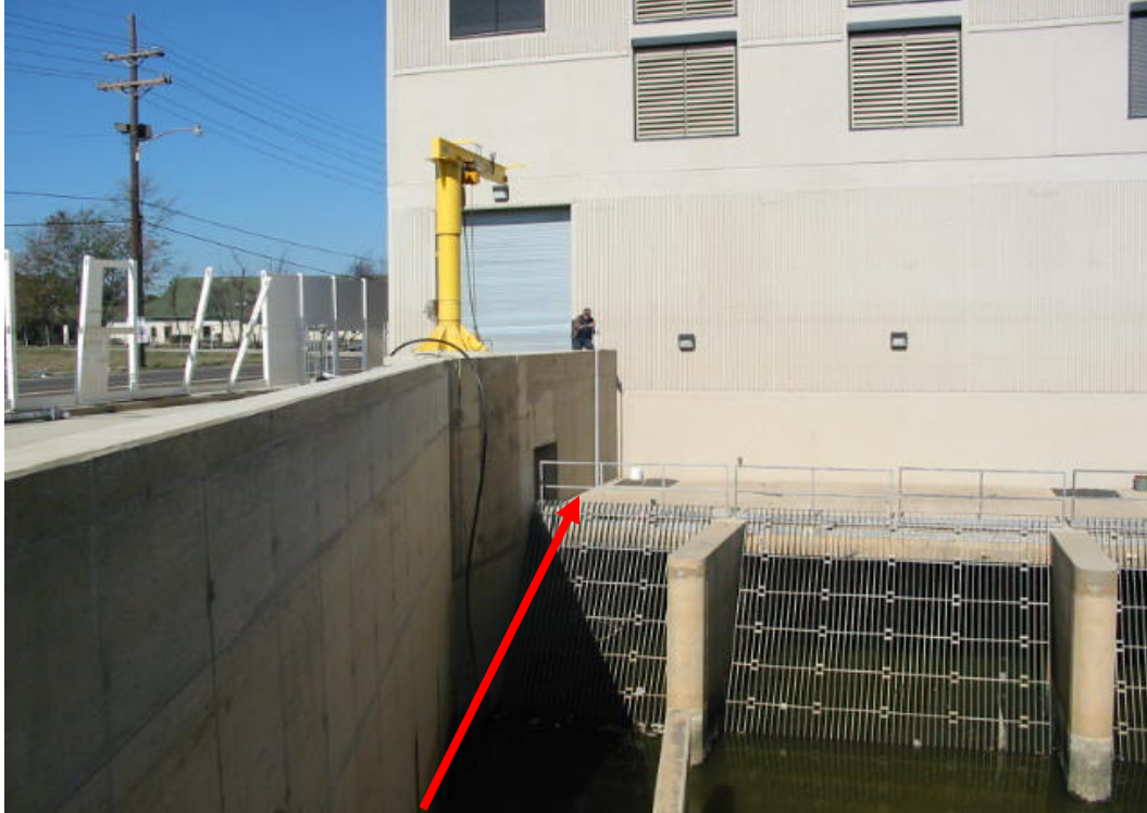
Finished Floor #1 = -11.60 feet NAVD88(2004.65) Field Book 060852
