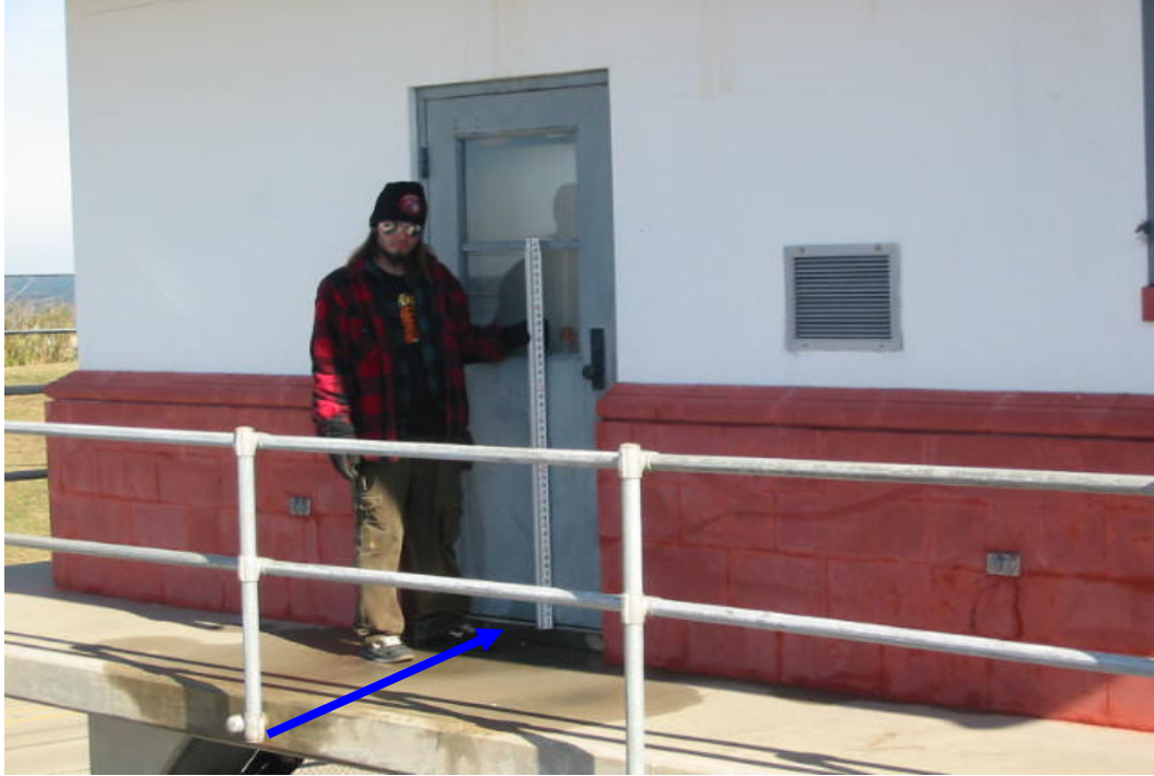
Finished Floor = 14.93 feet NAVD88(2004.65) Field book 060851
