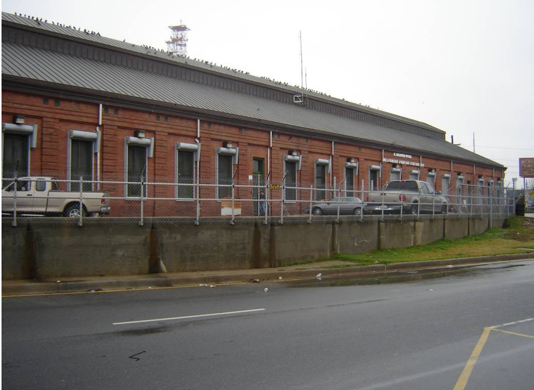
OP #1 Pump Station
