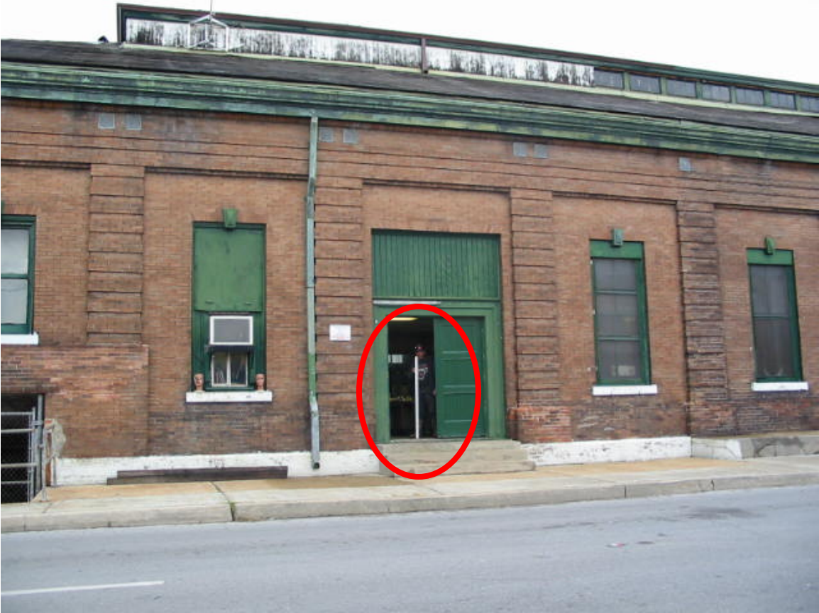
OP #2 PUMP STATION
