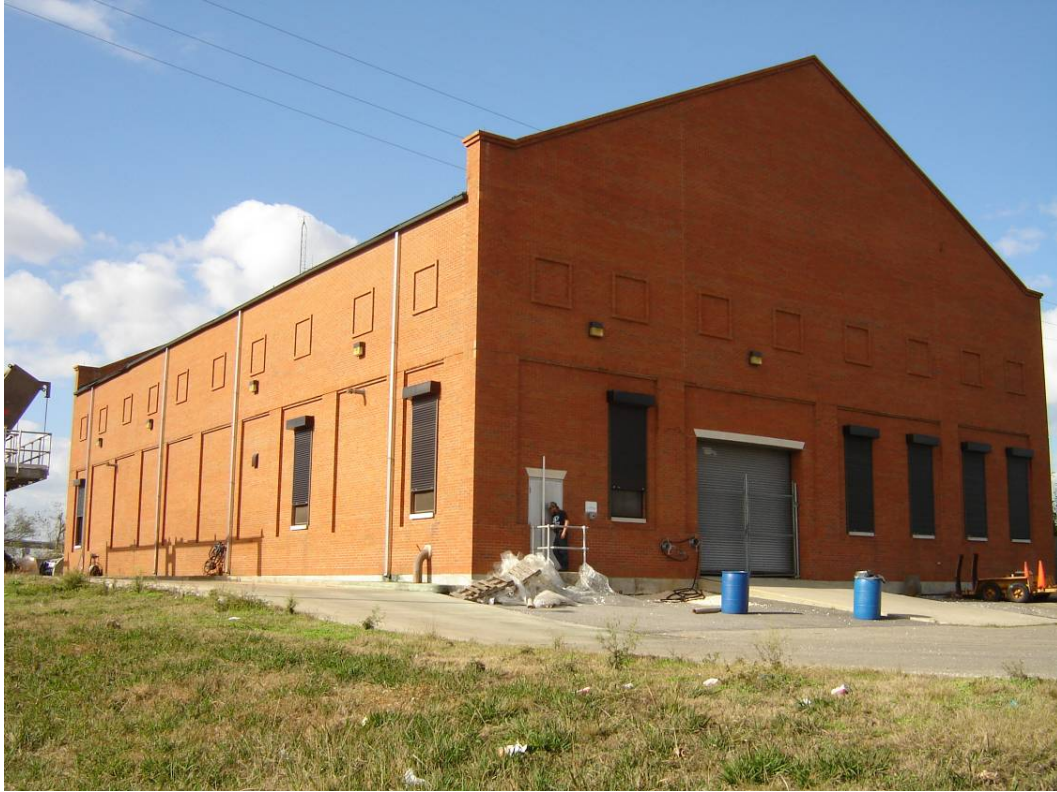
OP 11 PUMP STATION
