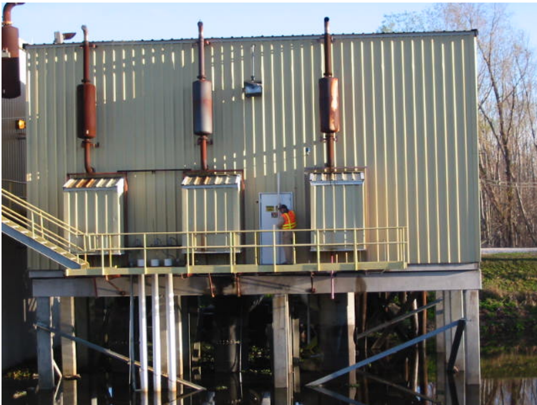
Finished Floor #2 = 8.39 feet NAVD88(2004.65) Field Book 060858
