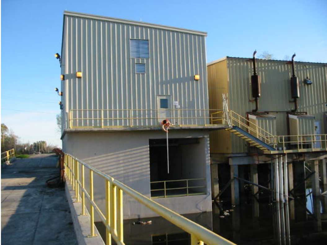
Finished Floor #1 = 14.21 feet NAVD88(2004.65) Field Book 060858
