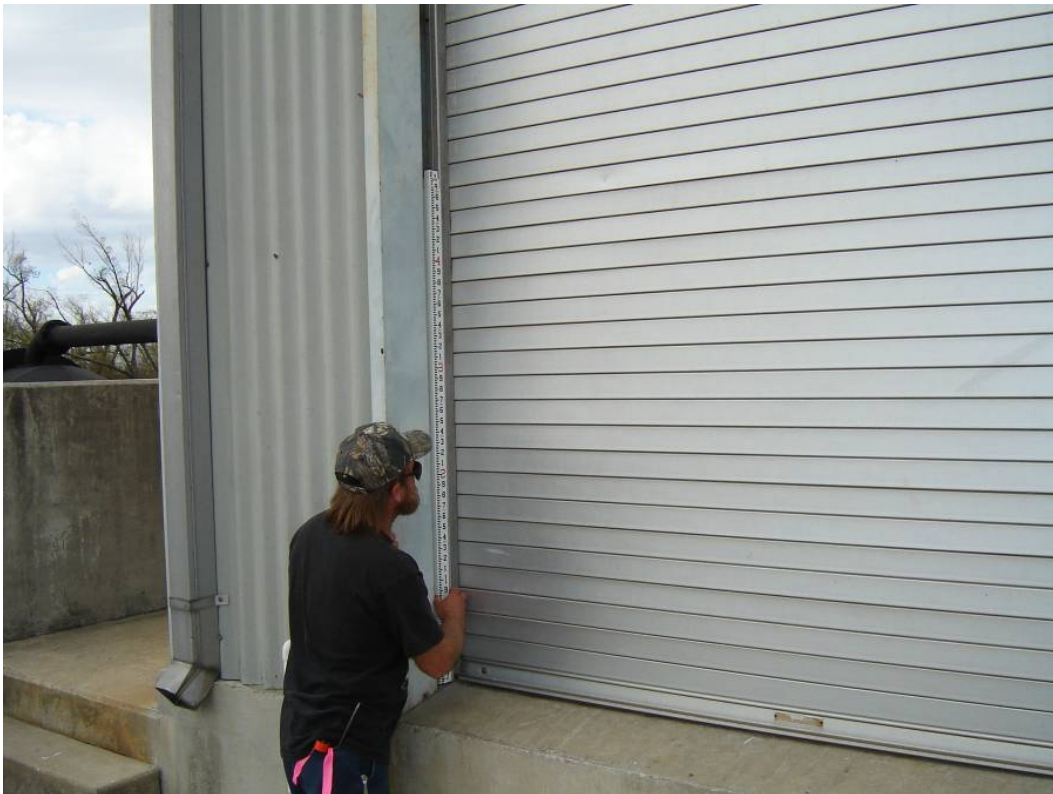
Finished Floor = 9.52 feet NAVD88(2004.65) Field Book 060852
