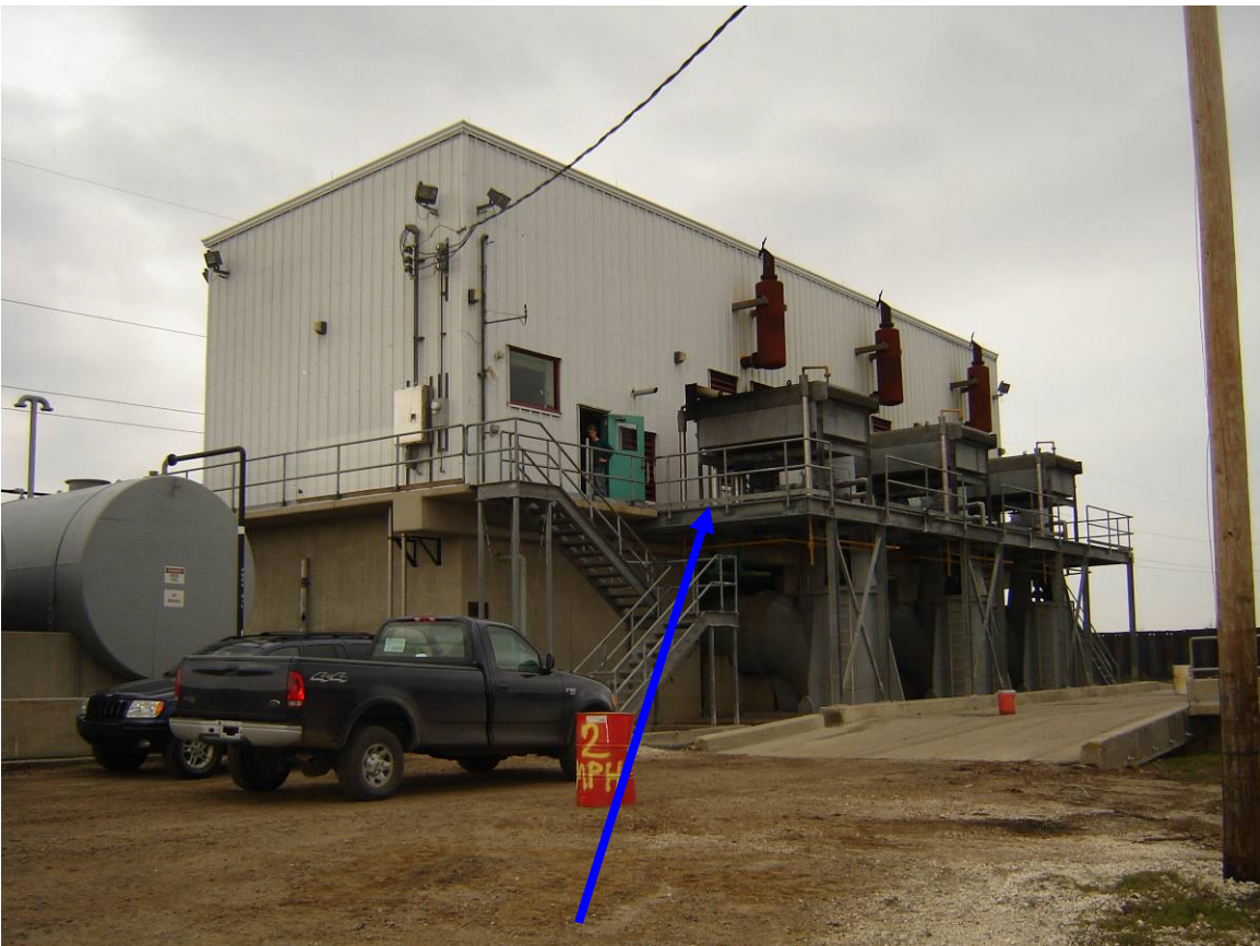
Finished Floor = 1.25 feet NAVD88(2004.65) Field Book 060851
