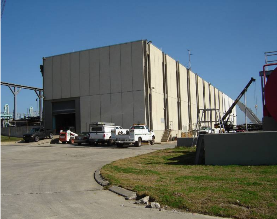
Elmwood Canal Pump Station JP-03
