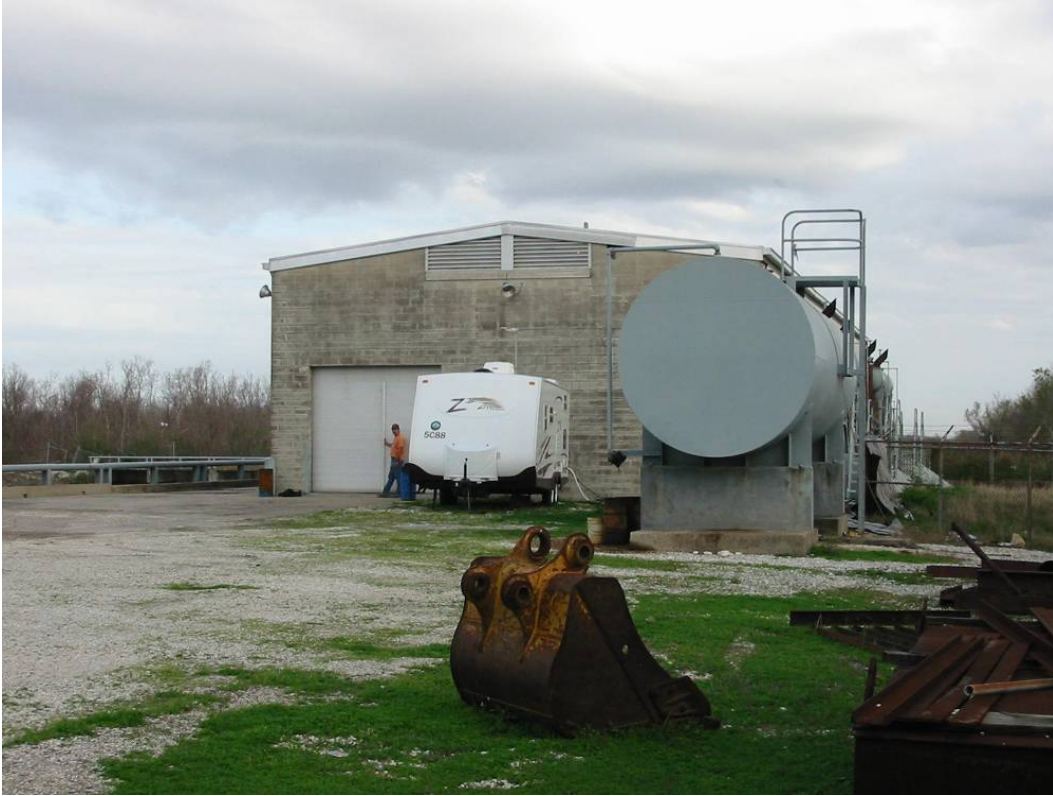
SCARSDALE PUMP STATION
