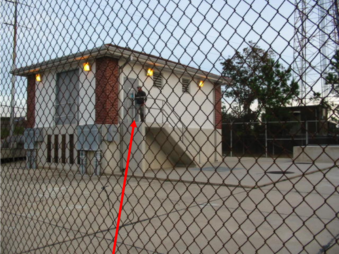
Finished Floor = 2.65 feet NAVD88(2004.65) Field Book 060851
