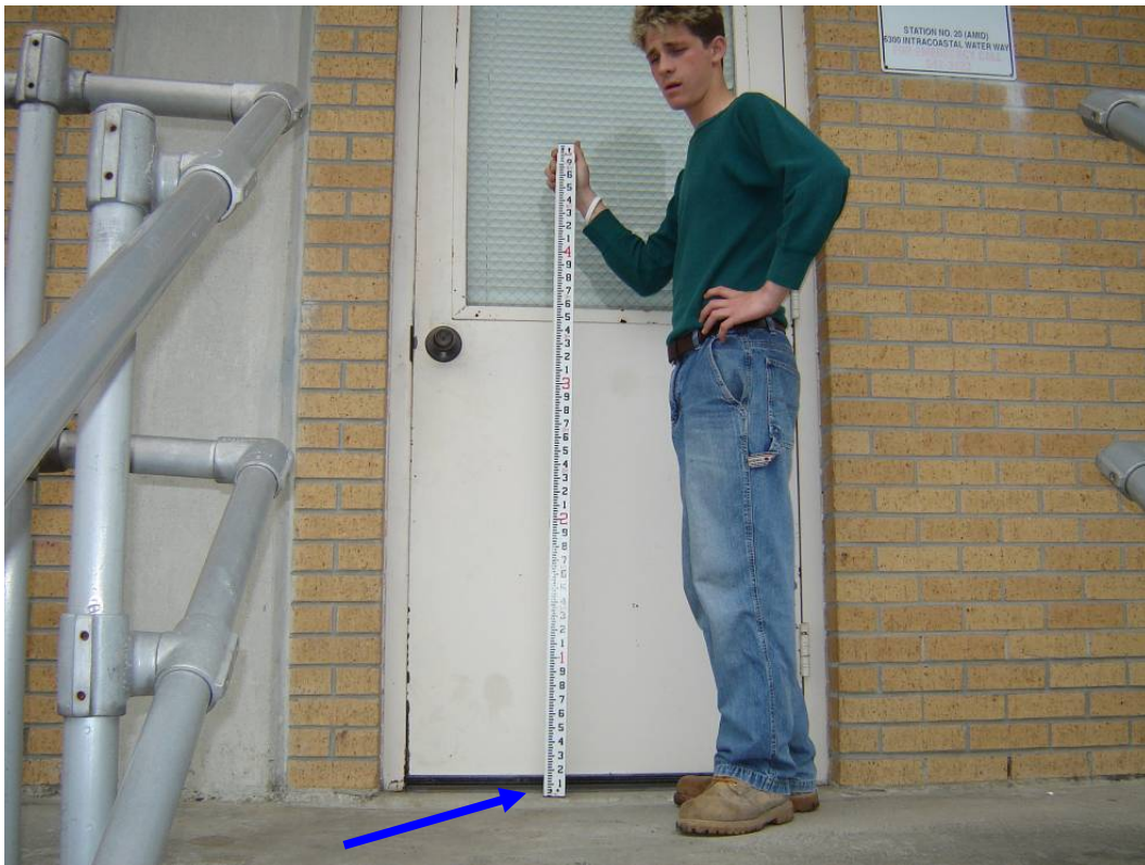
Finished Floor (Upper) = 19.20 feet NAVD88(2004.65) Field Book 060851
