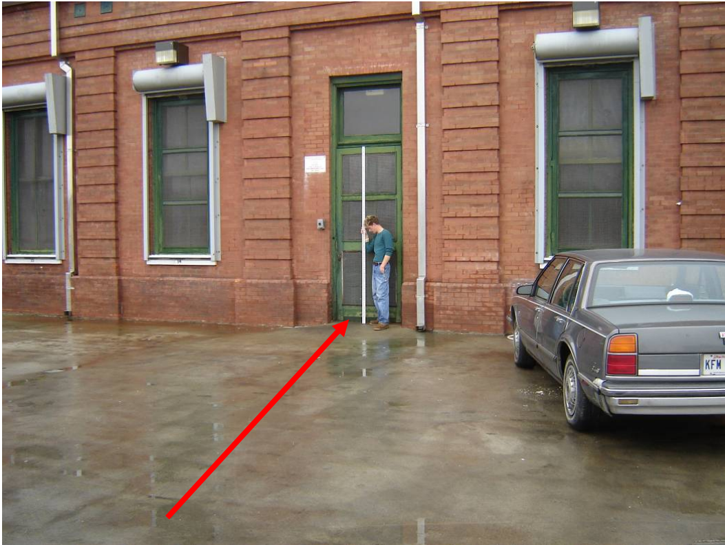
Finished Floor = 1.65 feet NAVD88(2004.65) Field Book 060851
