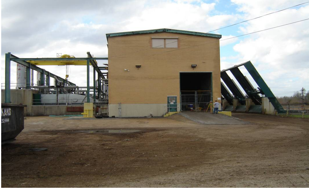
OP #13 PUMP STATION
