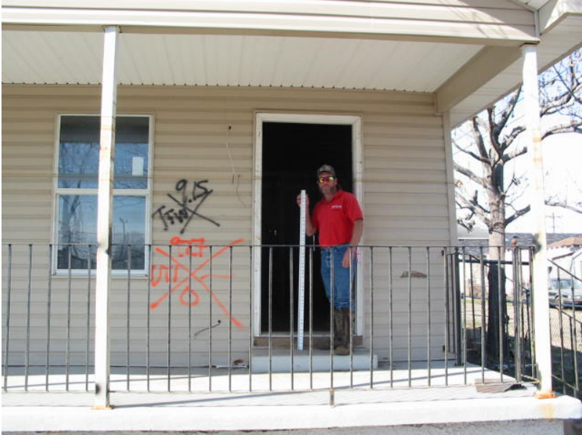
Corner Of Peoples and Edge - Top Step at front door = -3.87' NAVD88(2004.65) Bk. 060851, Pg. 6
