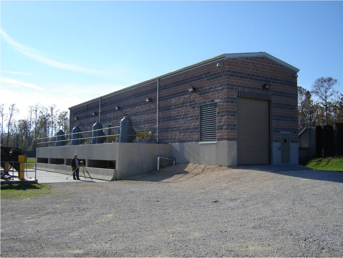
Westminister Pump Station
