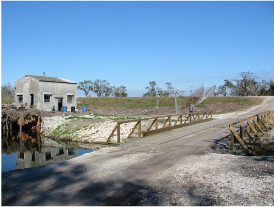
Belair Pump Station
