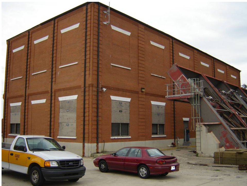
Citrus Pump Station OP 10
