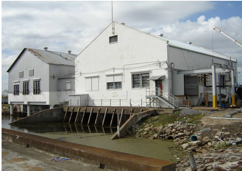
BELLE CHASE #1 Pump Station
