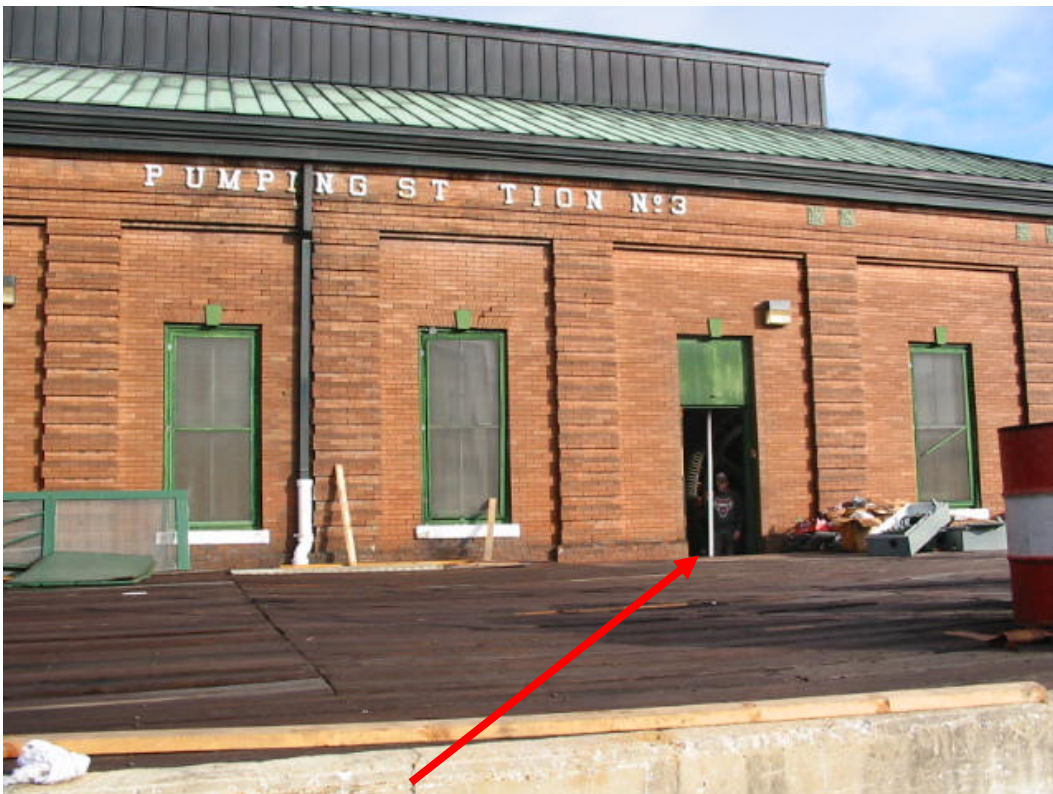
Finished Floor = 1.23 feet NAVD88(2004.65) Field Book 060851
