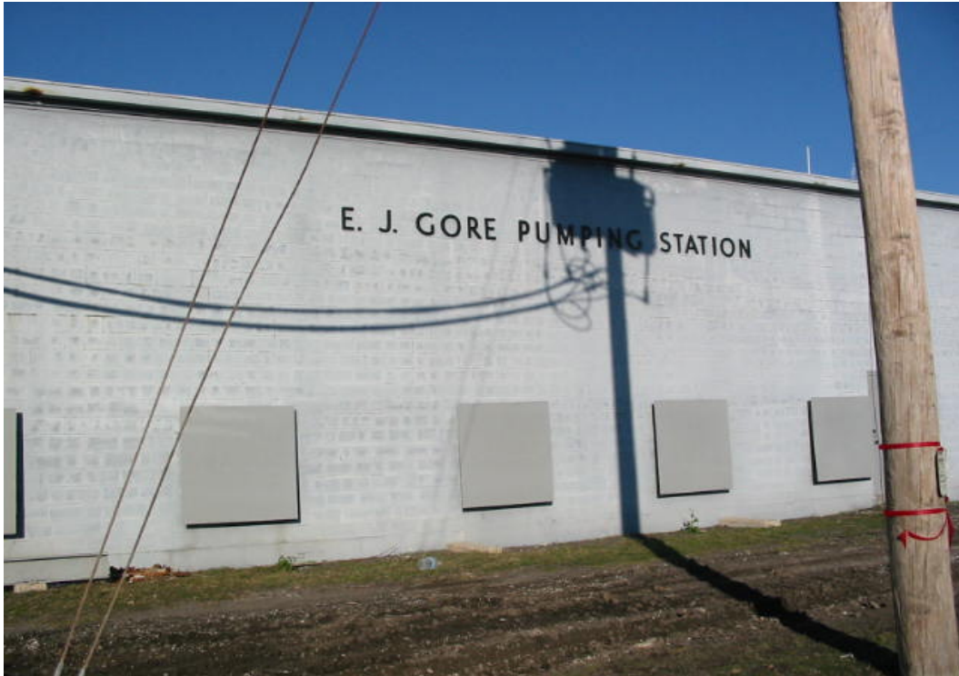
E.J. Gore Pump Station
