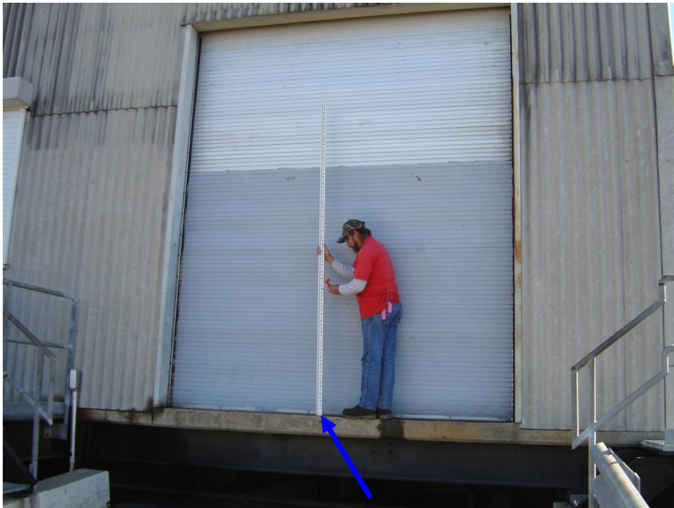
Finished Floor = 17.05 feet NAVD88(2004.65) Field Book 060854
