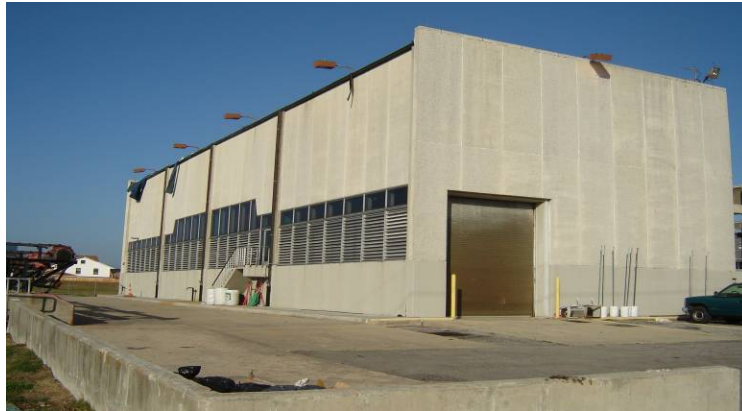
Pump Station JP-01
