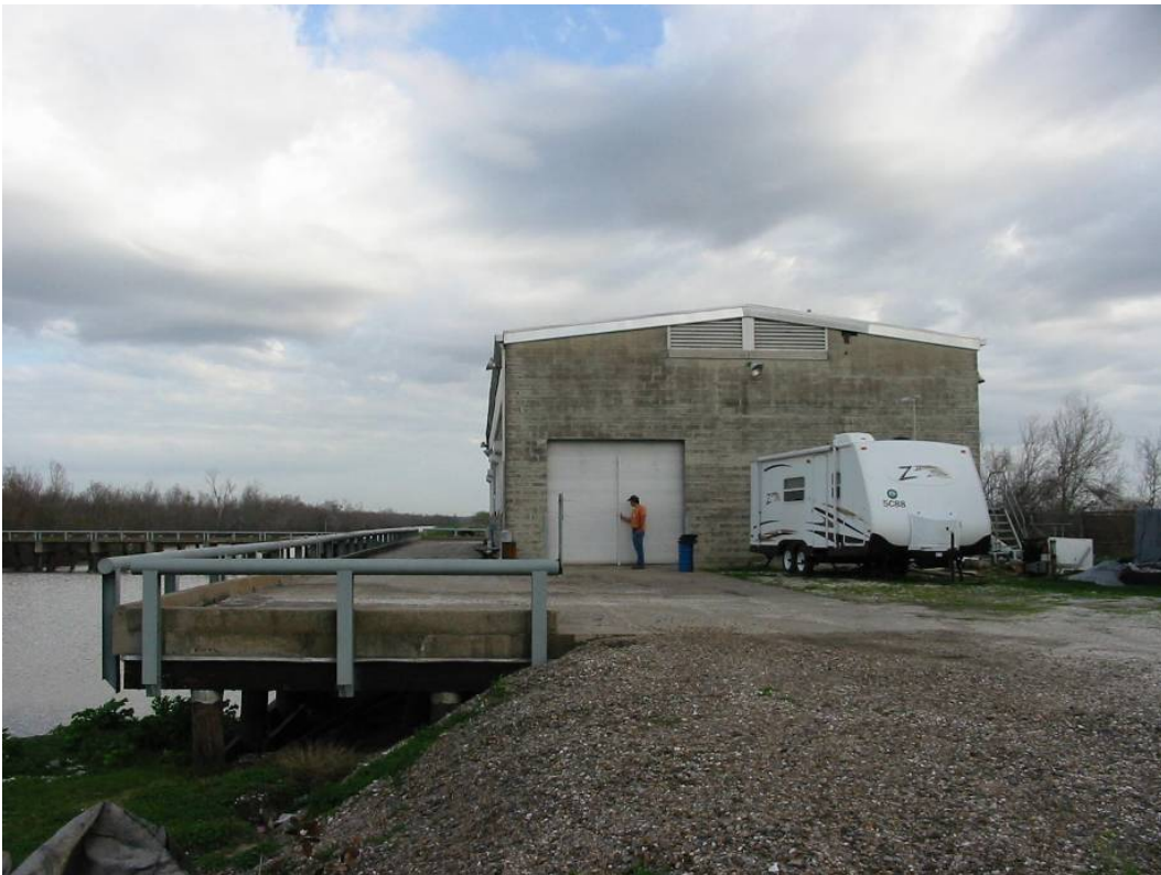
Finished Floor = 11.08 feet NAVD88(2004.65) Field Book 060852
