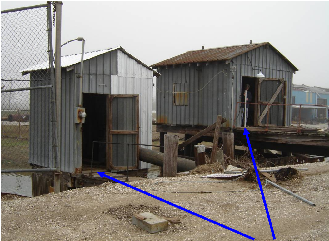
POINTE A LA HACHE PUMP STATION WEST 1 & 2
