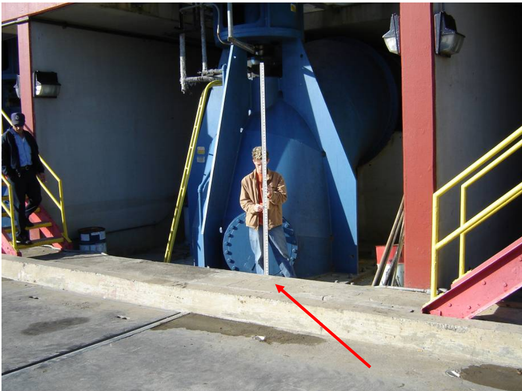
Finished Floor = -4.26 feet NAVD88(2004.65) Field Book 060852
