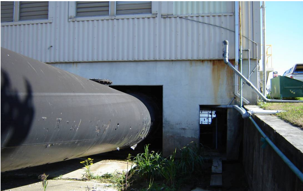
Ames Pump Station
