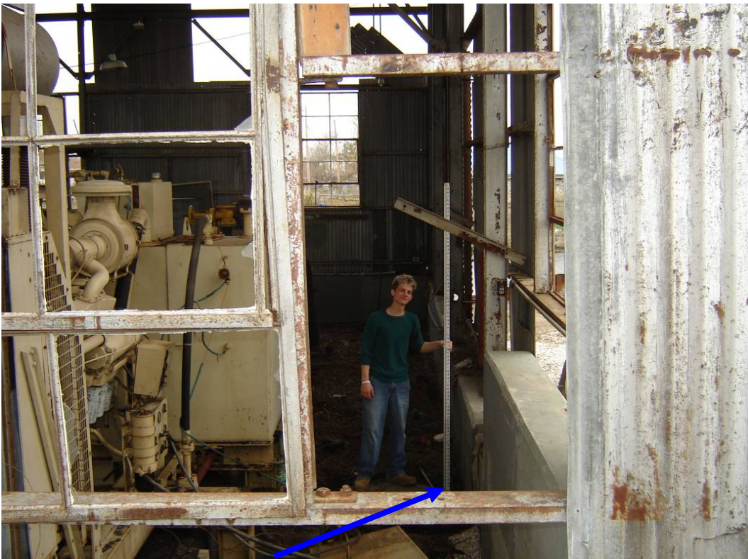
Finished Floor = 1.91 feet NAVD88(2004.65) Field Book 060851
