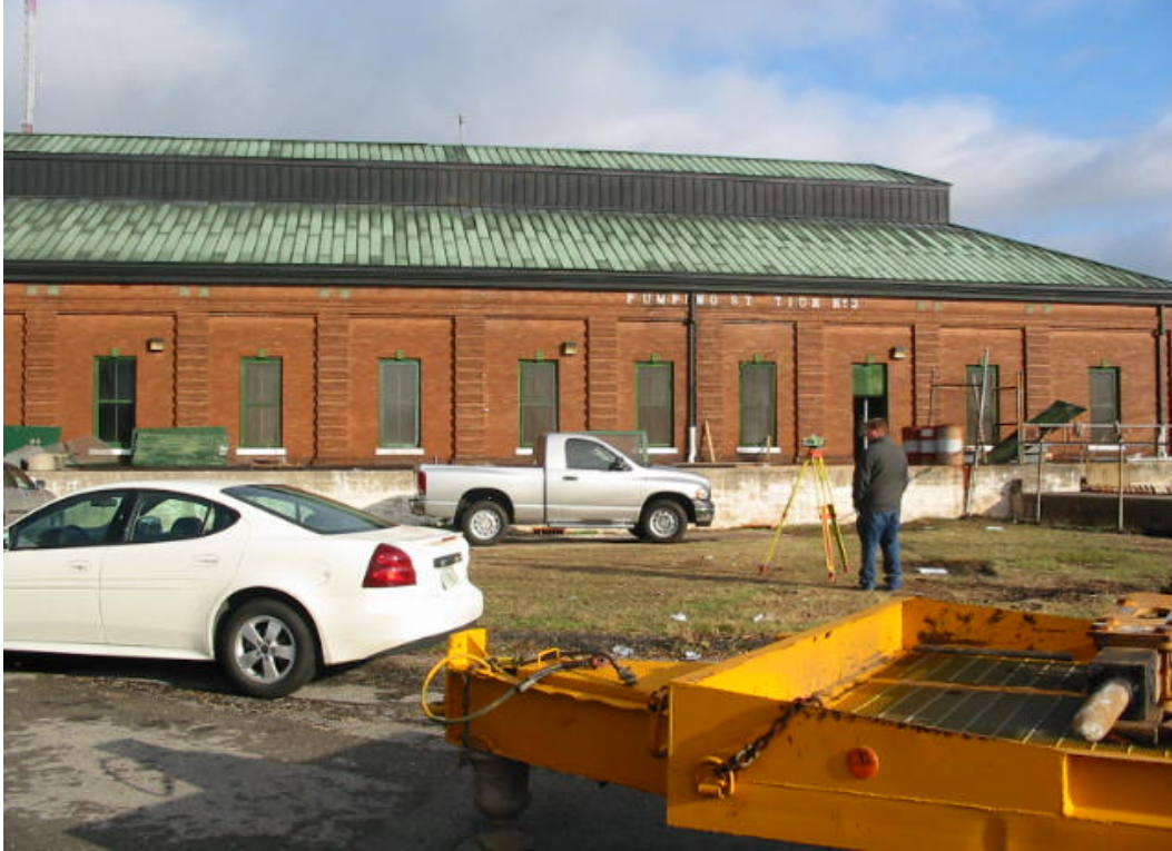
OP #3 Pump Station
