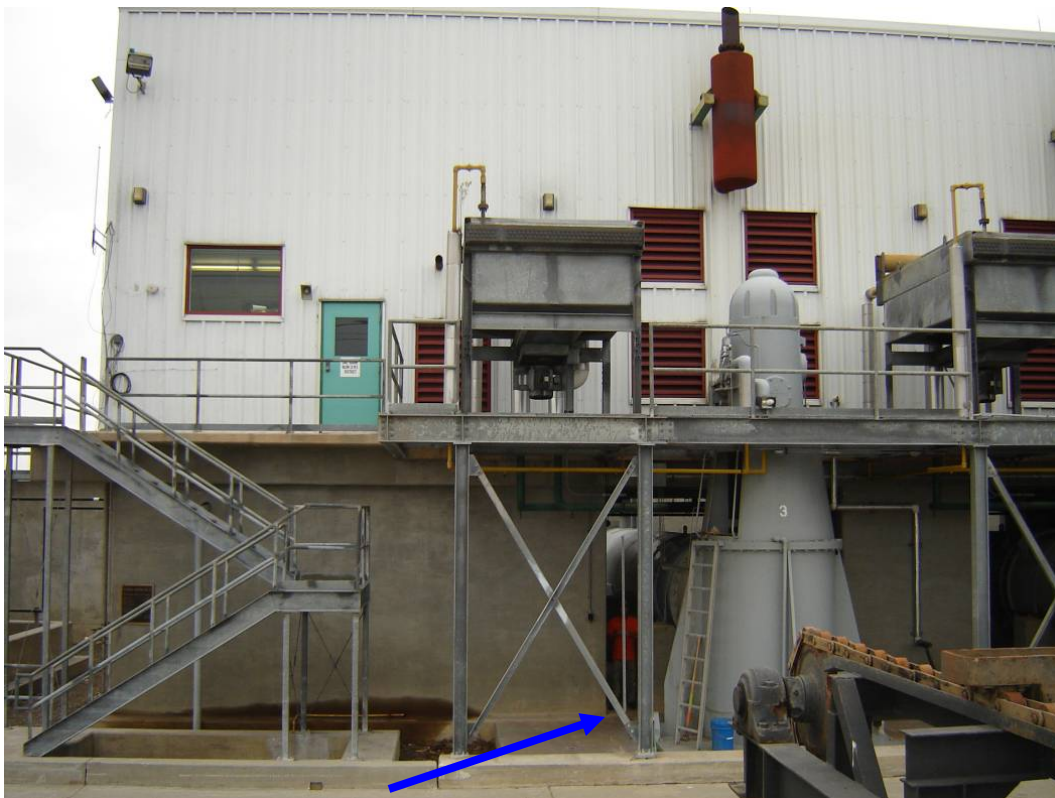
Finished Floor #2 = 2.50 feet NAVD88(2004.65) Field Book 060851
