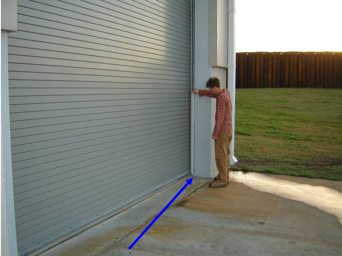
Finished Floor = -2.20 feet NAVD88(2004.65) Book # 060852
