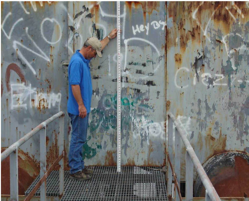
Finished Floor = 1.56 feet NAVD88(2004.65) Field book 060851
