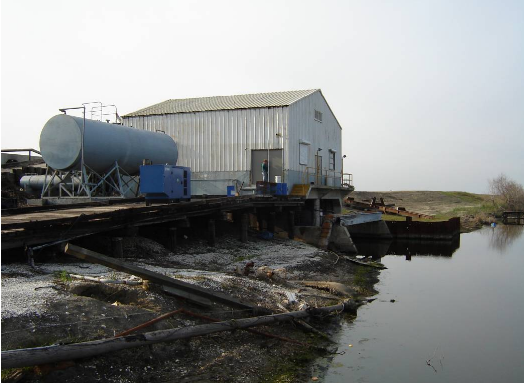
HAYES PUMP STATION
