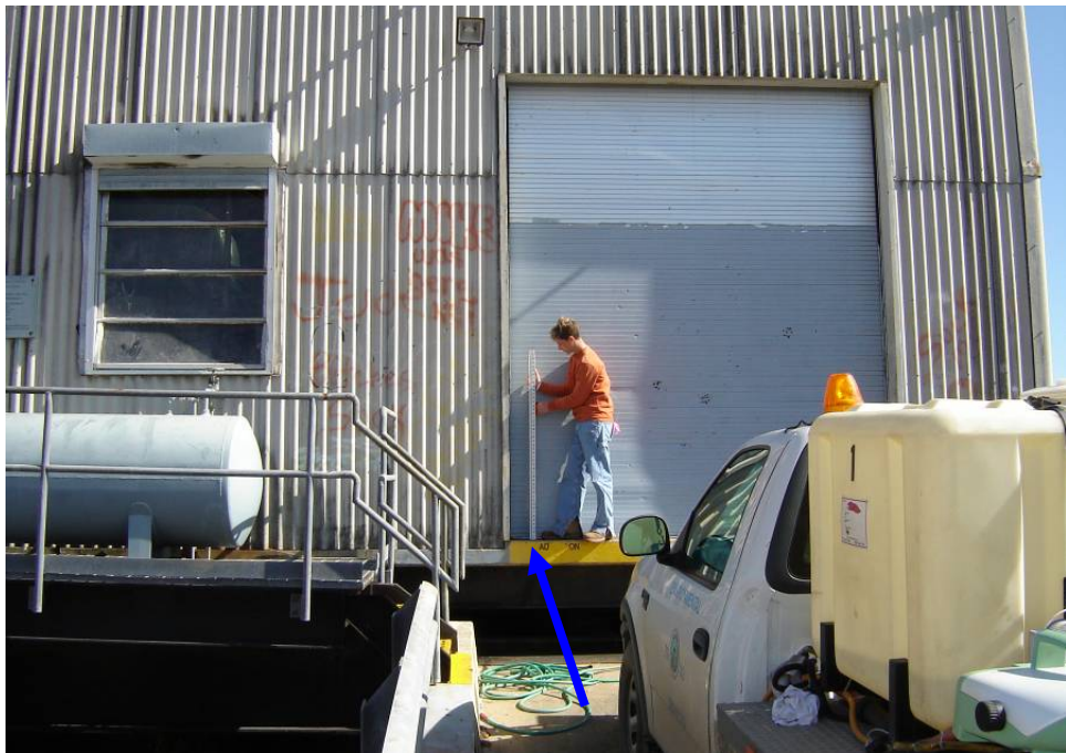
Finished Floor #3 = 17.11 feet NAVD88(2004.65) Field Book 060854
