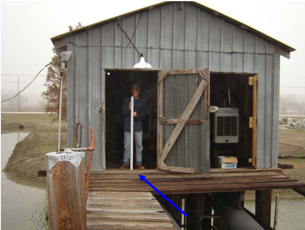
Finished Floor #2 = 6.82 feet NAVD88(2004.65) Field Book 060854
