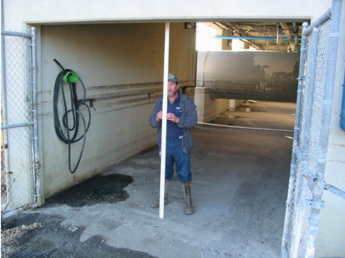
Finished Floor = 1.24 feet NAVD88(2004.65) Field Book 060851
