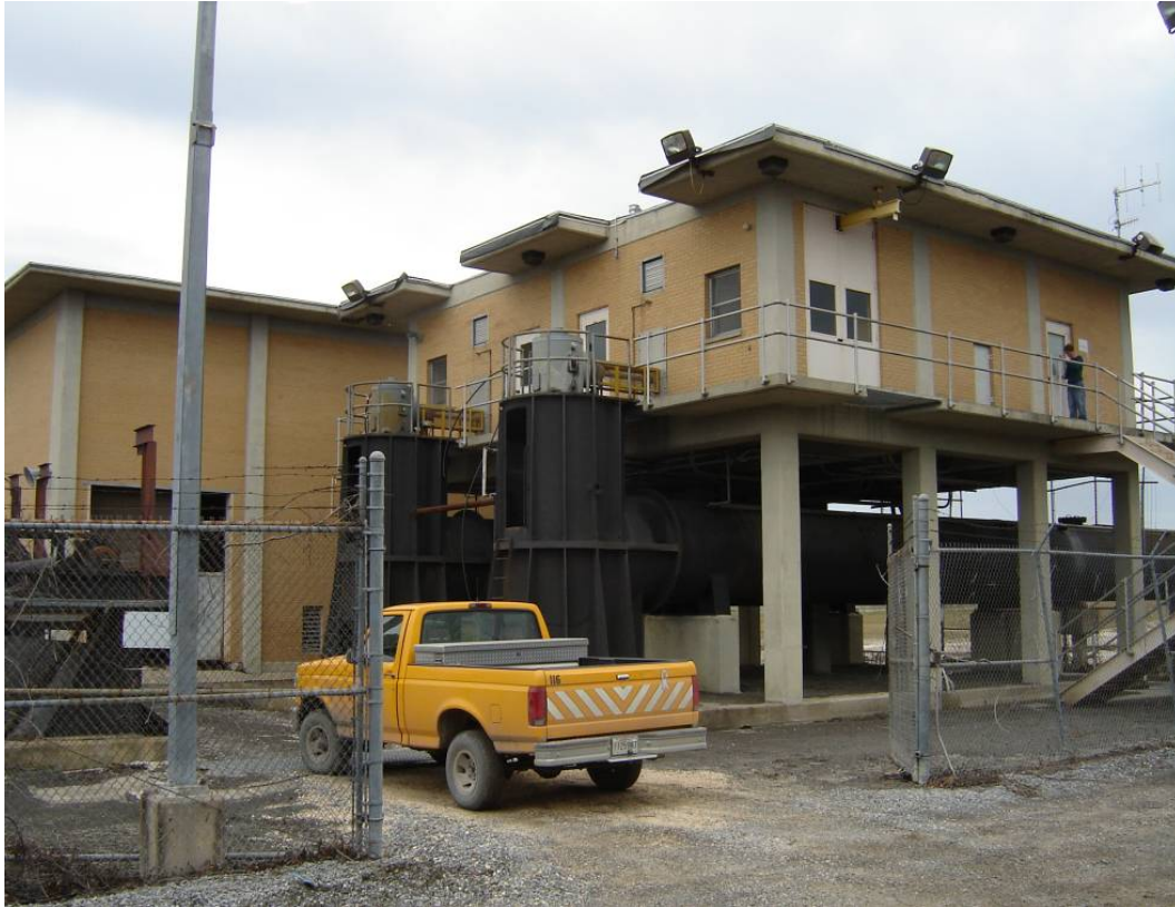
OP 20 Amid Pump Station
