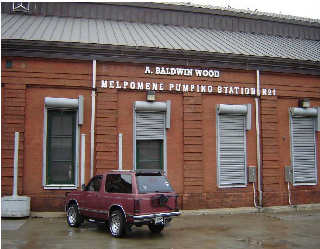
OP #1 Melpomene Pump Station #1
