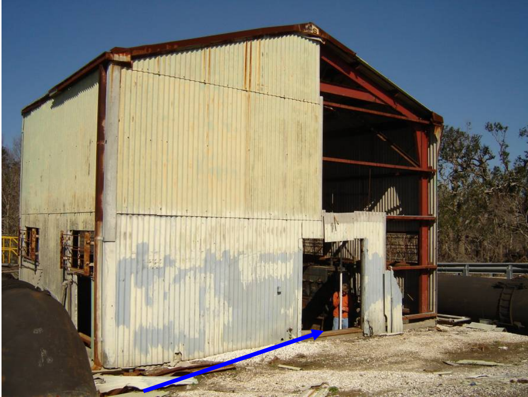
Finished Floor #2 = -0.38 feet NAVD88(2004.65) Field Book 060854
