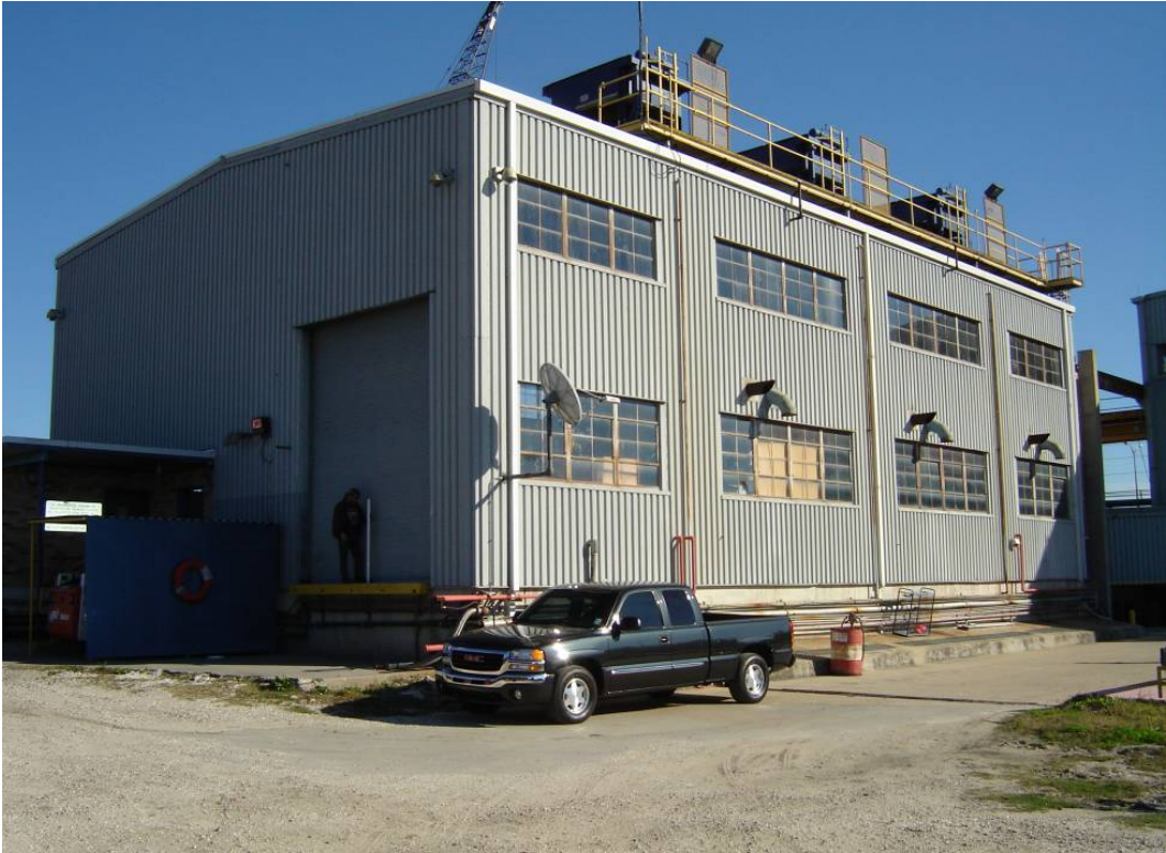
Cousins #1 Pump Station
