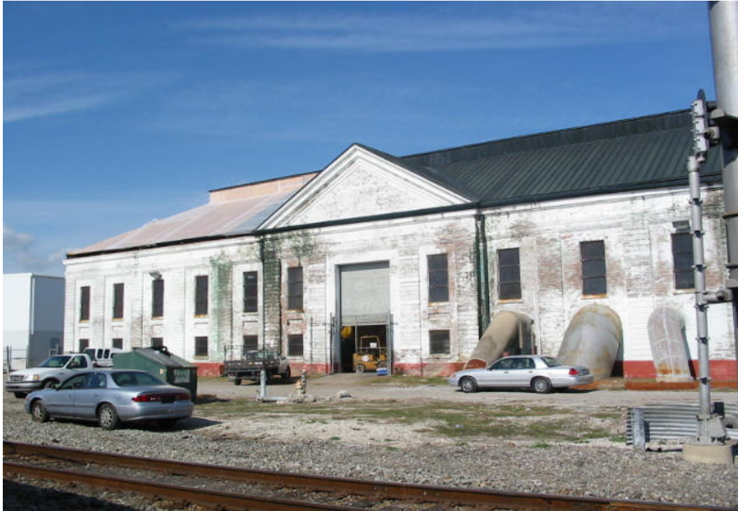
OP 17 Pump Station
