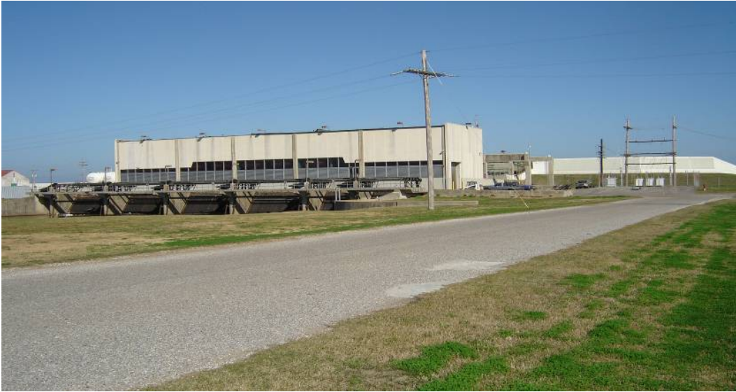
Pump Station JP-04
