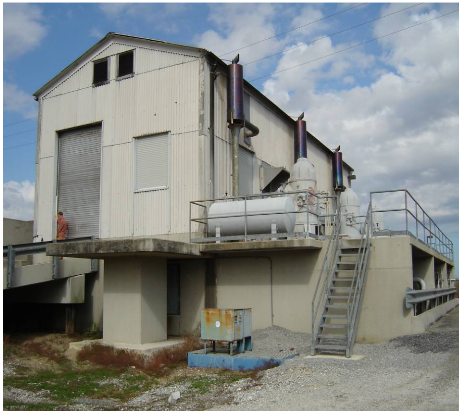
Belle Chase #2 Pump Station
