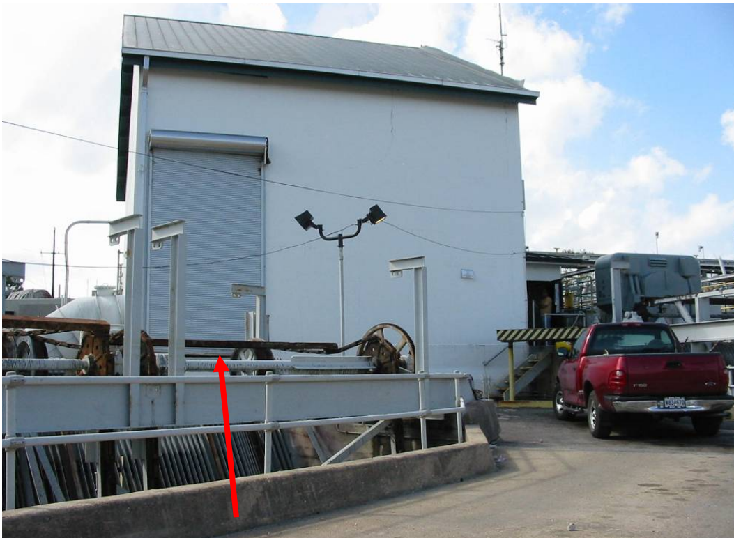
Finished Floor = 2.53 feet NAVD88(2004.65) Field Book 060851
