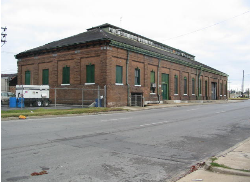
OP #2 Pump Station
