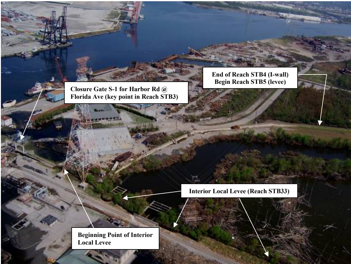
Figure 6-23. Area Showing Beginning of Interior Local Levee @ IHNC
