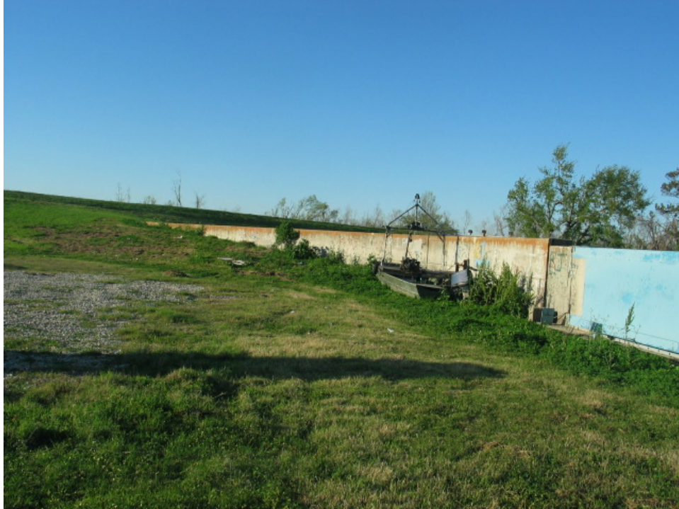
Figure 6-19. Caernarvon Canal Floodwall Tie-in to Higher MRL (Gate is for Highway 39 closure)
