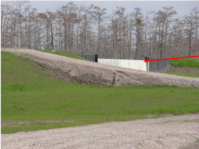
Pipeline crossing (ramp)
