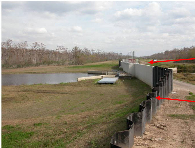
Cross Bayou Drainage Structure
