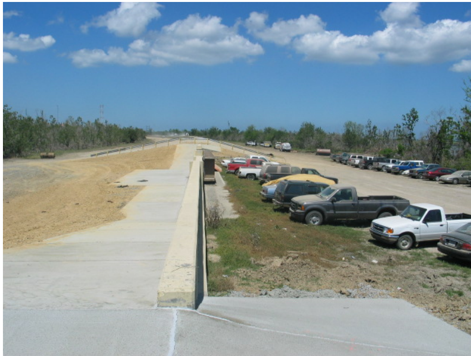
Figure 6-33. New Scour Protection Around Reach STB10 (Viewed from Bienvenue Control Structure side looking northwest)
