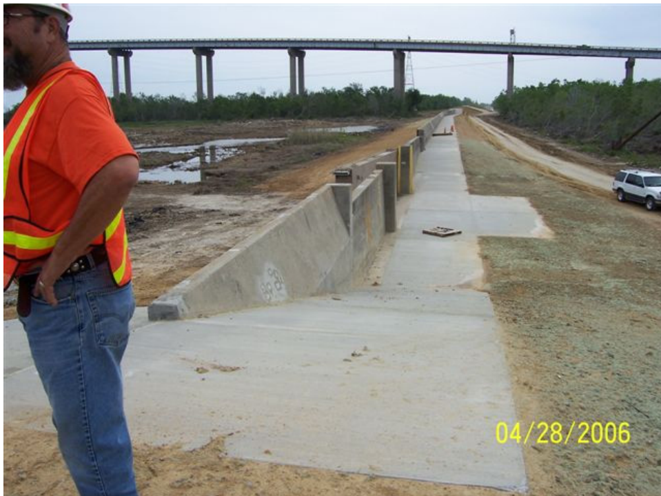
Figure 6-32. TFG Repairs to Paris Road Floodwall
