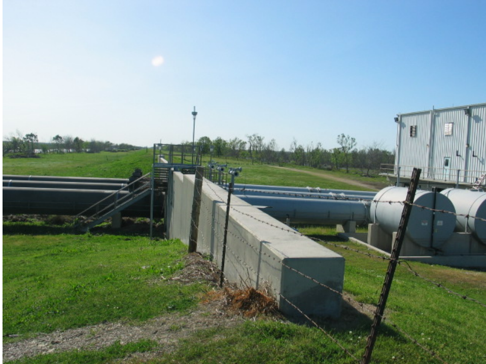
Figure 6-17. Floodwalls Surrounding Pump Station #8 Pipes (Viewed Looking West Along Caernarvon Canal)
