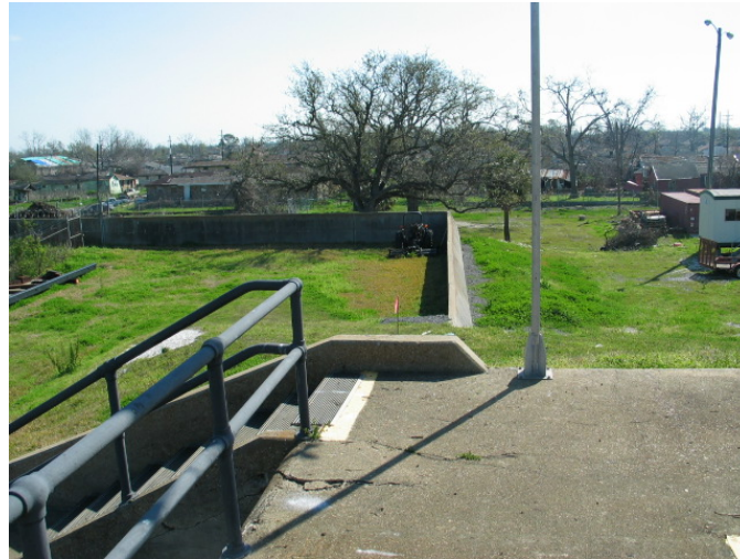
Figure 6-3. I-wall Section Tying into IHNC Lock Wall (Standing on top of lock wall and looking away from IHNC)
