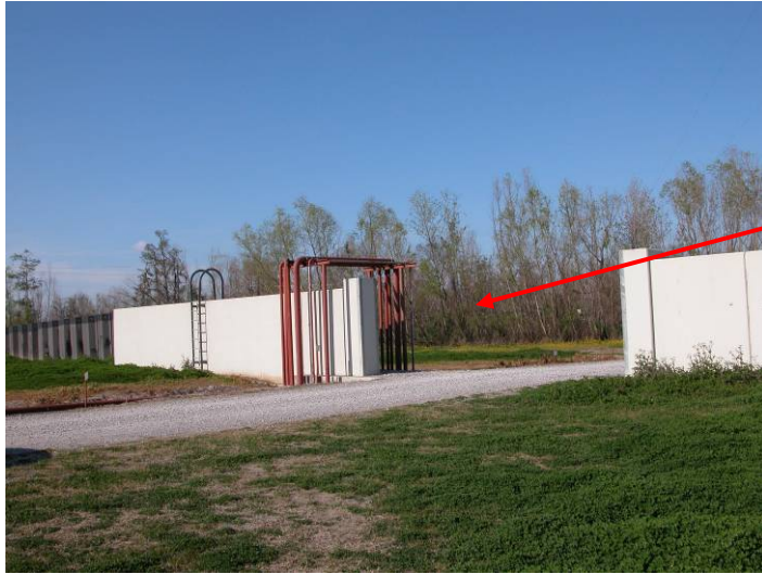
Closure Gate for Industrial plant
