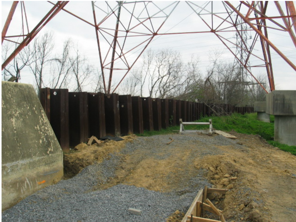
Figure 6-24. Close-up of Beginning of Interior Local Levee
