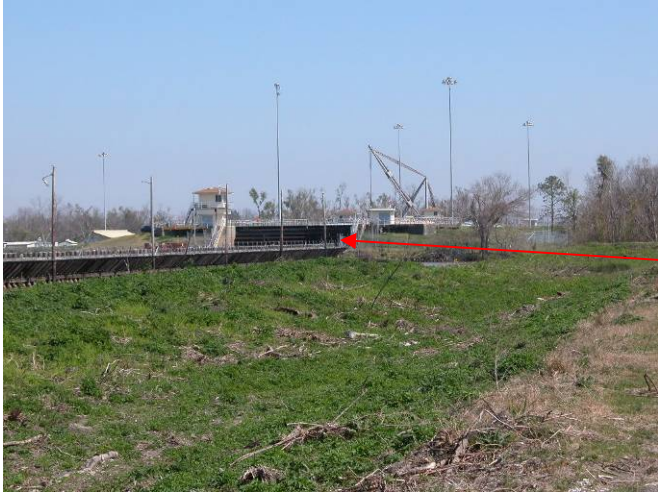
South end of Algiers Lock
