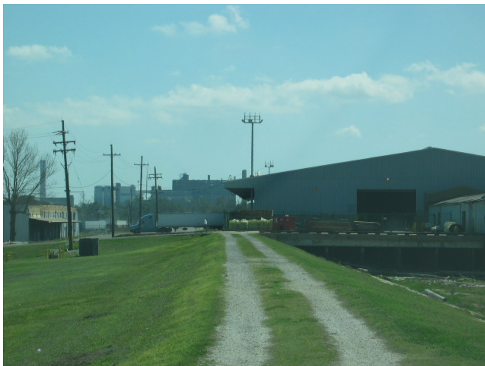
Figure 6-22. End Reach STB31 Where Levee Ties into Dock Facility (Viewed from Reach STB30 side)
