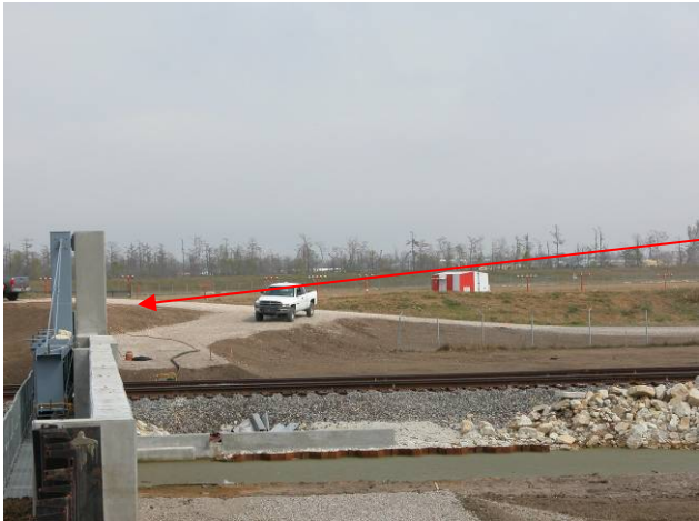
Railway Gated Crossing at Airport Levee (not constructed during Katrina )
