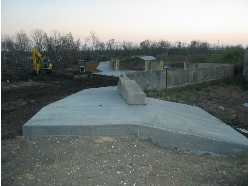
Figure 6-31. New Scour Protection Around Reach STB6
