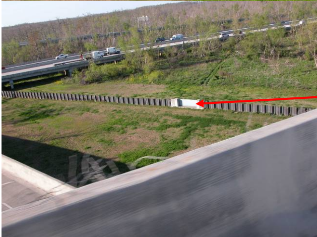
I 310 Floodwall with 24 ft closure gate
