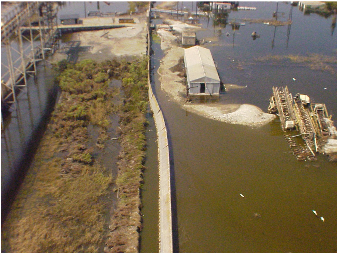
Figure 2-10. Floodwall Failure at Bulk Loading Facility/Elaine PS
