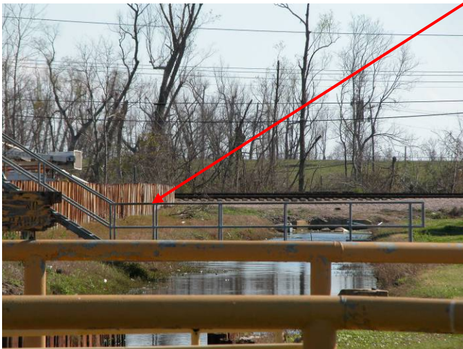
St. Charles – Jefferson Levee at South side of US 61
