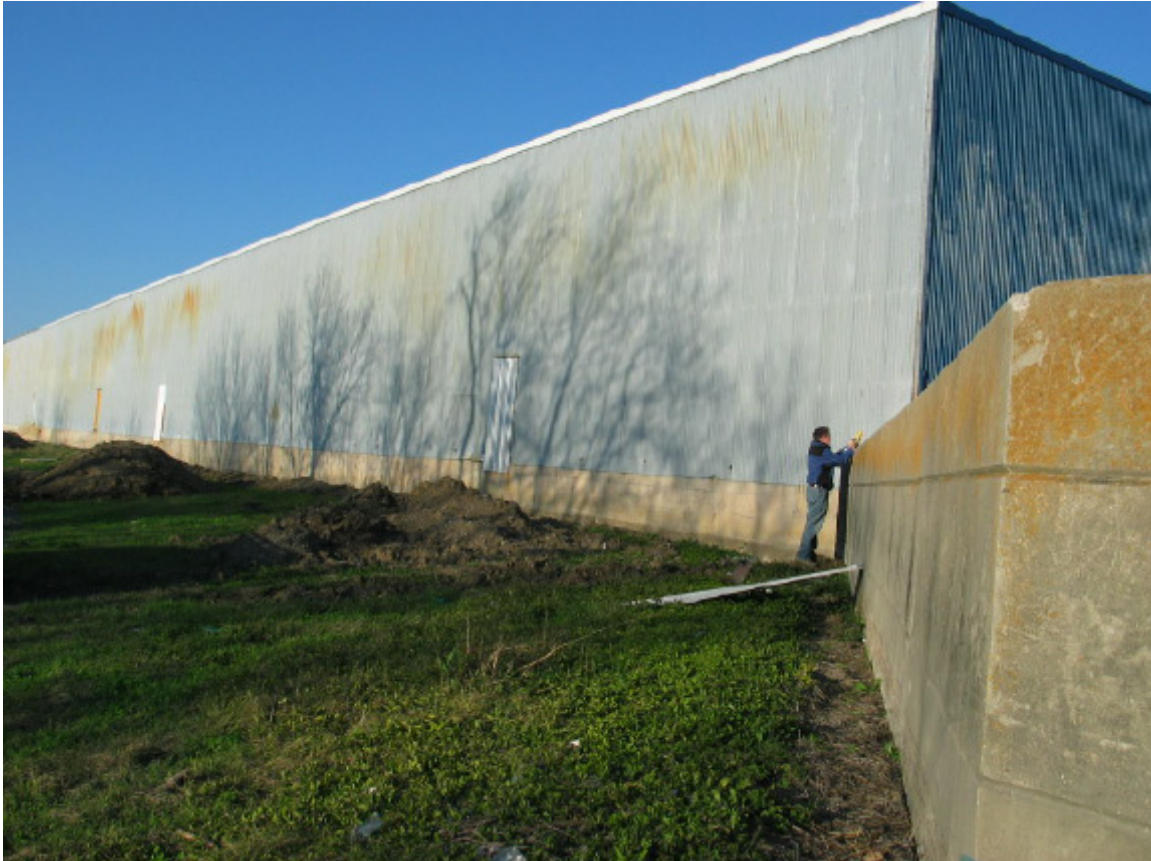
Figure 2-13. Floodwall Serves as Building Foundation (Dupuy Storage Facility – IHNC East)
