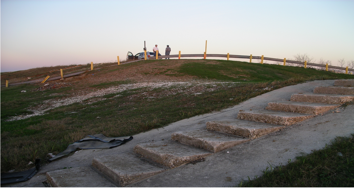
Figure 2-5. Begin Lakefront Levee at Citrus Lakefront and Paris Road (Lakefront Levee @ El. 19.0 +/- and Citrus Lakefront Levee @ 13.5+/-)
