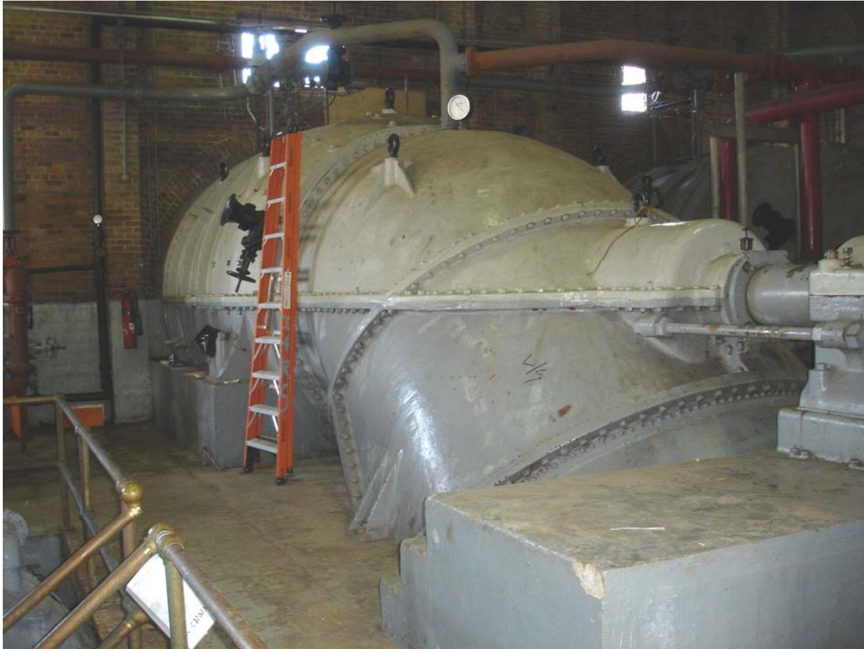
Figure 7. Large Horizontal Shaft Pump
