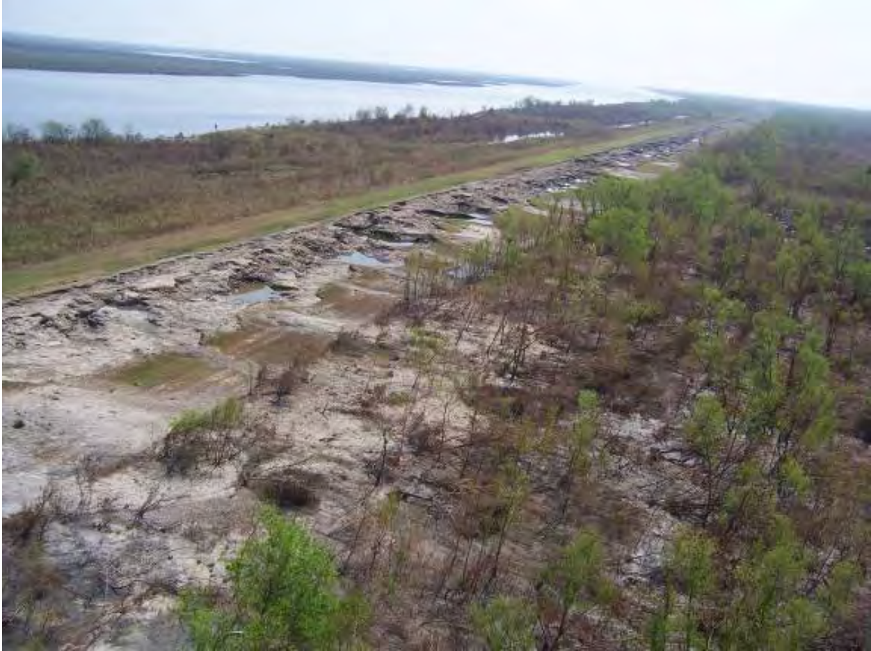
Figure 14-145. Scour Depths Below the Original Levee Footprint
