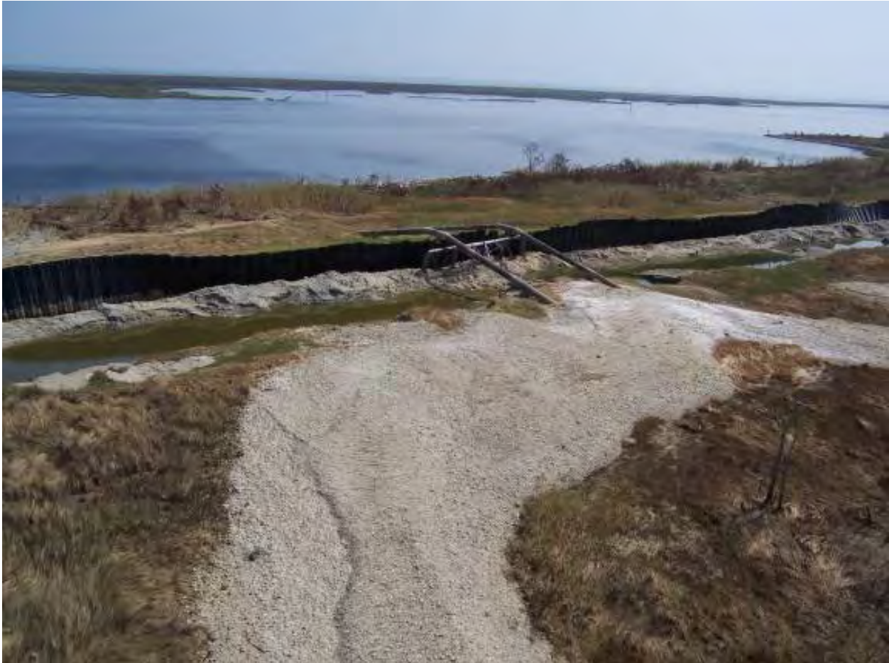
Figure 14-121. Damaged Sheetpile Section (Utility Crossing), With Scour on the Protected Side. B/L Sta 590+70 is centerline of the two pipelines
