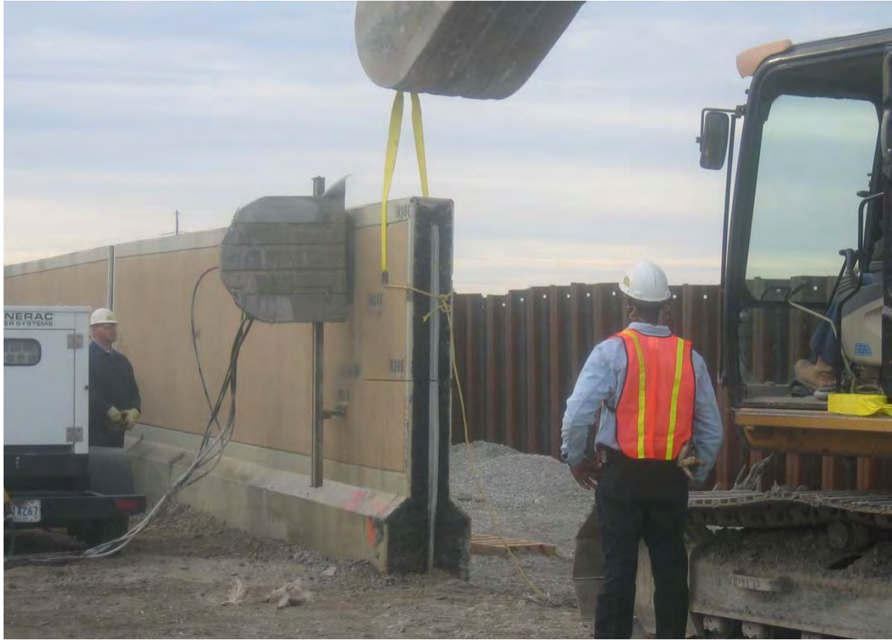
Figure 15-6. Sawing of Sample from Wall Panel H38
