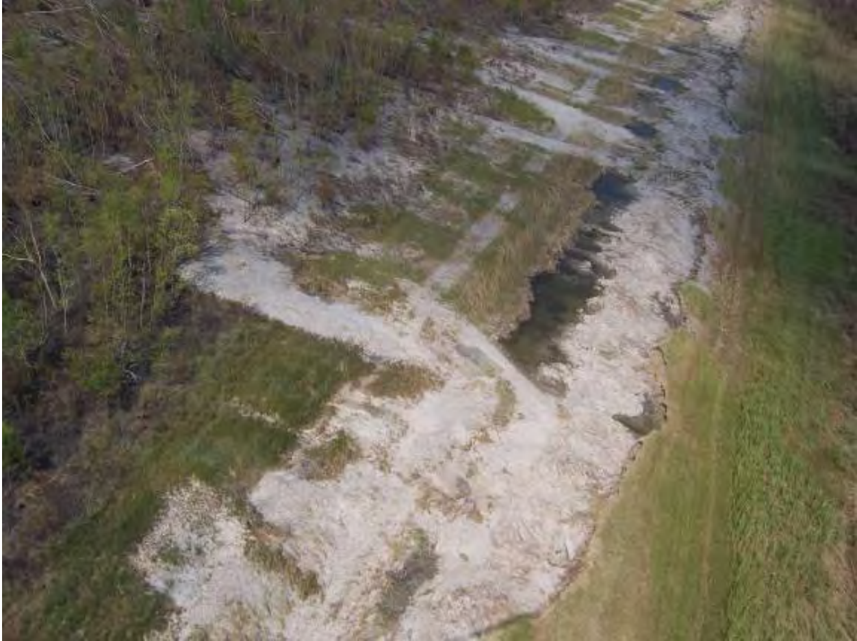
Figure 14-117. More Missing Levee
