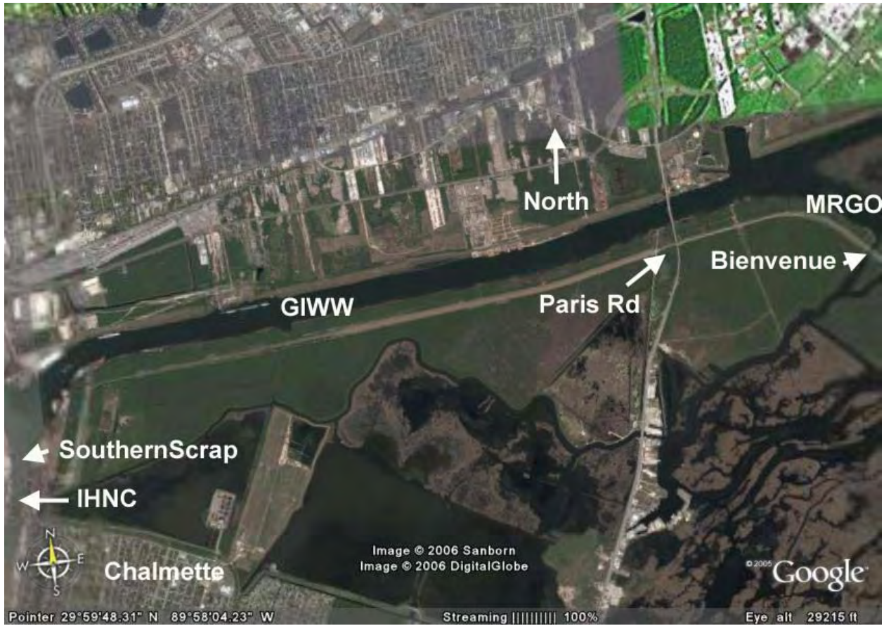
Figure 14-82. Photo of St. Bernard and Orleans Parish Levee System From IHNC East (north of Florida Ave.) to Bayou Bienvenue
