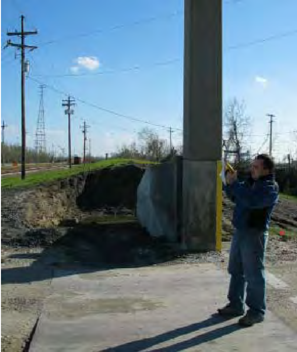
Figure 13-75. IHNC Floodgate E5 Transition to Levee
