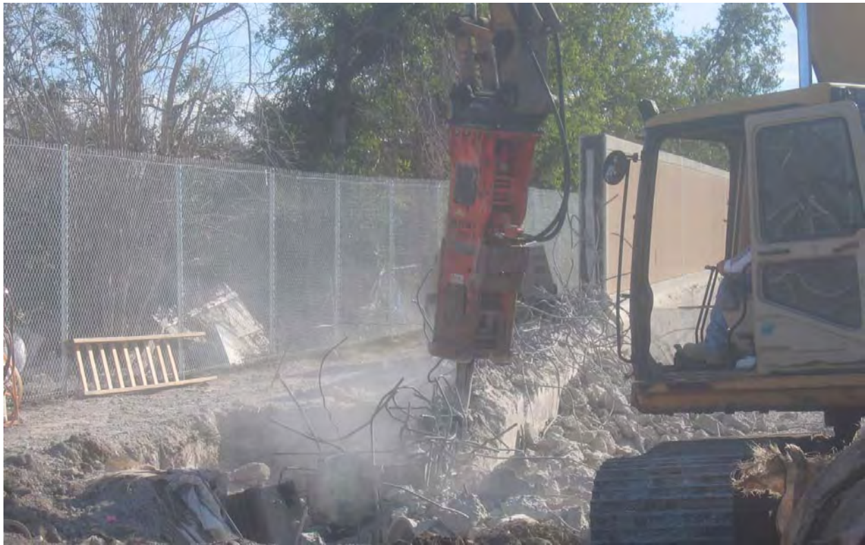
Figure 15-18. Hoe Ram Demolishing Lower Portion of Wall Panel H38
