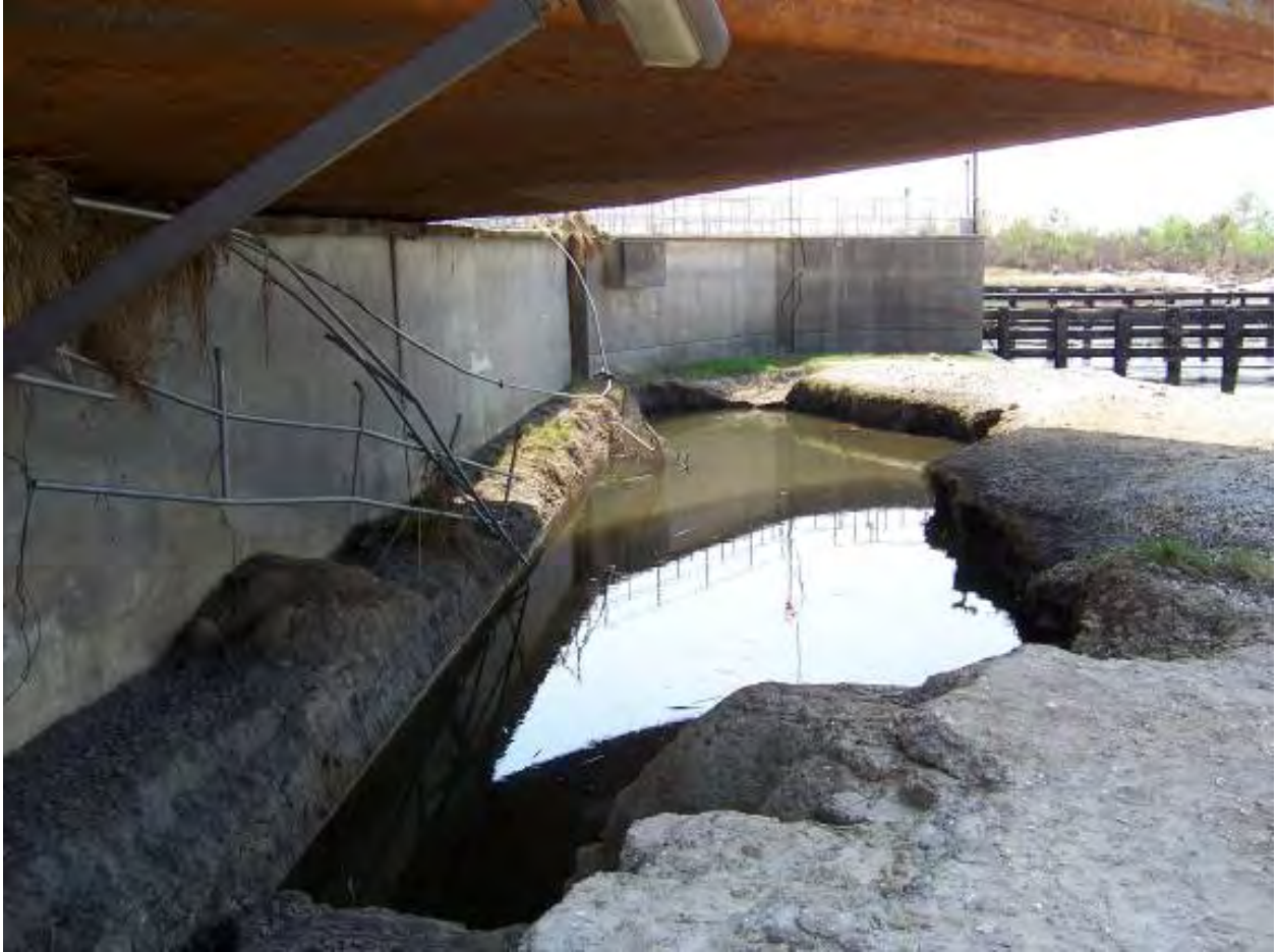
Figure 14-110. Barge Resting on T-Wall
