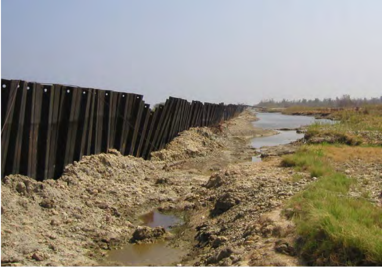
Figure 14-123. Note Sheetpile Elevation Differences
