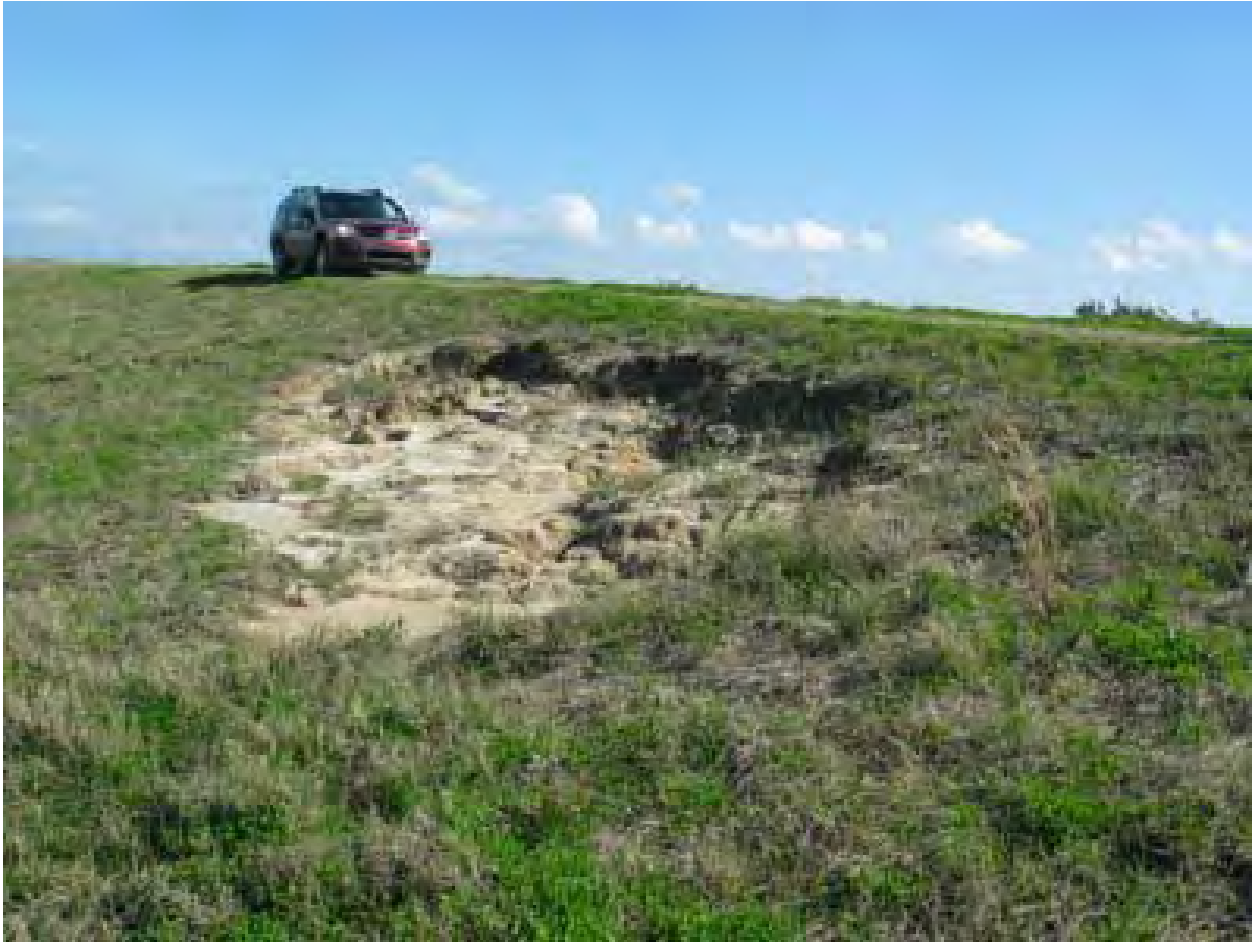
Figure 13-44. Closeup of Landside Slope Erosion at N 30deg 0 min 2.29sec W 89deg 58min 27.29sec
