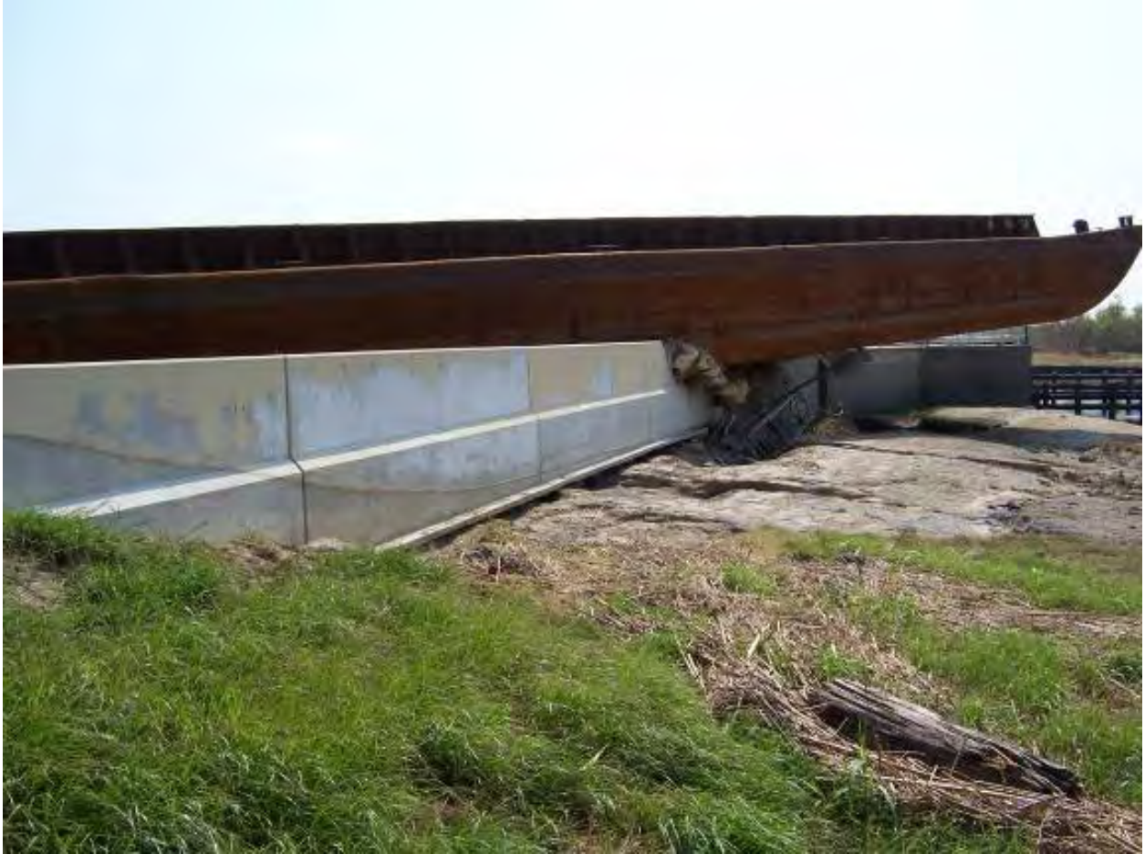
Figure 14-111. View East, From Protected Side
