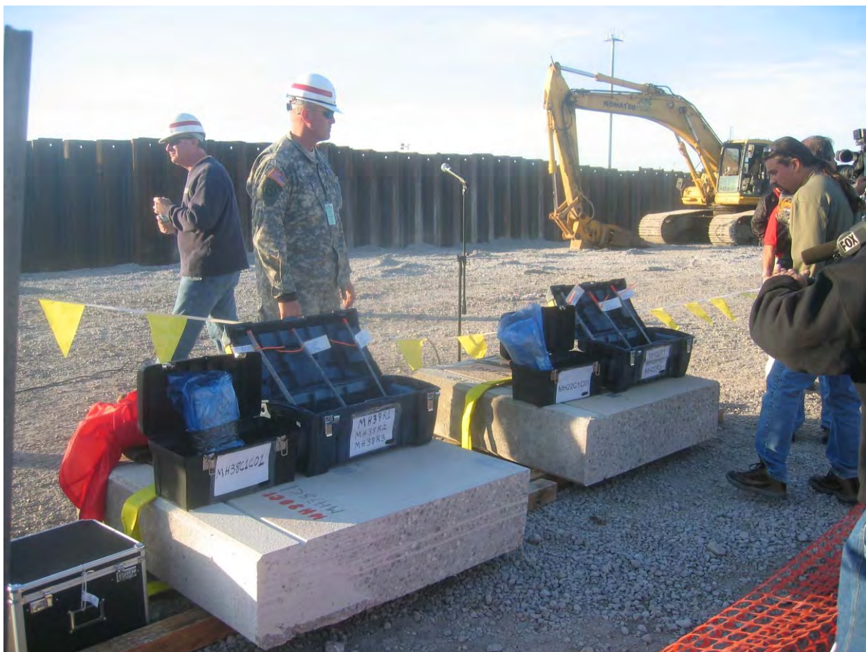
Figure 15-16. Wall Panel Samples, Cores and Rebar Samples
