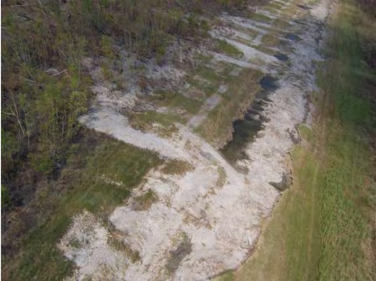
Figure 13-64. 2,300 ft. of Levee Between Bayou Bienvenue (Sta 383+00) and Bayou Dupre (Sta 704+00) That Only Lost 50% of Height
