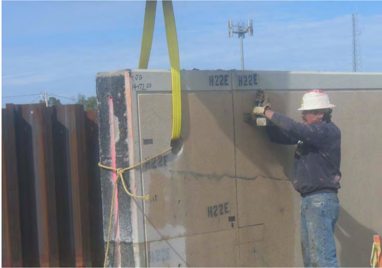
Figure 15-9. Sample Being Removed from Wall Panel H22
