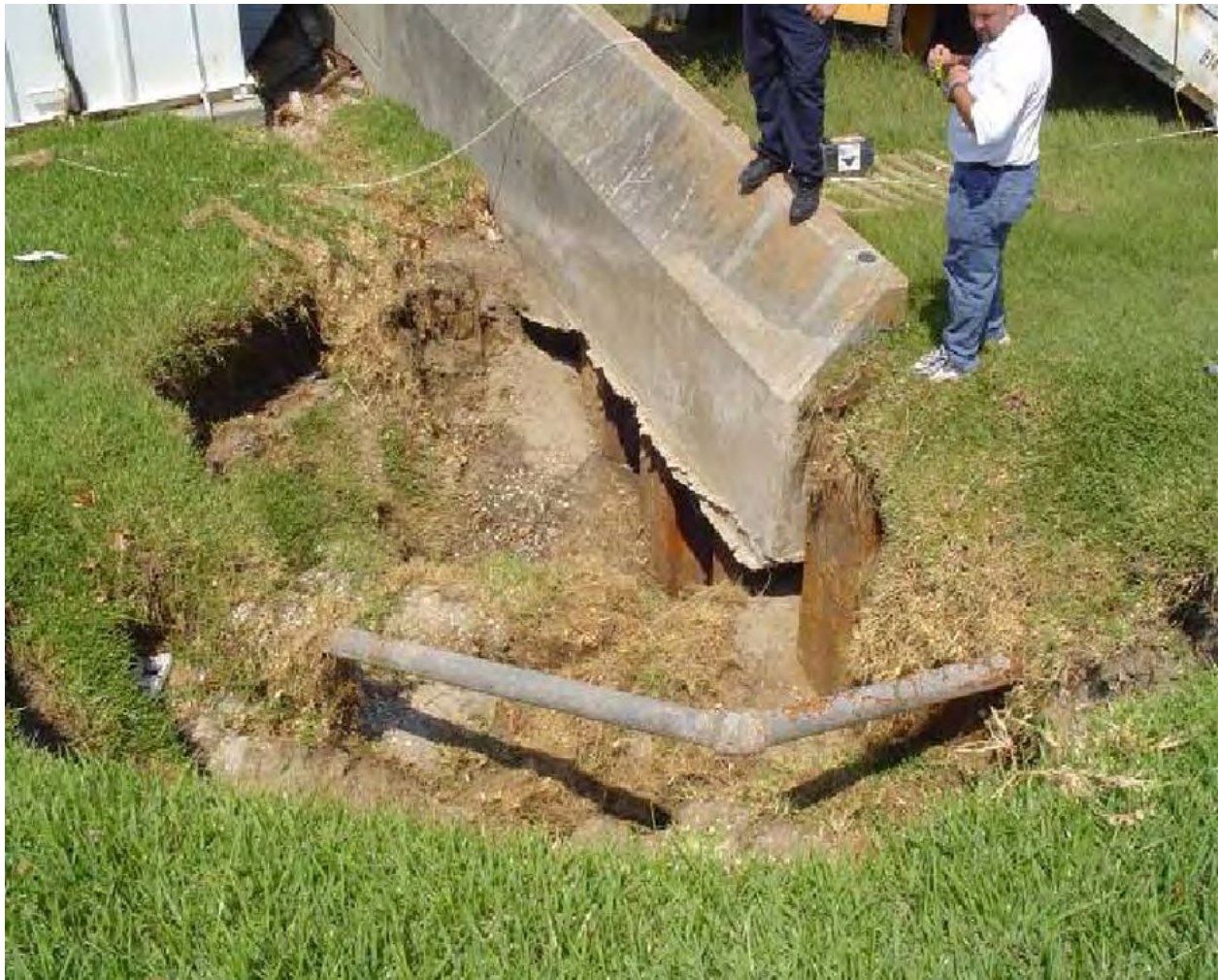
Figure 13-79. IHNC Lock I-wall transition to levee
