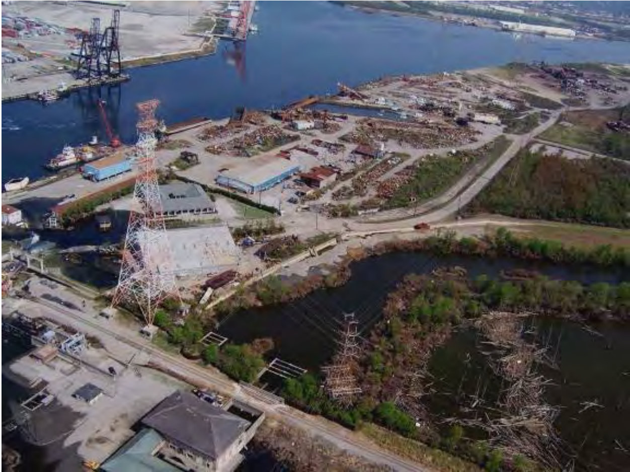
Figure 14-84. Floodwall Between Fla Ave (IHNC East) and Southern Scrap Facility
