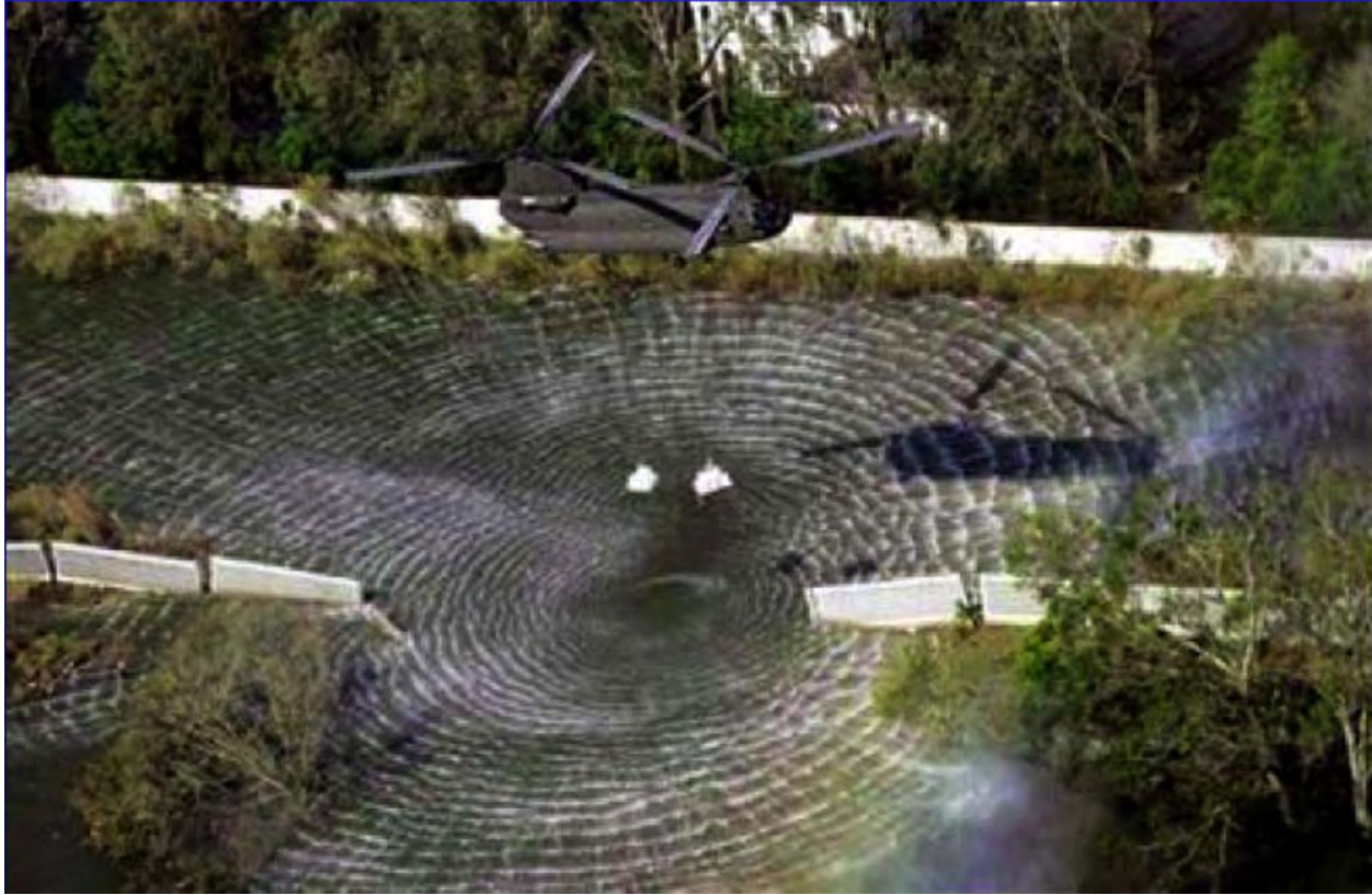
Figure 8-1. The South Breach at the London Avenue Canal Occurred at 6:00 AM to 7:00 AM on August 29, 2005. The breach, on the east side of the canal, was approximately 60 feet wide.
