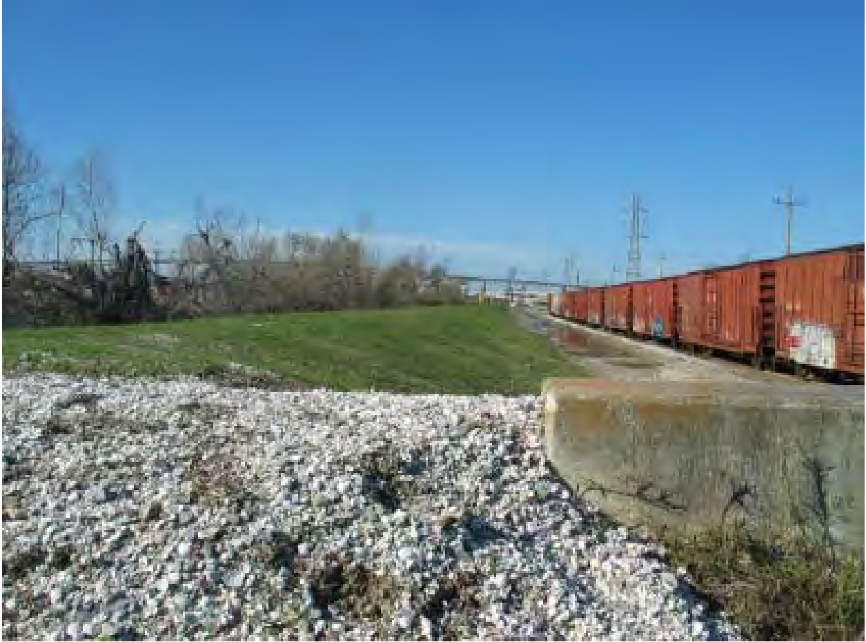
Figure 14-44. E4 Scour Repaired
