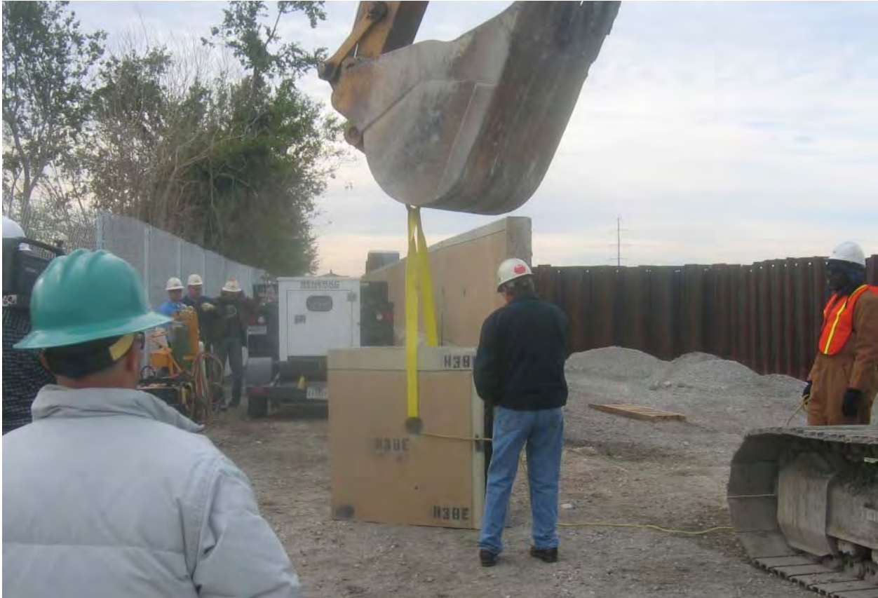
Figure 15-7. Removal of Sample from Wall Panel H38
