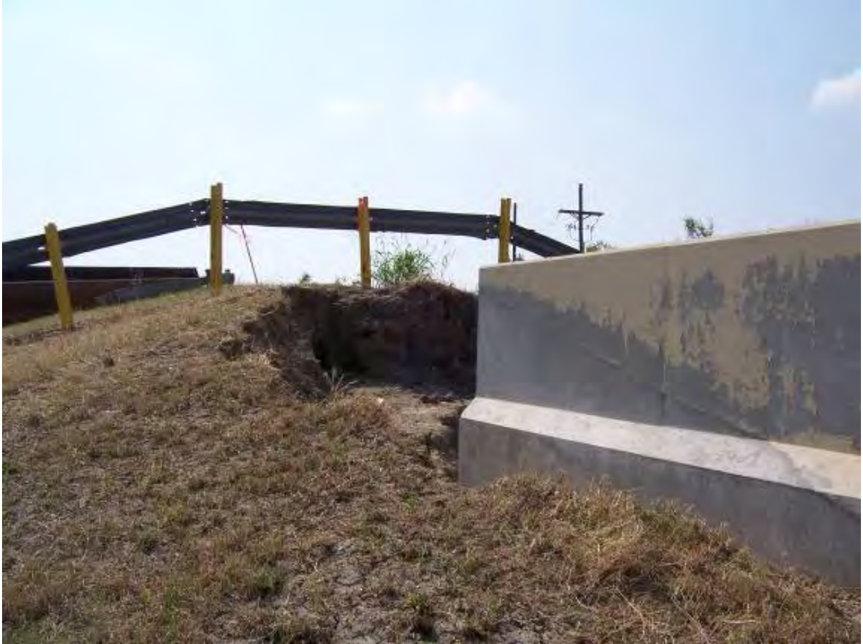
Figure 14-104. View Looking East Toward the Bayou Bienvenue Control Structure
