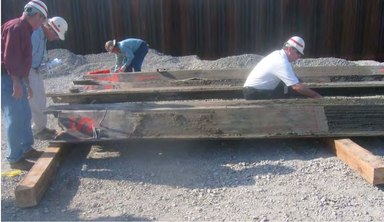
Figure 15-25. Sheet Piling Extracted from North End of Breach
