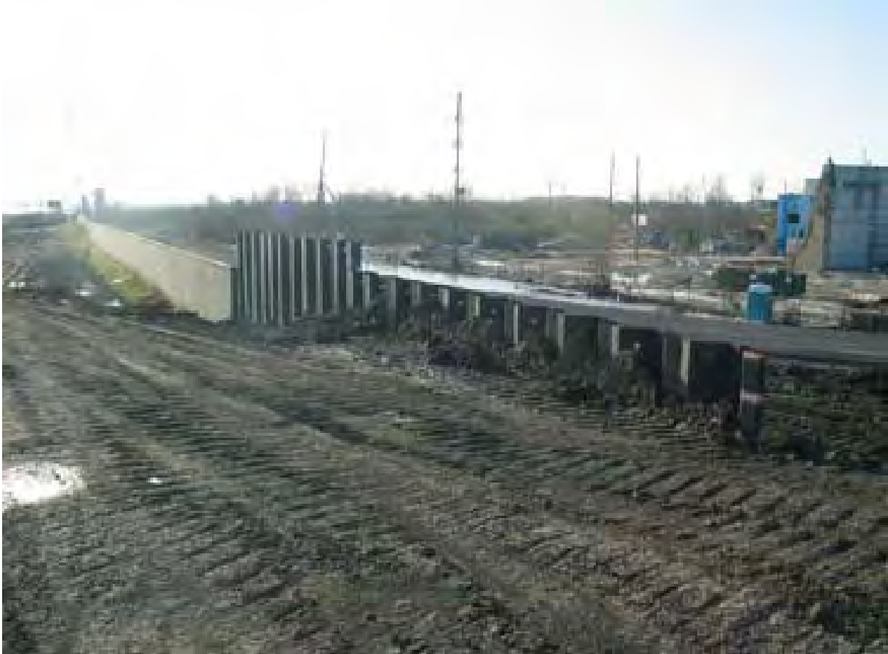
Figure 12-50. NOE3_J. Repair Sheetpile View to the West
