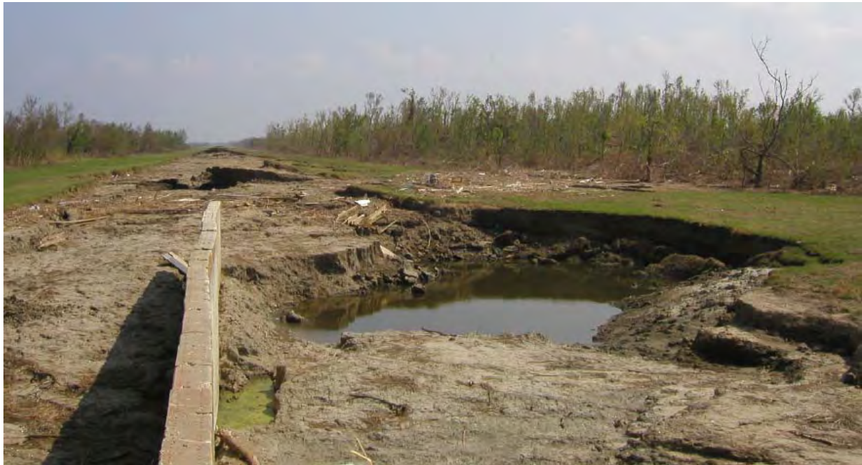
Figure 13-65. Wall / levee on the Southeast Side of Bayou Dupre Control Structure
