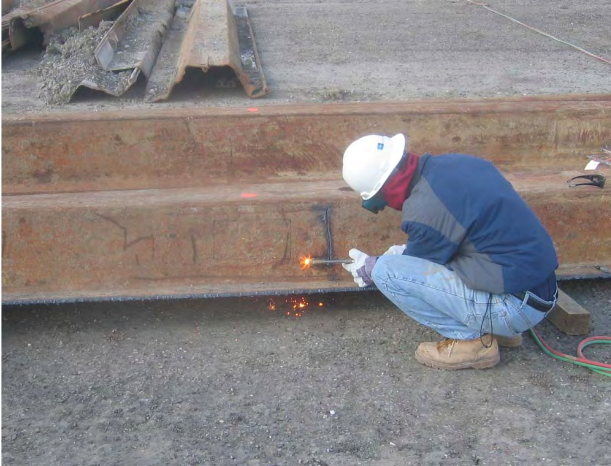
Figure 16-2. Flame Cutting of Material Samples from Piling IHNC-SP-WS-B2
