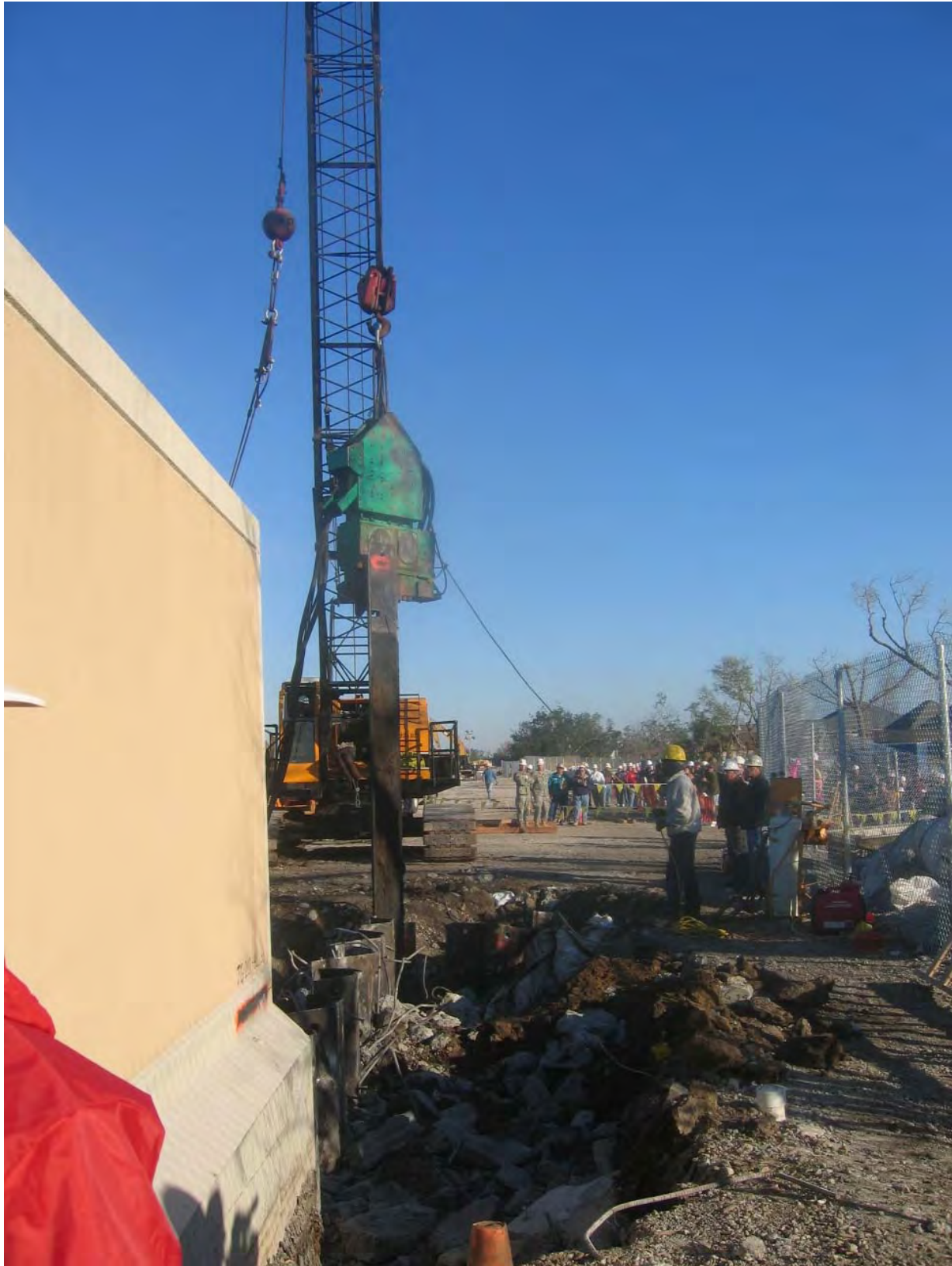
Figure 15-20. Extraction of Sheet Piles MH38SP2 and MH38SP3
