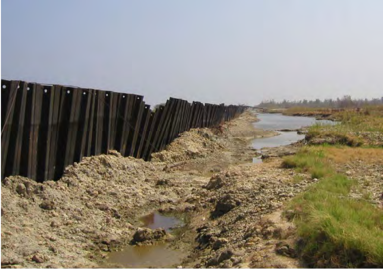
Figure 13-28. Sheetpile Between Bienvenue and Dupre Control Structures. Note the sheetpile elevation differences
