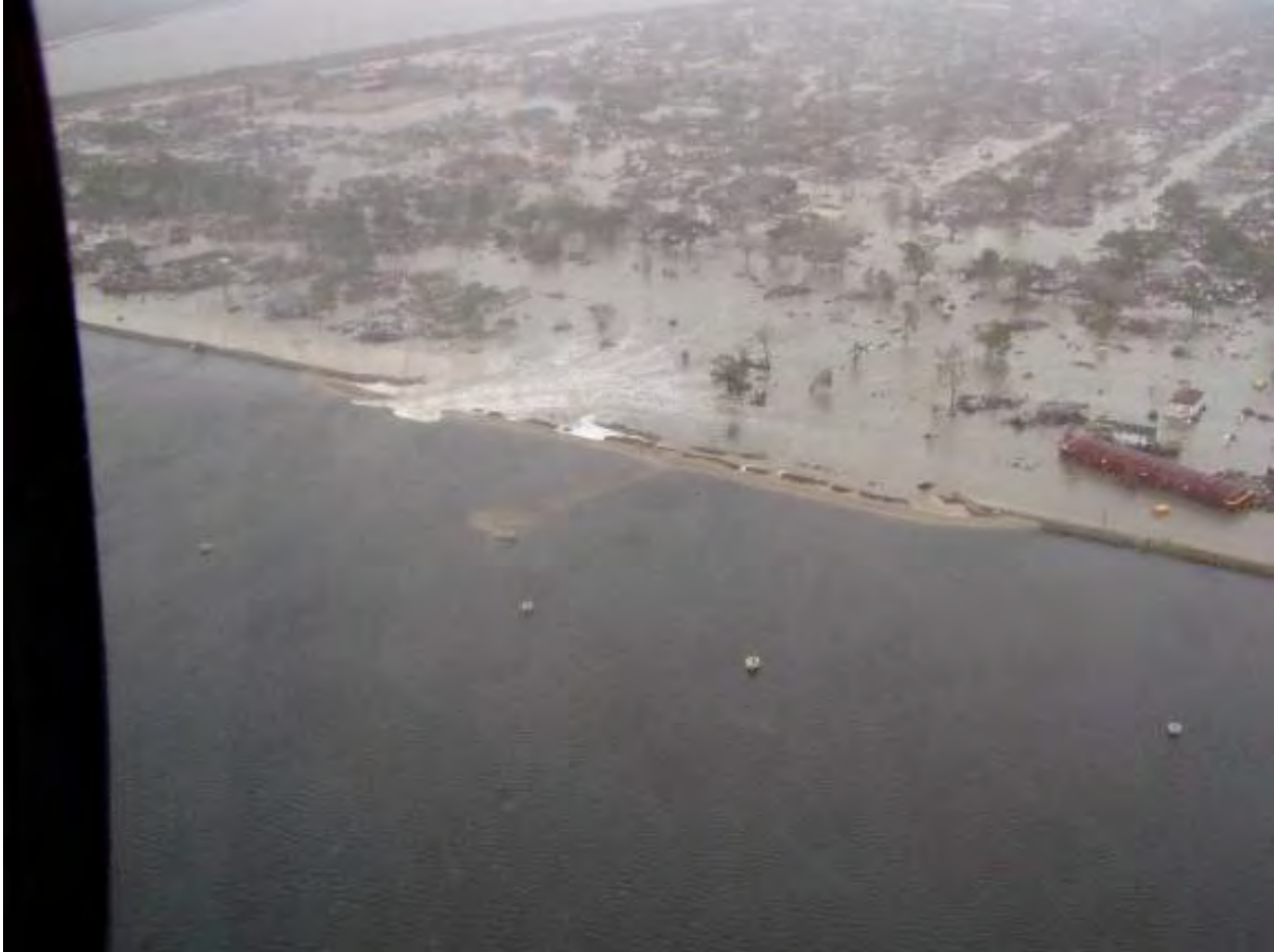
Figure 14-23. During Katrina; View to East Side of IHNC South of GIWW. Breach began approximately 300 ft north of Claiborne Ave.
