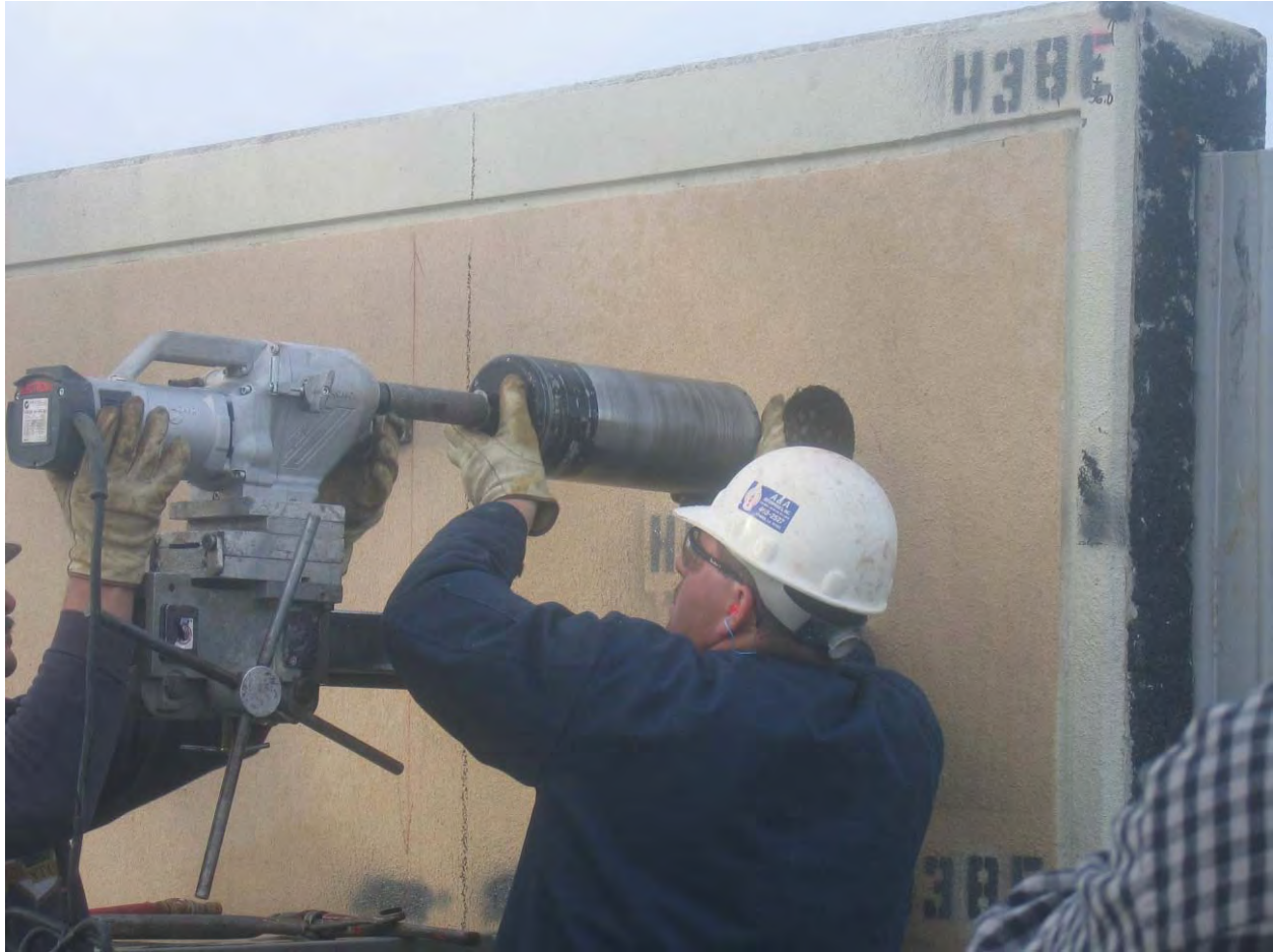
Figure 15-4. Core Being Removed from Panel H38
