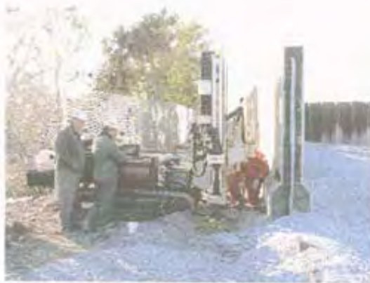
Photo 1 - Geoprobe Rig for PS/SCPT testing at South End of Breach of 17 th Street Levee at Station 17+78 where sheet piles were exposed by USACE PS Cased Borehole (white PVC cap visible)
