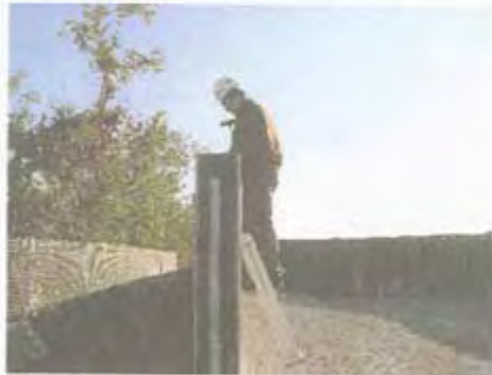
Photo 6 (Fig. 4) - Vertical downward impact to top of wall
