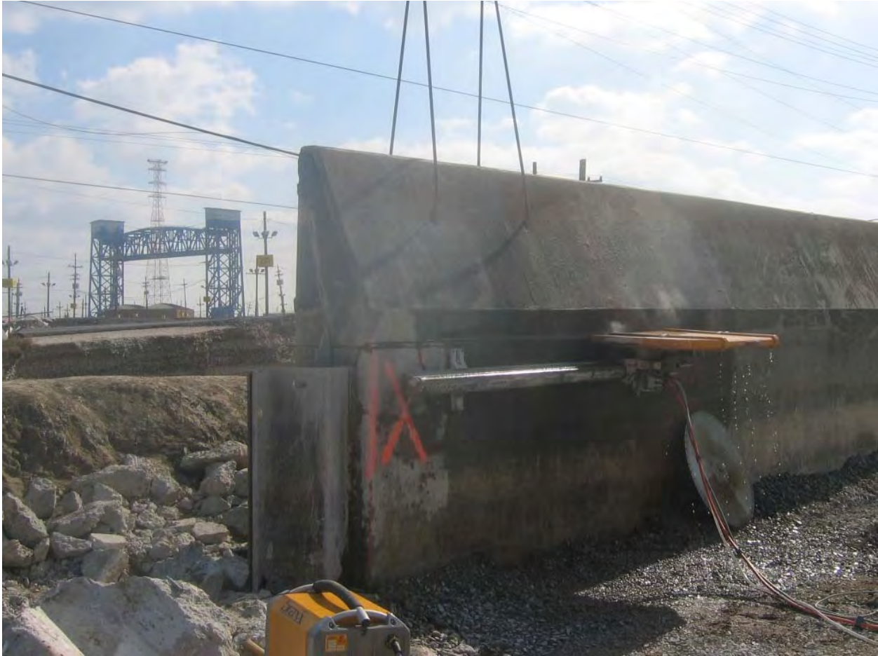
Figure 16-1. Sawcutting Concrete Wall Sample
