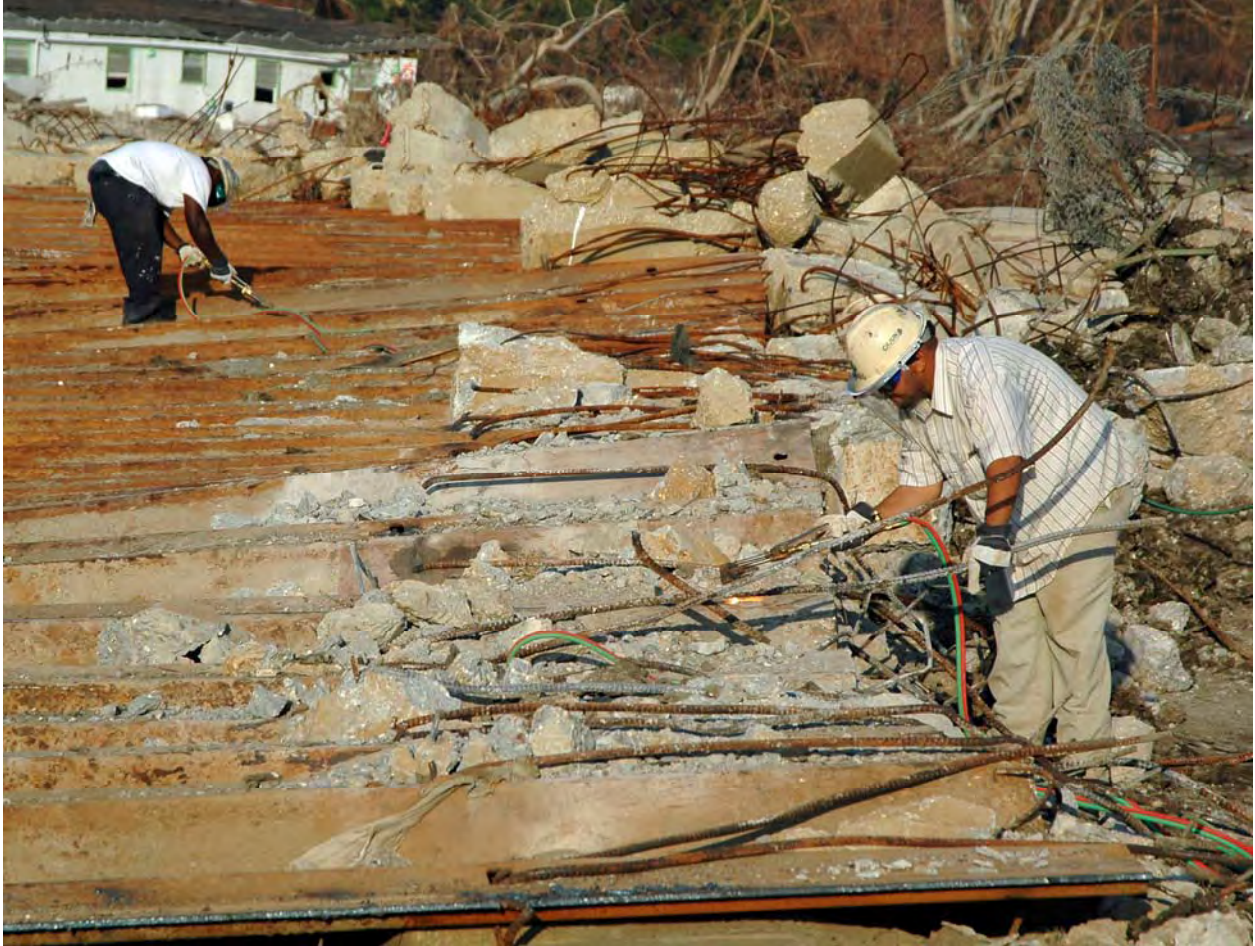
Figure 14-27. Demolishing Flattened I-Wall North of Claiborne Ave.
