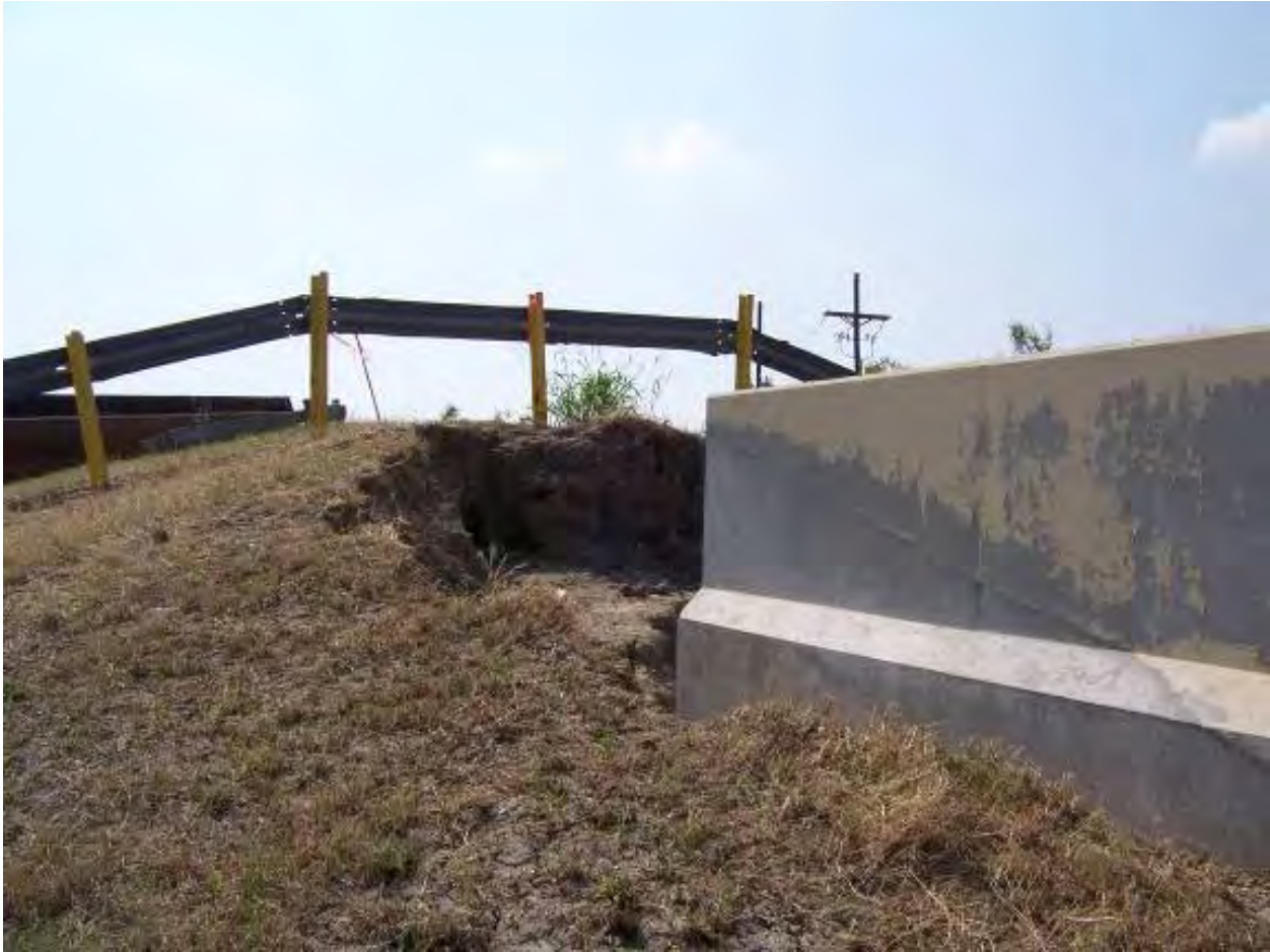
Figure 13-73. Floodgate S5 Near Bienvenue Control Structure
