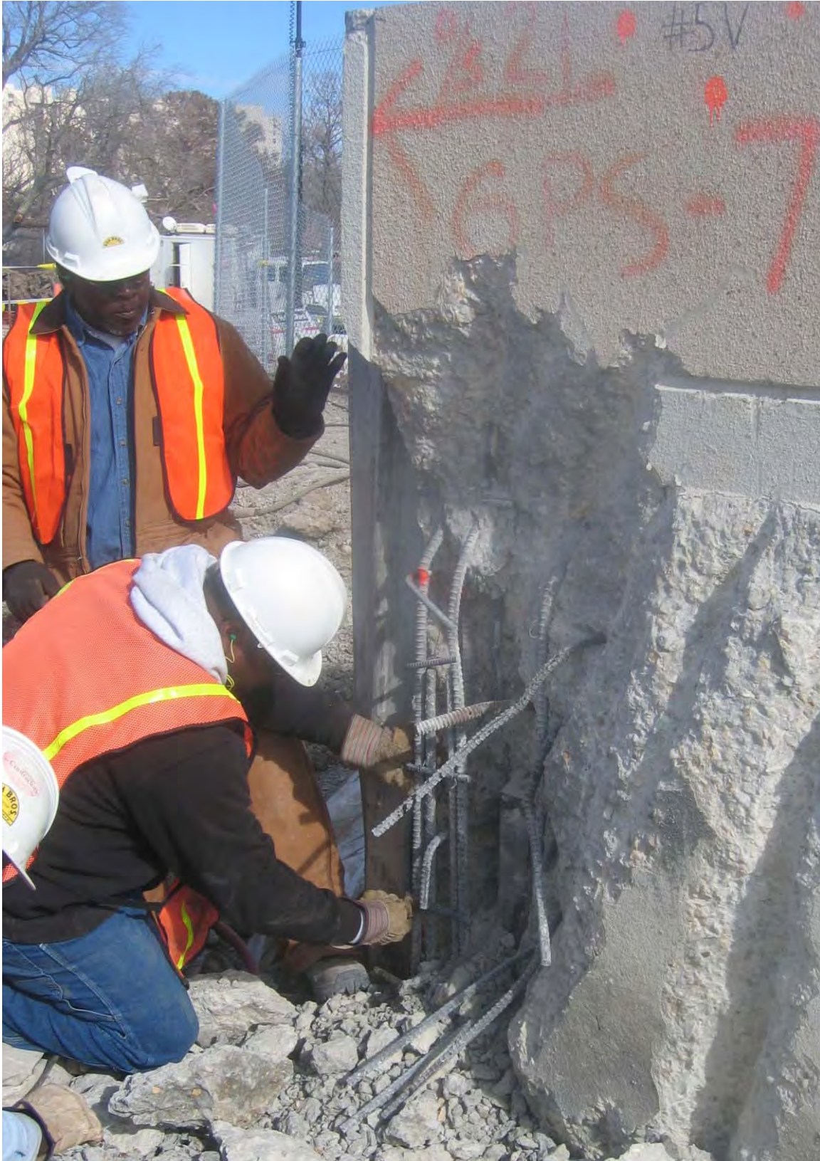
Figure 15-15. Number 6 Rebar Sample Being Taken from Panel H38
