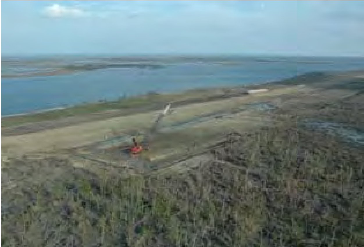
Figure 14-133. Repair Contract Work Borrow Pit and Dragline on Protected Side Right-of-Way
