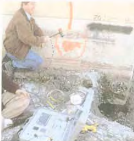
Photo 5 (Fig. 3) - Angled downward impact to chamfer of wall at ~ el. 5.75
