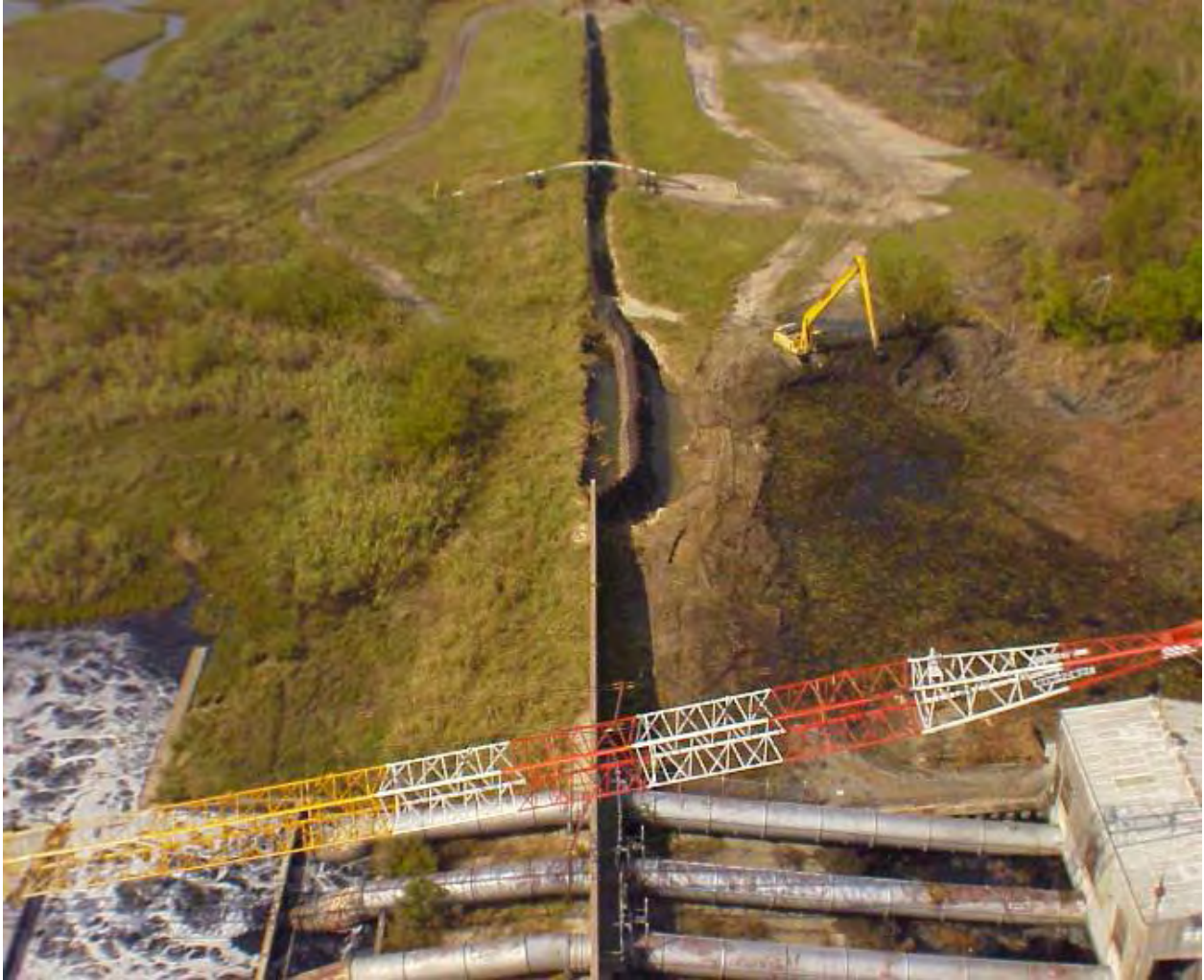
Figure 12-24. NOE2_D View from Above
