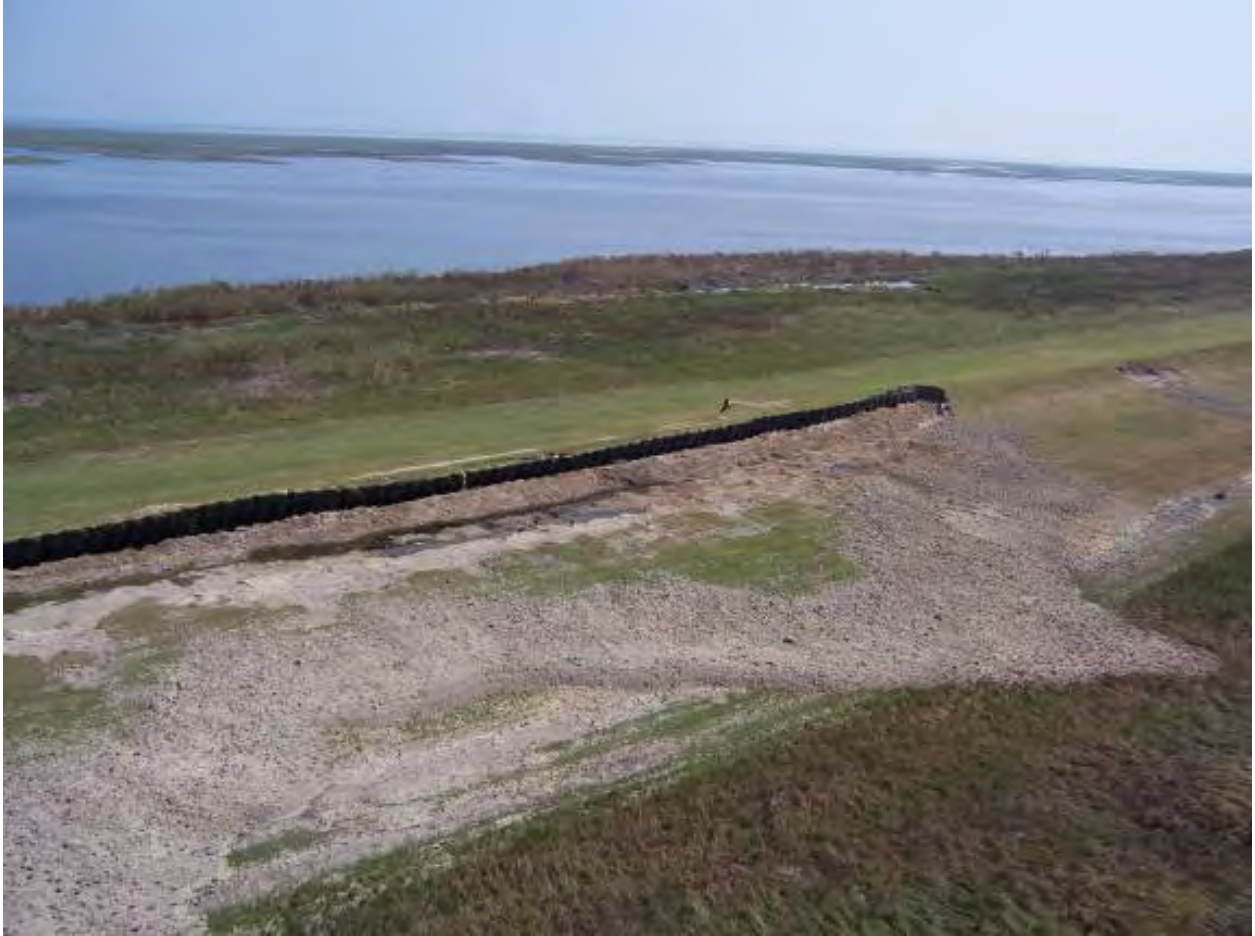
Figure 14-151. End of Sheetpile Wall at B/L Sta 980+58
