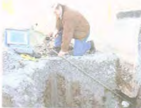
Photo 7 (Fig. 5) - Angled impact to 1 inch diameter, 6 ft long steel rod held at an angle on sheet pile side at 0.5 ft below concrete - protected levee side
