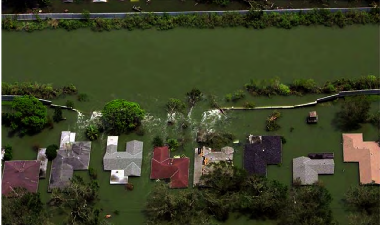
Figure 8-2. The North Breach at the London Avenue Canal Occurred at 7:00 AM to 8:00 AM on August 29, 2005. The breach, on the west side of the canal, is approximately 410 feet wide.
