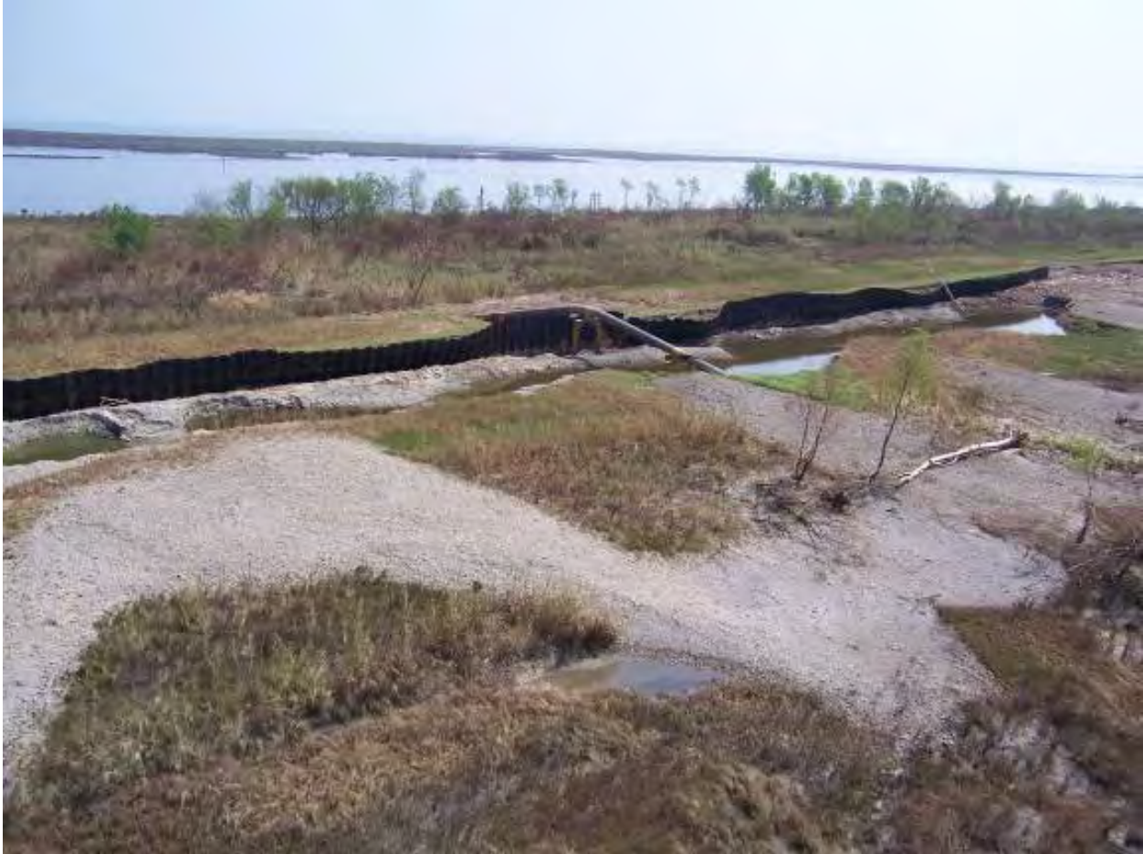
Figure 13-29. Sheetpile Reach Along the MRGO Southeast of Bayou Bienvenue at Approximate B/L Sta 600+00. Top of sheetpile was elevation 17 ft (MSL) and levee crown elevation was approximately 12 ft (MSL), for an exposed sheetpile height of approximately 5 ft. Storm surge on the MRGO was approximately 18 ft, resulting in approximate overtopping velocity of 20 ft per second with approximate 250 lbs/ft impact force. The end of the sheetpile section with transition to the severely eroded levee is approximate B/L Sta 604+15
