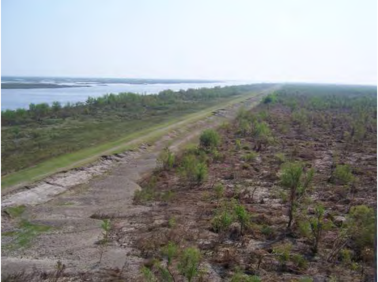
Figure 14-146. Scour on Landside (Protected Side) of Levee
