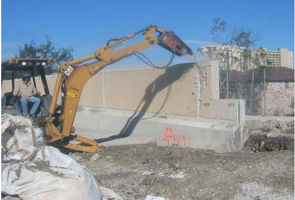
Figure 15-12. Demolition of Concrete for Rebar Sampling at Panel H22
