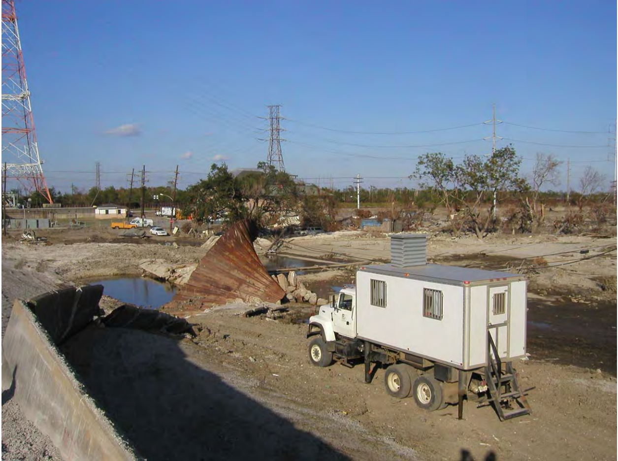
Figure 14-31. CPT Truck at Levee Toe on Protected Side at the Southernmost I-Wall Failure Transition Between Florida Ave and Claiborne Ave., View Toward Pump Station
