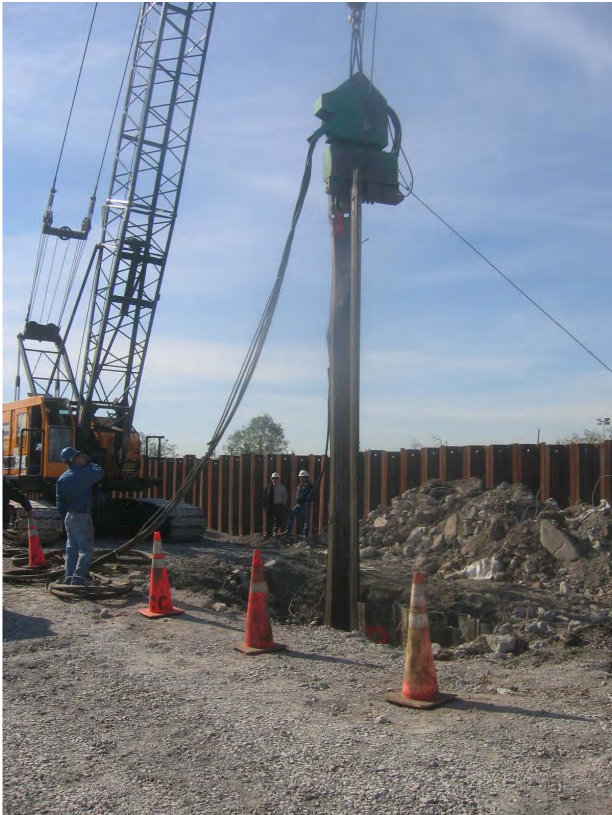
Figure 15-23. Extraction of Sheet Piling MH22SP1 and MH22SP2
