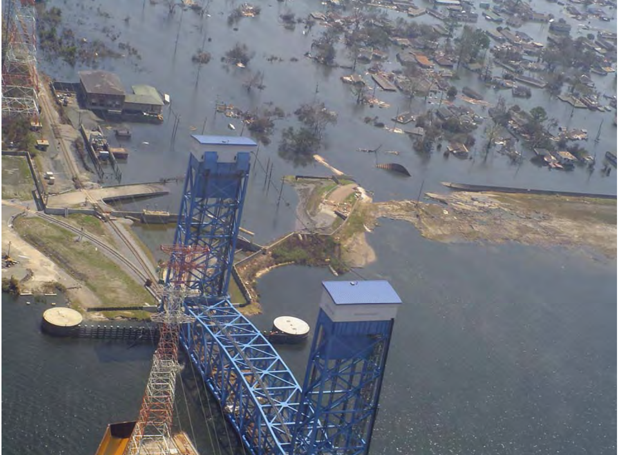
Figure 14-29. Florida Ave Bridge, View East. I-Wall Failure is Seen to Right of Bridge
