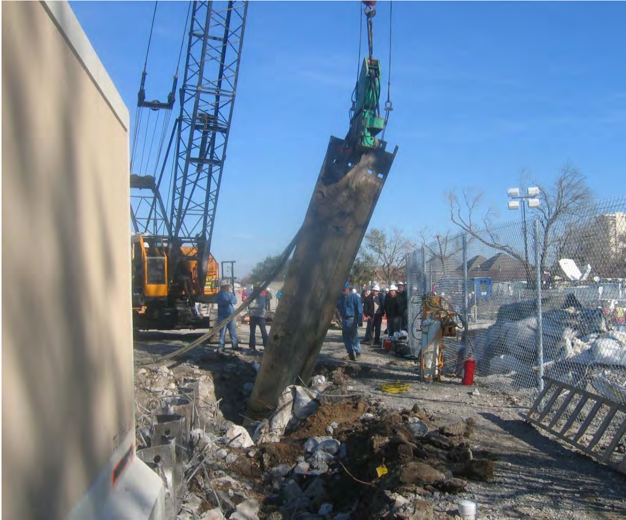
Figure 15-21. Extraction of Sheet Piles MH37SP1 and MH37SP0
