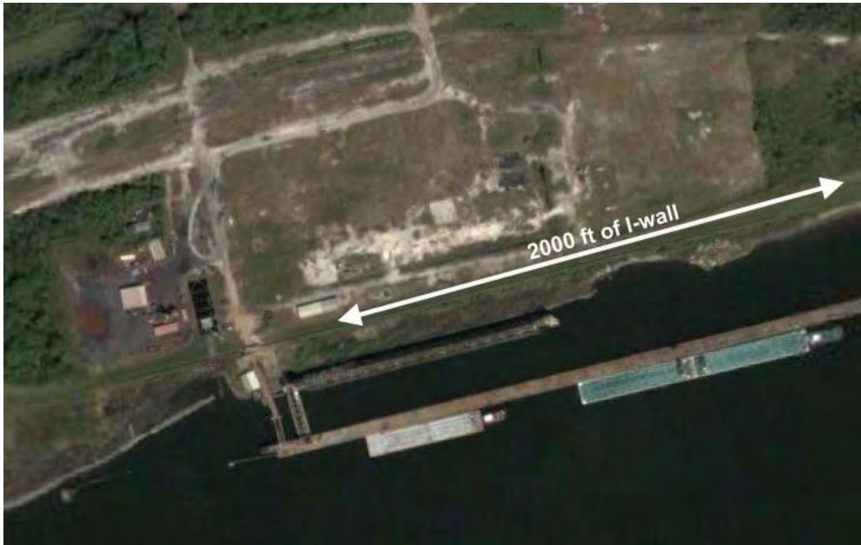
Figure 12-57. NOE4_D. Bulk Loading Facility on the GIWW. Note Tool Shed Metal Building Location
