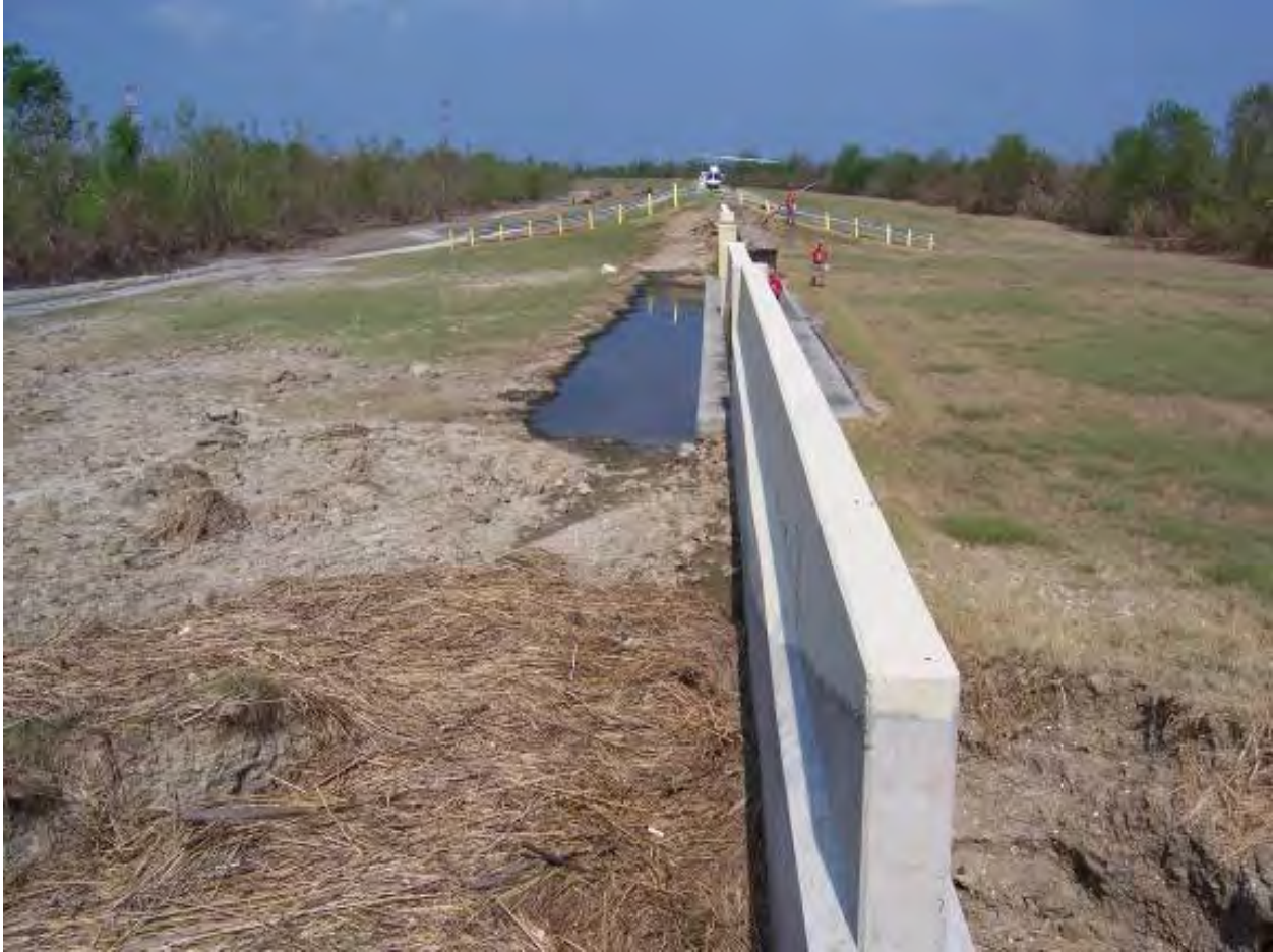
Figure 14-106. View West From Bienvenue Control Structure Toward the Unused Floodgate Structure
