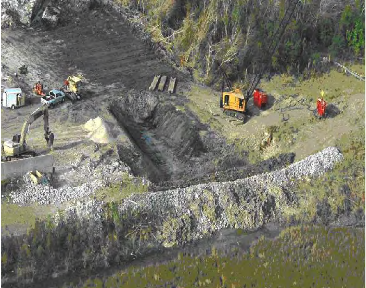
Figure 12-49. NOE3_I. Repair Progress
