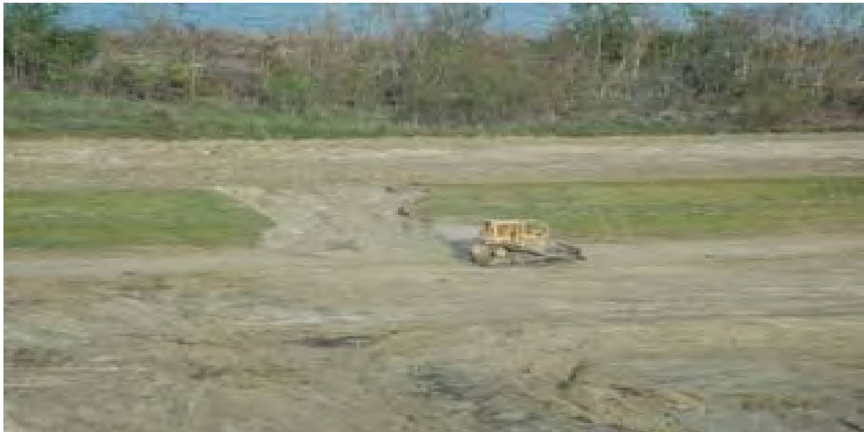
Figure 14-130. Repairs Underway, Filling Scour Holes
