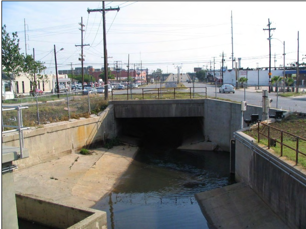
Photo 3. Broad Street Canal Entering Pump Station #1
