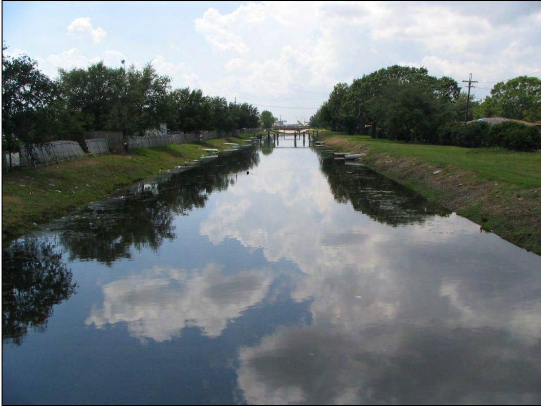
Photo 7. Interior Canal # 3 from Bissonet Dr. near Veterans Blvd.
