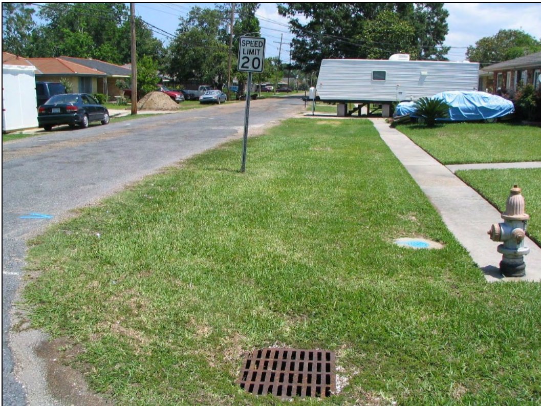
Photos 1, 2, and 3. Typical Streets and Inlet – Jefferson East Bank
