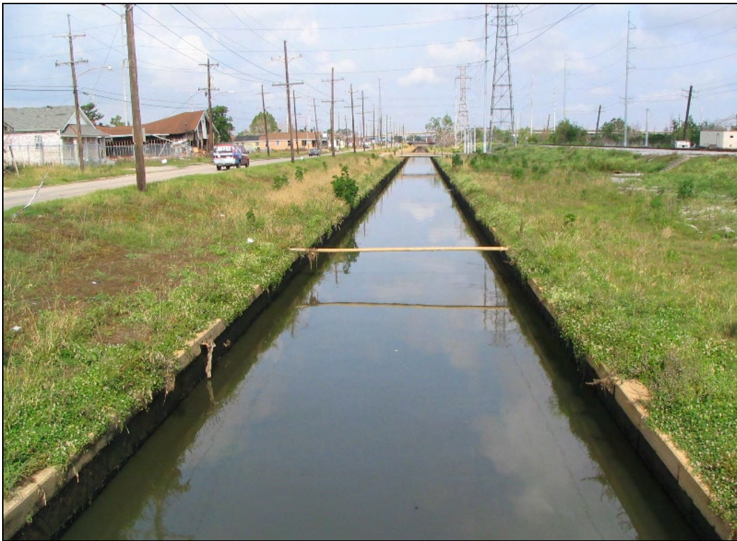
Photo 5. Florida Avenue Canal from Louisa Street
