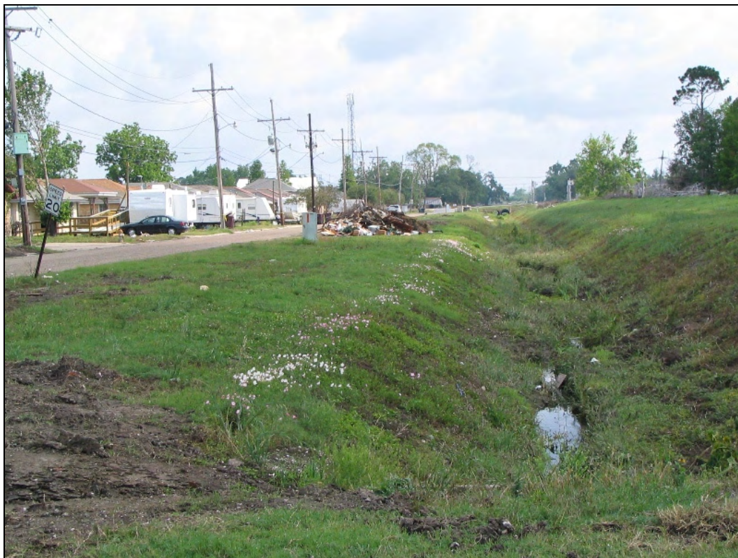
Photo 3. Typical Roadside Ditch Collector
