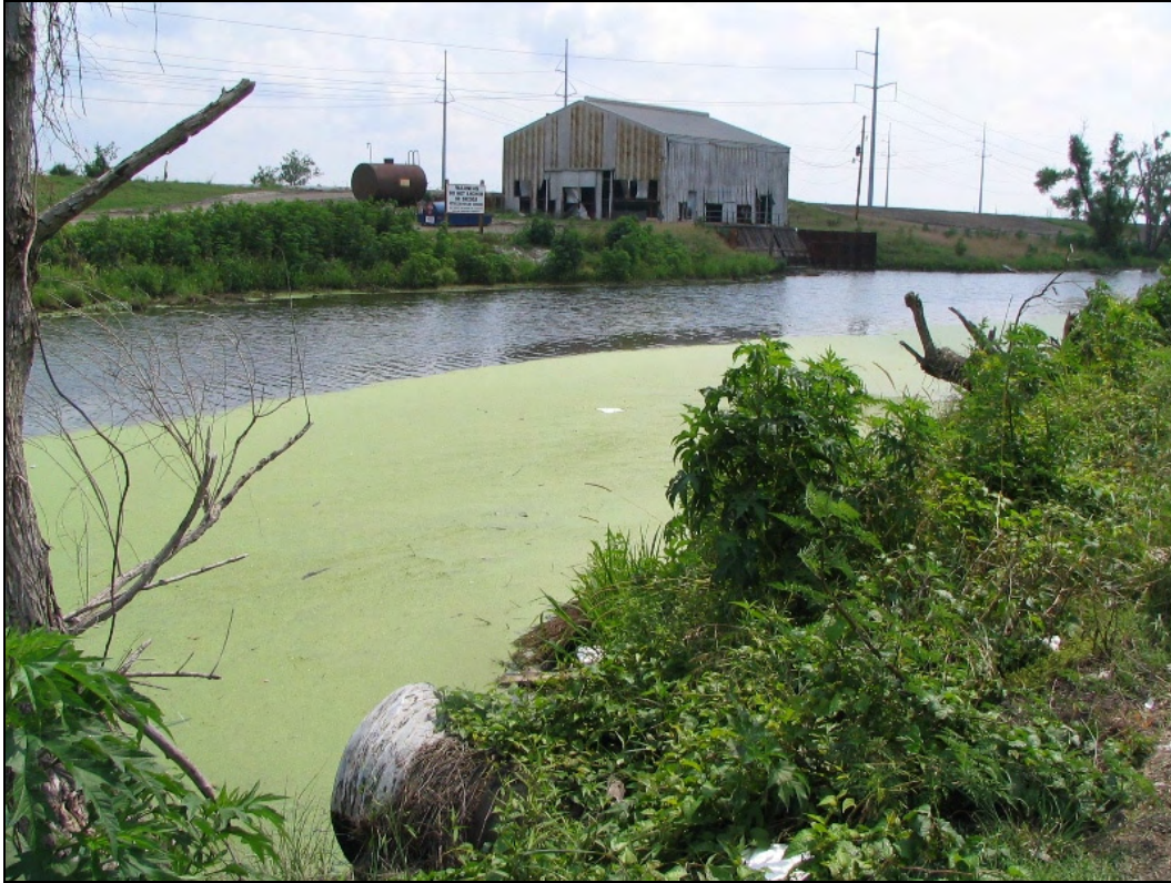
Photo 6. Forty Arpent Canal and at Pump Station #3, Bayou Villere
