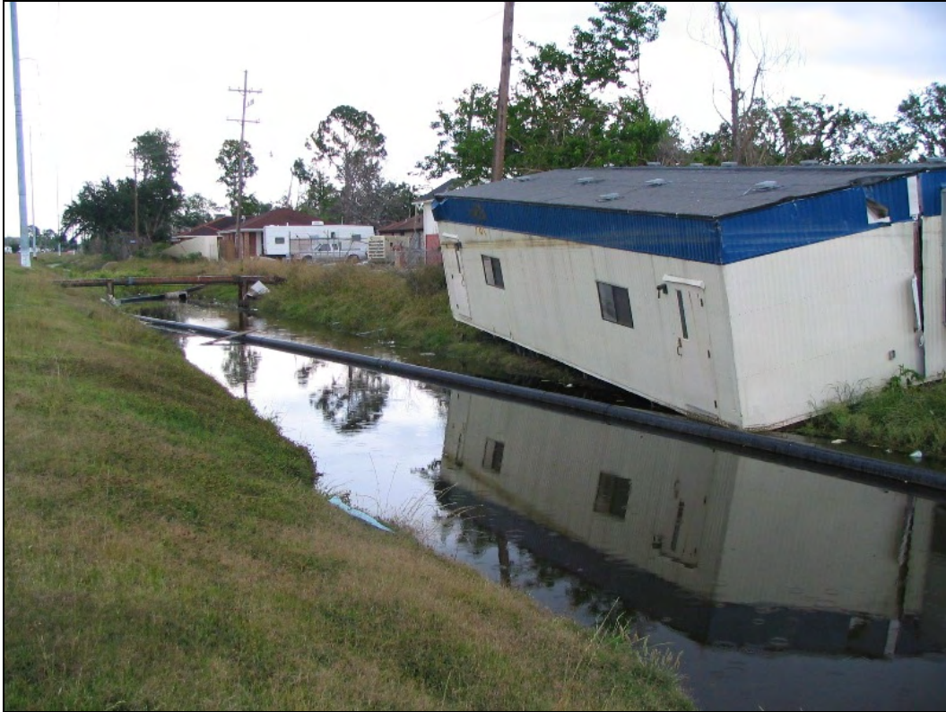
Photo 6. Dwyer Canal near Crowder Blvd.
