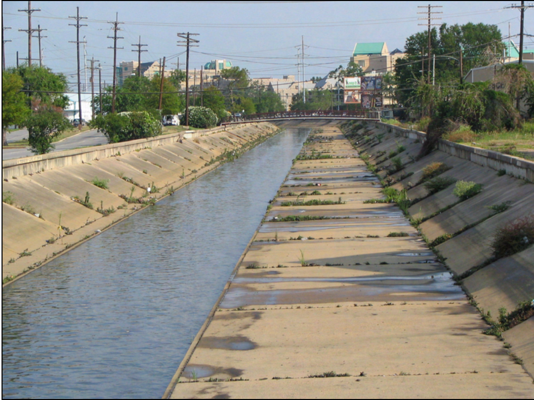
Photo 6. Palmetto Canal from Jefferson Davis Parkway
