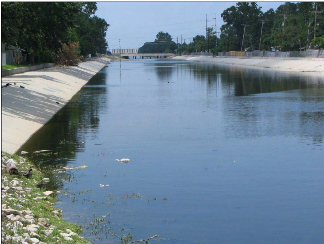
Photo 8. Elmwood Canal (interior) from Kawanee Ave.
