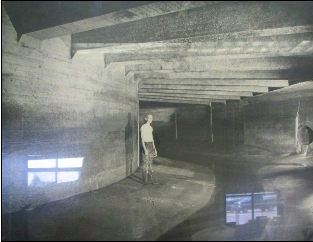
Photo 4. Claiborne Canal after Construction
