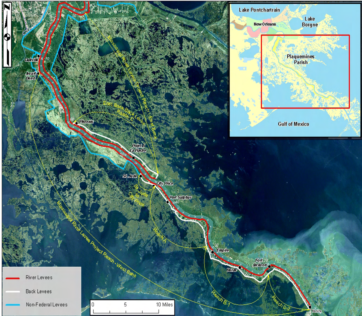
Figure 25. Extent of NOV Hurricane Protection in Plaquemines Parish. The NOV consists of six distinct reaches; Reach C, Reach St. Jude to City Price, Reach A, Reach B1 and Reach B2.
