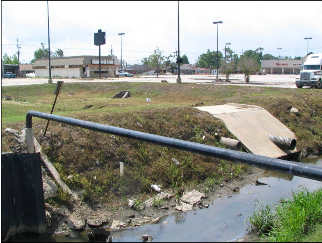
Photo 7. Onsite Detention Basin on Judge Perez Dr.
