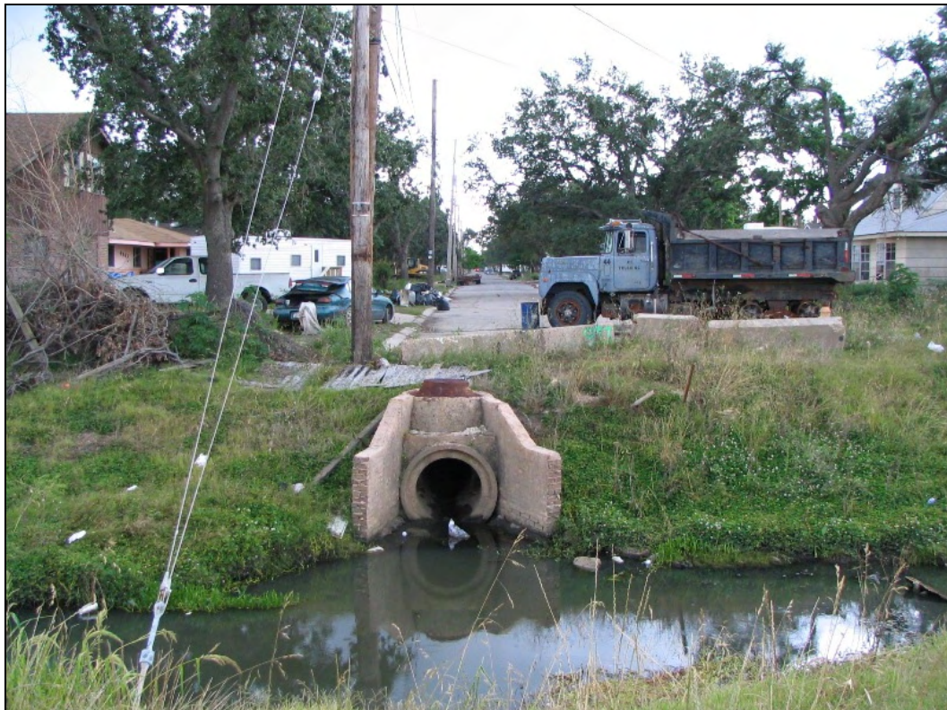
Photo 3. Storm Sewer Outfall into Dwyer Canal
