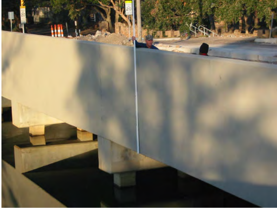
Figure 66. Typical low chord measurement—London Avenue Canal Bridge No 4 (IPET/3001, Inc.)
