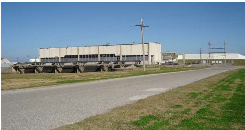
Pump Station JP-04
