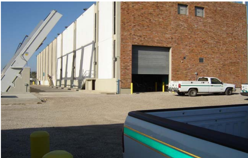
Pump Station JP-02
