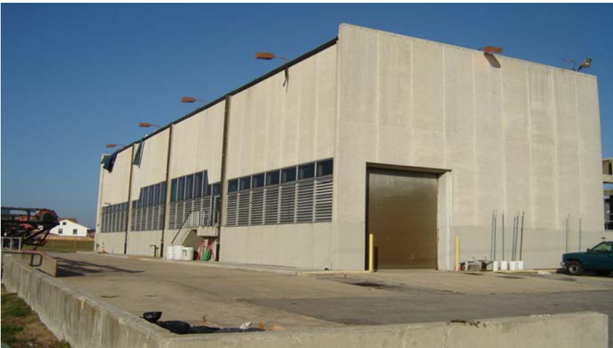
Pump Station JP-01
