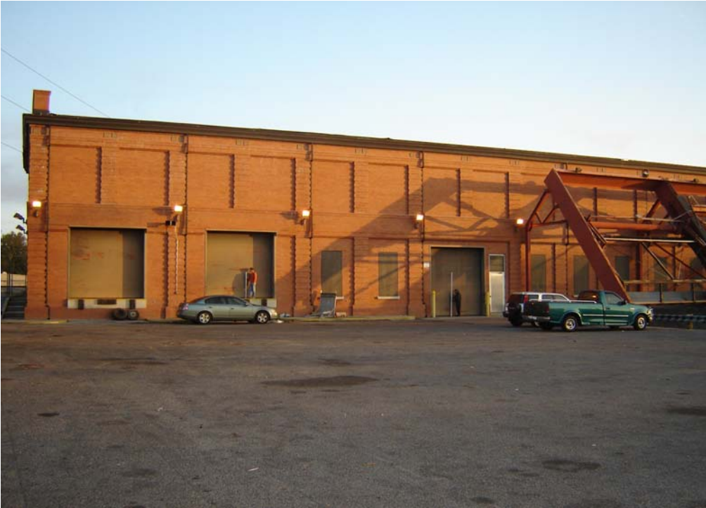
OP-6 Pump Station
