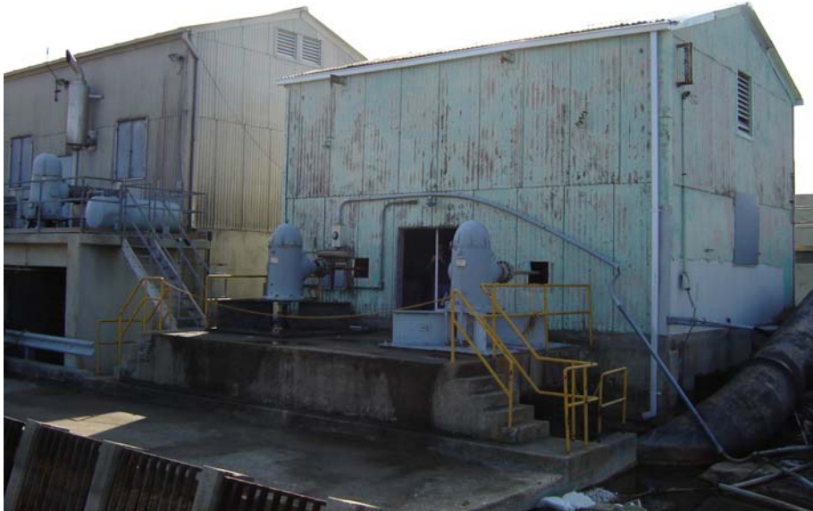
SUNRISE #1 PUMP STATION
