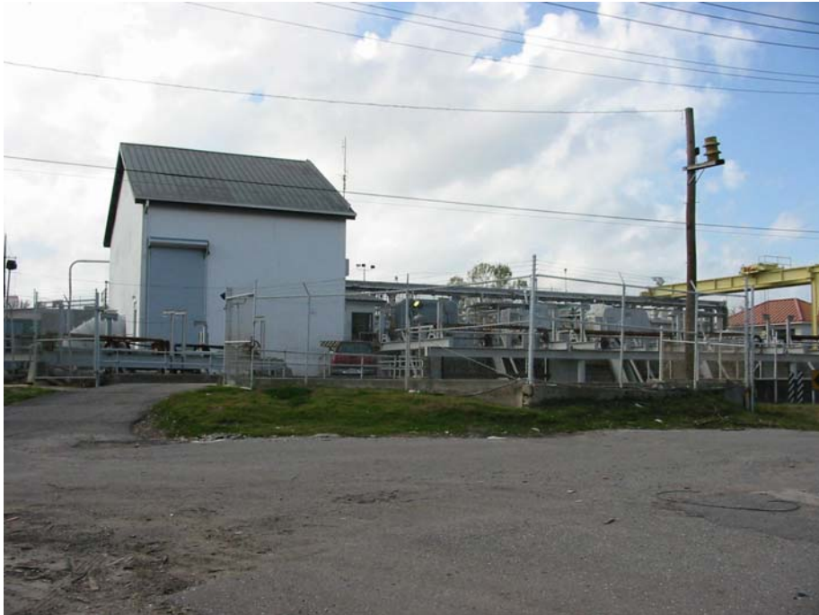
OP #4 PUMP STATION
